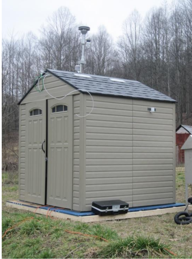
Figure 26. Photograph of equipment shelter at residence.
