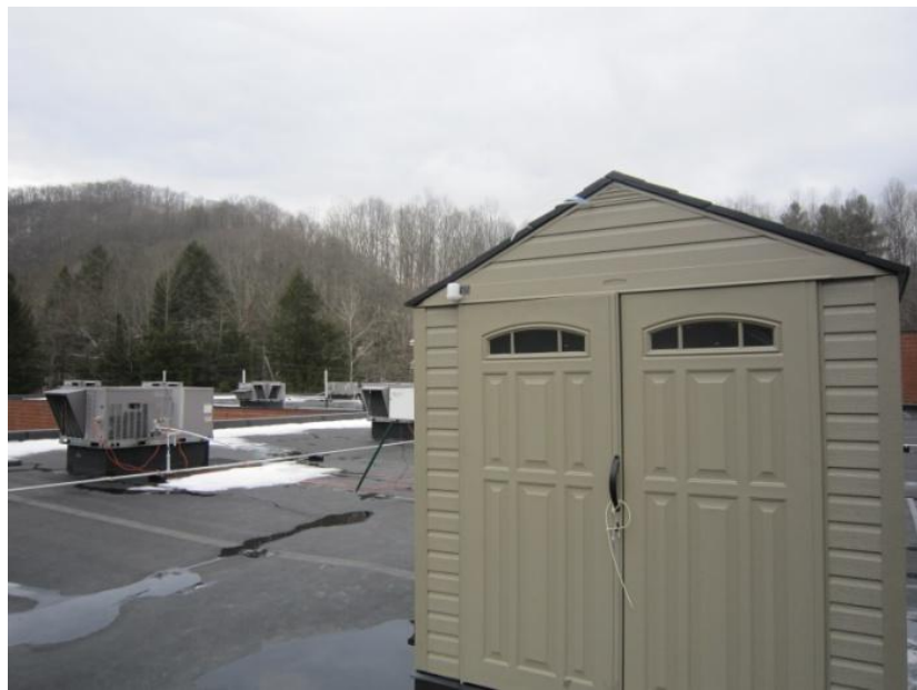
Figure 27. Photograph of equipment shelter at school.
