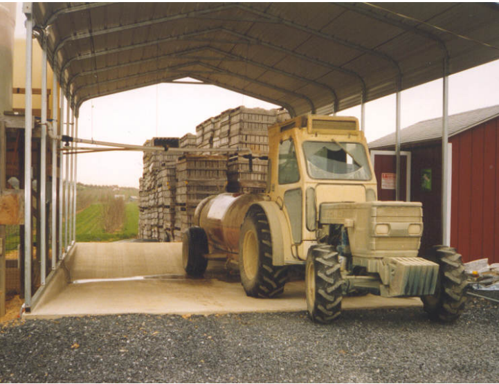
PESTICIDE HANDLING AND CONTAINMENT FACILITY IN A COMMERCIAL ORCHARD, BERKELEY COUNTY
