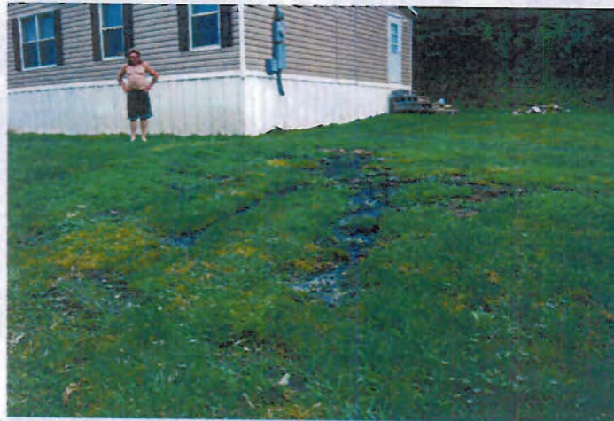
Septic waste from failing tank comes up in yard where the project later installed a new system
