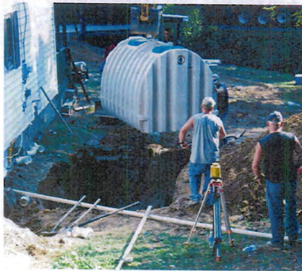
Installing new septic tank
