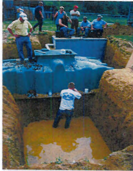
Peat module installation
