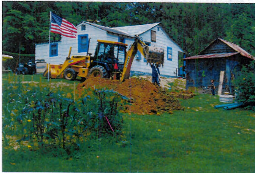
Beginning installation at home on Flat Creek
