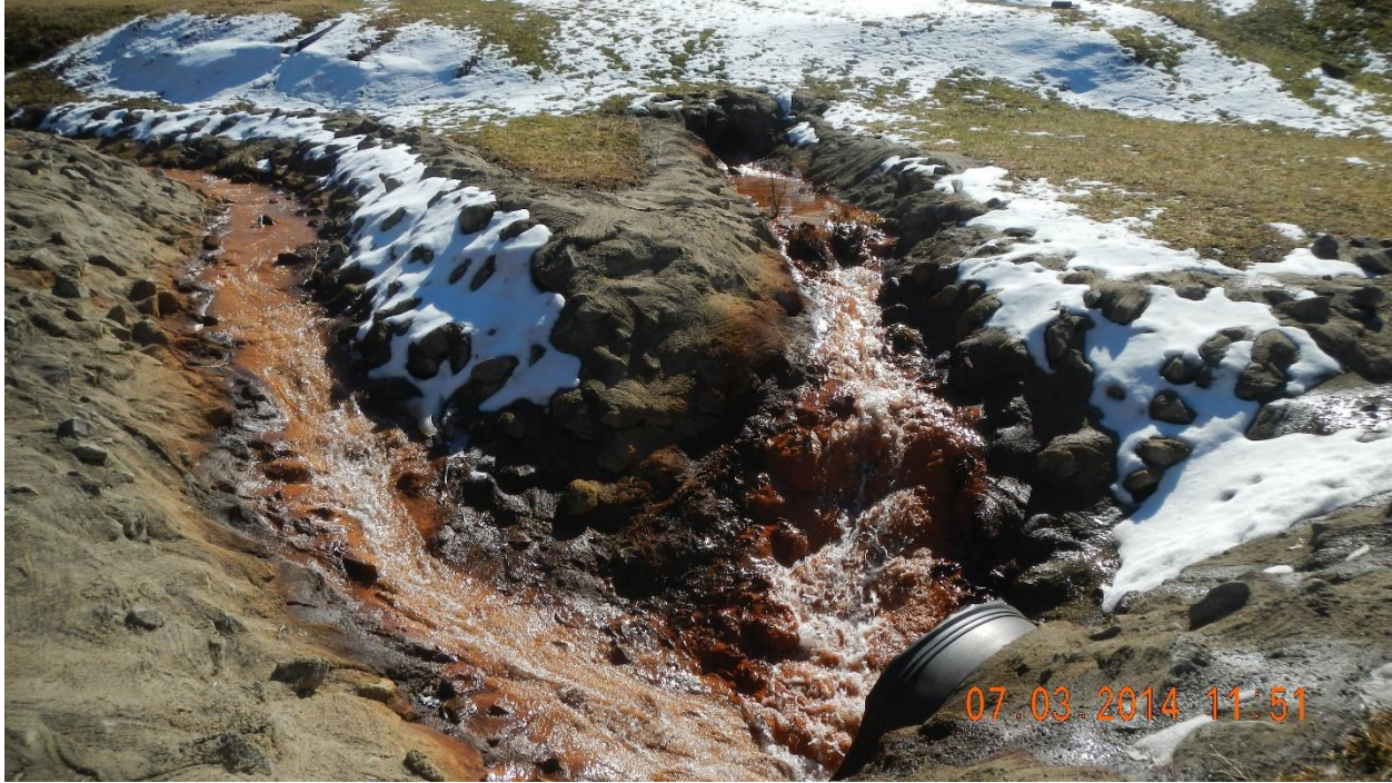
Figure 15: Wet seals with mine drainage flowing on grouted channel at the Robey Mine sample site.
