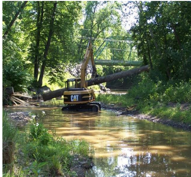
Contractor's work along Sleepy Creek, Morgan County
