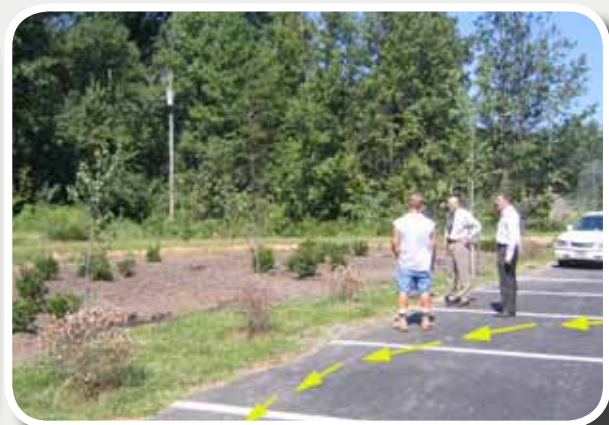
Some site runoff by-passes bioretention because of inadequate slope of filter strip.
