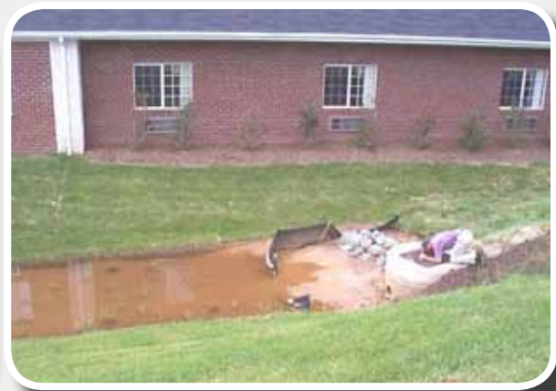
Bioretention area does not drain because of improper soil media, soils compacted during installation, and/or filter fabric under media
