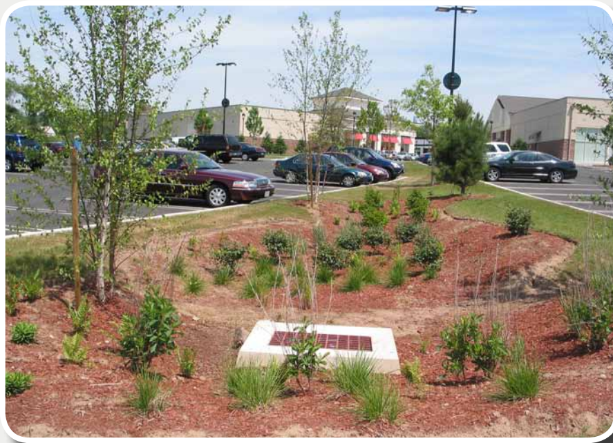
Figure 2.3 Parking lot runoff directed into a bioretention facility reduces thermal impacts (Source: National Nonpoint Education for Municipal Officials Network)
