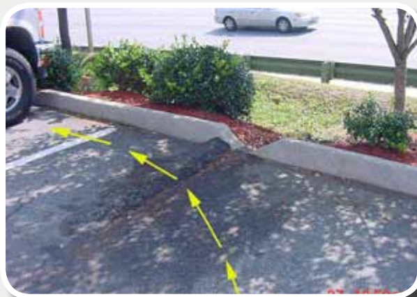
Site runoff by-passes bioretention swale because of small elevation changes during construction.
