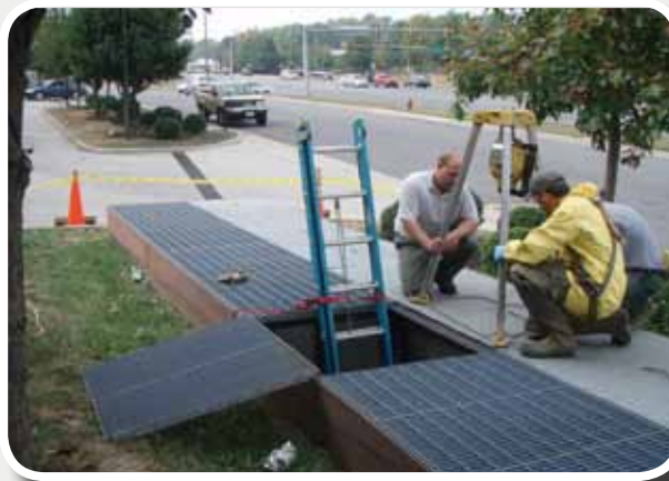
Underground Sand Filter
