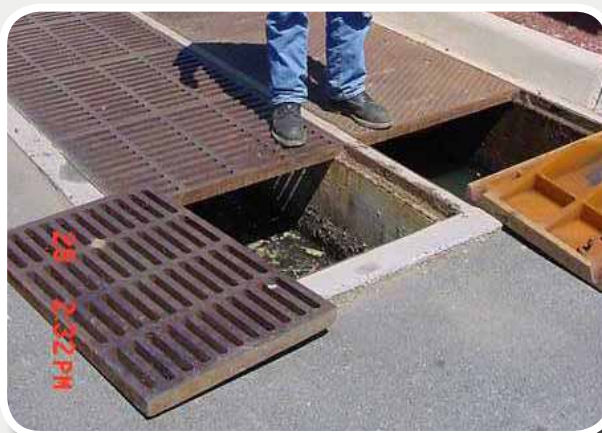
Perimeter Sand Filter
