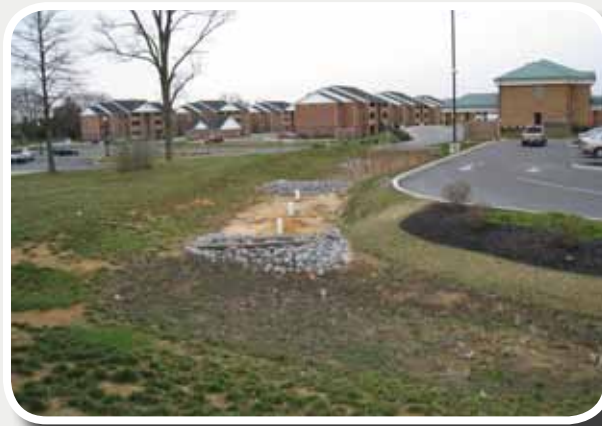
Surface Sand Filter
