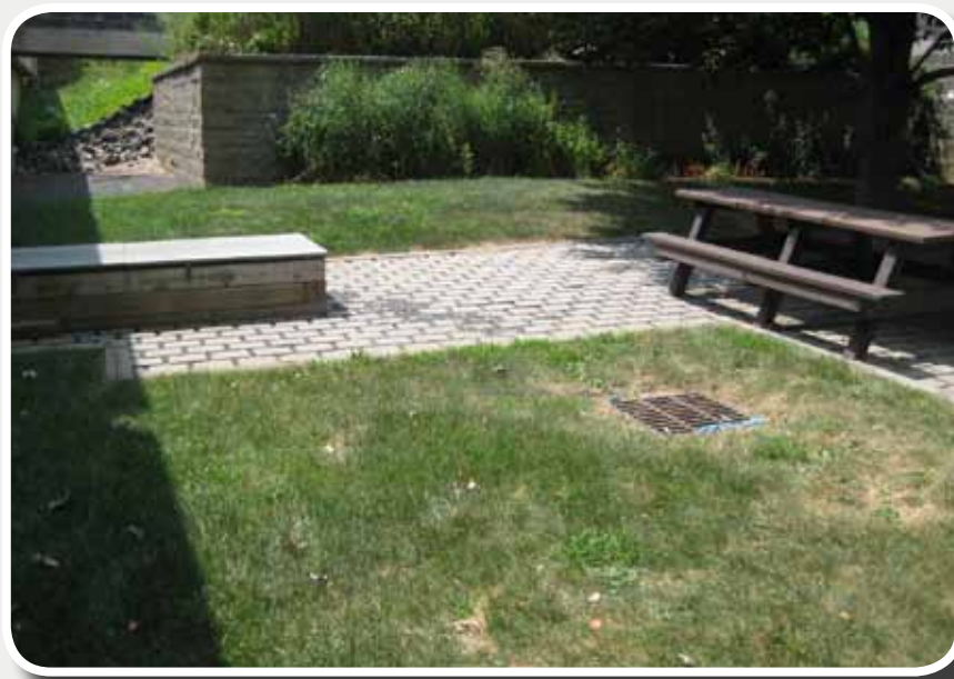
Figure IN-8. Example of an Infiltration Trench with Surface Cover
