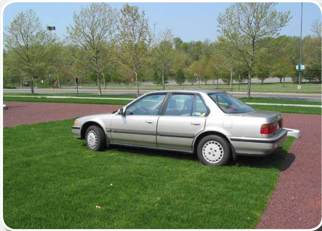
Figure 2.1. Pervious pavers used for overflow parking (Source: National Nonpoint Education for Municipal Officials Network)
