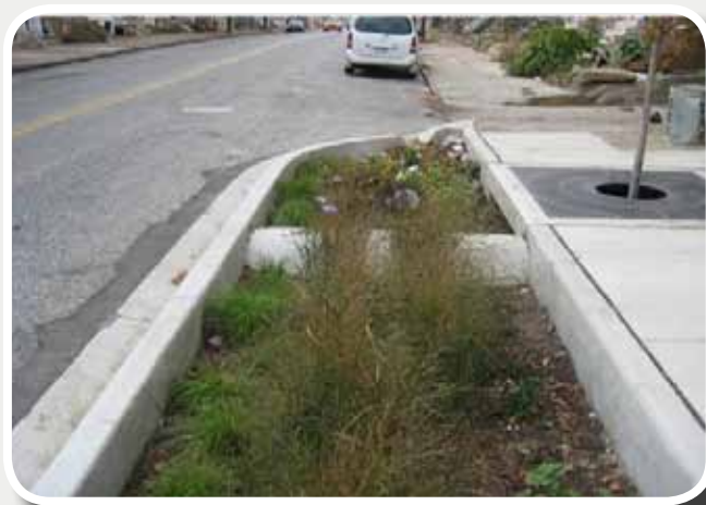
Street Bioretention – curb extension linked with tree box
