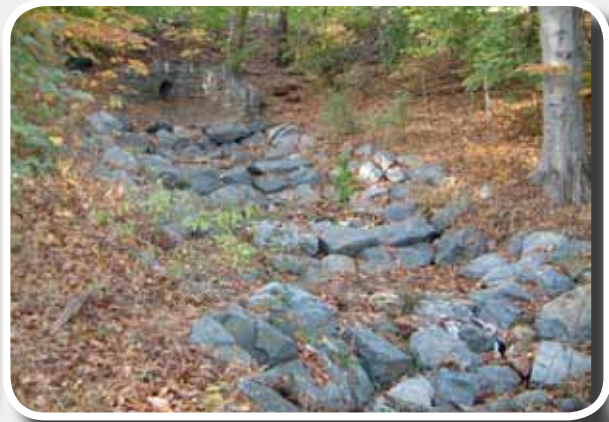
Before (Left): Eroded outfall. After (Right): Outfall restored using RSC design.
