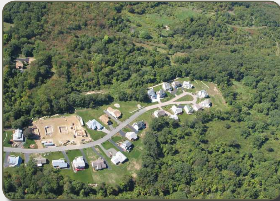
Figure 2.6. During construction of this subdivision, clearing was limited to the minimum area necessary, protecting native soils (Source: National Nonpoint Education for Municipal Officials Network)
