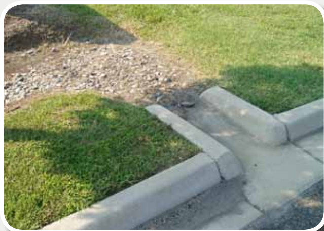
Figure IN-7. Examples of pretreatment forebay (left) and sand filter cell (right)
