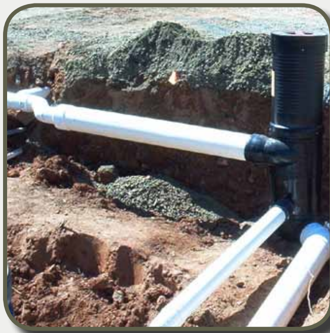
Figure RH-14. Installation of Vortex Filter prior to backfill. (Source: Rainwater Management Solutions)
