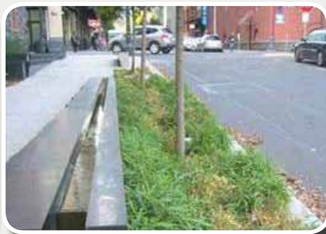
Extended tree pits within right-of-way
