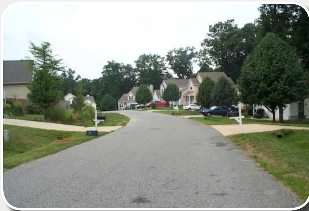
Figure BSD-2. Reduced Street Width
