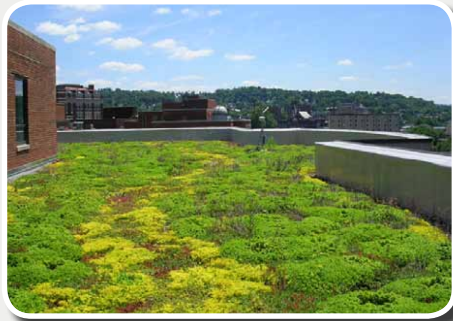
Extensive Vegetated Roof (Source: WVDEP)
