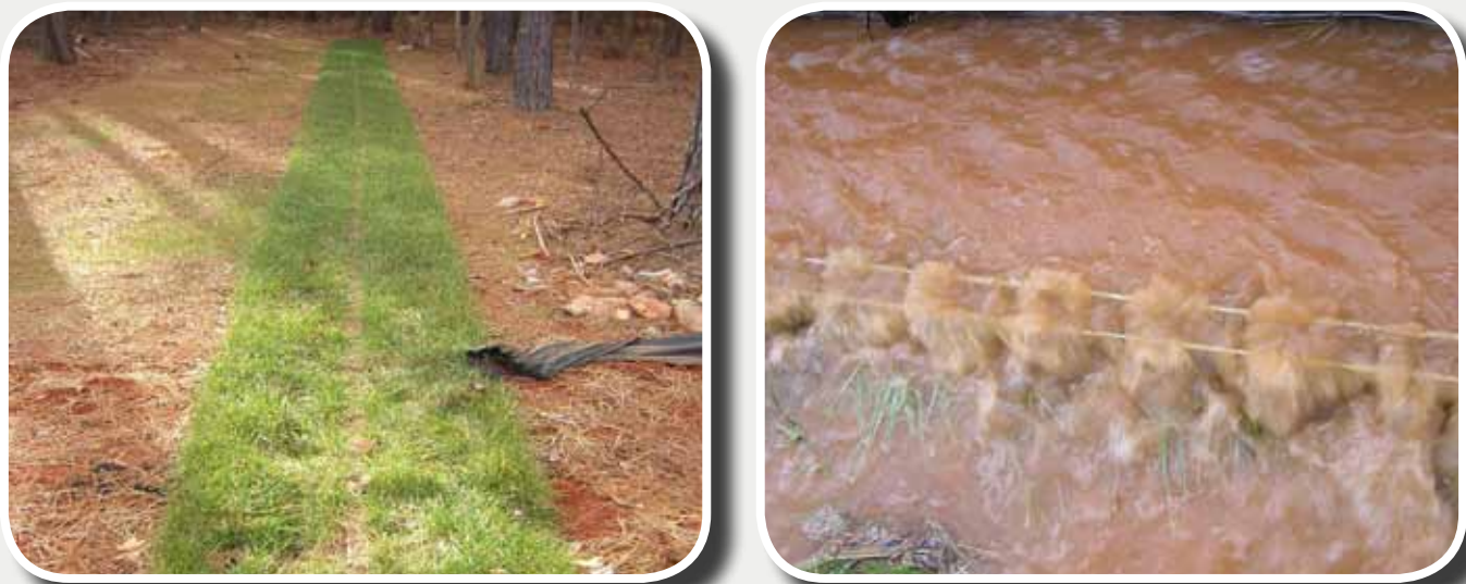
Figure SF-8. Image of Slotted Trench Drain Level Spreader into Conservation Area (Source: CONTECH Construction Products, Inc.)
