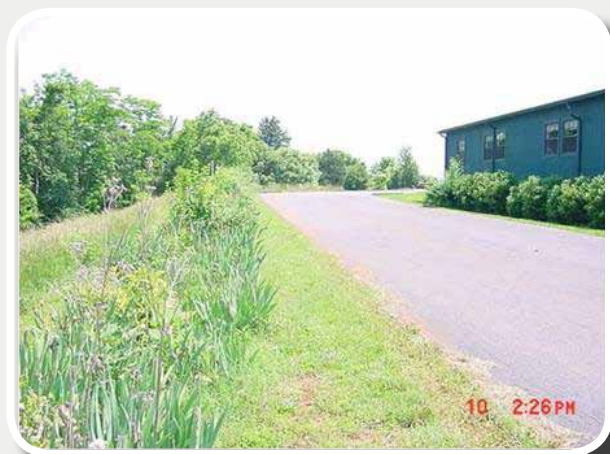
Sheet Flow from small impervious area to Vegetated Filter Strip
