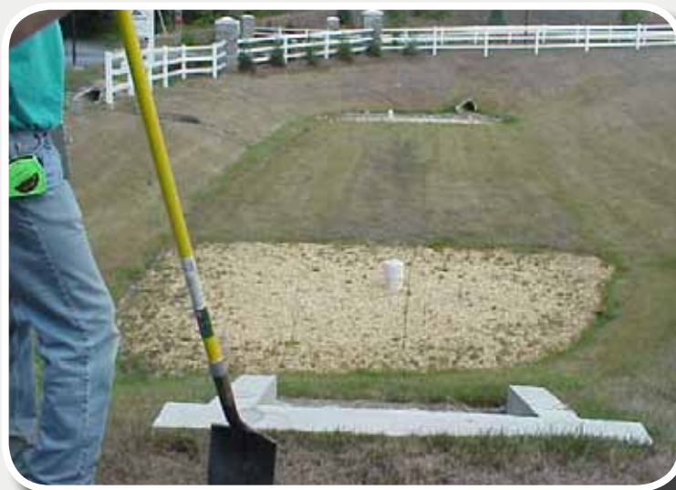
Figure FP-8. Gravel forebay and top soil and turf cover over the sand media (Source: Chesapeake Stormwater Network)
