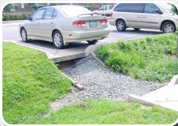
Curb inlets to bioretention swale have eroded because of improper sizing of stone.
