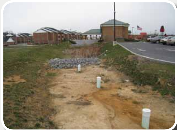
Figure IN-7. Examples of pretreatment forebay (left) and sand filter cell (right)
