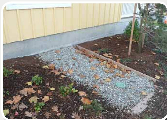
To Treat Roof Runoff or Other Small Areas of Impervious Cover (Micro-Scale)
