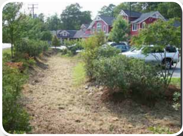
Figure FP-6. Examples of Pre-Treatment Applicable to Filtration Practices
