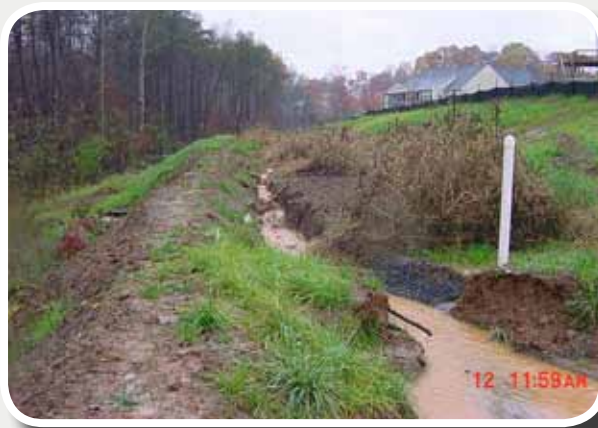
Bioretention swale, installed too early during active construction, has become clogged with sediment.
