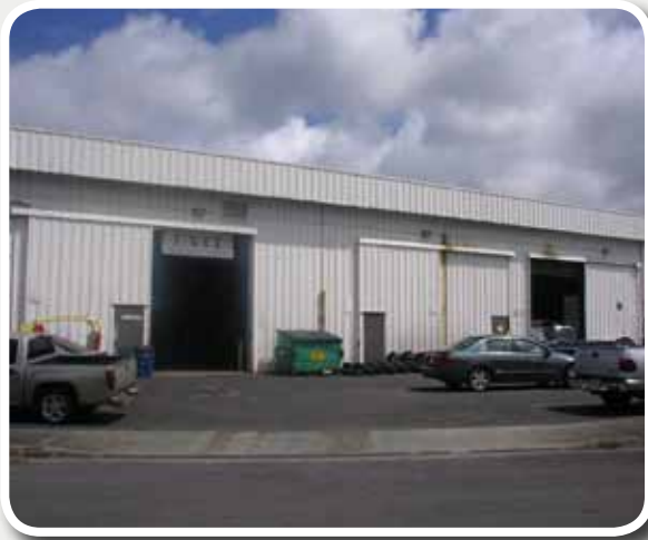
Vehicle Maintenance Facilities
