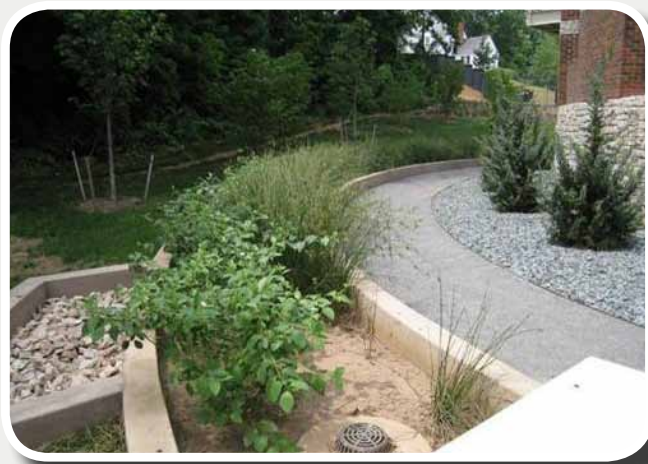
Adjacent to building to catch roof runoff
