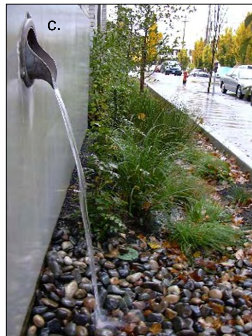
Figure 3: Runoff from larger rooftops can be treated in cisterns (a), infiltration areas (b), or bioretention planting beds (c).
