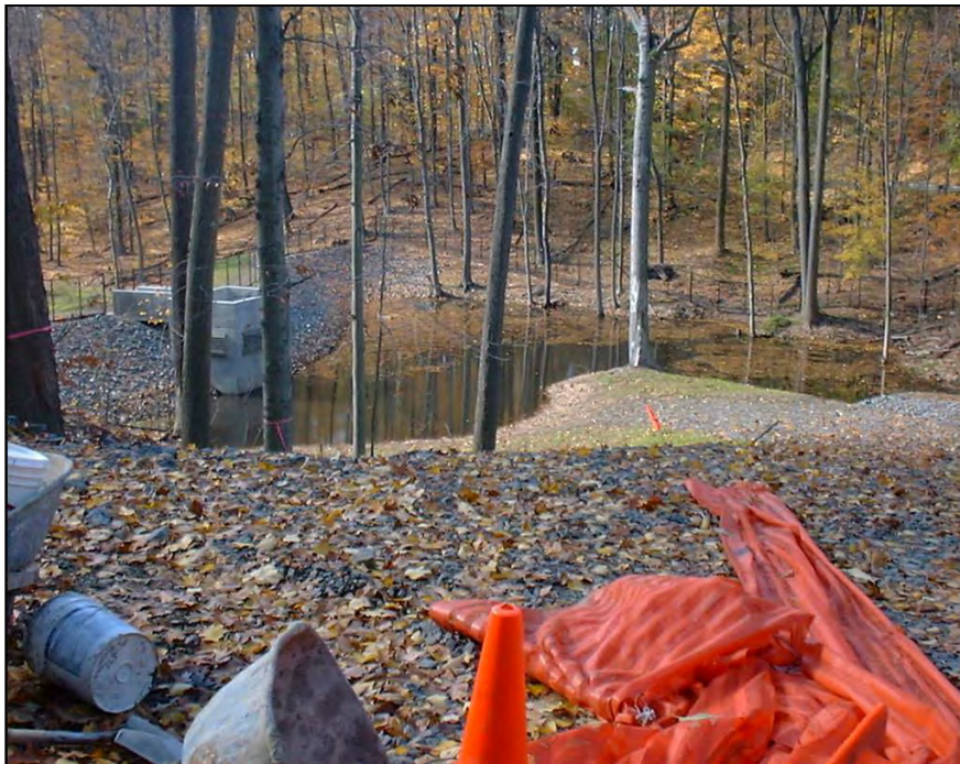
Figure 11: Construction access and staging is always a challenge for crossing retrofits
