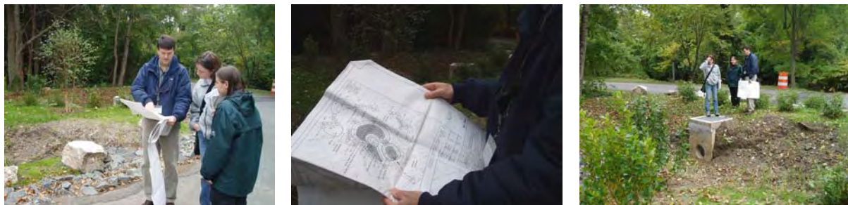
Figure 4.7: While comparing an existing stormwater treatment practice to the original plans, the retrofit team realizes that the trash rack was never installed.
