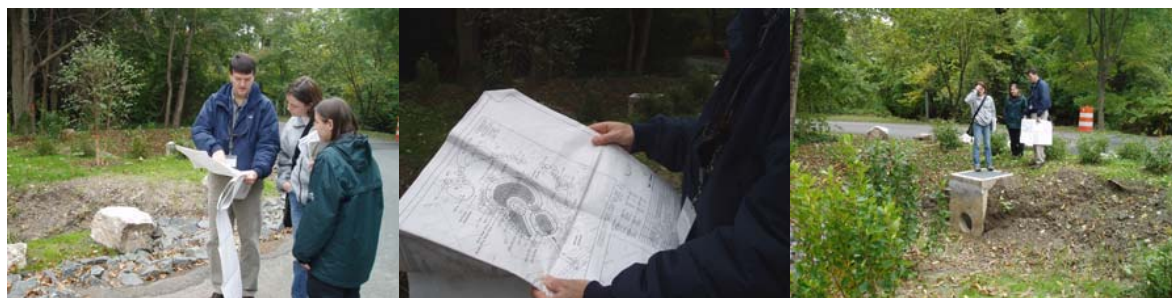
Figure 2. While comparing an existing STP to the original plans, the field team realized the trash rack was never installed.
