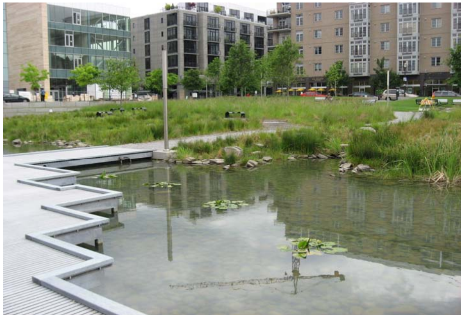
Tanner Springs Park in Portland, Oregon includes a constructed wetland for managing runoff from nearby buildings
