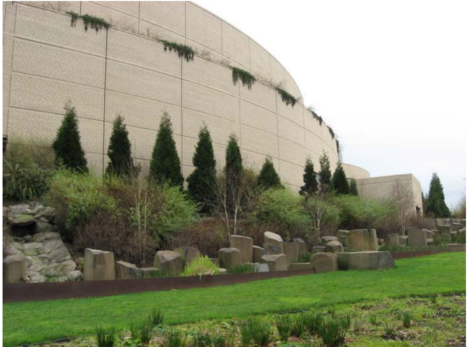
The Oregon Convention Center saves $15,600 annually on its stormwater bill by managing roof runoff in rain gardens along the side of the building.
