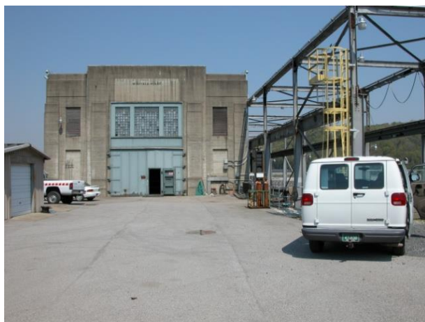
Figure 11-9. Photo of the Winfield Locks & Dam.
