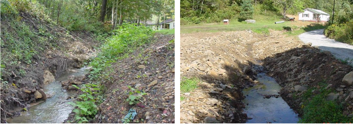
Figure 2-41. Examples of poor bank vegetative protection.
