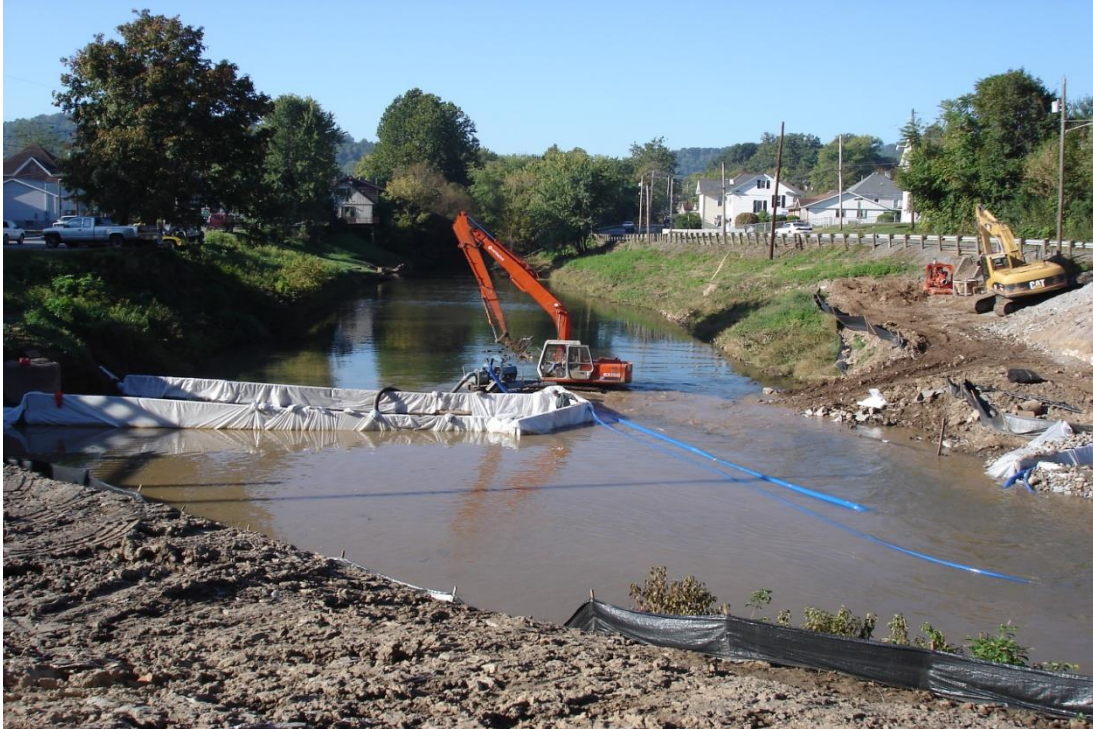
Figure 2-33. Example of Channel Alteration actively occurring due to an installation of sewage pipes across a stream channel.
