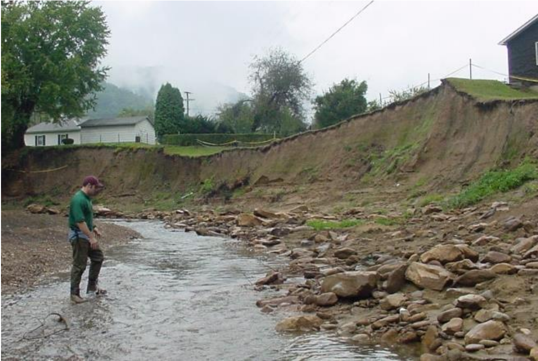
Figure 2-40. Example of heavy erosion (photo right).
