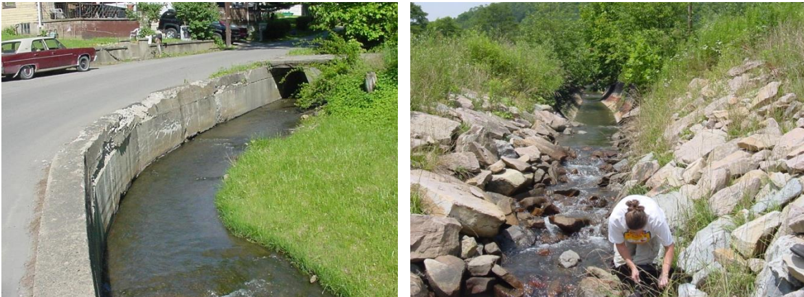
Figure 2-32. Examples of varying degrees of Channel Alteration (concrete channel on left and rip/rap channel on right).
