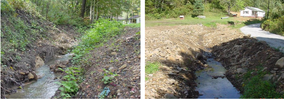
Figure 2-41. Examples of poor bank vegetative protection.
