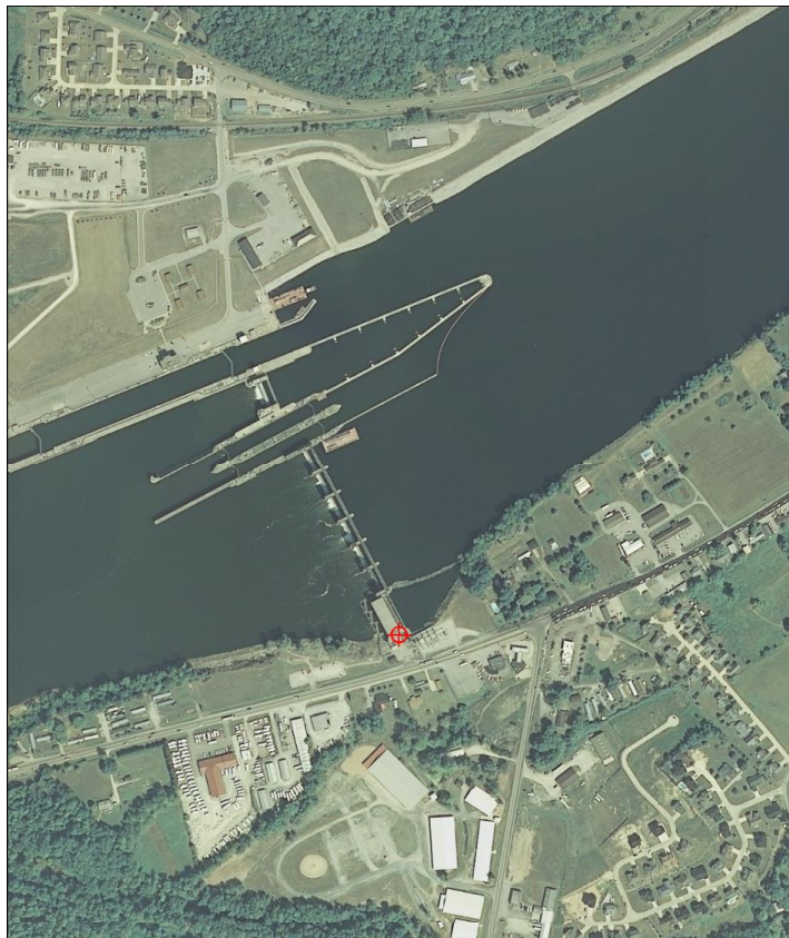
Figure 11-9. 2003 Aerial Photo of the K-(31.7) Kanawha River Ambient Sample Site at Winfield Locks & Dam, WV.
