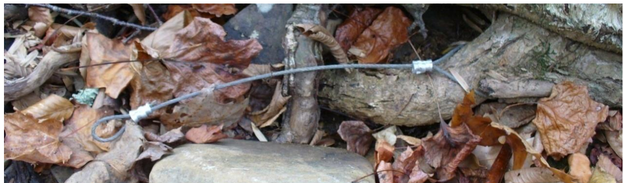
Figure 13-10. Picture of semi-permanent anchor of fixed length in field.
