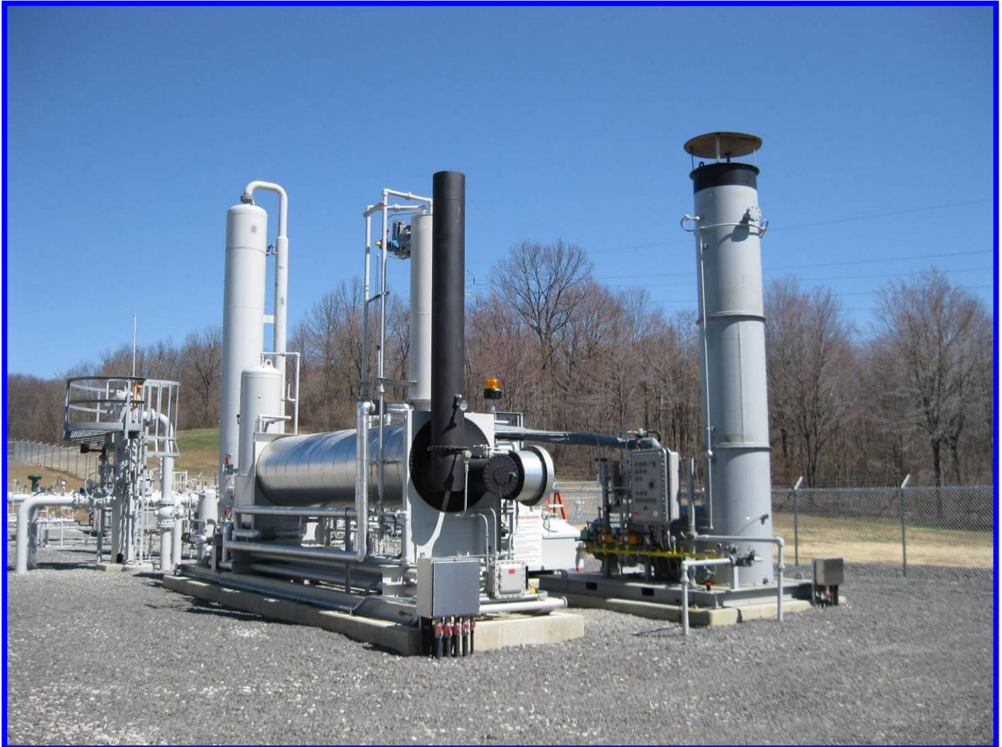
Typical Regenerator, Contactor, and Thermal Oxidizer, provided by Frederick Logan Company, Inc.
