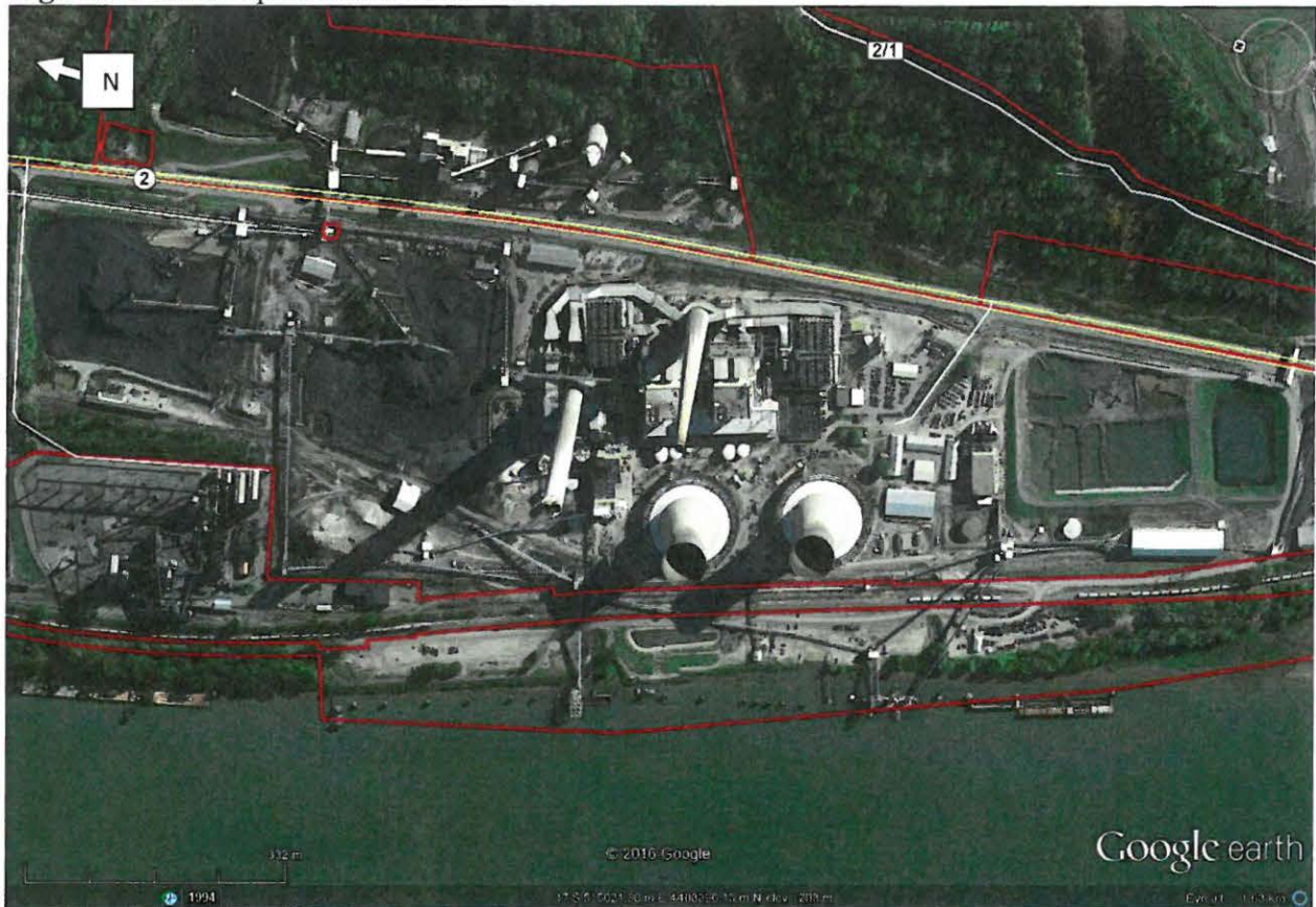
Figure 2. Close-up of Mitchell Plant.
