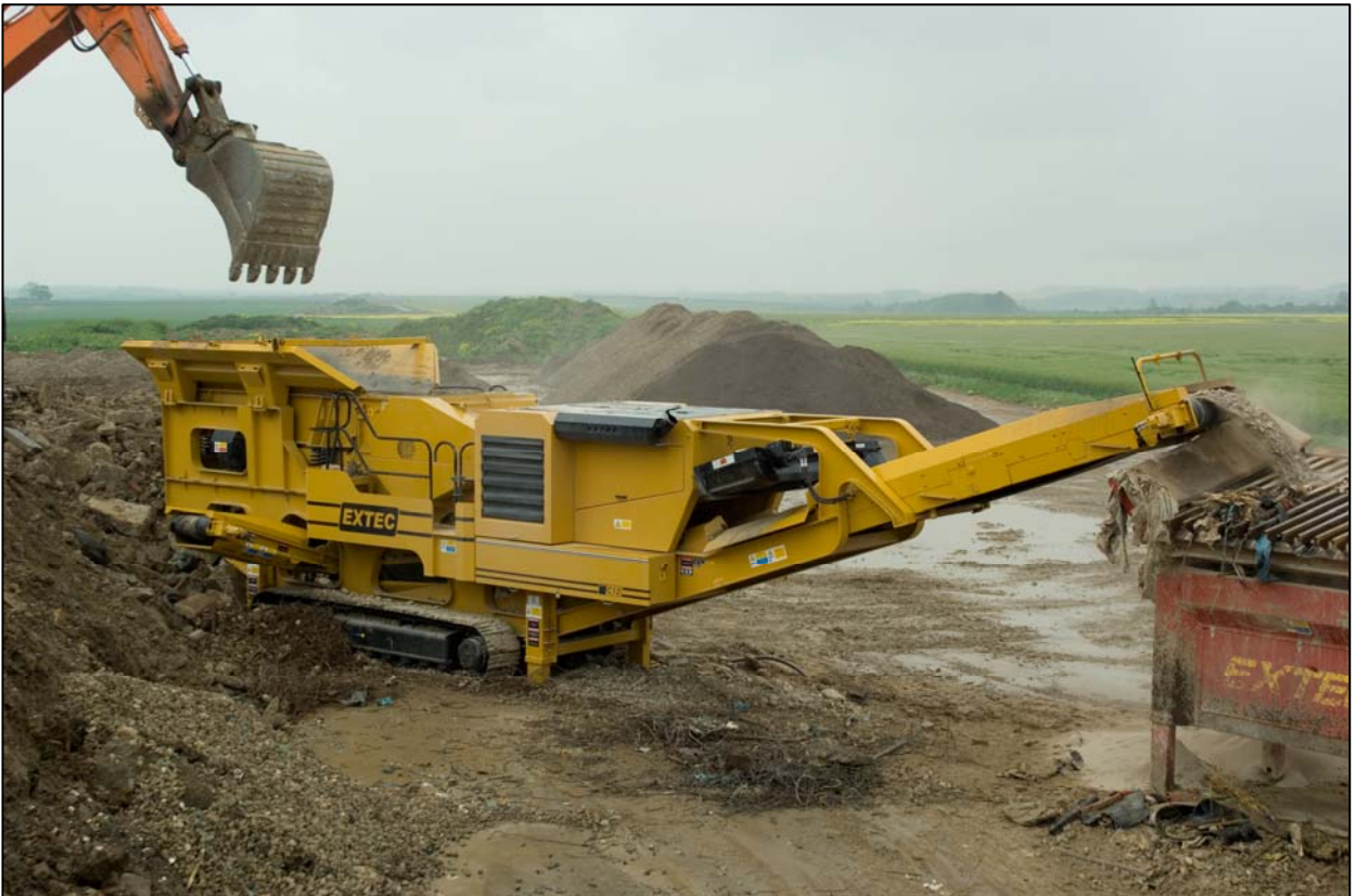
Waste recycling application
