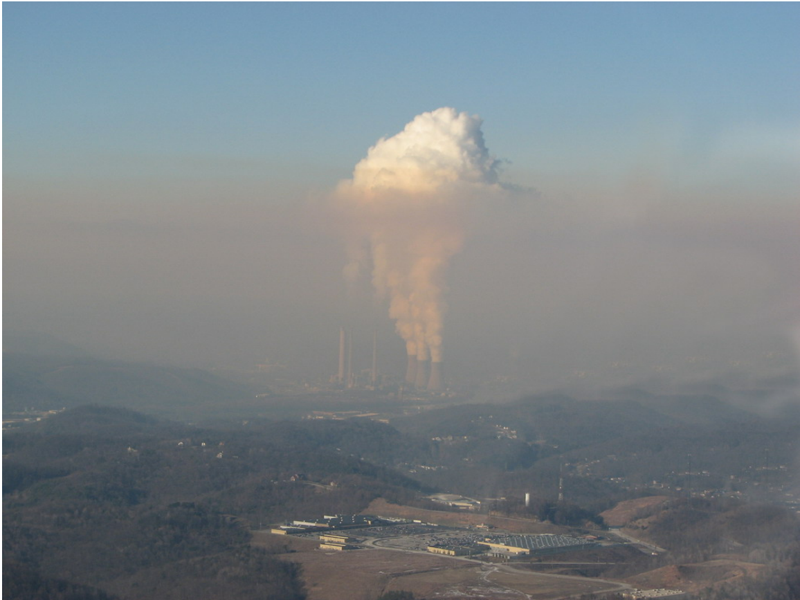
Photograph ES-1. Looking north from above Institute. Note the Cross Lanes Wal-Mart in the foreground. Note also: The active boiler exhaust stacks—the most slender ones of the taller stacks shown—are approximately 900 feet tall. That would indicate that the inversion layer above the plant was approximately 2,500-3,000 feet above the Kanawha Valley floor.
