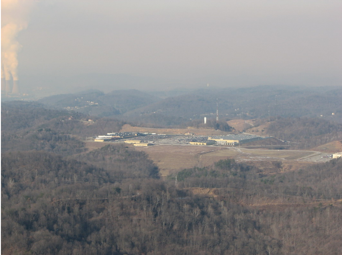
Photograph 3-4. Looking north from above Institute. Note the Cross Lanes Wal-Mart at the photograph's center. Note, too, the Amos plant at the extreme northwest edge of the upper left quadrant of the photograph.
