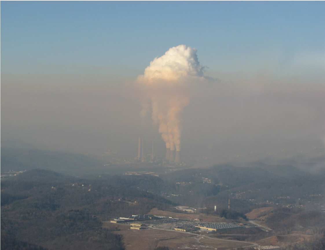
Photograph 3-7. Looking north from above Institute. Note the Cross Lanes Wal-Mart in the foreground. Note also: The active boiler exhaust stacks—the two most slender of the four taller stacks shown—are approximately 900 feet tall. That would indicate that the inversion layer above the plant was approximately 2,500-3,000 feet above the Kanawha River Valley floor.
