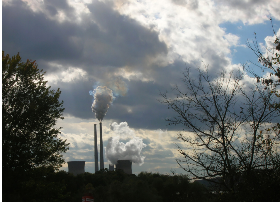
West Virginia coal-fired power plant
