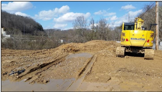
Figure 1 – Looking north through Area 3 at soils to be capped.
