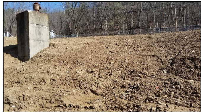
Figure 4 – Looking northeast up slope of Area 4. Seep/spring is located in approximate center of photo. Reinforcement to begin at concrete tower on left and extend across photo left to right.
