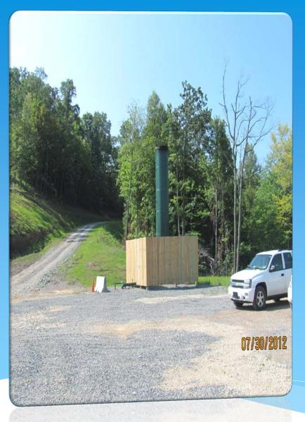
Storage Vessel – Combustor Control Device "Thermal Vapor Incinerator"
