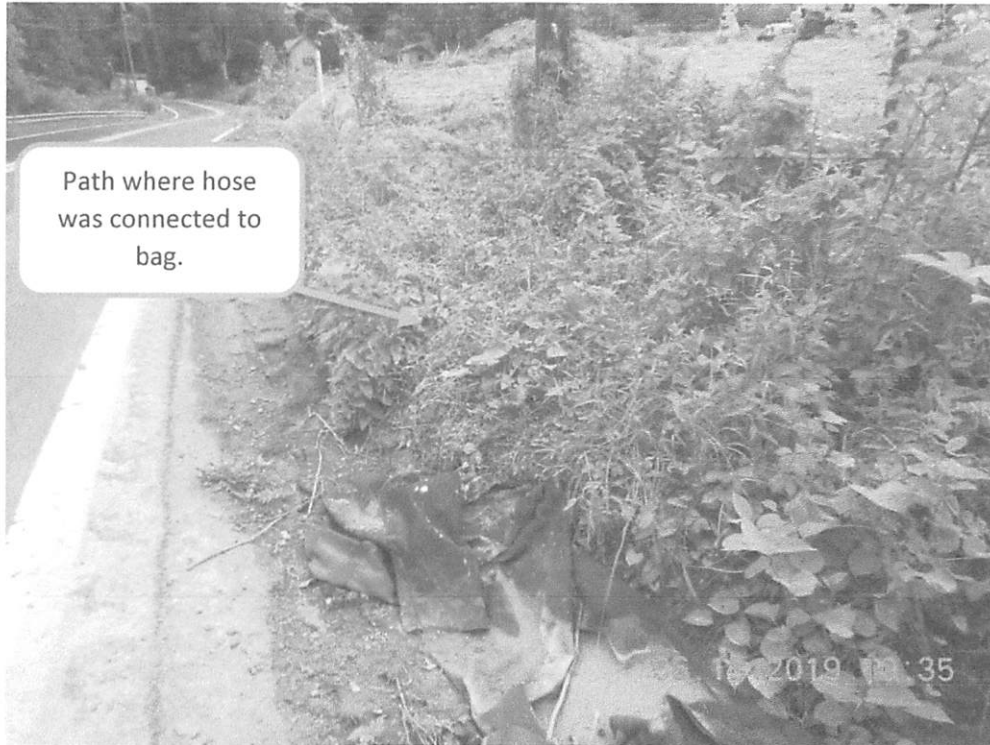
Dewatering bag in Rt. 76 conveyance.
