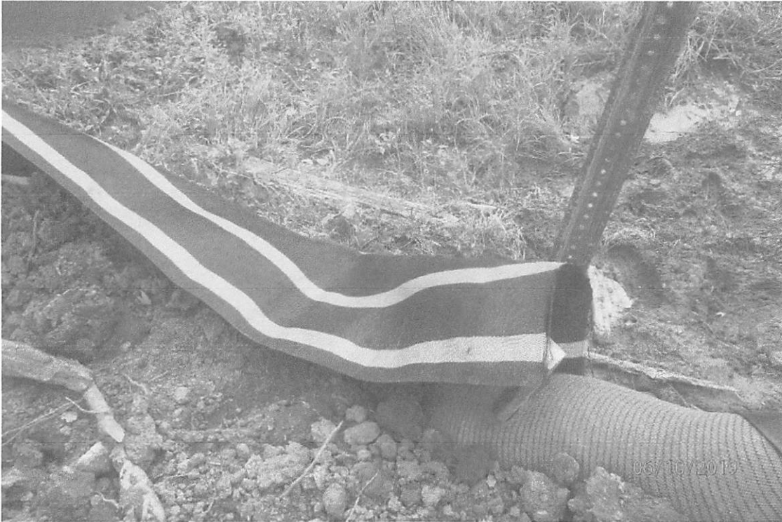
Improperly merged perimeter control and temporary bridge BMP at the UNT 23 crossing.
