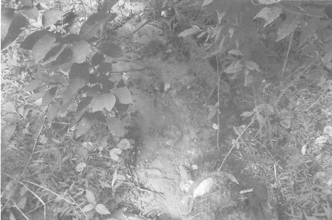
Offsite sediment deposits originating from the site adjacent to 447+00 as a result of the lack of installed waterbars and the associated fill slope erosion.
