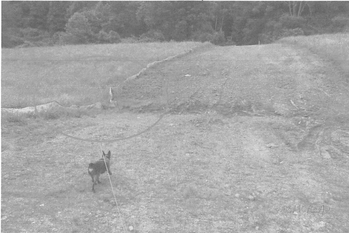
Project area adjacent to 400+50 (WL-18) showing where run-on stormwater is overwhelming the installed BMPs.
