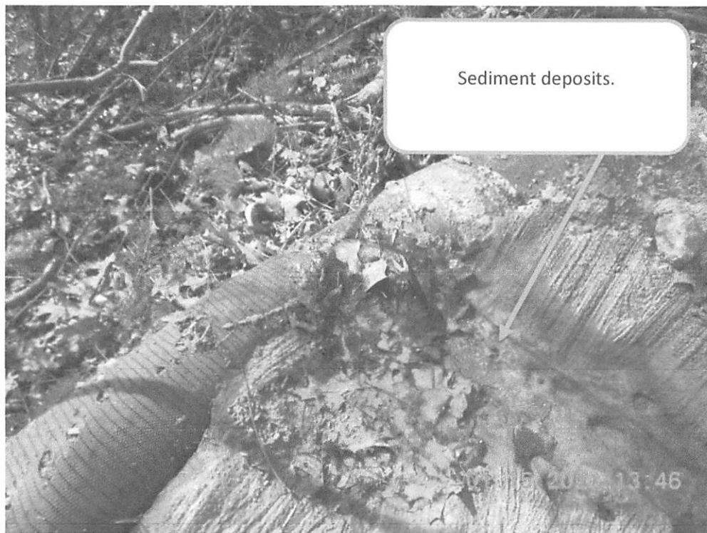
Concrete slurry outlet protection overtopped perimeter controls, allowing sediment laden water to leave site without going through an appropriate device.
