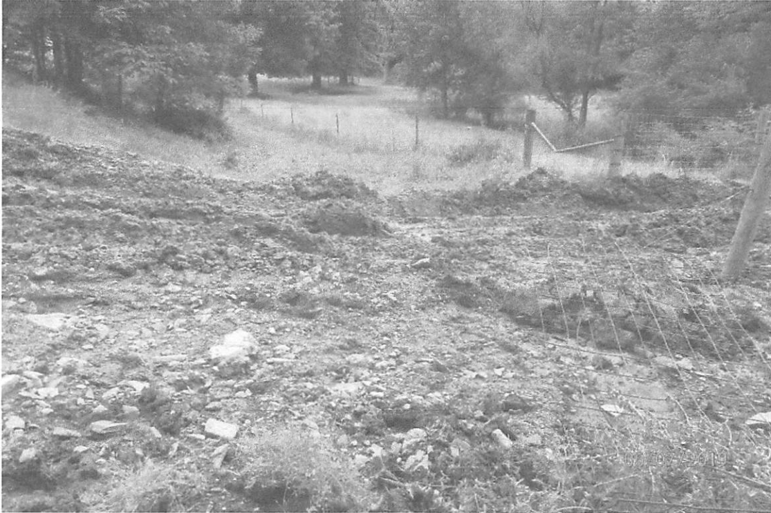
Project area adjacent to 482+85 showing the area where the upslope ephemeral stream is allowed to flow across the project with no BMPs in place.
