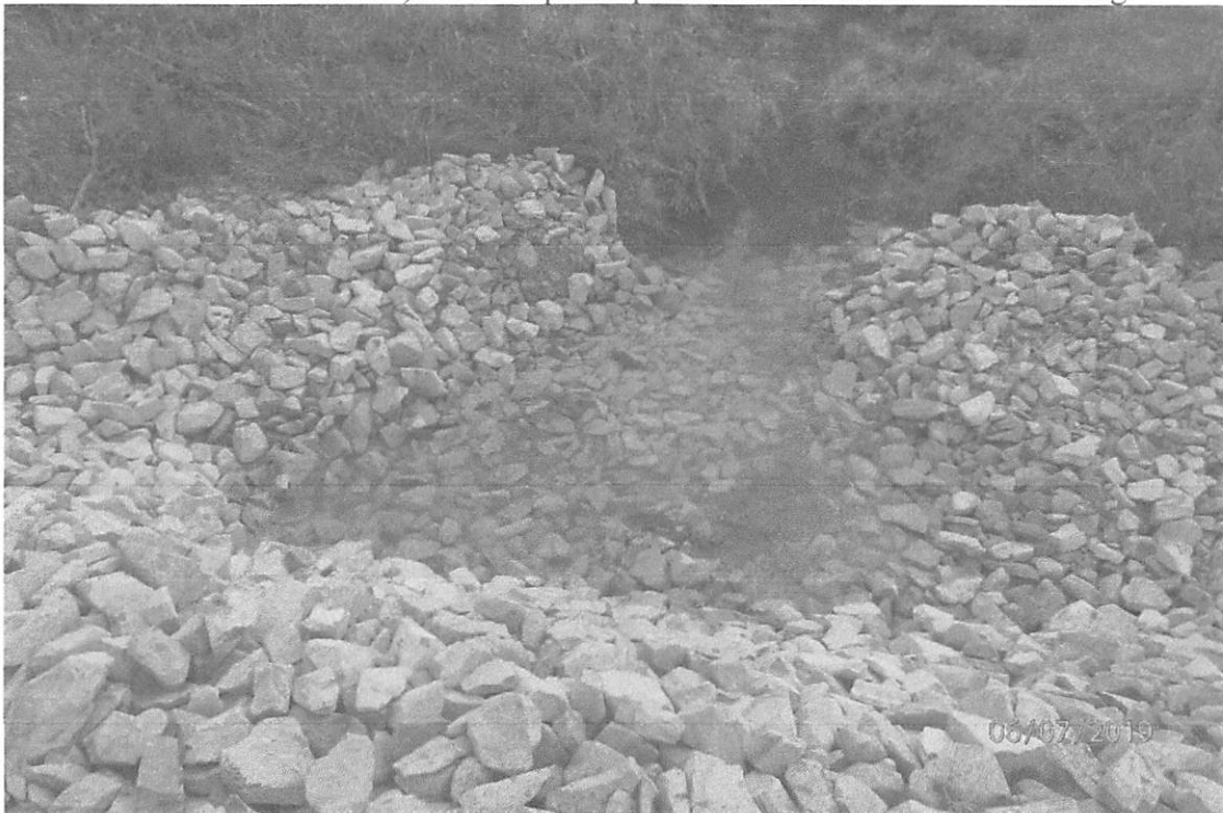
Stone that was placed in the stream by the site operator during the inspection at UNT Beards Run (39° 15.098' X 80° 10.735'). CNA deposits pictured upstream of the crossing.
