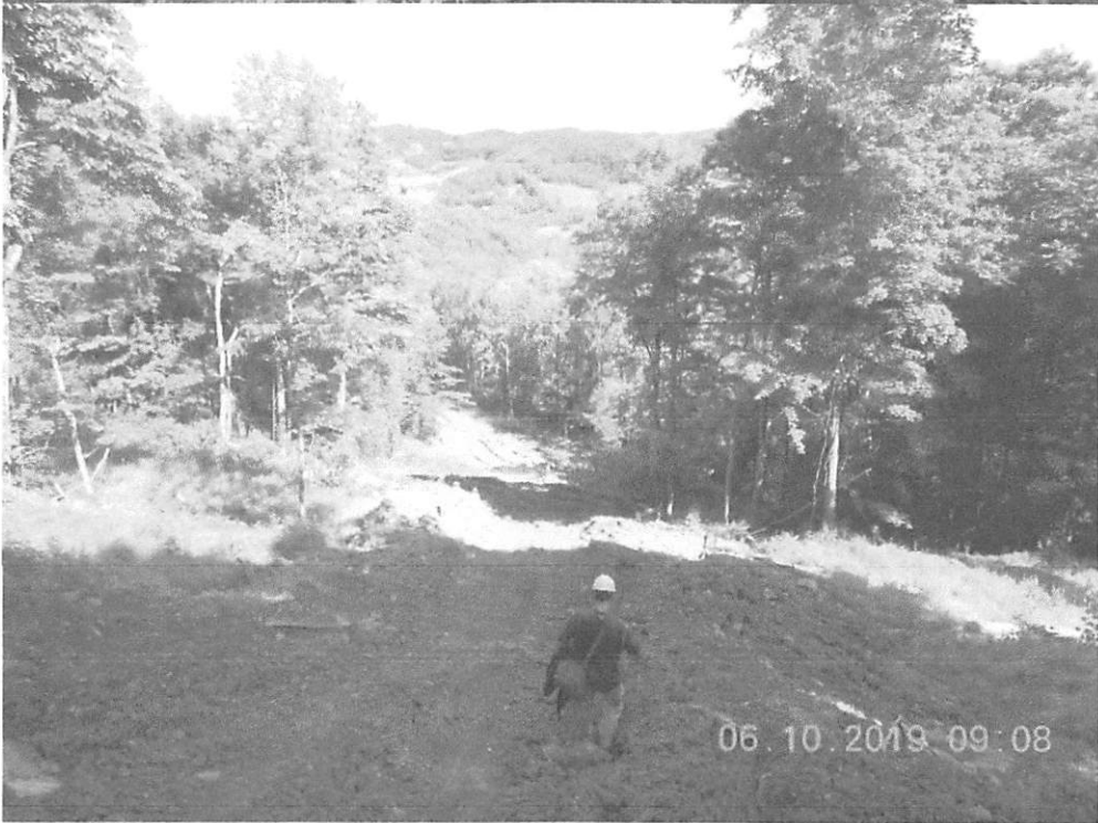
Station 265+50, SWPPP requires 10 water bars. This section of ROW was entrenched, and all water stayed on right of way until about Station 271+00.
