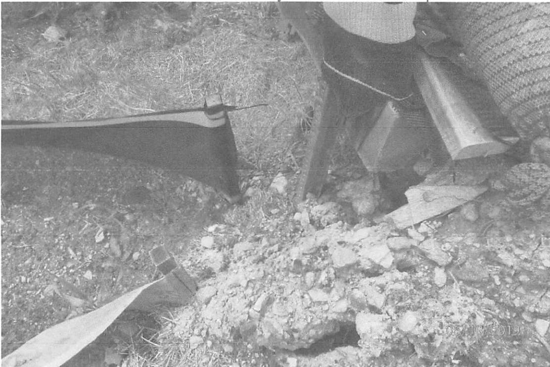
Improperly merged perimeter control and temporary bridge BMP at the UNT 22 crossing.
