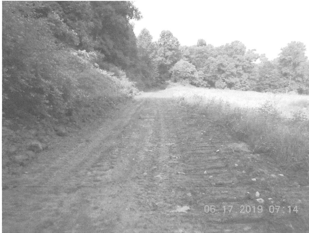
No controls were installed on this section of AR 5.
