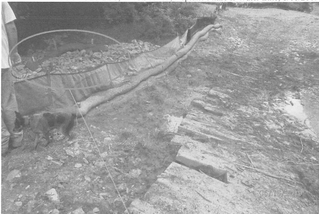
Project area adjacent to 365+00 (WL-14) showing a perimeter control with evidence of being overtopped and the need to modify the approved SWPPP.
