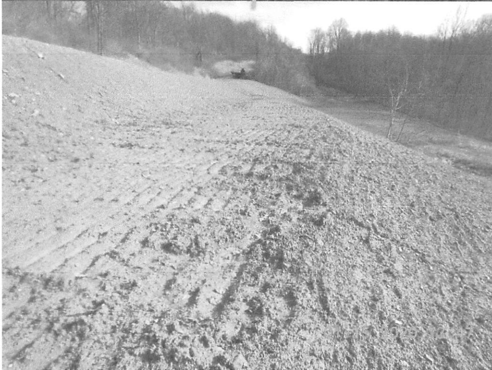
Erosion rills on fill slope due to lack of fill slope protection.
