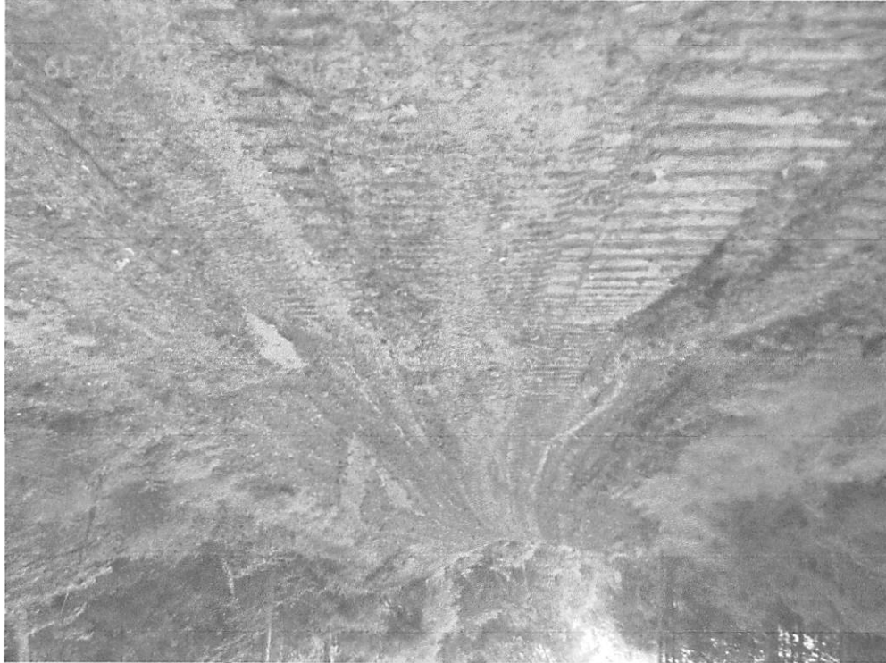
Erosion rills forming at the end of water bars that are lacking terminus treatment.
