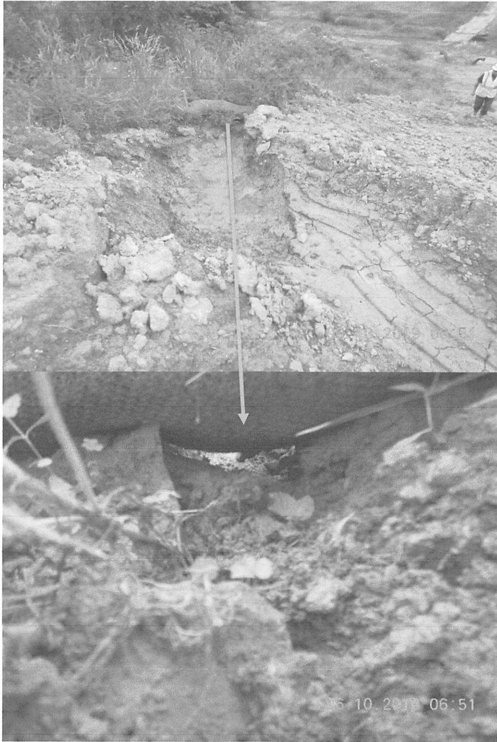
Bypass on water bar terminus treatment.
