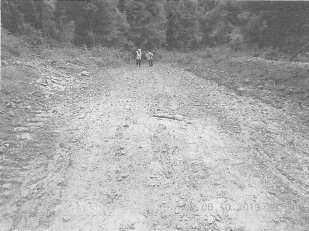
Station 214+00 to 219+50, SWPP calls for SS2 slope interceptors and 10 water bars with terminus treatment.
