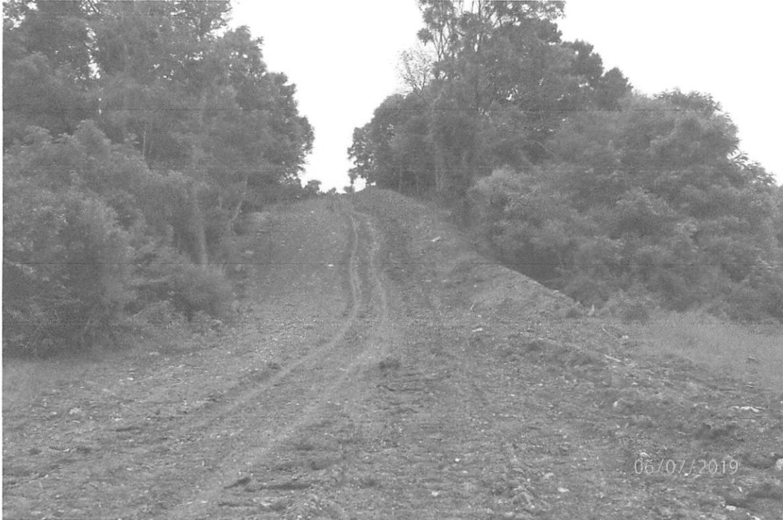
Hillside upslope of 490+00 showing the lack of installed water bars and silt saver 2 slope interceptors.
