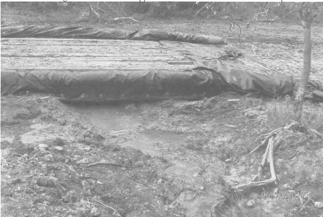
WL-28 showing the area where sediment laden water from the project is leaving the site without going through an approved device. The approved SWPPP does not indicate the need for BMPs in this area even though it is evident that a stream of water is present.
