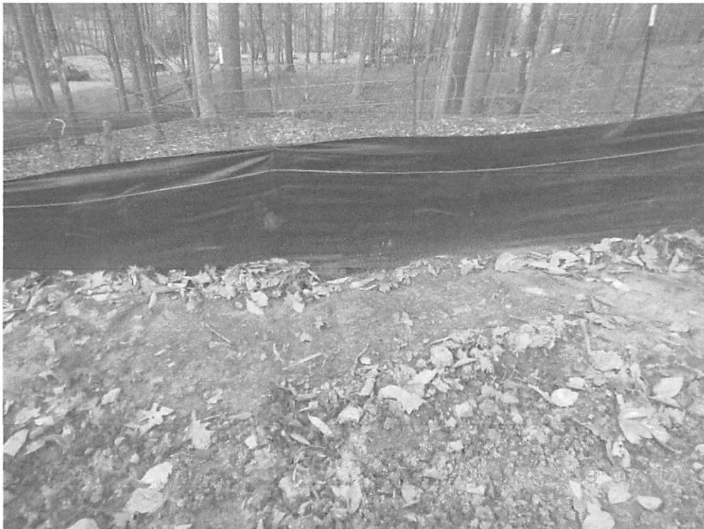
Stat. 217+25, Perimeter controls throughout site were nonfunctional due to bypasses. Silt fence not toed-in correctly.
