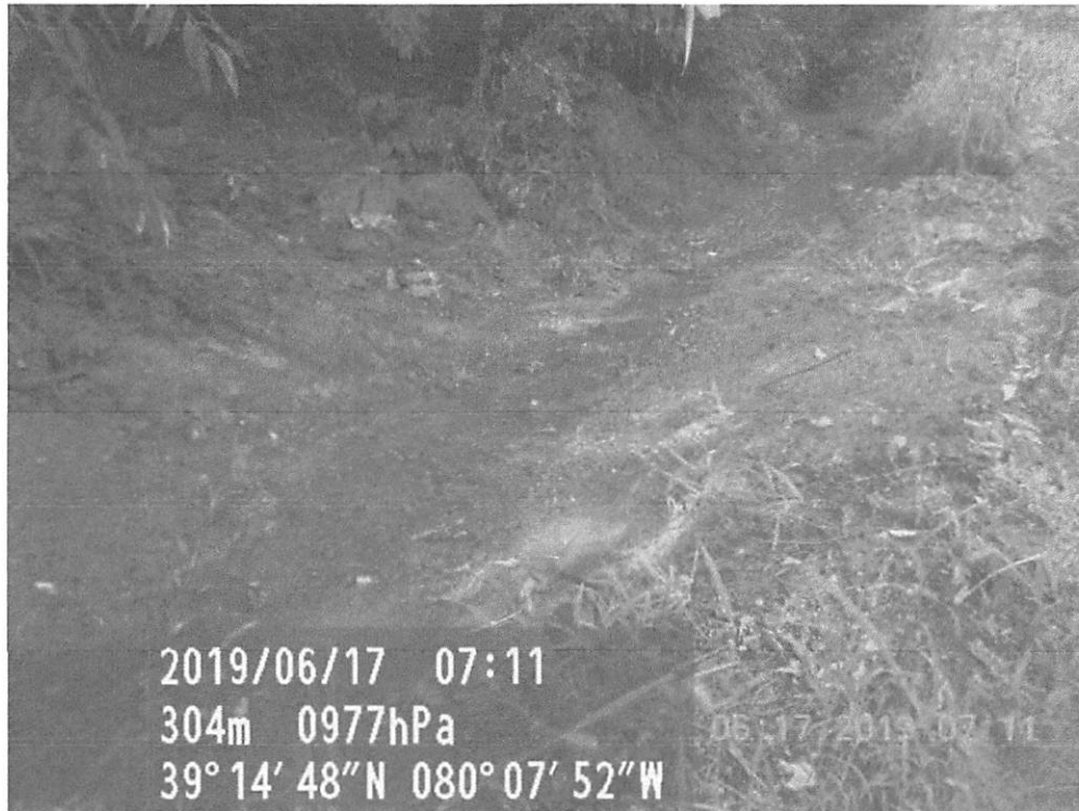
Ditch line along AR 5 is an unlabeled UNT of Simpson Creek for about 100 ft. The clean water division had been excavated and was not stabilized.
