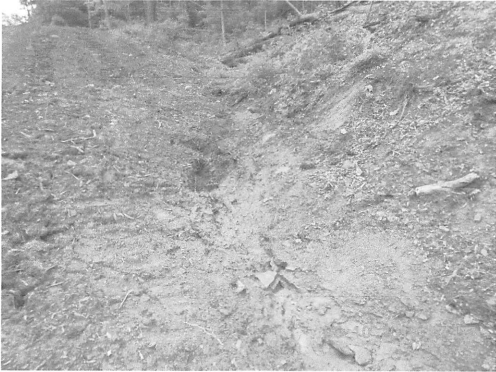
Head of first unlabeled UNT at Station 211+00 is blocked.
