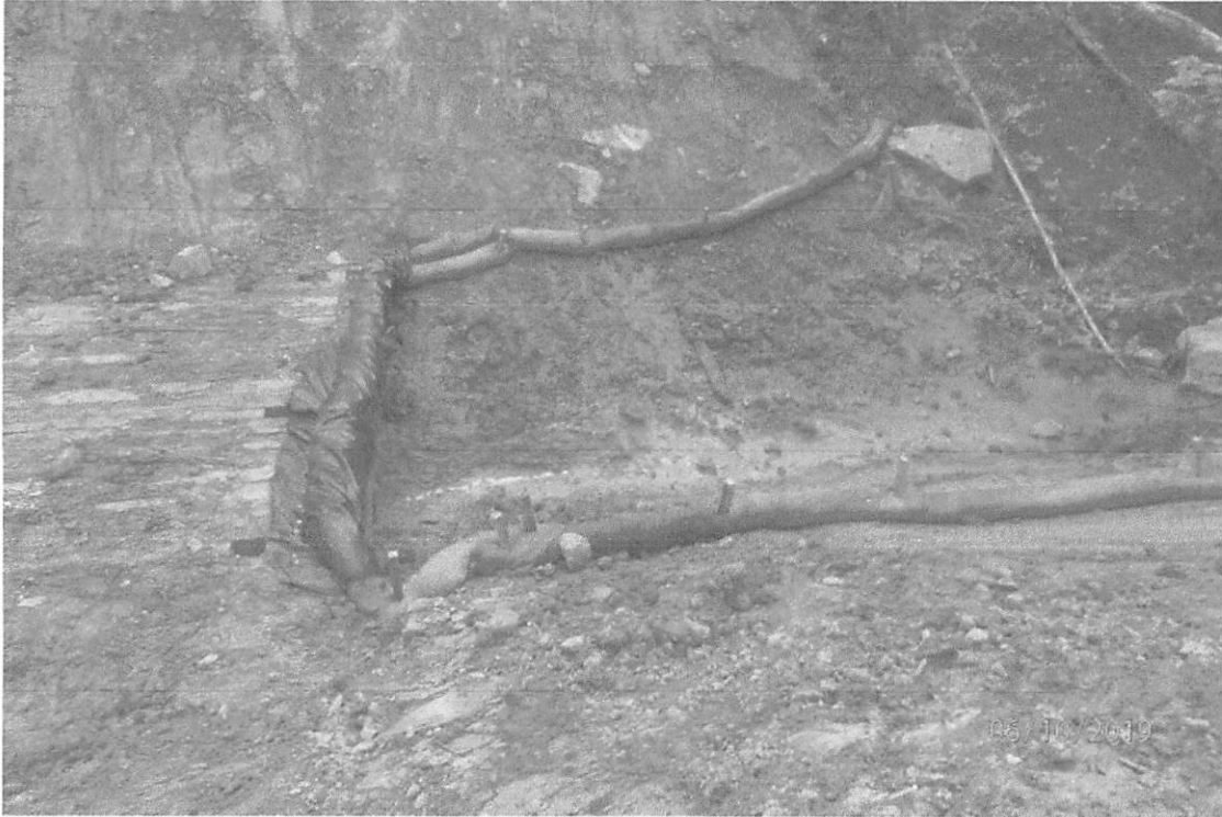
UNT 24 crossing showing the area where a stream crossing took place without the pump-around or flume crossing in place.
