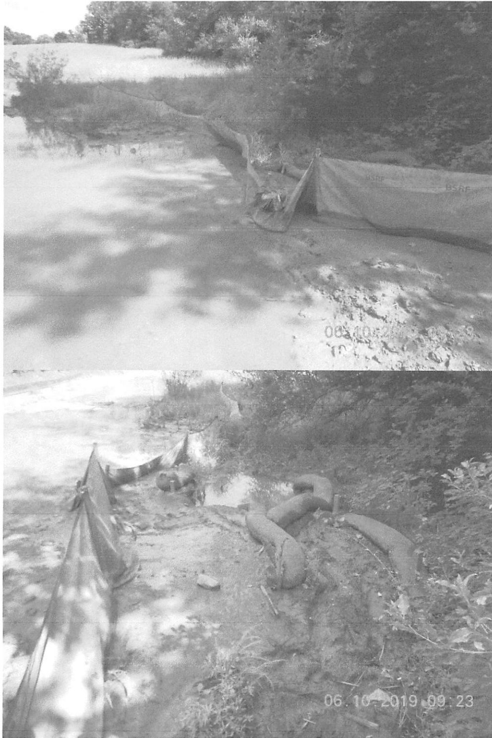
Station 258+00, WL 5 perimeter controls in disarray.
