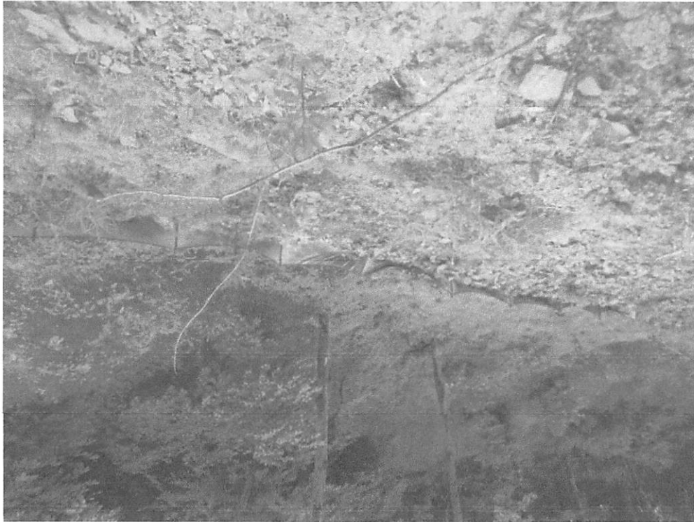
Erosion rills forming at the end of water bars that are lacking terminus treatment.
