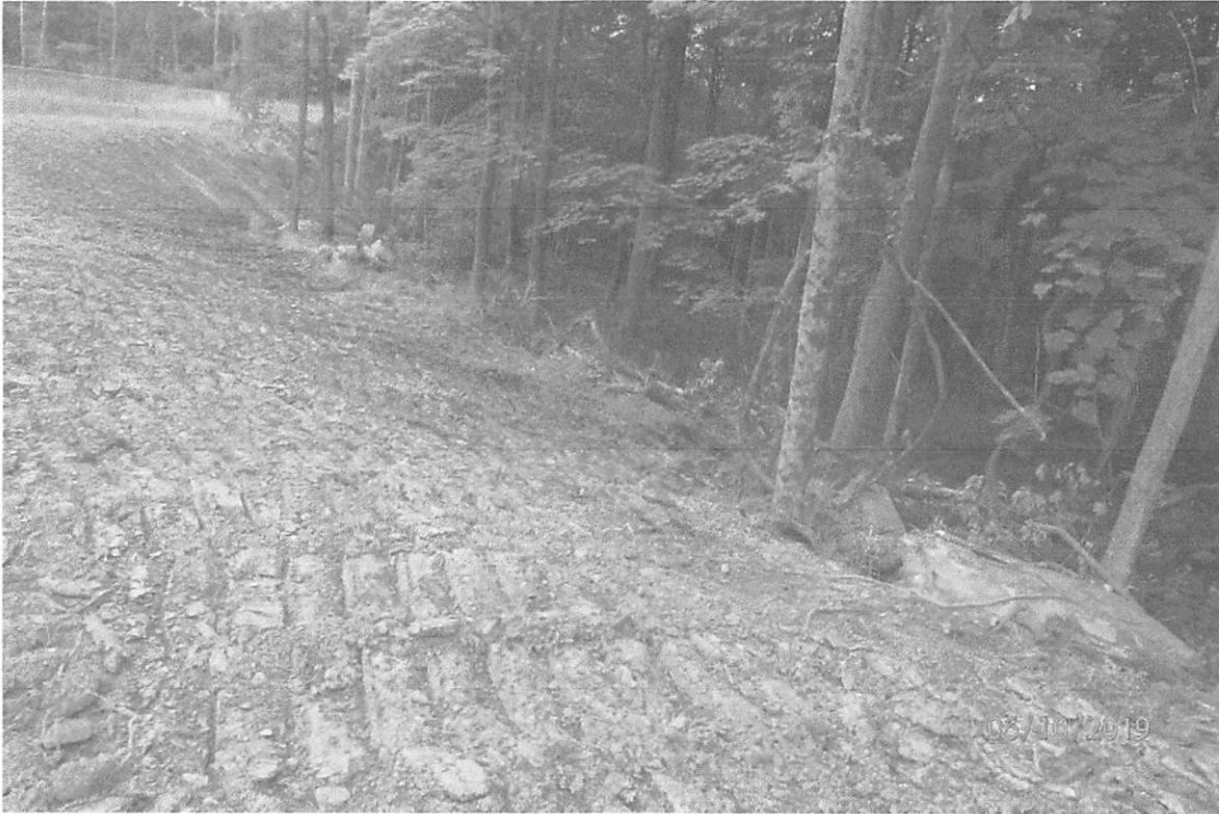
Area lacking perimeter controls that are indicated in the approved SWPPP adjacent to 519+00.
