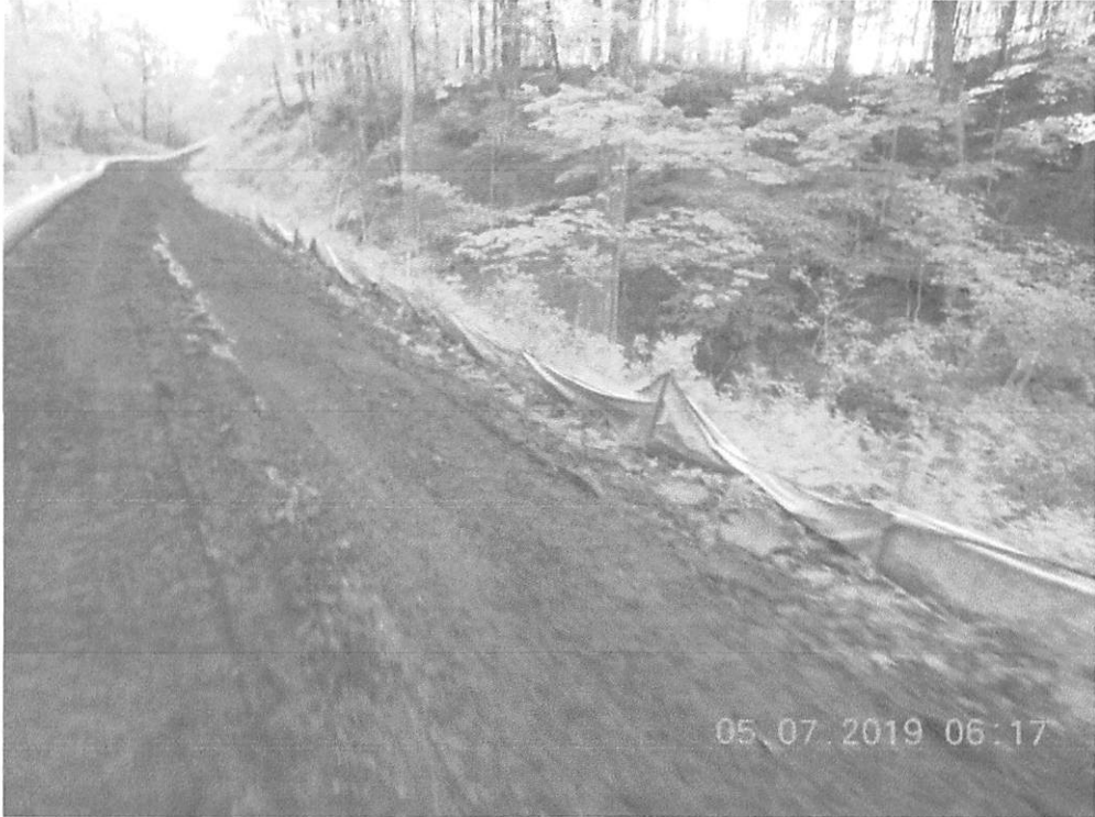
Lack of controls, as observed and documented on May 7, 2019.
