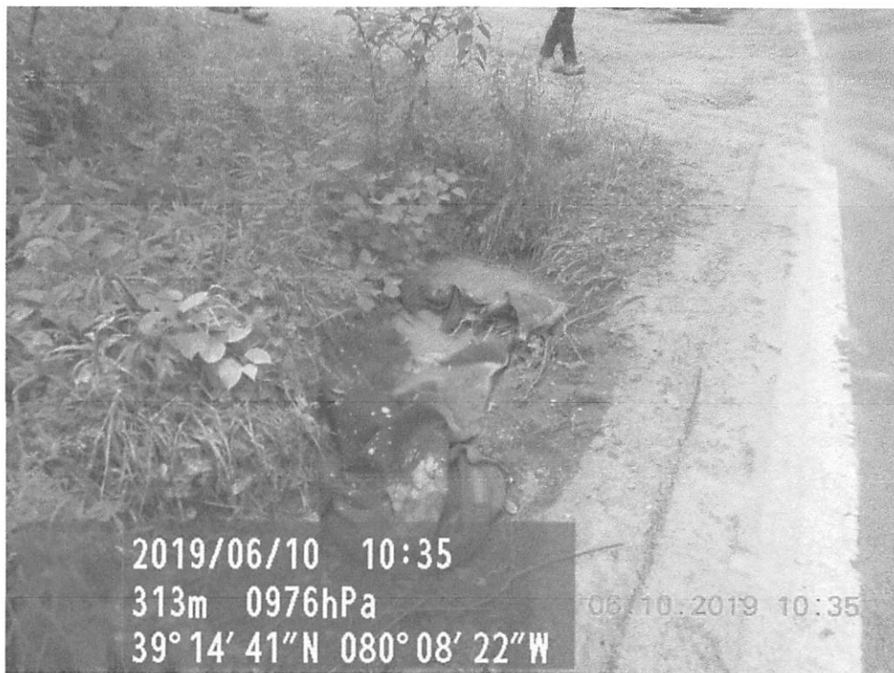
Sediment deposit on bottom of Rt. 76 conveyance.
