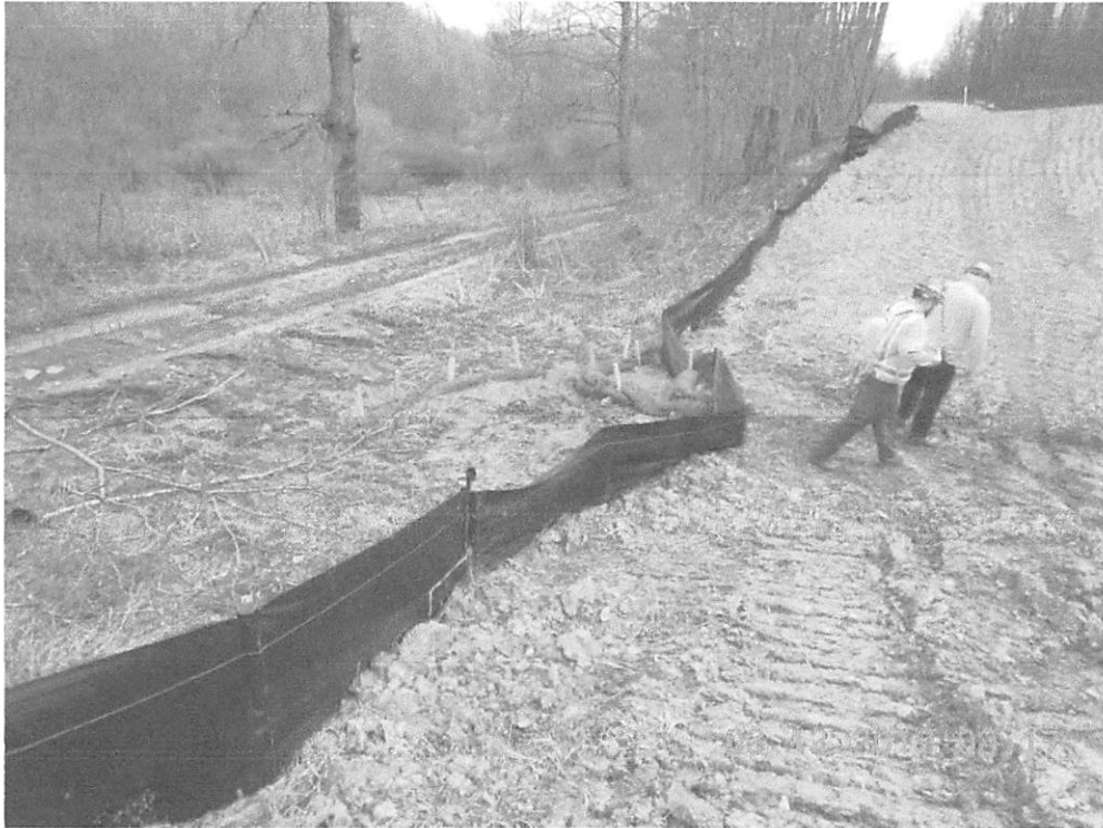
Stat. 175+00, CFS was not conjoined with SF correctly, creating a bypass.
