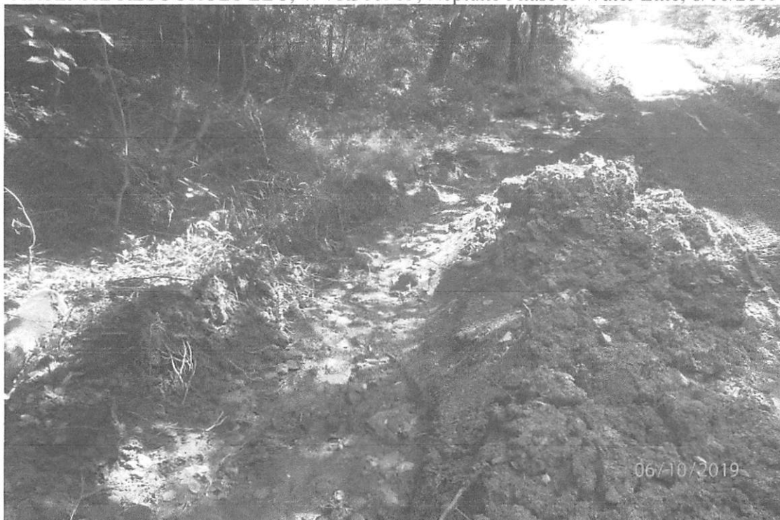
Ephemeral UNT Simpson Creek showing instream disturbance and the lack of installed BMPs to prevent sediment laden water from entering the stream.
