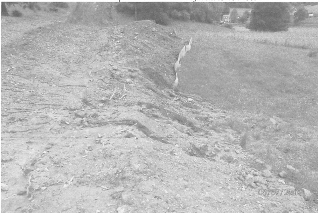
Unmaintained perimeter controls adjacent to 485+50.
