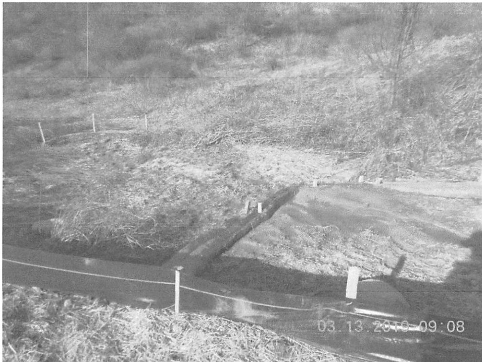
Stat. 155+50, Sediment deposit off site.
