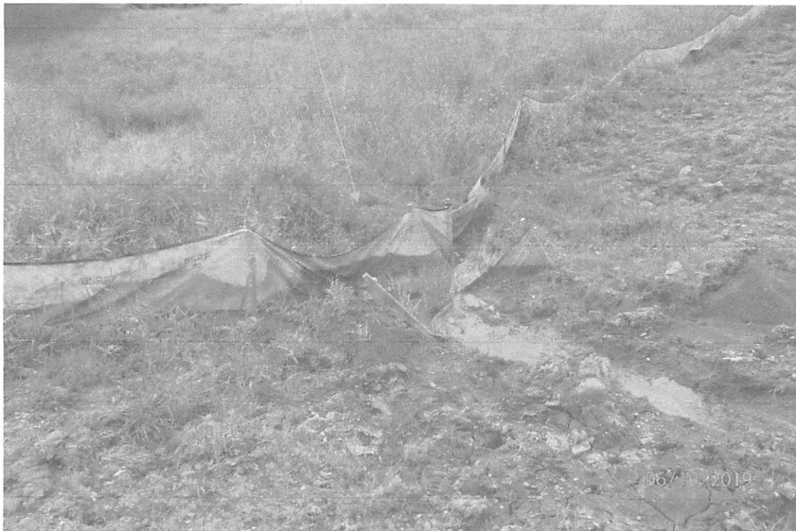
Installed BMPs adjacent to 400+50 that show evidence of being overtopped and are in need of maintenance.
