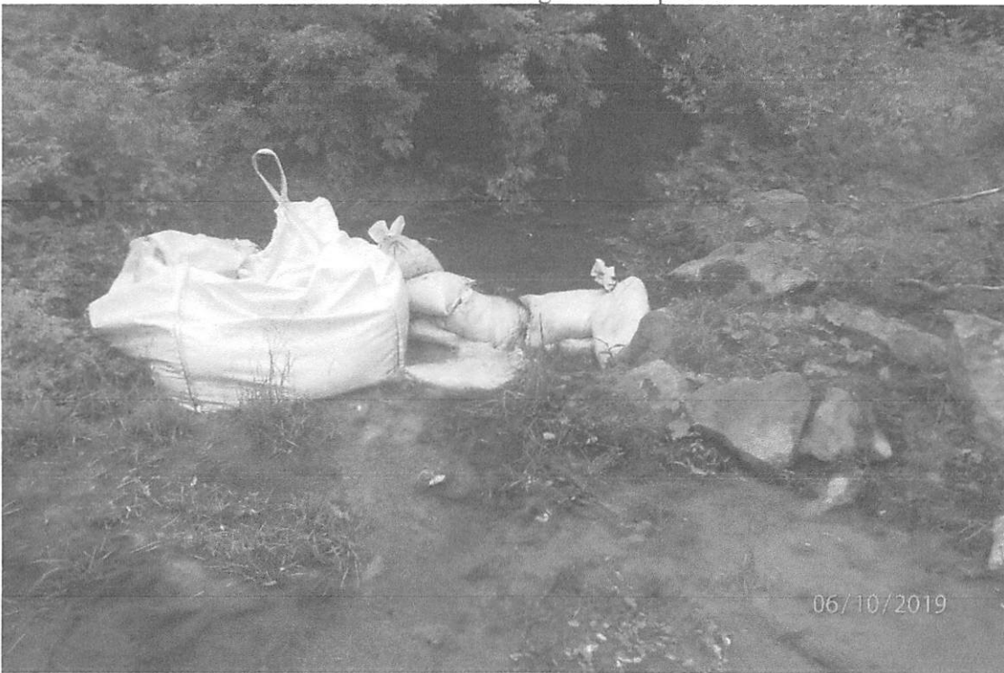
Instream solid waste in UNT 19 as a result of the contractor leaving the sand bag coffer dam in the stream after the stream crossing was completed.
