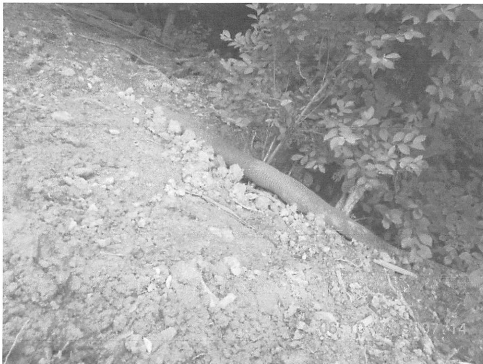
Inequivalent CFS was installed instead of SS2, as required by the SWPPP. CFS is riddled with bypasses and could allow sediment laden water to leave site.
