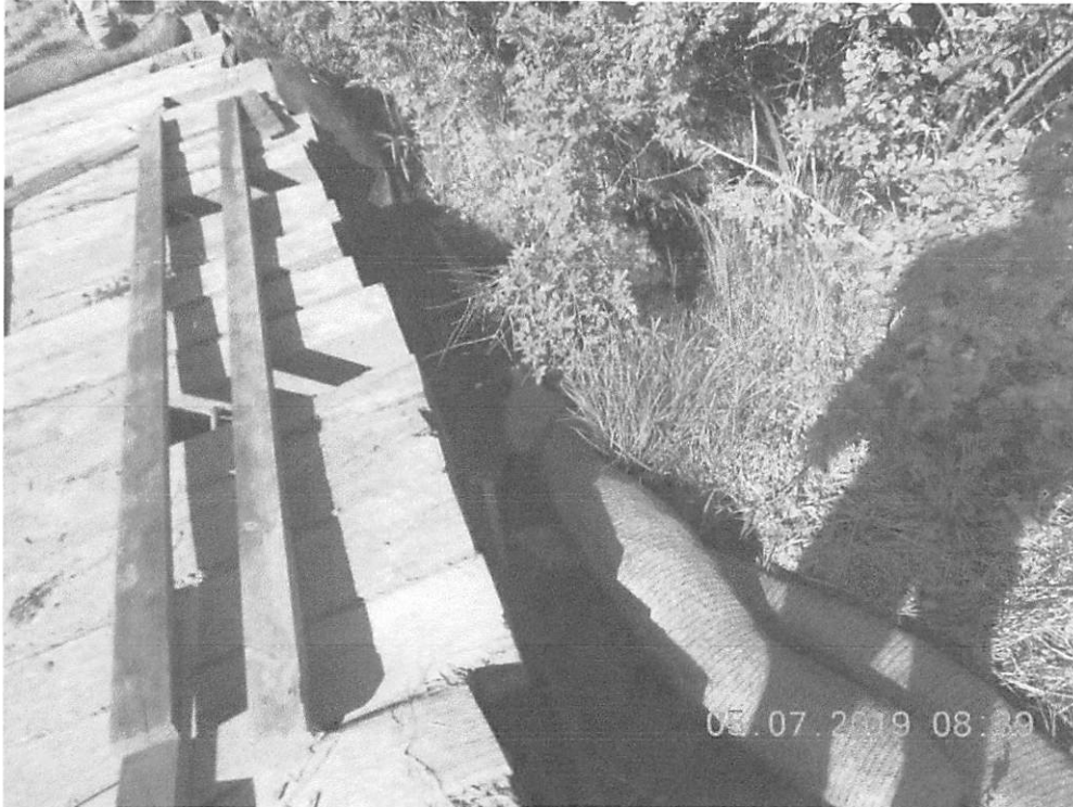
Maintenance at Station 185+00, bridge controls.
