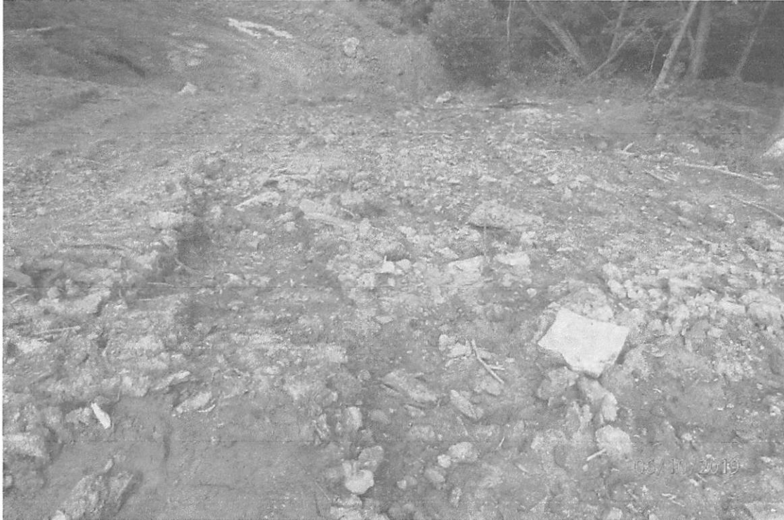
Project area upslope of 447+00 showing the lack of waterbars indicated in the approved SWPPP. The approved SWPPP indicates that 9 waterbars should be installed, but only 3 were in place.
