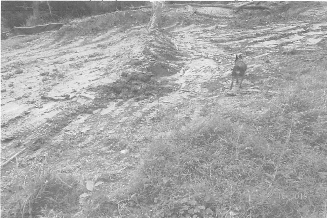
Waterbar in the Beards Run watershed that lacks waterbar terminus BMPs indicated in the approved SWPPP.
