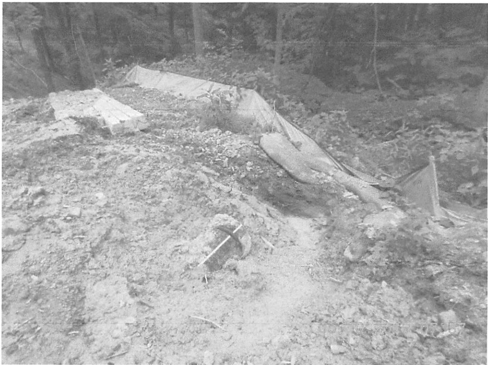
Station 211+00, Outfall for flume pipe for first unlabeled UNT at this location.
