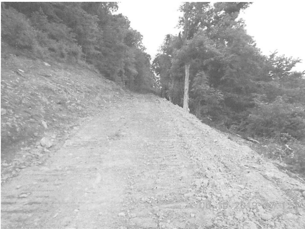
SWPPP requires 6 water bars along with SS P2 slope interceptors as perimeter controls. However, continuous 8" CFS was installed.
