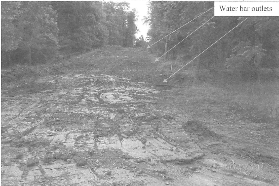
Improperly installed waterbars in the Beards Run watershed showing waterbar outlets that do not have positive drainage and allow water to flow back onto the right-of-way.
