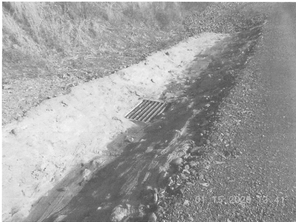
Drop inlet in concrete slurry diversion ditch with no inlet protection and sediment deposits present from unstable area above the diversion ditch.
