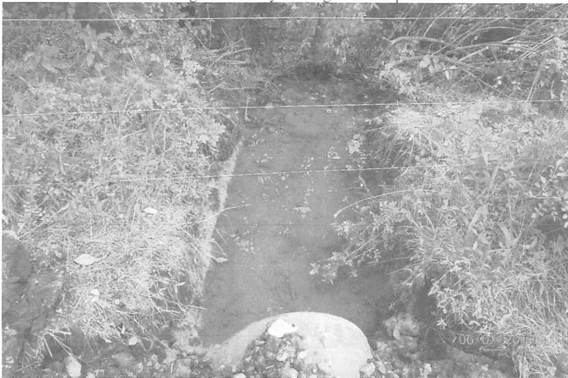
Area where sediment laden water leaves the site without going through an approved device.
