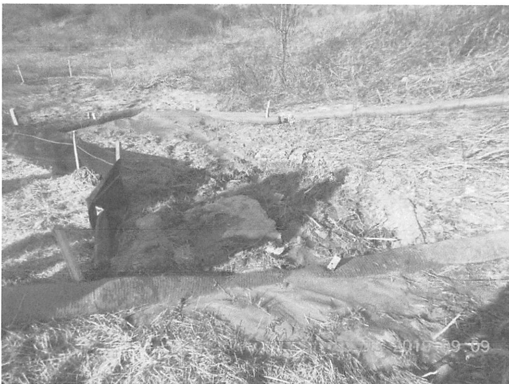
Maintenance is lacking throughout project site.
