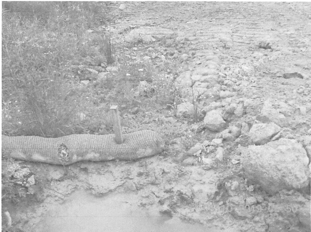
Bypass on water bar terminus treatment. 8 inch CFS installed, but SWPPP requires 18 inch.
