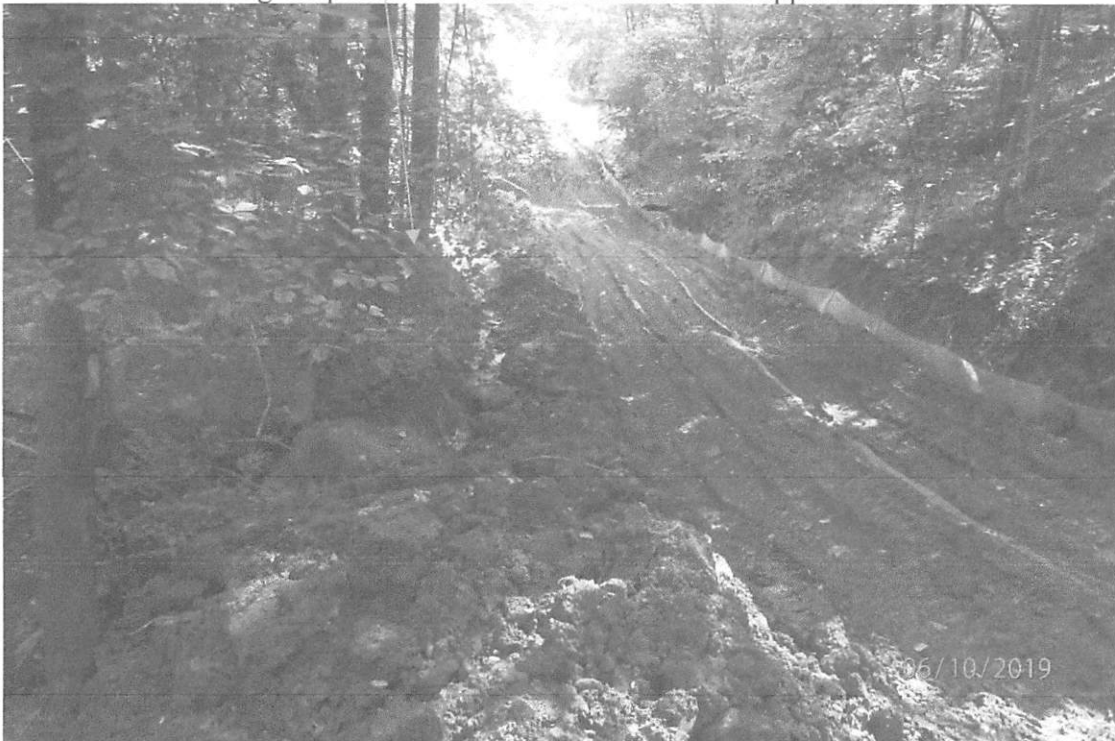
Access Road 7 showing the lack of installed perimeter controls indicated in the approved SWPPP.
