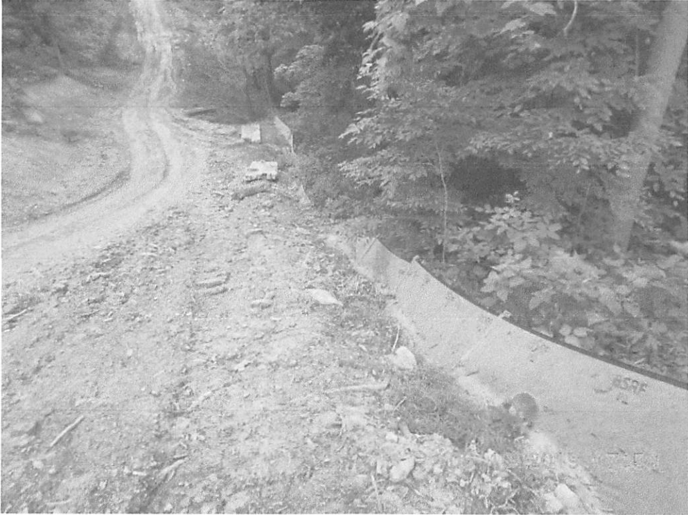
Station 208+00, Erosion rill is present, and SS2 is overwhelmed with sediment.
