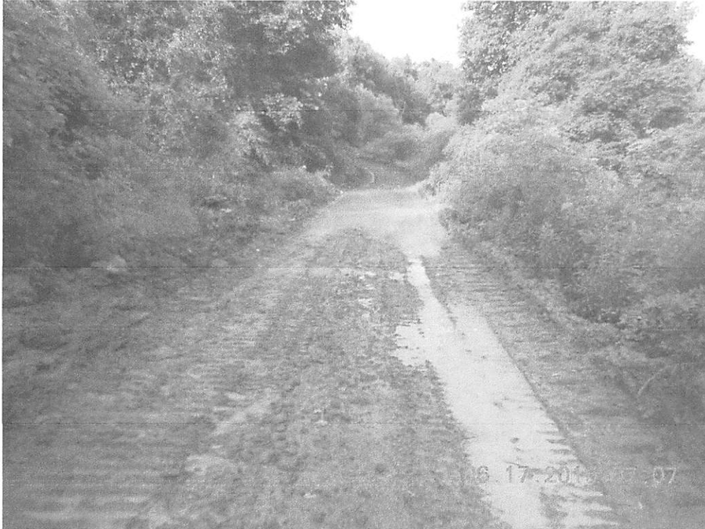
SWPPP indicates that all unpaved roads on the site shall be graveled or have other durable surface. AR 5 was not graveled and shows signs of significant wear.
