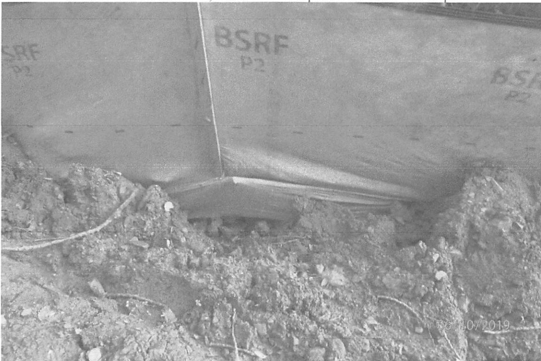
Improperly installed perimeter control on access road 9 showing an area where sediment laden water can bypass treatment under the BMP.
