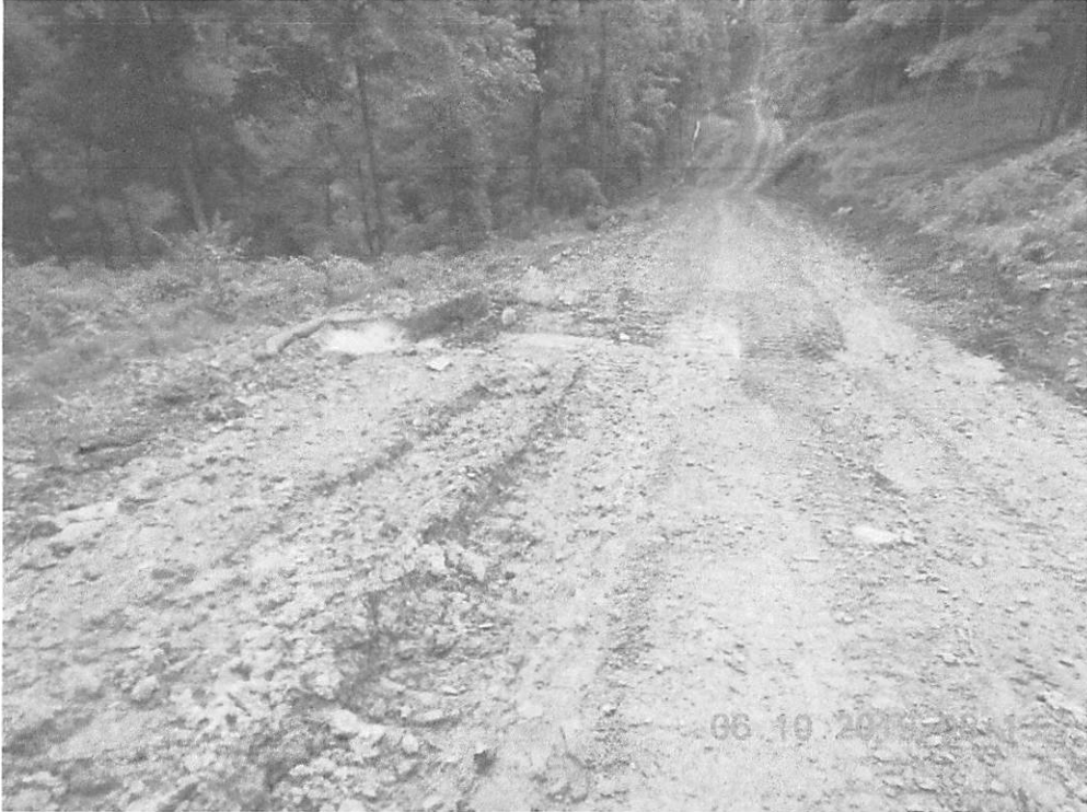
Water bar is ineffective, because water bypasses, resulting in erosion rills at the bottom of the slope.
