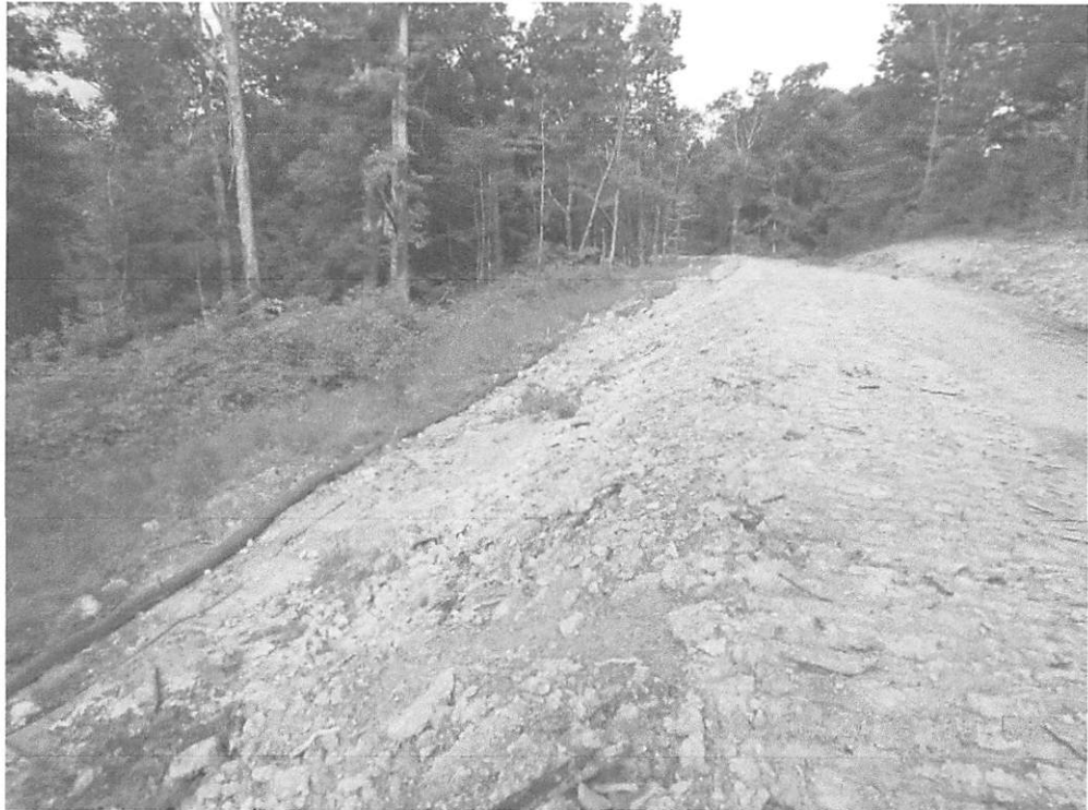
Station 260+00, SWPPP requires SS2 slope interceptors. When controls were damaged by pulling pipe strings, 8 inch CFS was installed in its place.
