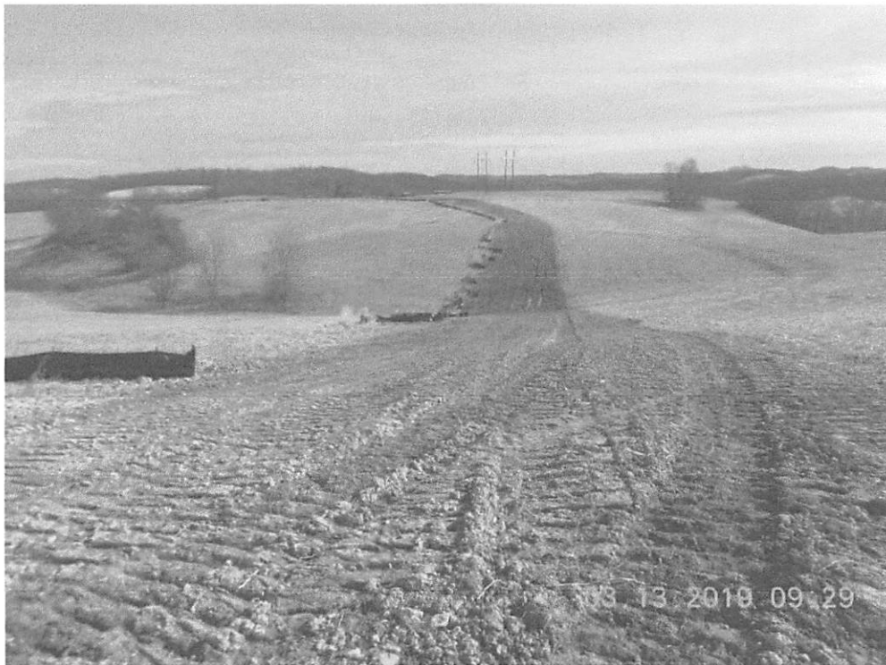
Stat. 147+75, Water bars were not installed as indicated in the SWPPP.
