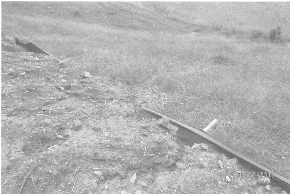
Unmaintained perimeter controls adjacent to 484+00.
