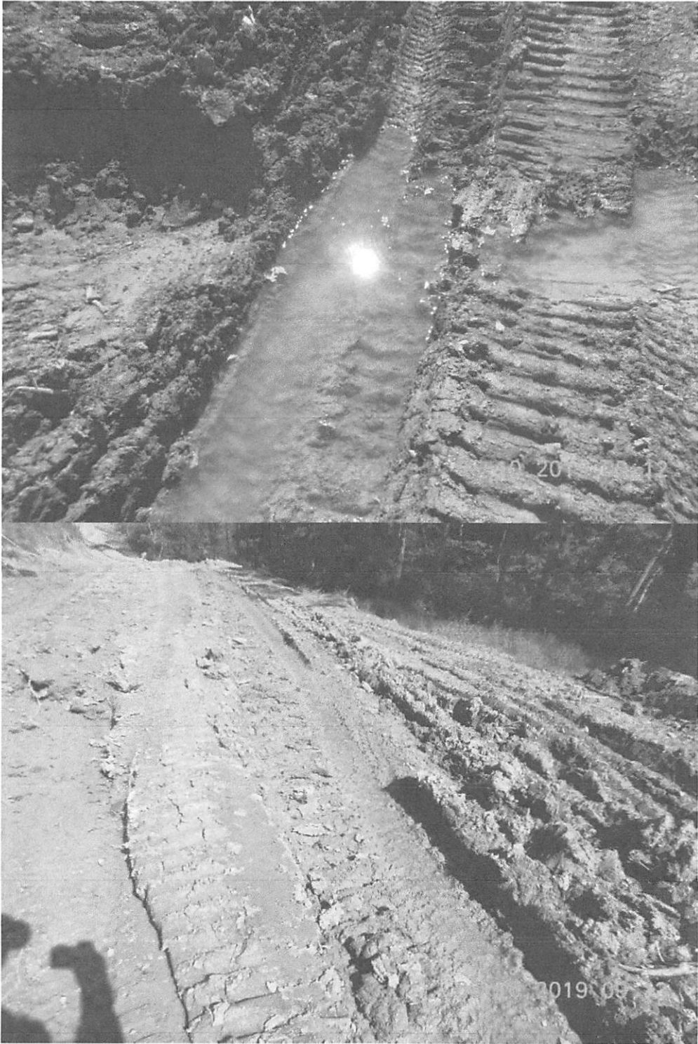
Station 271+00, Water bars are tracked through, causing them to fail. Water can bypass and form erosion rills in tracks.
