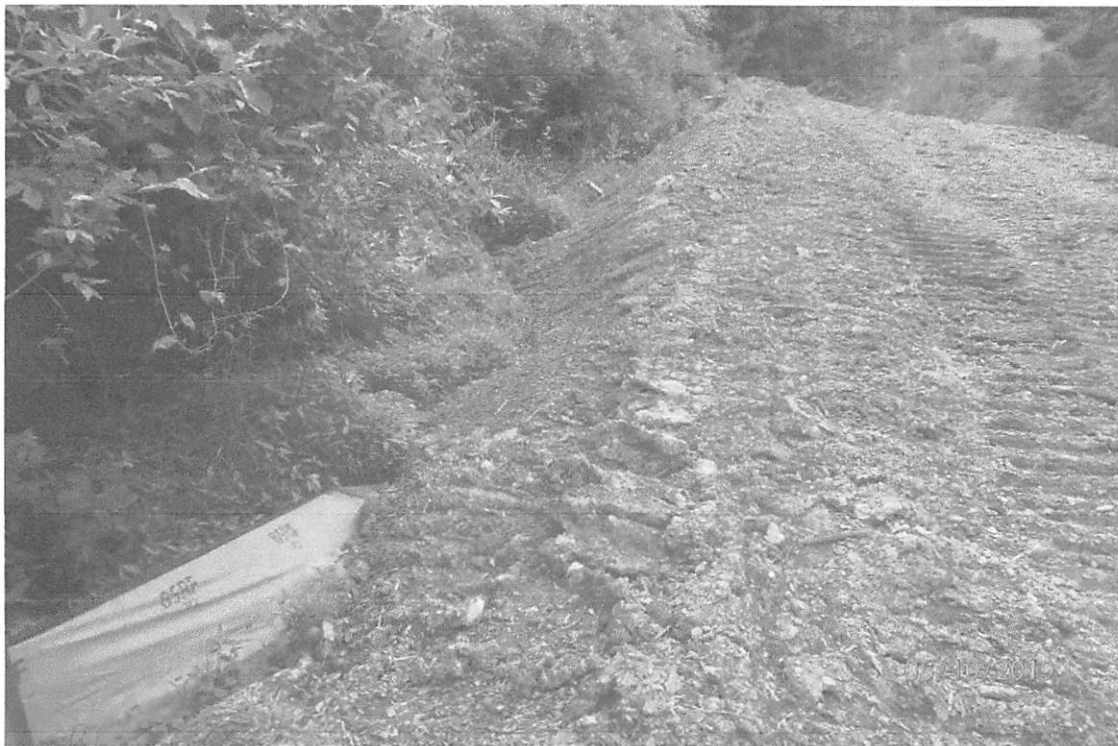
Perimeter control in need of maintenance in the Beards Run watershed.
