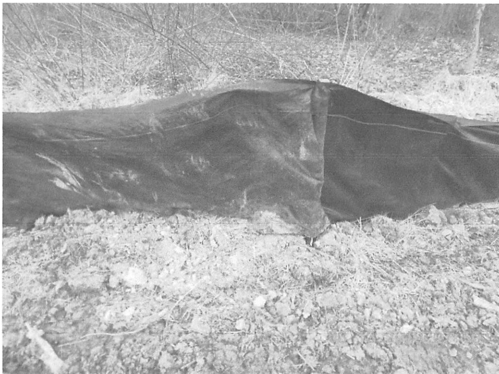
Stat. 193+00, SF failure from either not being conjoined or toed-in correctly.
