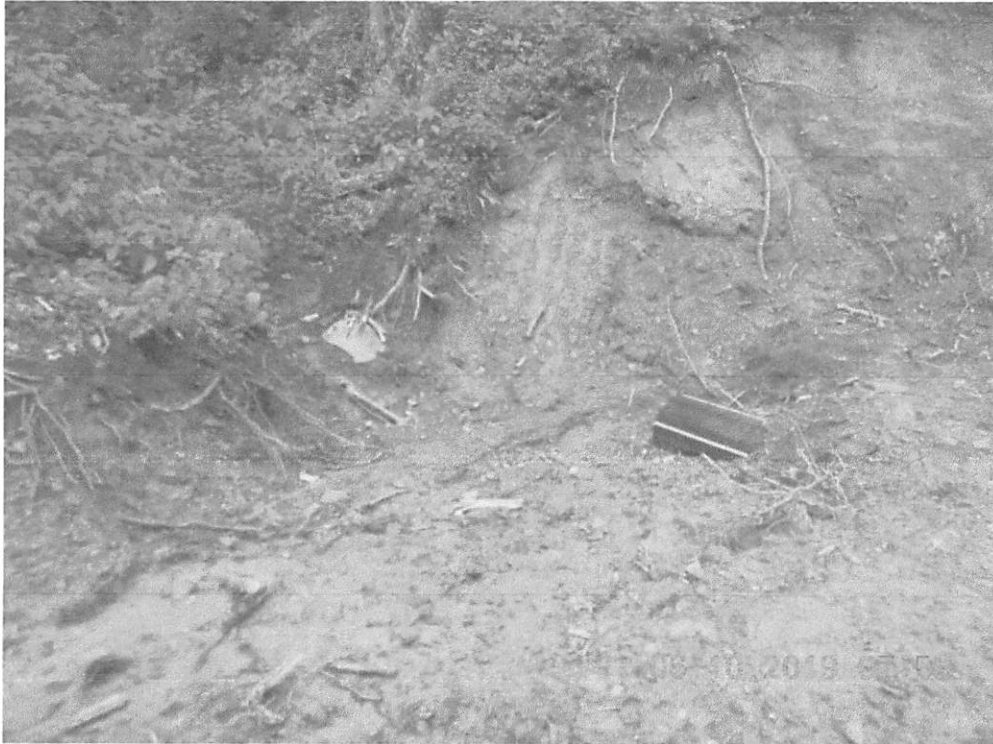
Second unlabeled UNT around Station 211+00. Head of culvert flume.
