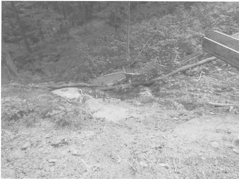
Tail of culvert around Station 211+00. Did not install an energy dissipater as detailed on Page ENV D10. Maintenance needed on perimeter controls.
