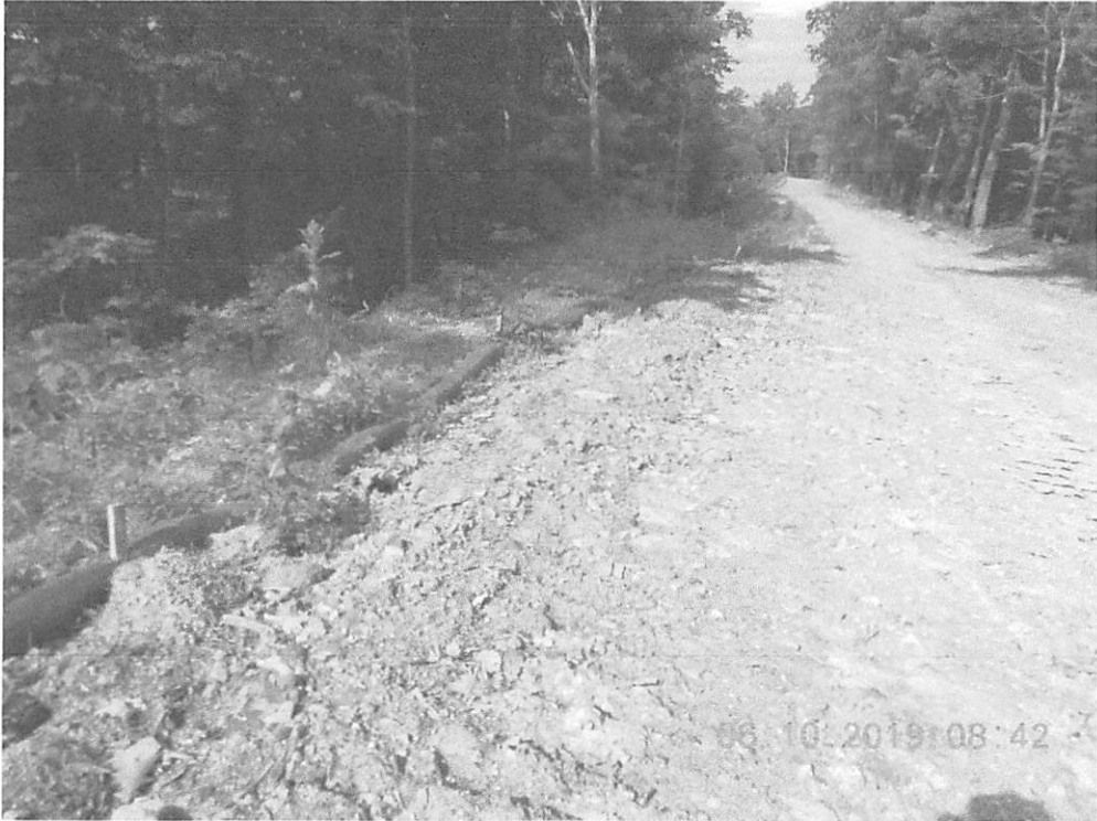
About Station 242+00, SWPPP calls for slope interceptor to be installed.
