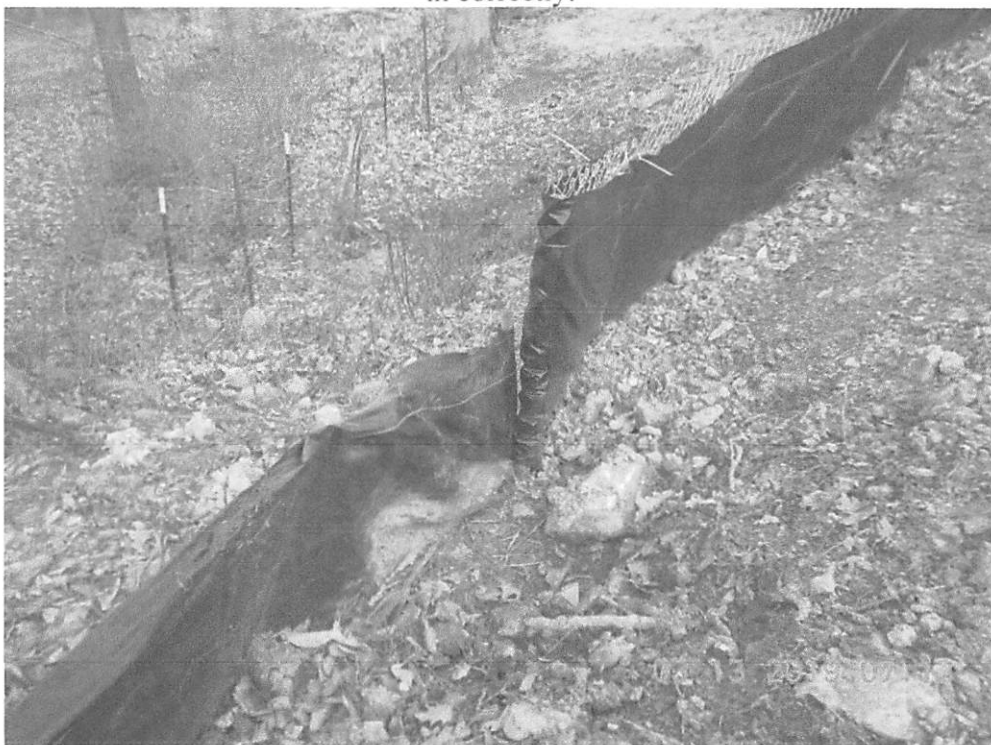
Stat. 213+75, Perimeter controls throughout site were nonfunctional due to bypasses. SSF not tied together with SF, creating a bypass.
