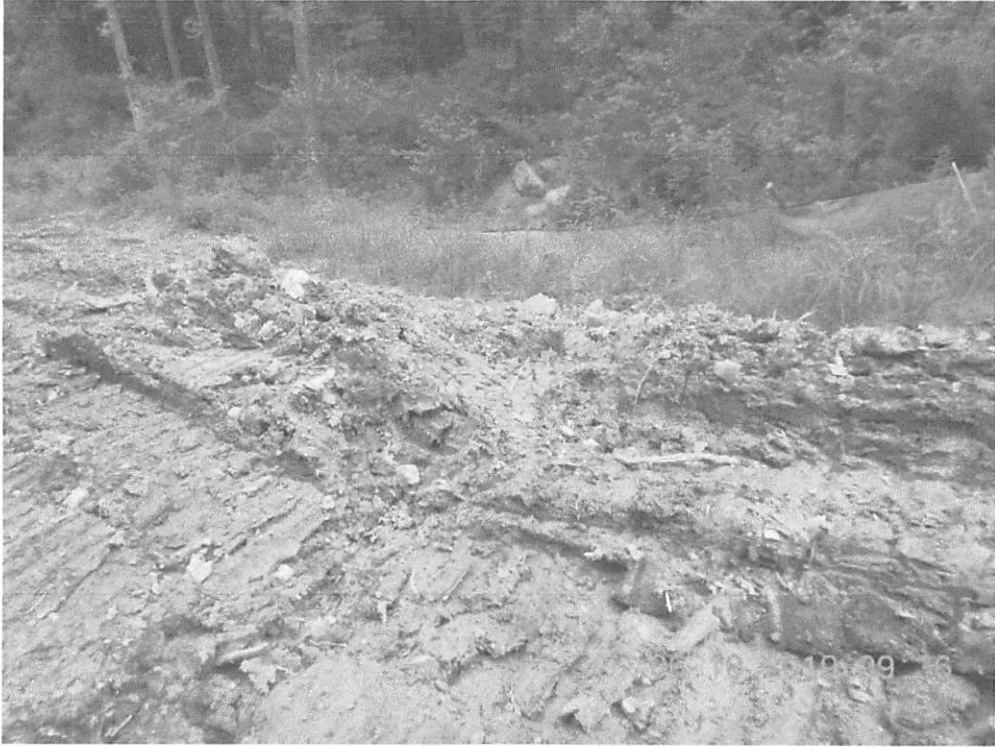
Station 301+00, Water bar with no terminus treatment. SWPPP requires SS2 slope interceptors.
