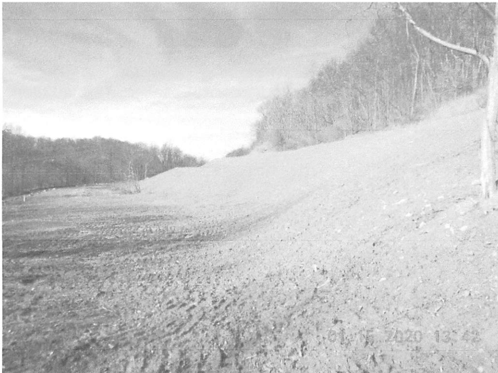
Area that failed to germinate and was not reseeded after 30 days.
