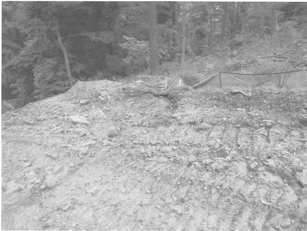
Station 207+50, Only water bar noted out of 9 required by SWPPP. Maintenance needed on sump. Water bar is ineffective, and erosion rills are starting to form.
