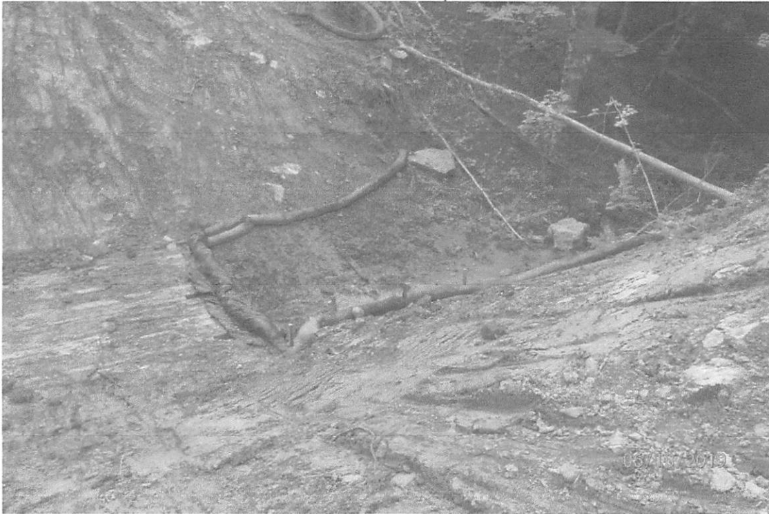
Improperly installed perimeter control at the UNT 26 crossing. The approved SWPPP indicates that silt saver 2 will be installed, but 8-inch compost filter sock was in place.
