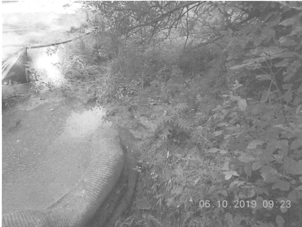
Bypass of WL5 perimeter controls
