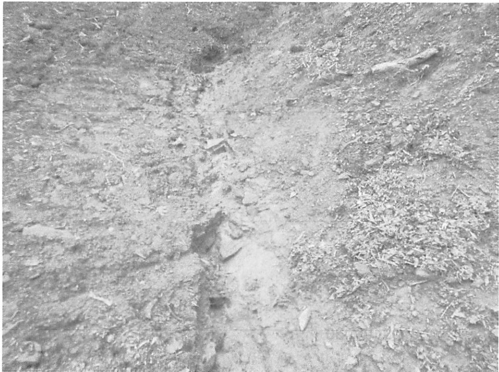
Clean water diversions at Station 211+00 between first and second unlabeled UNT.
