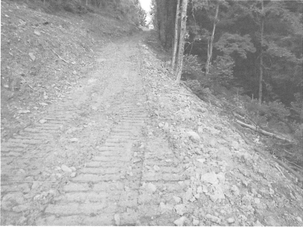
Station 199+50, No water bars installed. SWPPP requires SS2 slope interceptors.
