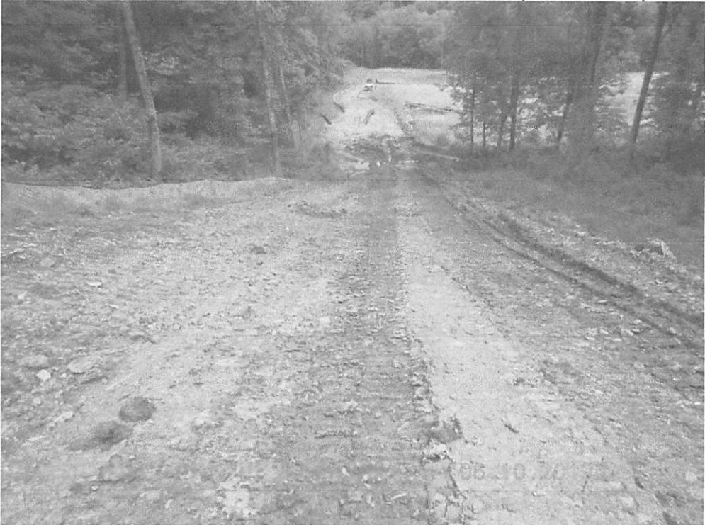
Station 304+00, WL 8, Required SS2 was not installed.
