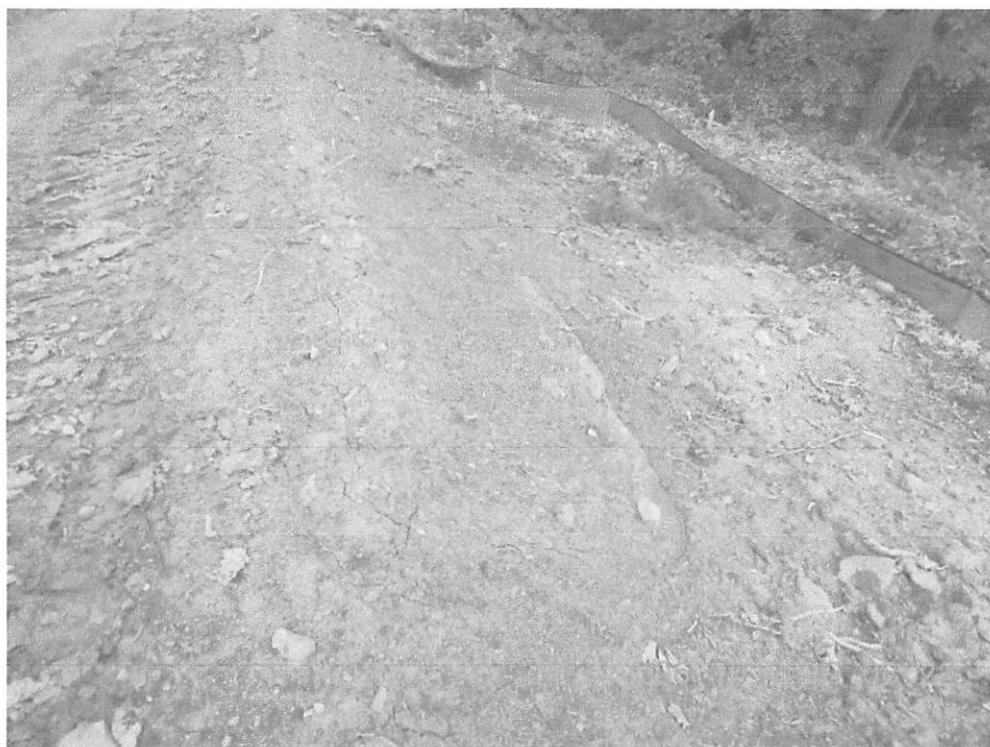
Station 220+50, Sumps needed maintenance.
