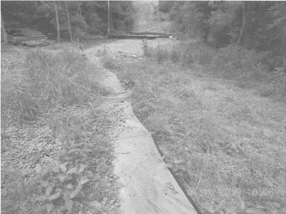
Station 311+00, Lack of controls had continued since the May 7, 2019 inspection.
