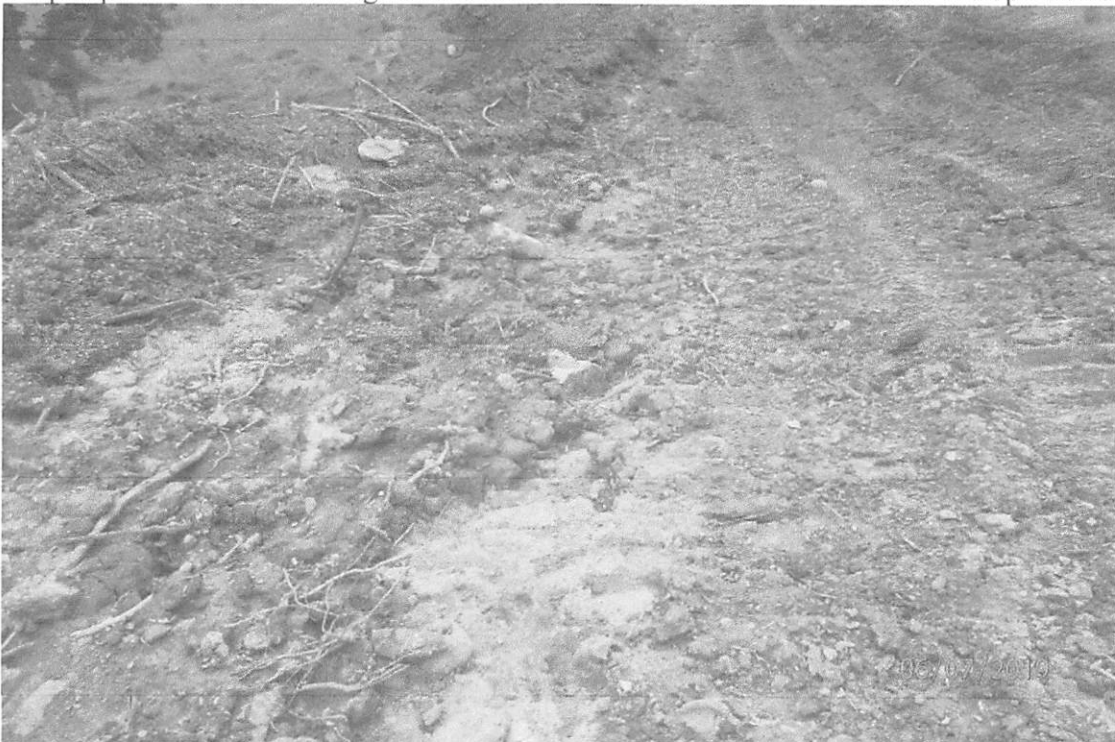
Hillside upslope of 490+00 showing the lack of installed water bars and silt saver 2 slope interceptors and the associated fill slope erosion.
