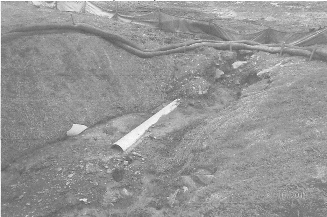
UNT – 14 showing area where groundwater from a coal mine opening flowed across the project area overwhelming the installed BMPs and causing deposits in the stream.
