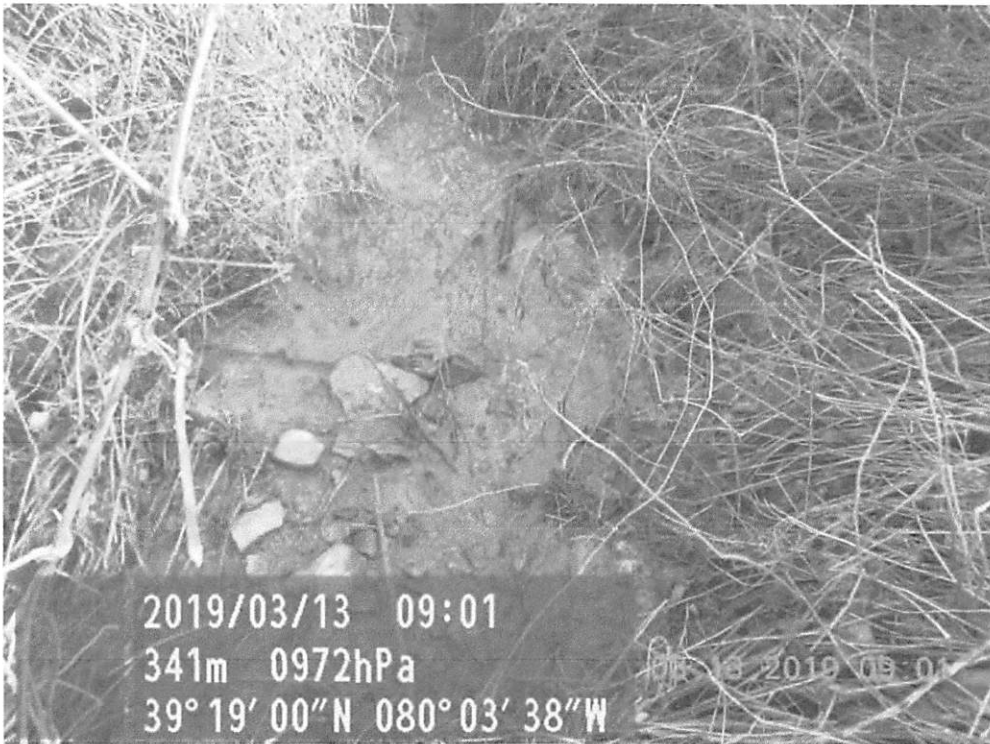
Stat. 156+00, UNT 17, Arsenal caused conditions not allowable in UNT of Shelby Run at 39°19'00" N 80°03'38" W
