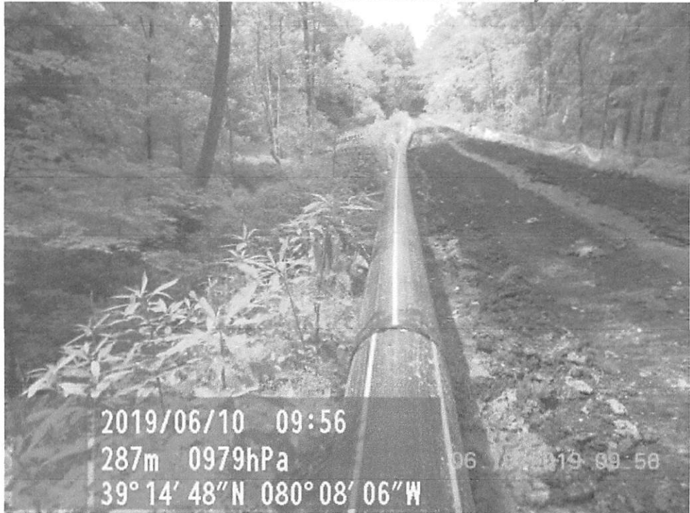
Station 317+00, Lack of controls had continued since the May 7, 2019 inspection.
