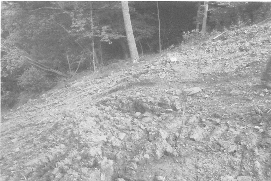
Waterbar in the Simpson Creek watershed that lacks waterbar terminus BMPs indicated in the approved SWPPP.
