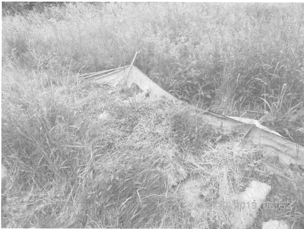
Station 193+00, P2 fence not functional.
