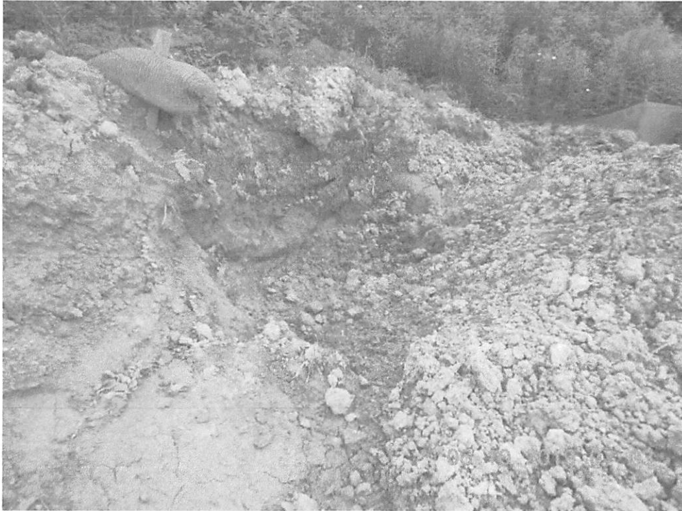
No water bar terminus treatment.
