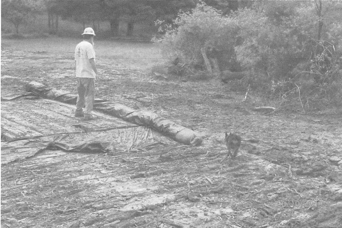
Wetland WL-28 showing an area where the approved SWPPP indicates the need for perimeter controls.
