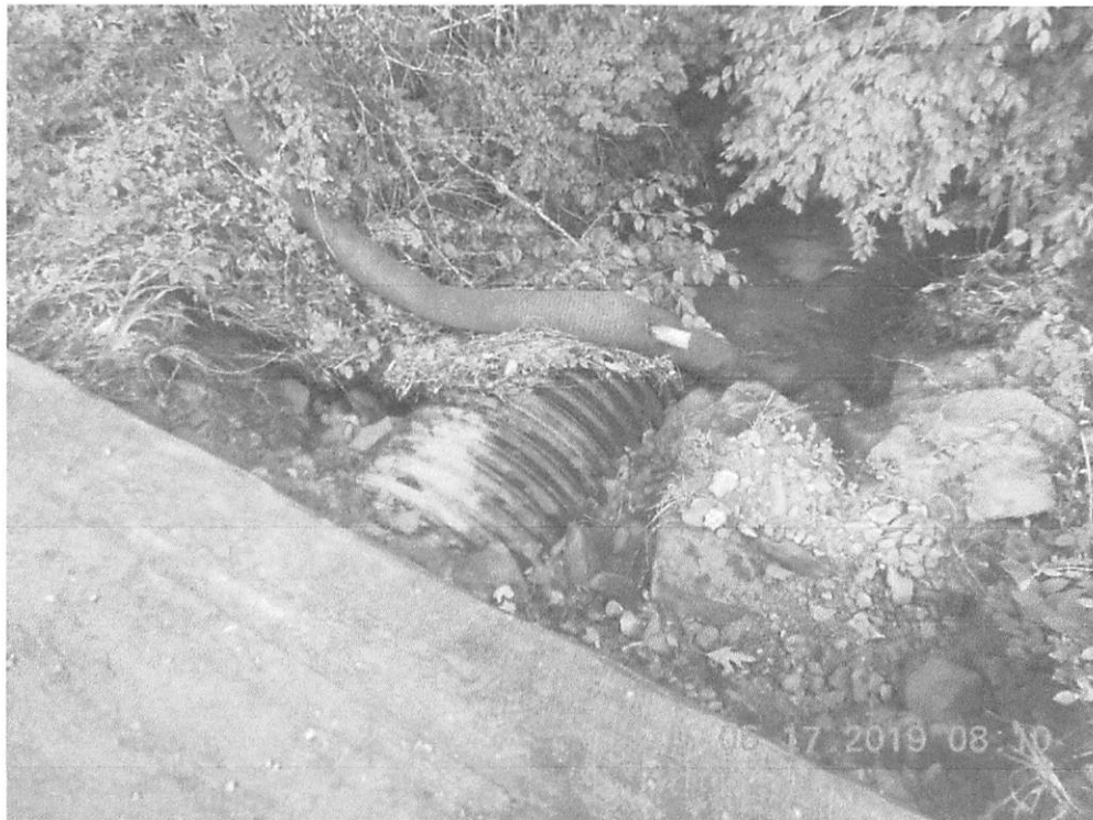
AR 5 construction entrance culvert overwhelmed.
