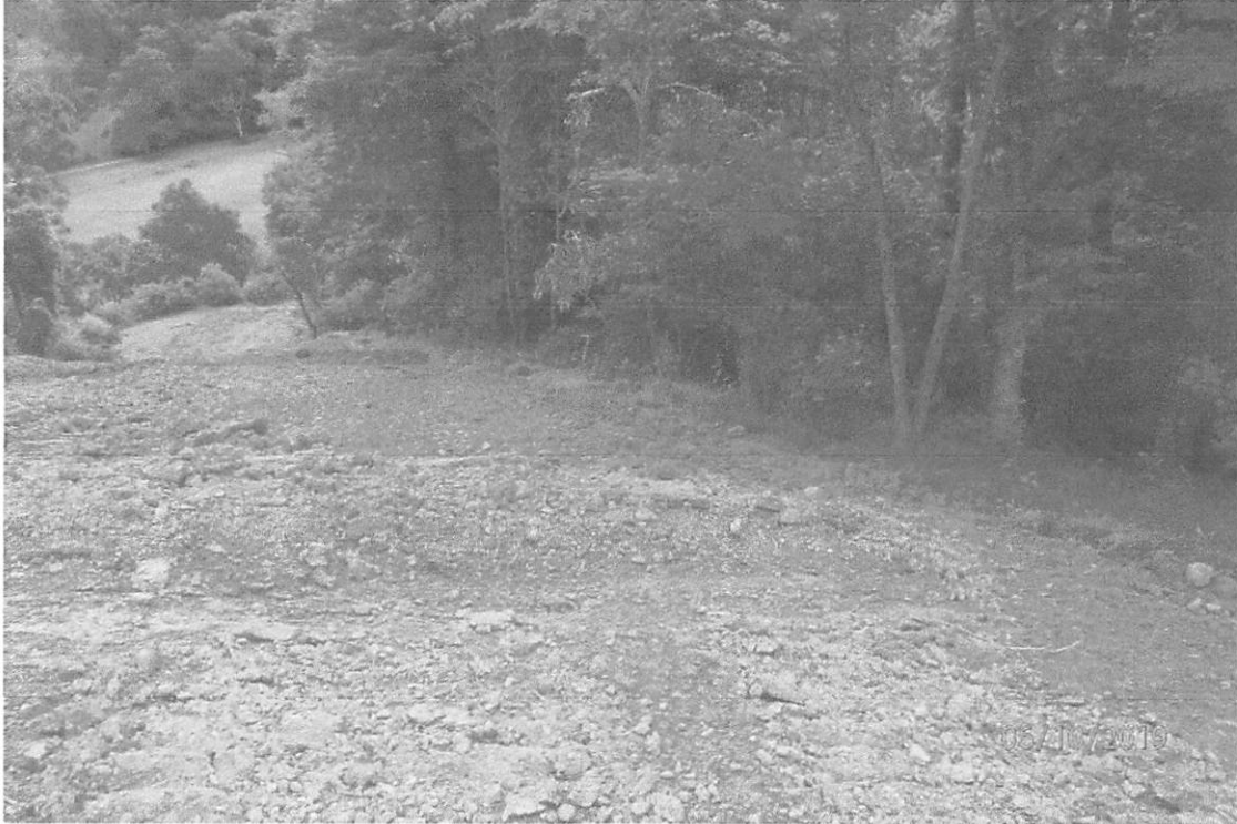
Waterbar in the Beards Run watershed that lacks waterbar terminus BMPs indicated in the approved SWPPP. Improperly installed waterbar (shallow height) pictured.
