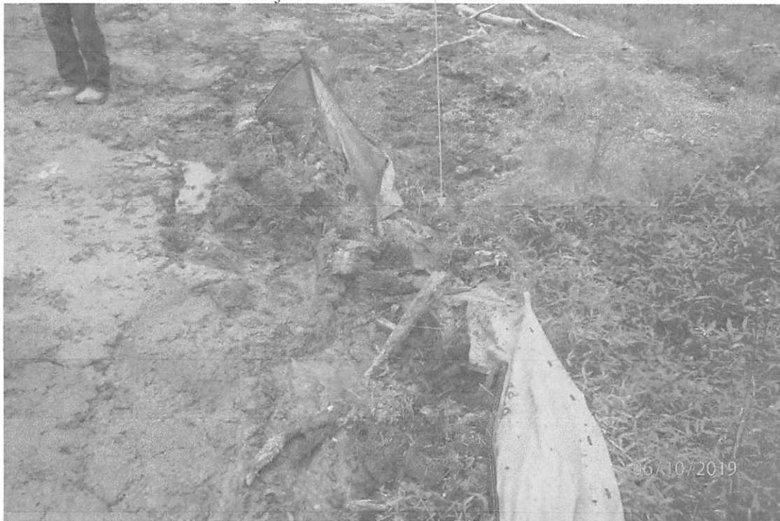
Perimeter control adjacent to WL-27 that is in need of maintenance.
