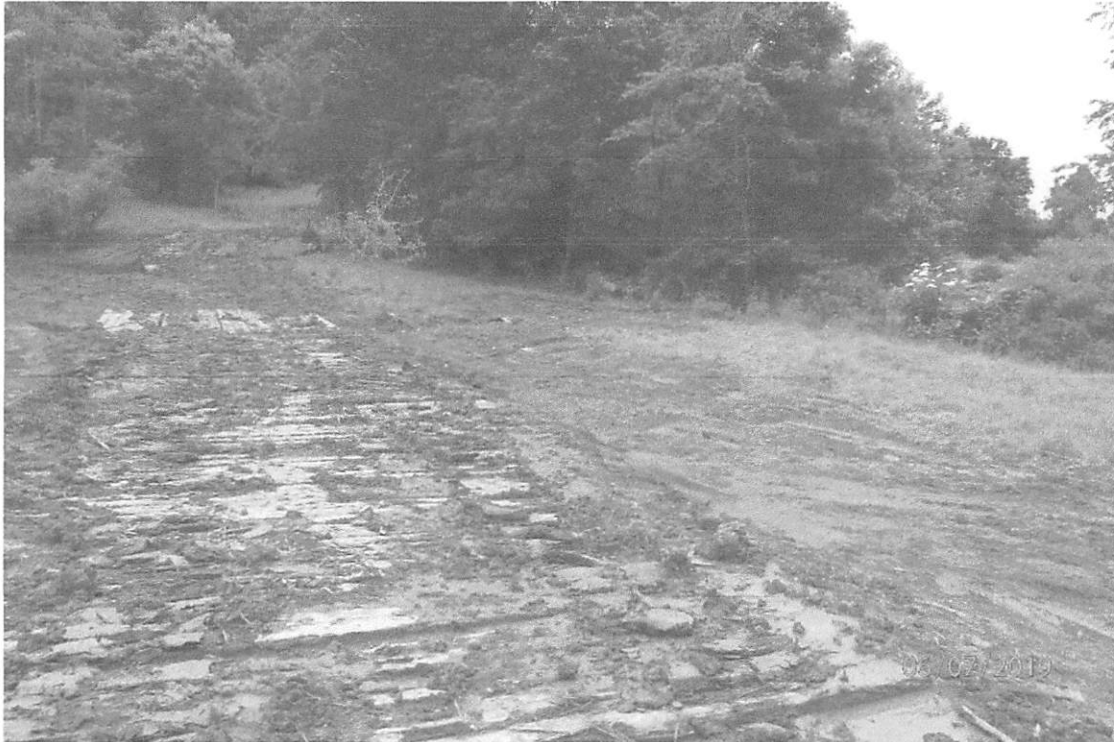
Wetland WL-28 showing the lack of installed perimeter controls that are indicated in the approved SWPPP.
