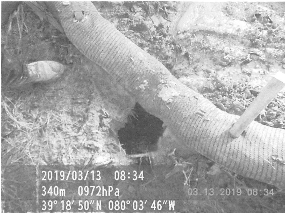
Stat. 164+00, CFS was not in contact with the ground, creating a bypass, allowing sediment laden water to leave site.
