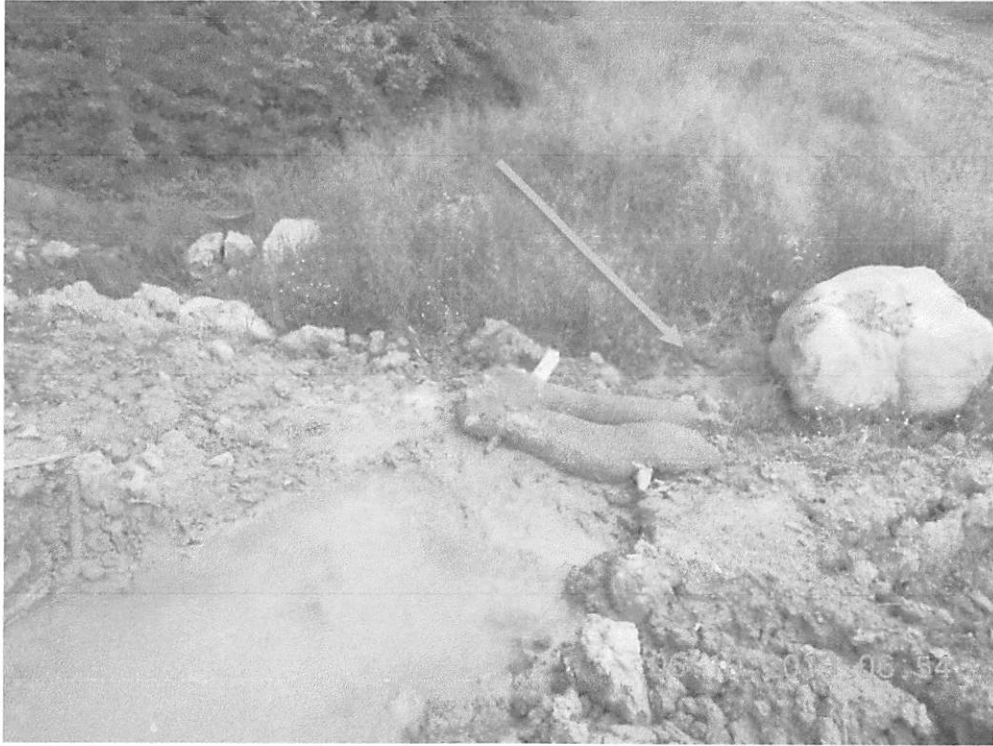
Station 192+00, Water bar terminus BMP not properly implemented, allowing sediment laden water to leave site.
