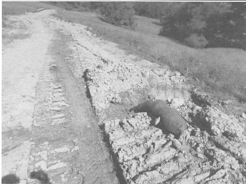
Station 274+00, SWPPP requires SS2 slope interceptors.
