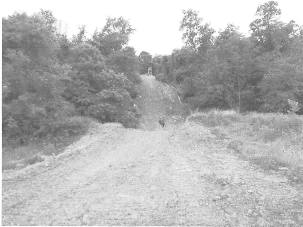
Station 192+50 to 195+50, 6 water bars should be installed with terminus treatment.
