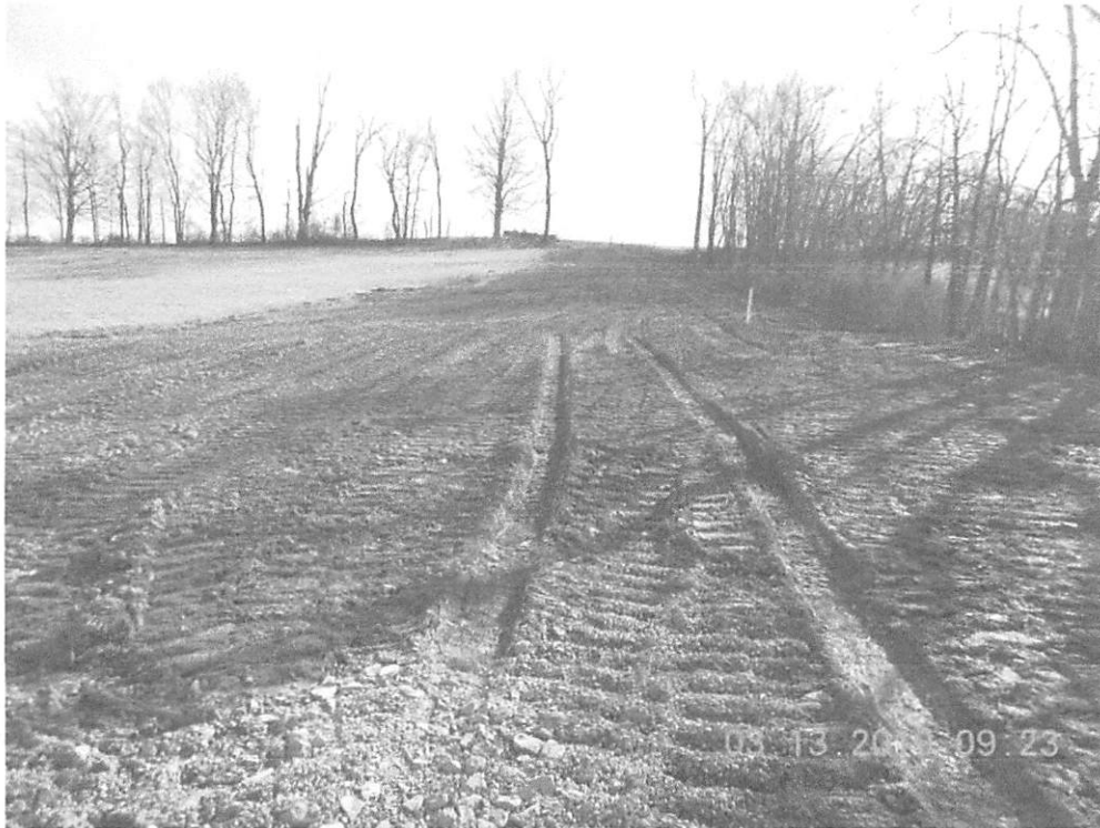
Stat. 142+00, Water bars were not installed as indicated in the SWPPP.
