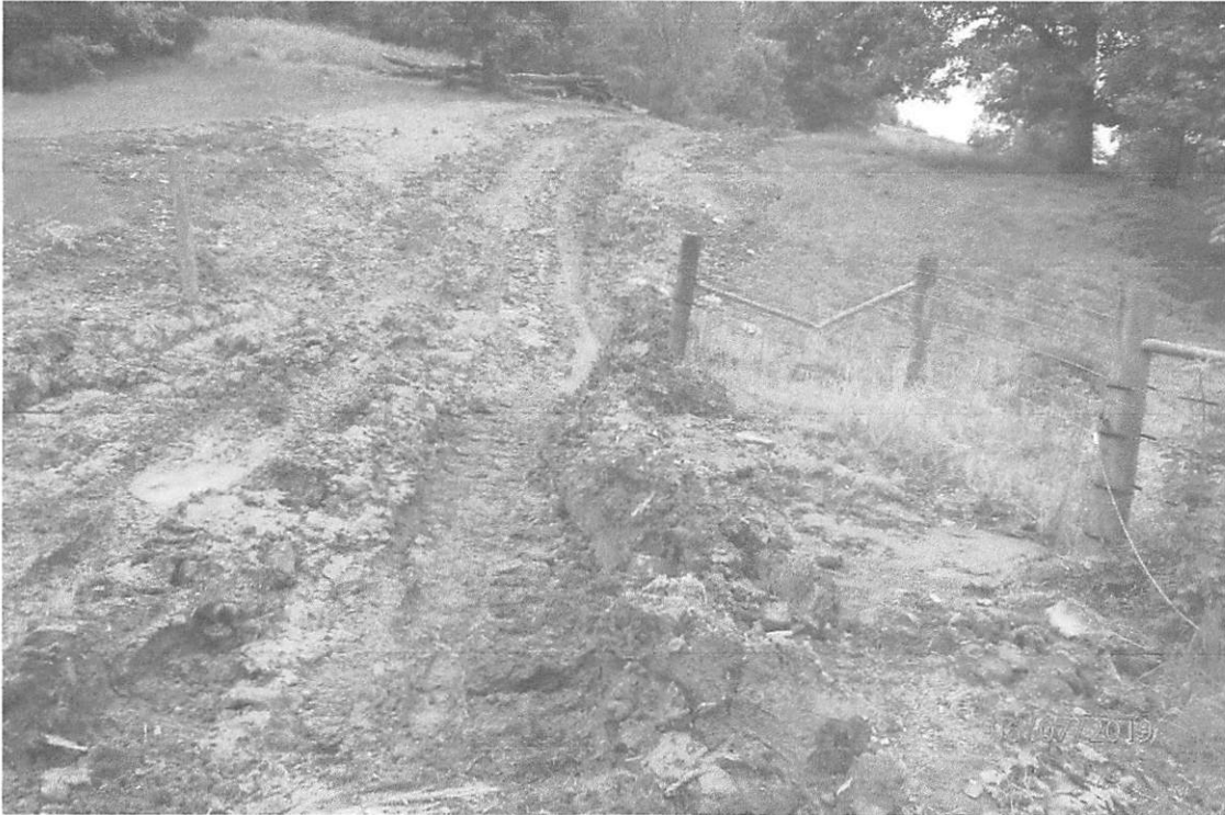
Project area adjacent to 482+85 showing the lack of installed silt saver 2 indicated in the approved SWPPP. The area past the fence is where a stream of run on stormwater is flowing across the project and the plan has not been modified to adequately handle the flow.
