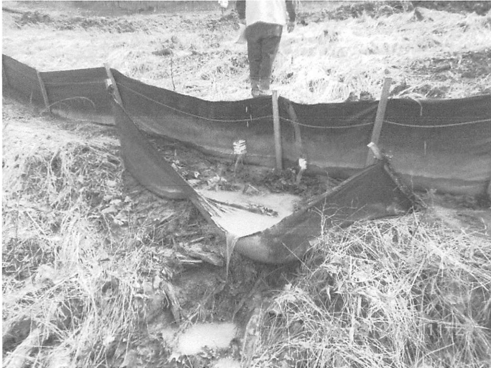
Maintenance is lacking throughout project site.
