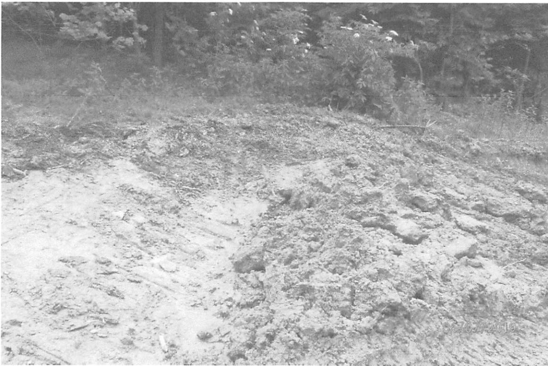
Improperly installed water bar upslope of 479+00. The water bar allows stormwater to flow back across the right of way. The water bar also lacks outlet treatment.
