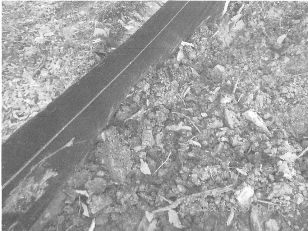
Stat. 213+75, SF not toed-in correctly.
