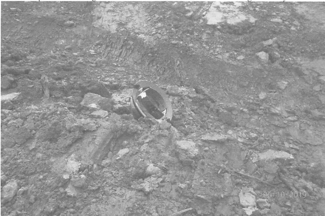
Improperly installed waterbar in the Beards Run watershed that is less than 12 inches high on the uphill side.
