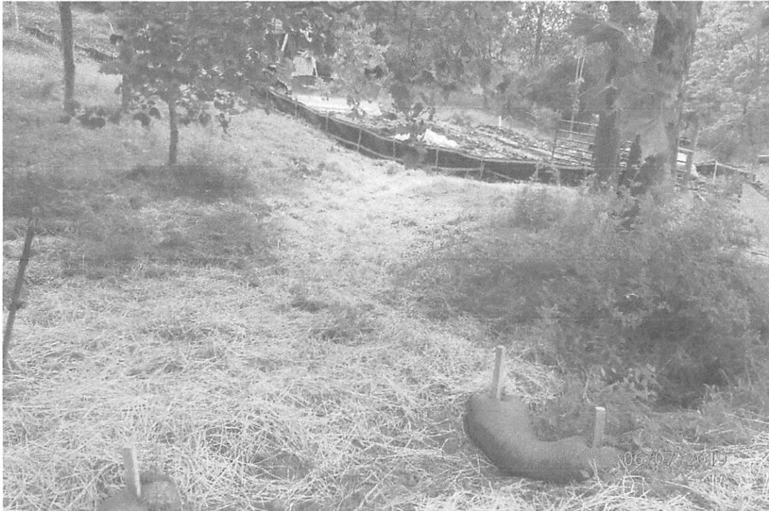
Offsite sediment deposits as a result of improperly installed water bars leading to the old CR 17 conveyance. Perimeter controls were recently installed in this area as well.
