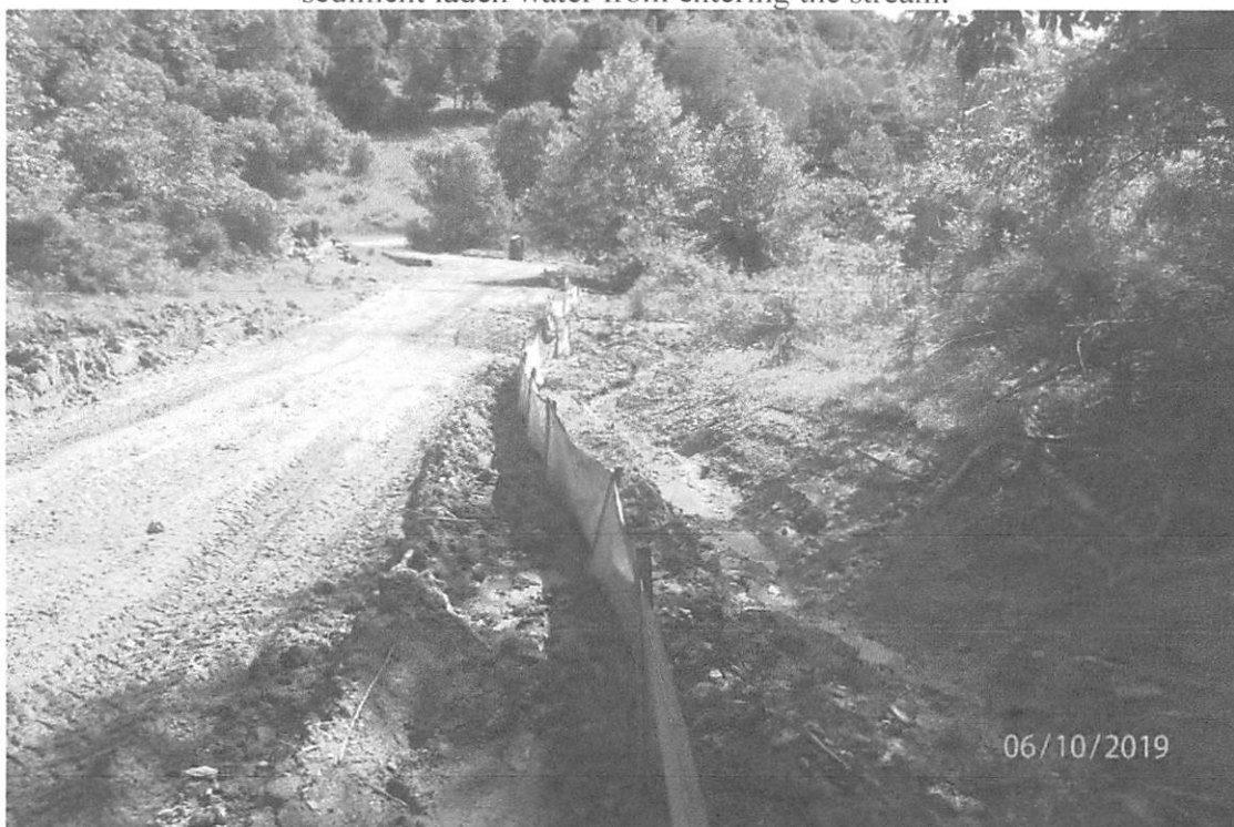
Access Road 7 showing the lack of a stabilized surface as indicated in the approved SWPPP.
