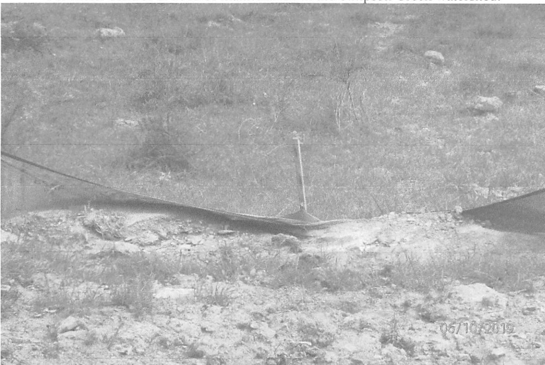
Perimeter control in need of maintenance in the Simpson Creek watershed.
