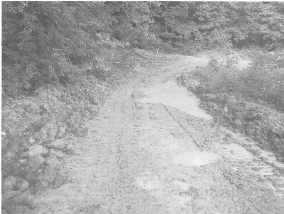
Ditchline from WL 8 along AR 5 is pinched shut.
