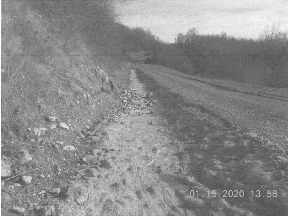
Rolling debris from unstable area above concrete slurry diversion ditch.
