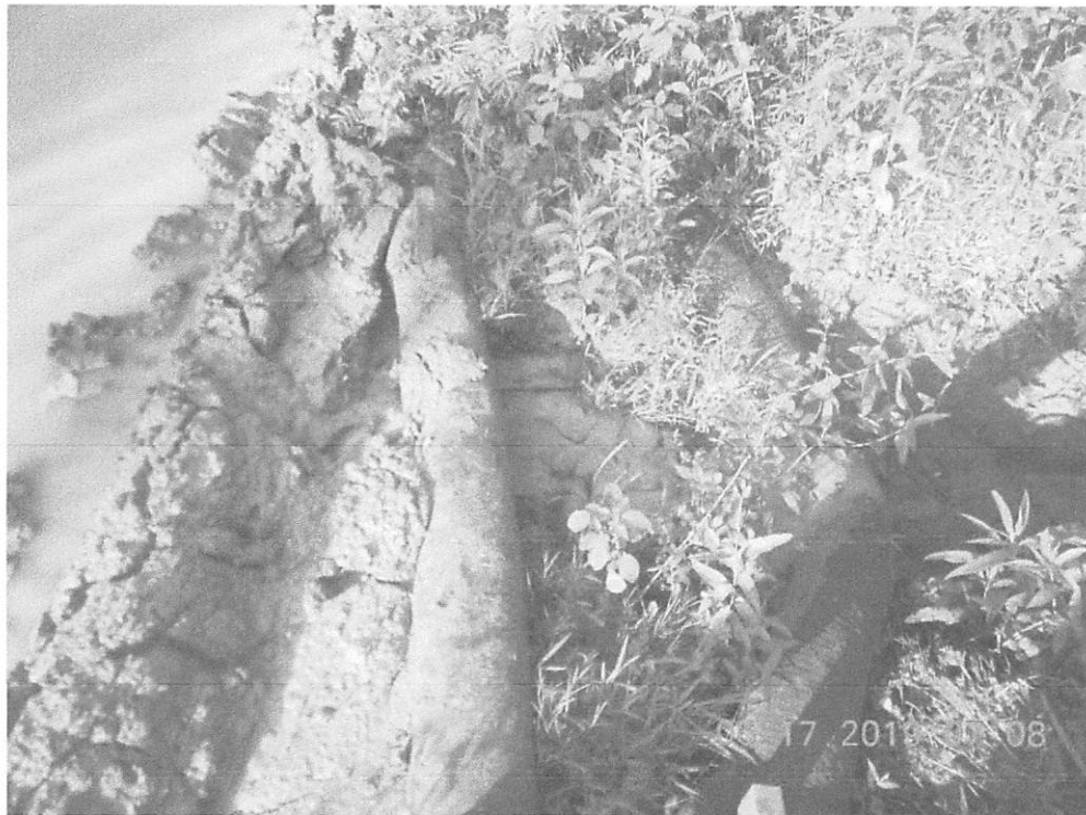
Sediment laden water entered the UNT of Simpson Creek at the mud hole that developed at the culvert where controls were not being maintained.
