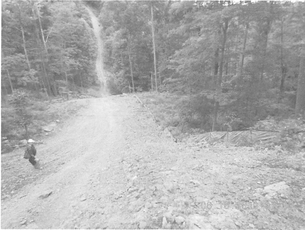
Station 207+00 to 211+00, SWPPP indicates 9 water bars with terminus treatment.
