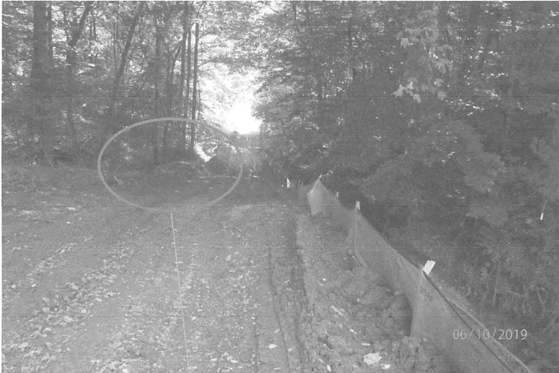
Access Road 7 showing the lack of a stabilized surface as indicated in the approved SWPPP. Area on the left lacking the perimeter controls indicated in the approved SWPPP.
