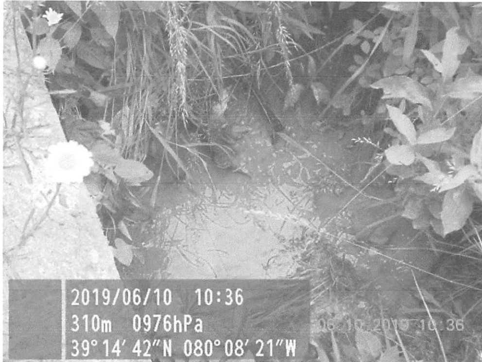
Sediment deposit on bottom of Rt. 76 conveyance caused conditions not allowable on the bottom of UNT of Simpson Creek (39° 14' 42'' N, 80° 08' 21'' W).
