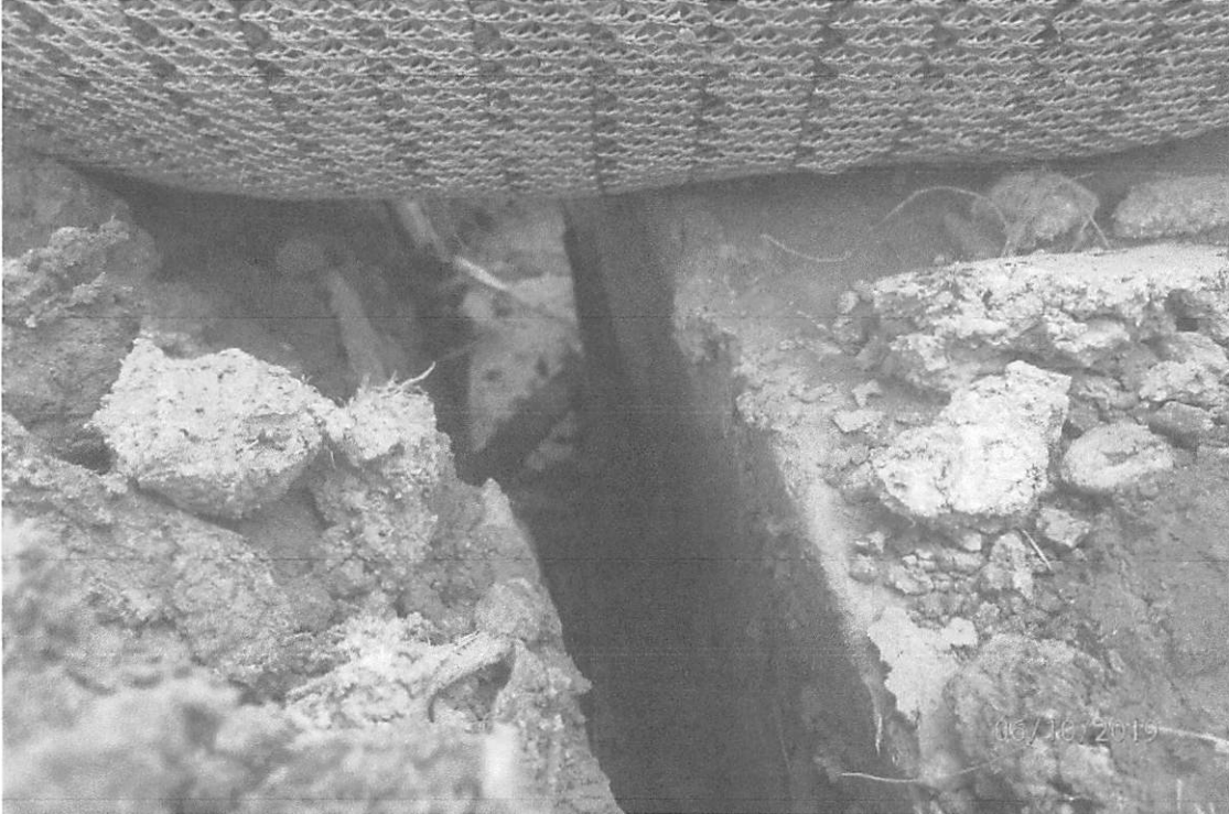
Improperly installed temporary bridge BMP at the UNT 23 crossing.
