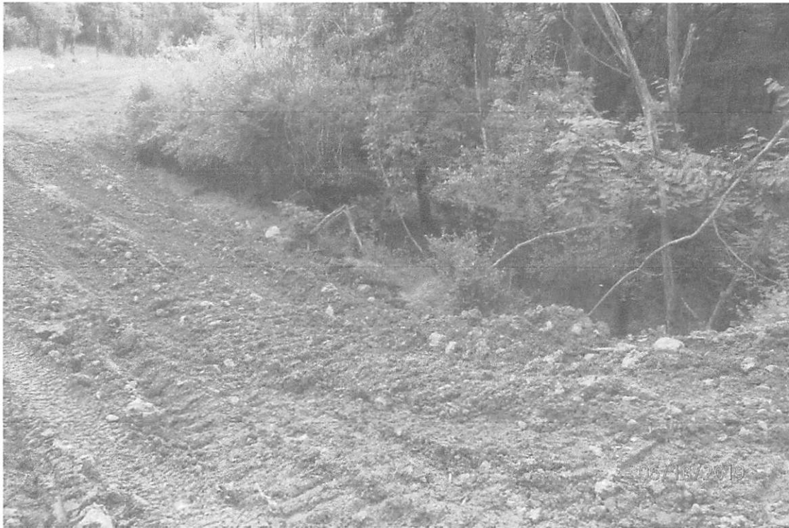
Project area showing the need for additional perimeter controls not indicated in the approved SWPPP adjacent to 467+00.
