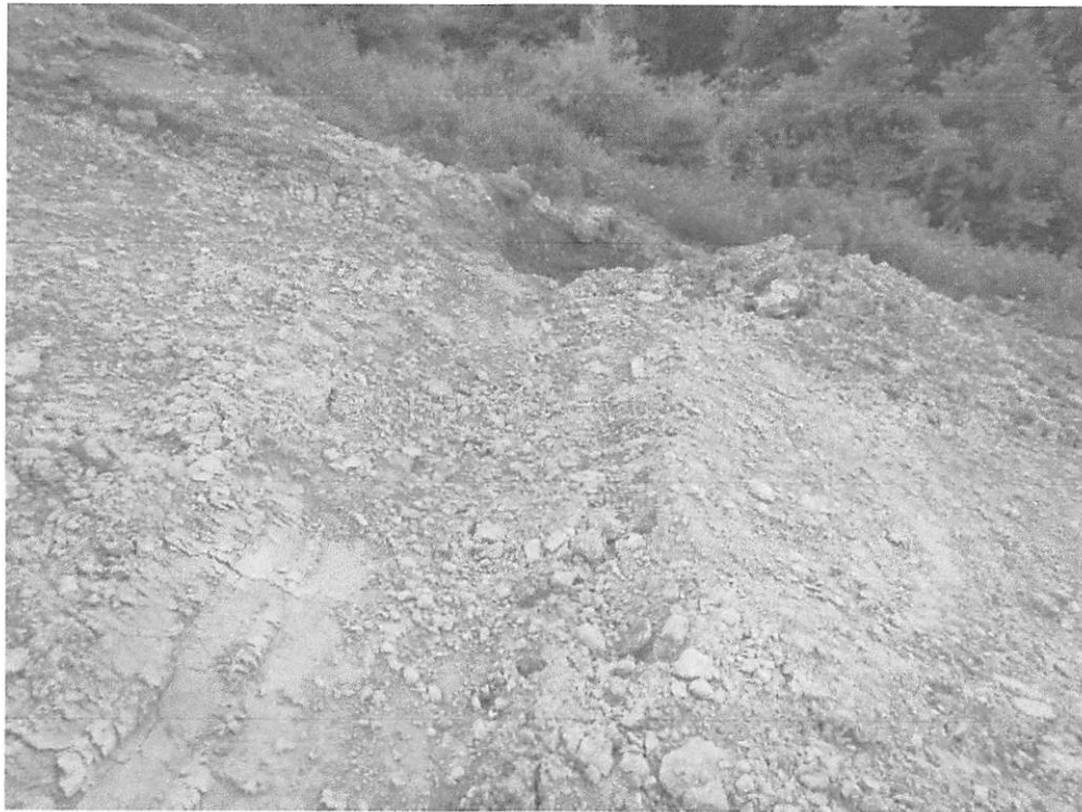
Station 192+00, Water bar terminus BMP not properly implemented, allowing sediment laden water to leave site.
