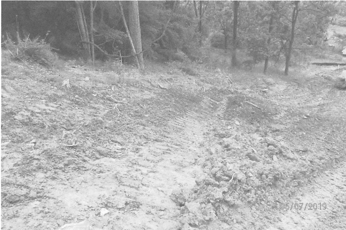
Improperly installed water bar upslope of 479+00. The water bar is installed at a steep angle and has a height less than 12". The water bar allows stormwater to flow back across the right of way. The water bar also lacks outlet treatment.
