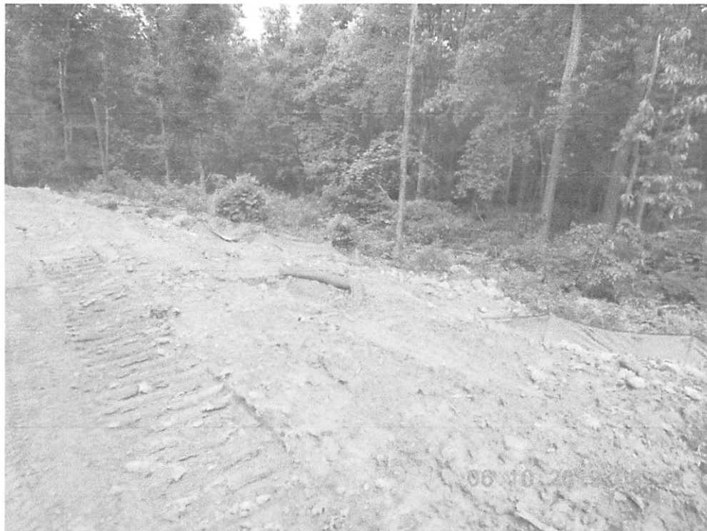
Station 220+00, Bypasses of perimeter controls.
