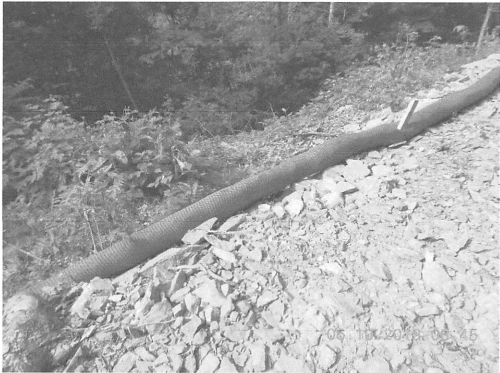
Bypasses in perimeter controls (Station 245+00).
