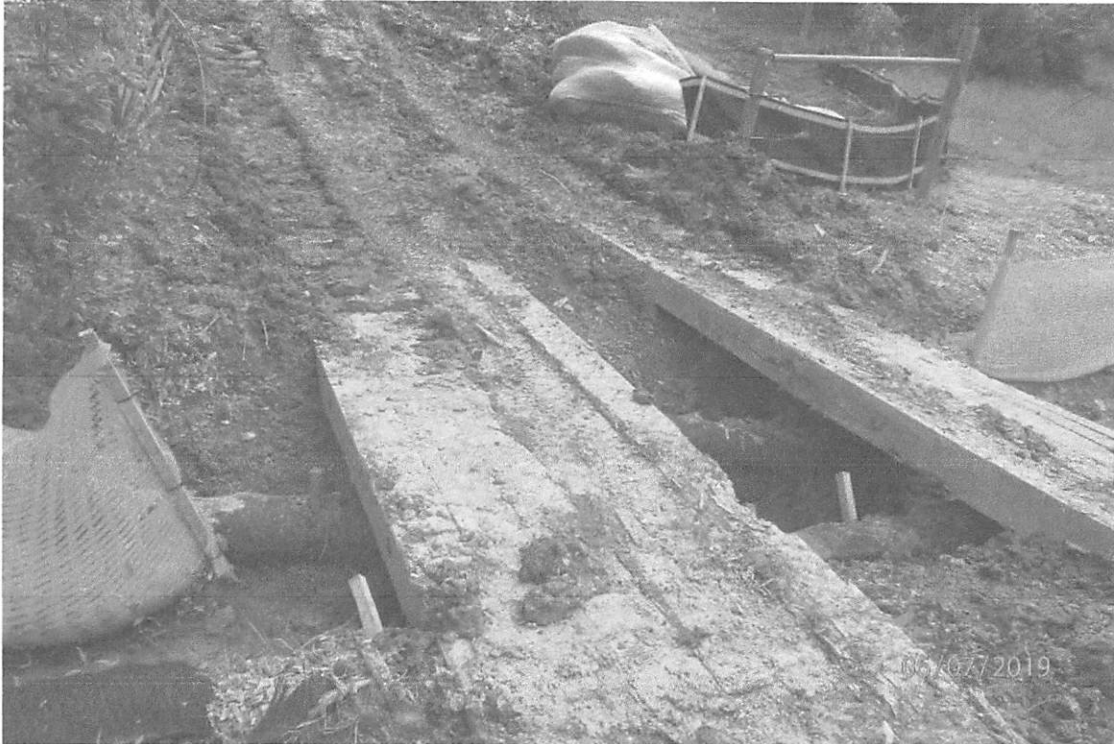
Timber mat crossing of UNT Beards Run conveyance of old CR 17 showing the lack of protection.
