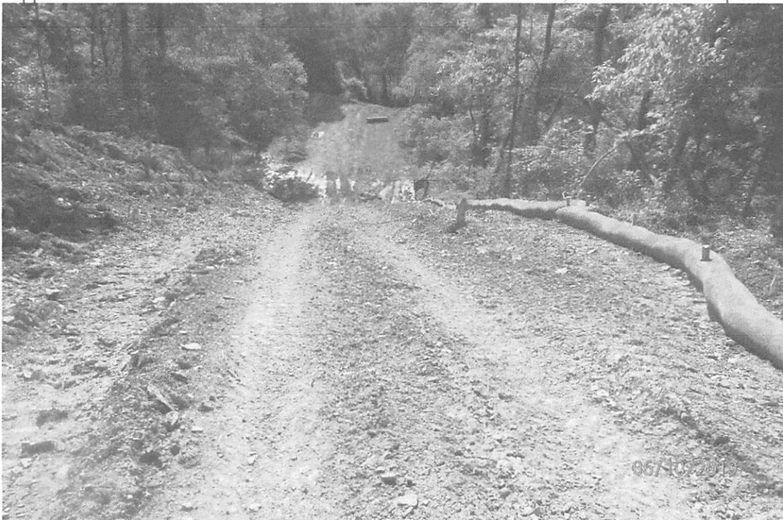
Project area upslope of 433+50 showing the lack of waterbars indicated in the approved SWPPP. The approved SWPPP indicates that 6 waterbars should be installed, but none were in place.
