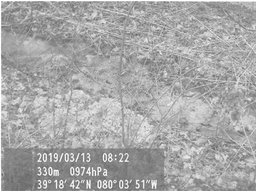
Stat. 175+25, Barnett Road Conveyance, Arsenal caused conditions not allowable in UNT of Shelby Run at 39°18'42" N 80°03'51" W
