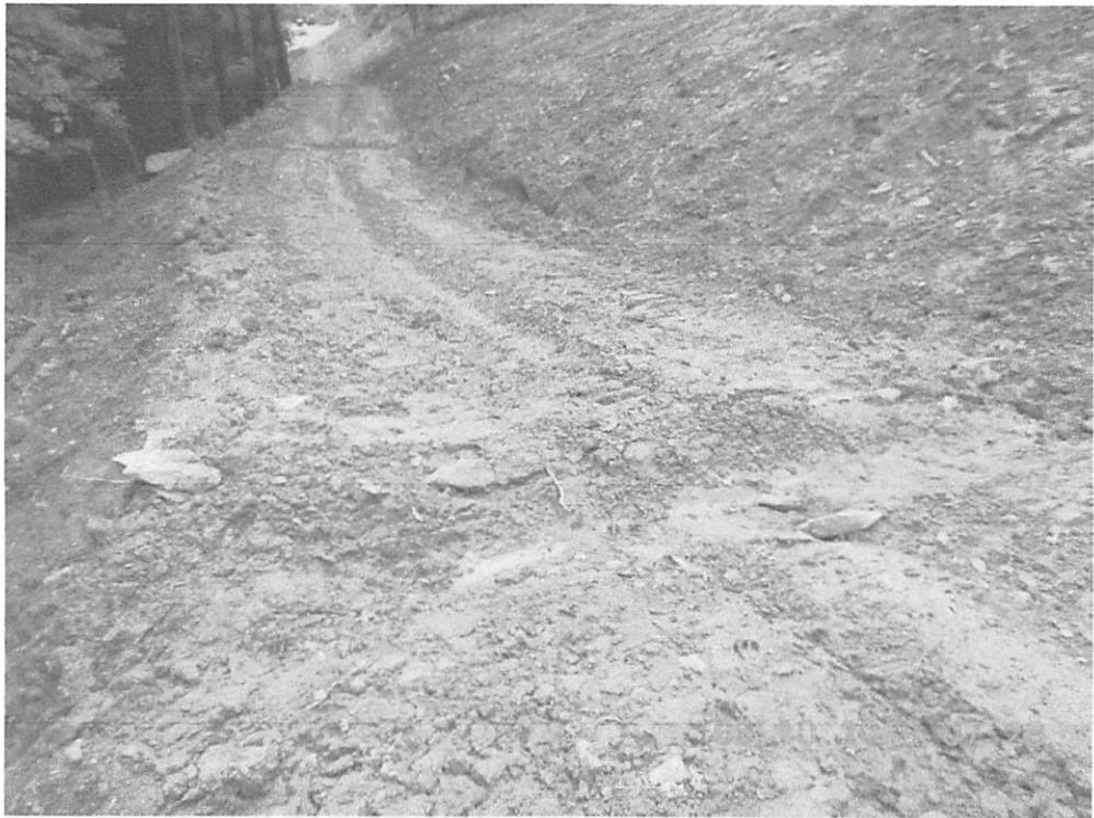
Station 205+00, Water bars with no terminus treatment installed.
