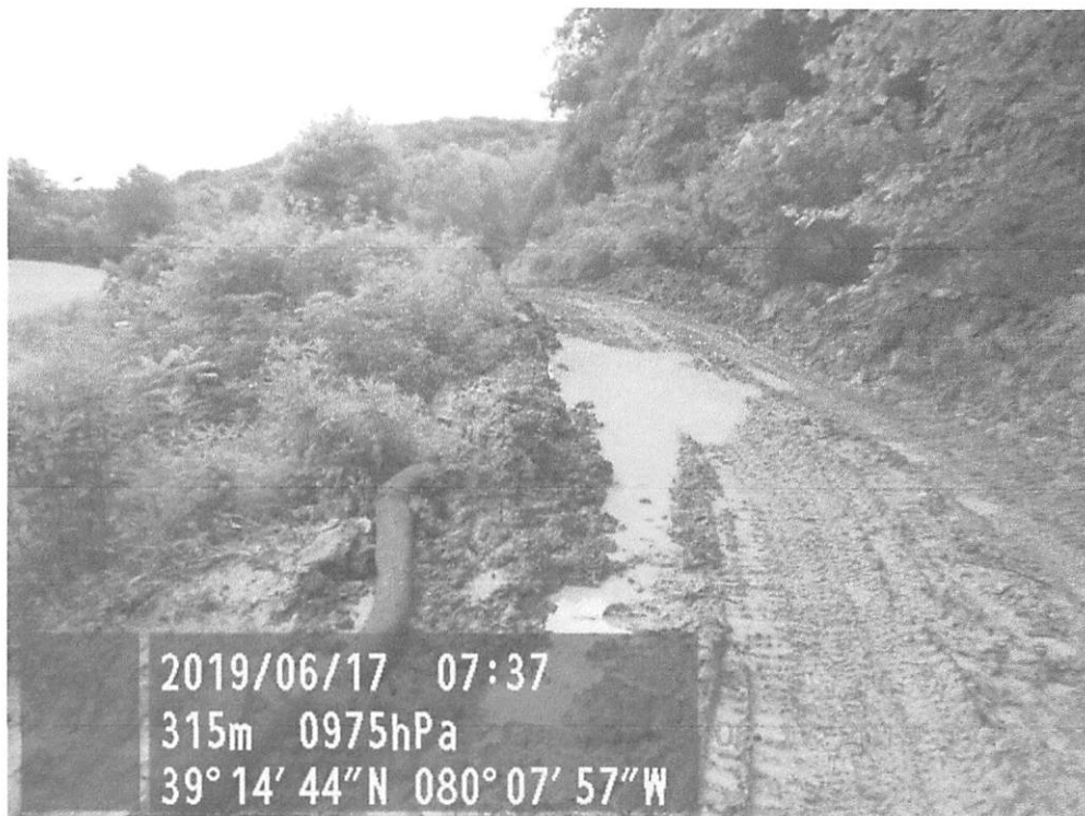
Controls overtopped by sediment on AR 5.
