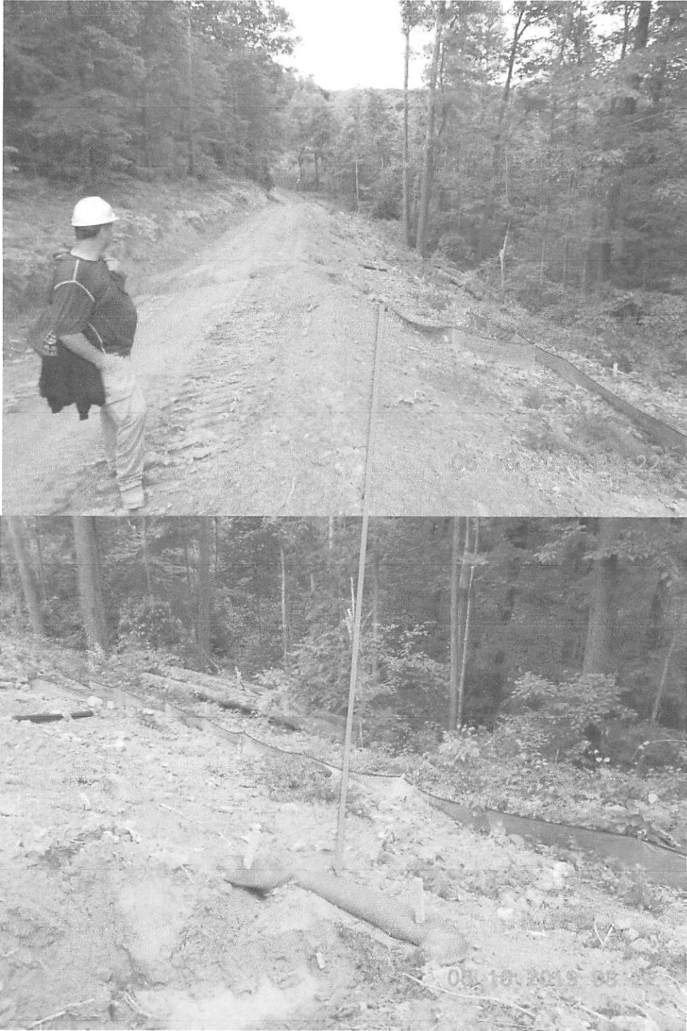
Station 223+00, bypass of terminus treatment. Maintenance needed on sump and perimeter controls.
