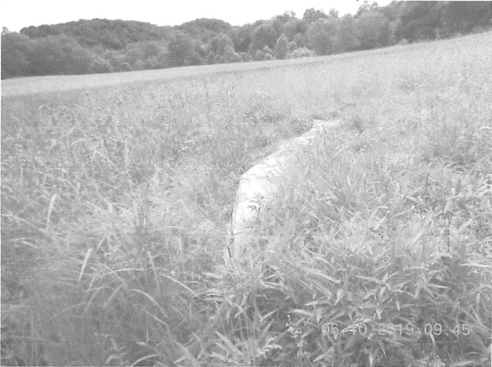
Controls continued to be down since the May 7, 2019 inspection.
