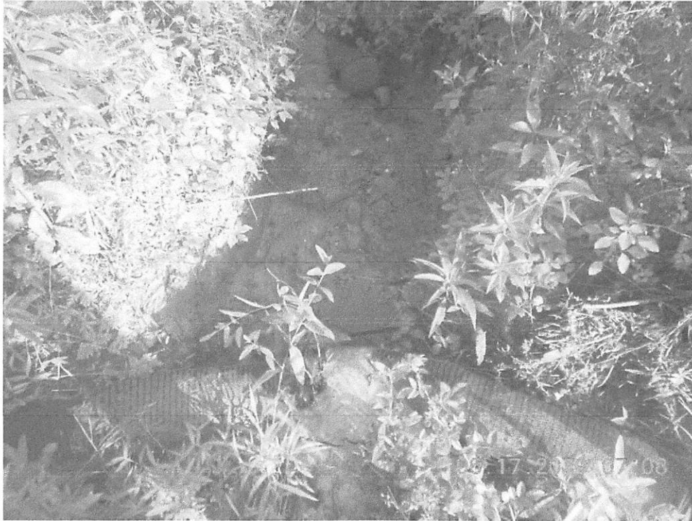
Culvert tail of UNT of Simpson Creek.
