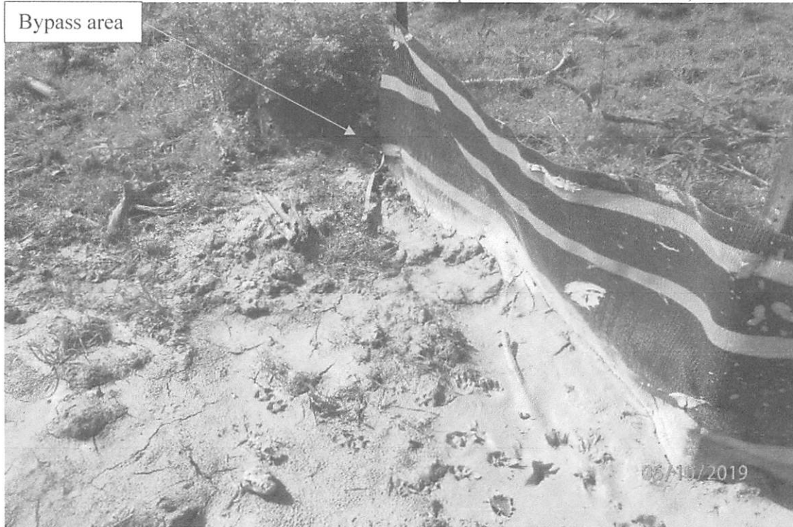
Improperly installed perimeter controls (no J-Hook) adjacent to 433+50, showing accumulated sediment deposits as a result of the lack of installed waterbars upslope of this location. Area of sediment laden water bypass.
