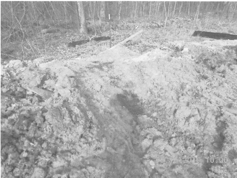
Stat. 112+00, Water bars terminus treatment was not implemented as detailed on page ENV D12 of the SWPPP.
