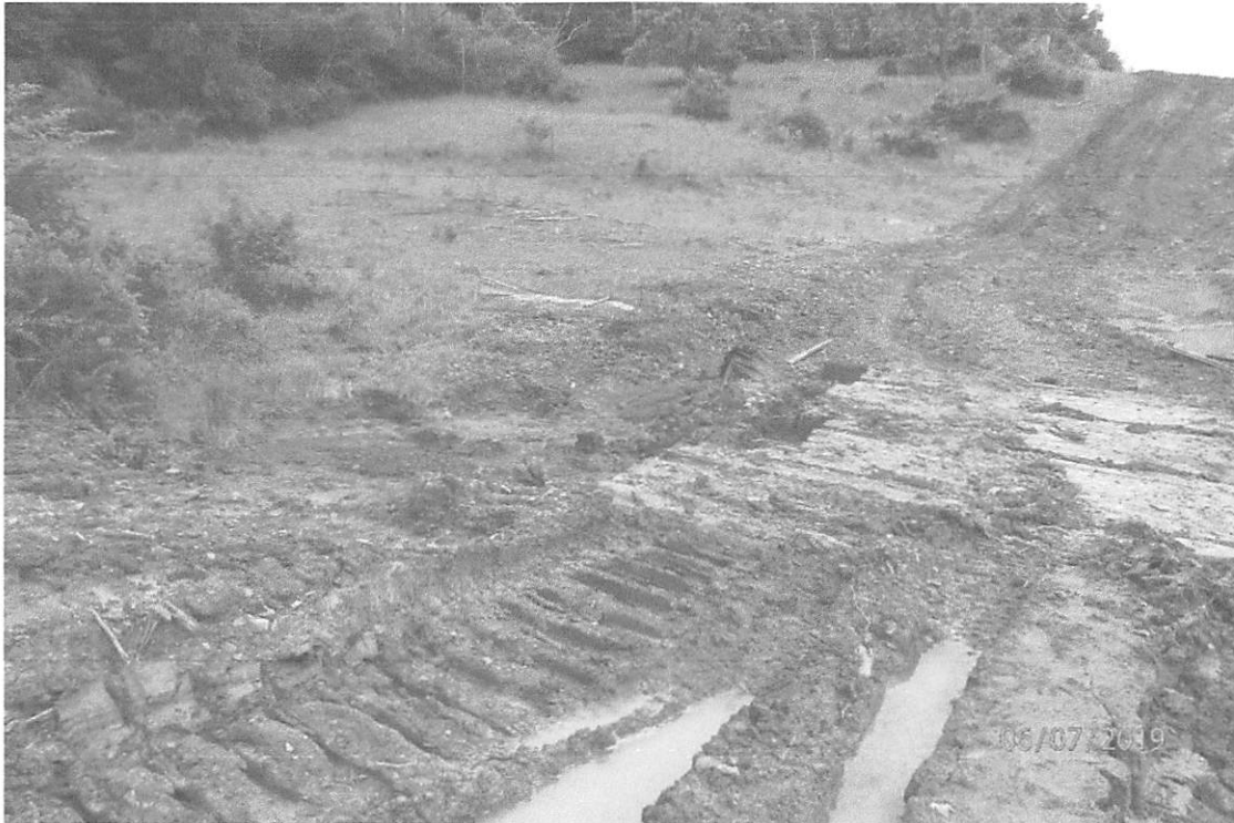
Installed timber mat crossing of UNT 23 showing its improper installation and need for maintenance.
