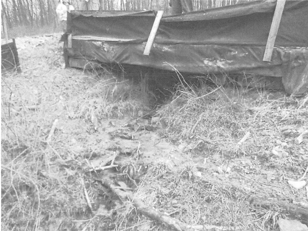
Failed to properly implement geo-wrap and perimeter controls on bridge at UNT 29, UNT of Otter Run, allowing sediment laden water to leave site and create sediment deposits on bottom of UNT of Otter Run.
