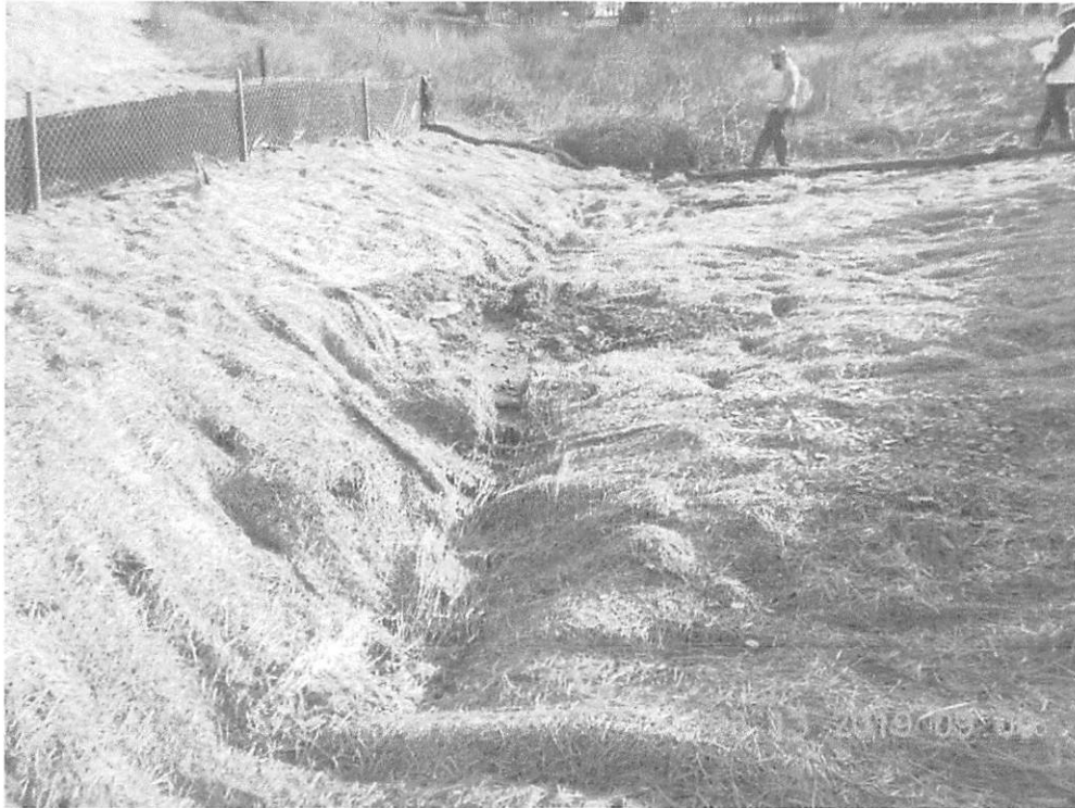
Stat. 156+00, UNT 17, Maintenance is lacking throughout project site.
