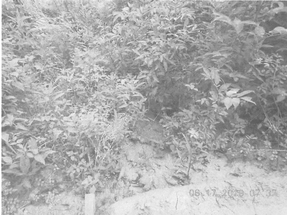
Culvert trail for WL 8 on AR 5. Maintenance needed on perimeter controls. Sediment deposited off LOD.
