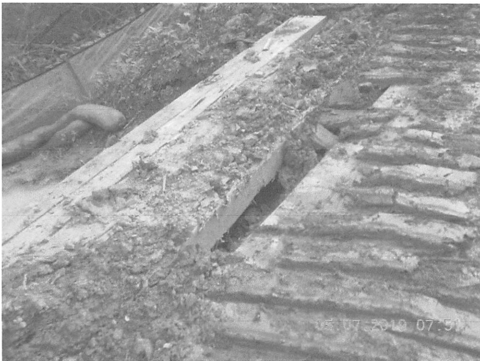
Bridge that was installed at Station 211+00 for UNT of Gabes Fork.
