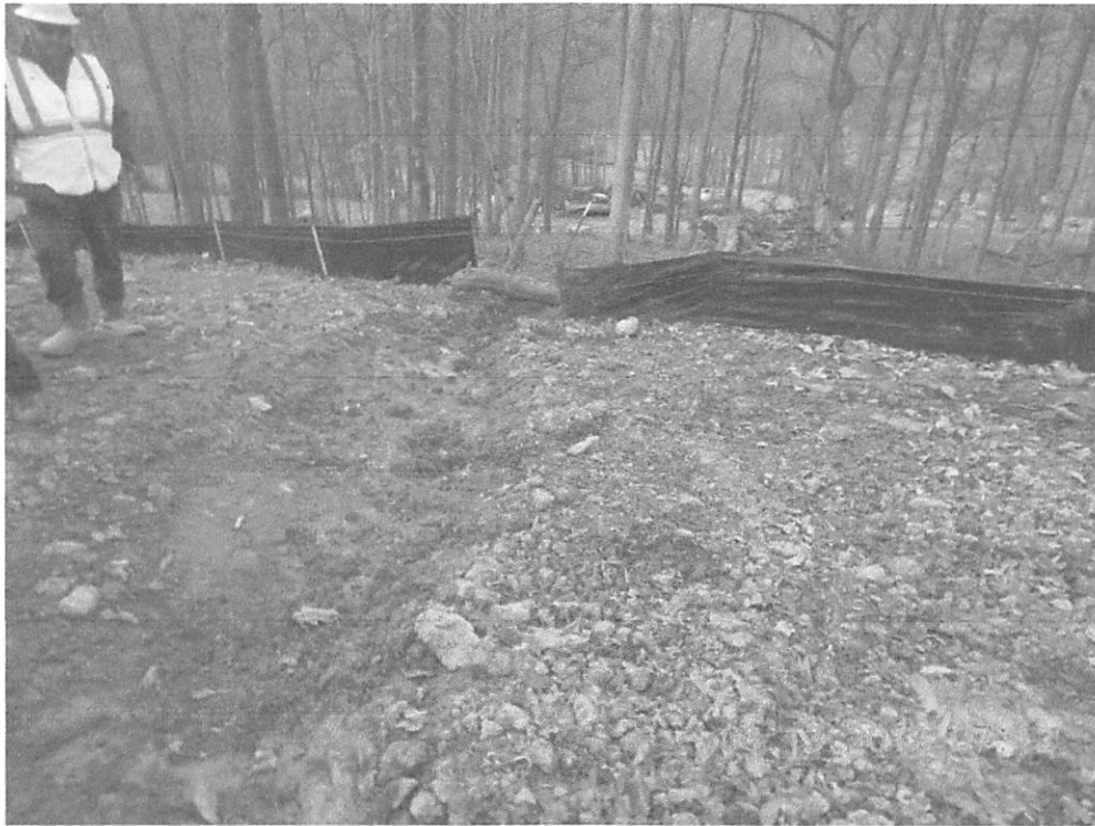
Stat. 218+00, Failure to implement water bar terminus treatment as detailed on page ENV D12 of the SWPPP.
