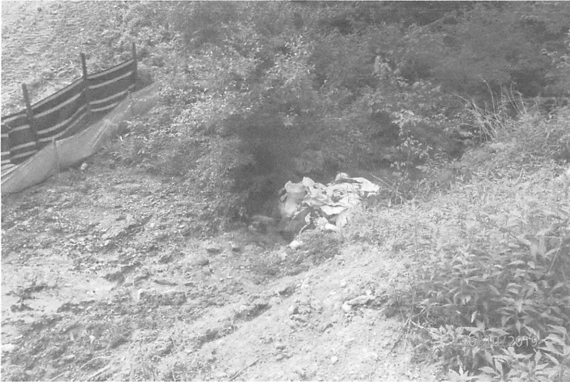
Instream solid waste in UNT 21 as a result of the contractor leaving the sand bag coffer dam in the stream after the stream crossing was completed.
