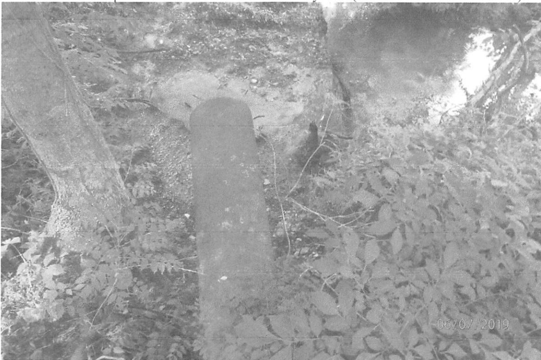
Offsite CNA deposits in Beards Run at the culvert outlet downslope of UNT Beards Run conveyance (39° 15.023' X 80° 10.561').
