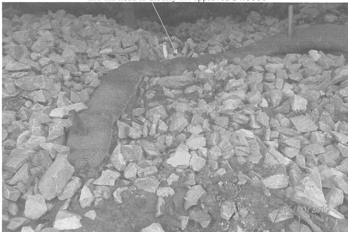
Improperly installed secondary compost filter sock BMP that was placed on large stone and allowed sediment laden water to bypass under the device. BMP and stone are placed off-site and in-stream at UNT Simpson Creek.
