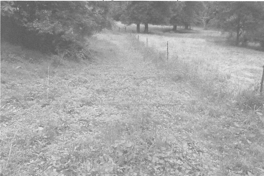
Offsite sediment deposits adjacent to 482+00 as a result of the lack of installed BMPs.
