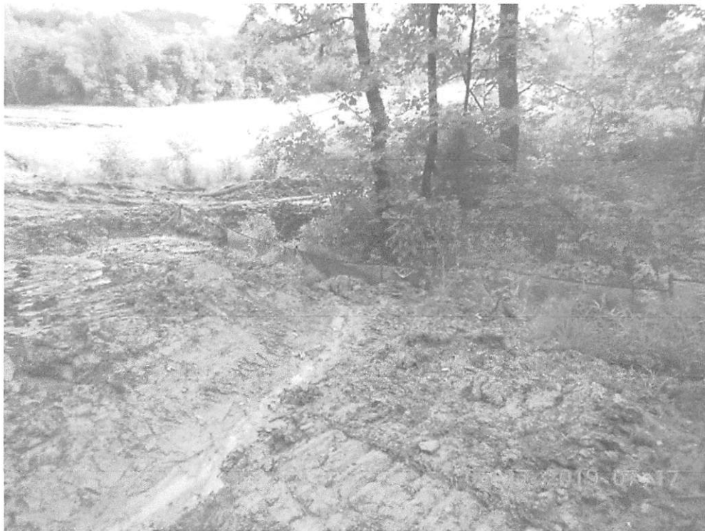
Water bars did not have proper terminus treatment, as indicated in the SWPPP, along with SS2 slope interceptors.
