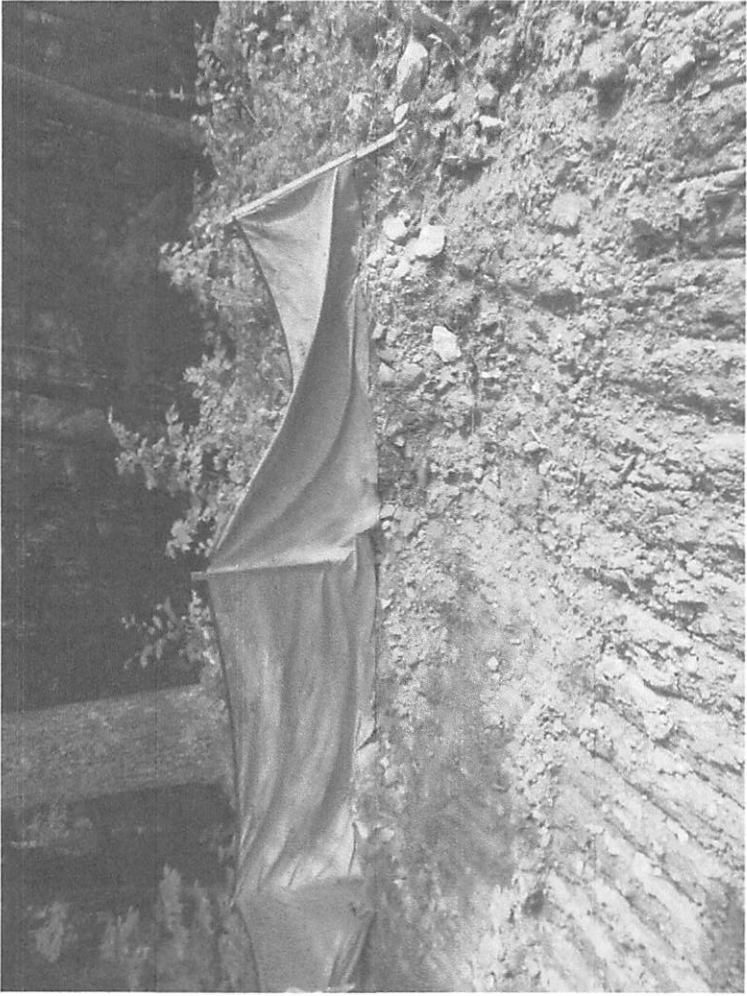
About Station 246+00, perimeter controls in disarray, holes in fabric, and SS2 not toed-in correctly.
