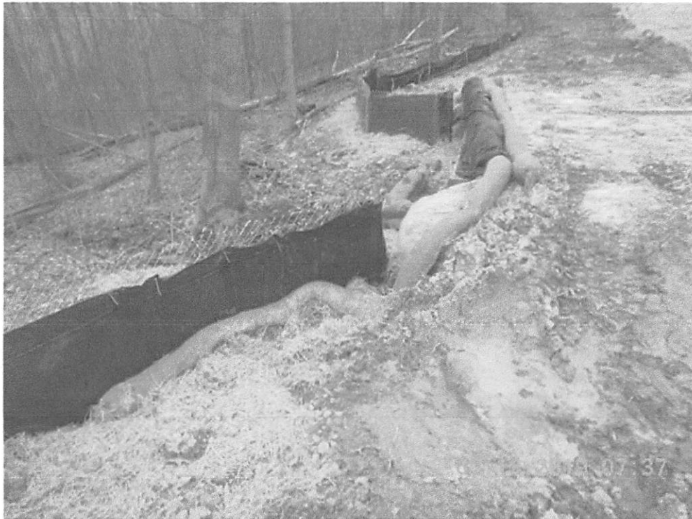
Stat. 210+00, Perimeter controls tied-in to bridging controls that had bypasses.
