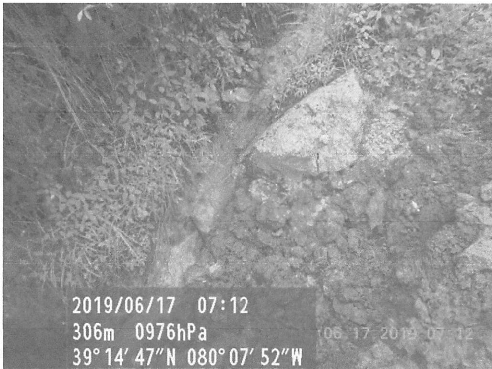
Conditions not allowable in the form of sediment deposits on the bottom of UNT of Simpson Creek (39°14'47"N, 80°07'52"W) resulting from roll-out off AR 5 in multiple locations.
