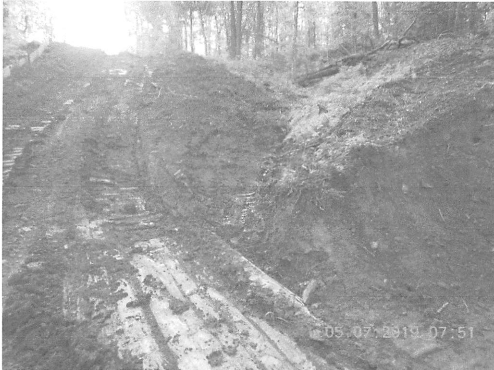
Station 211+00, unidentified UNT of Gabes Fork.
