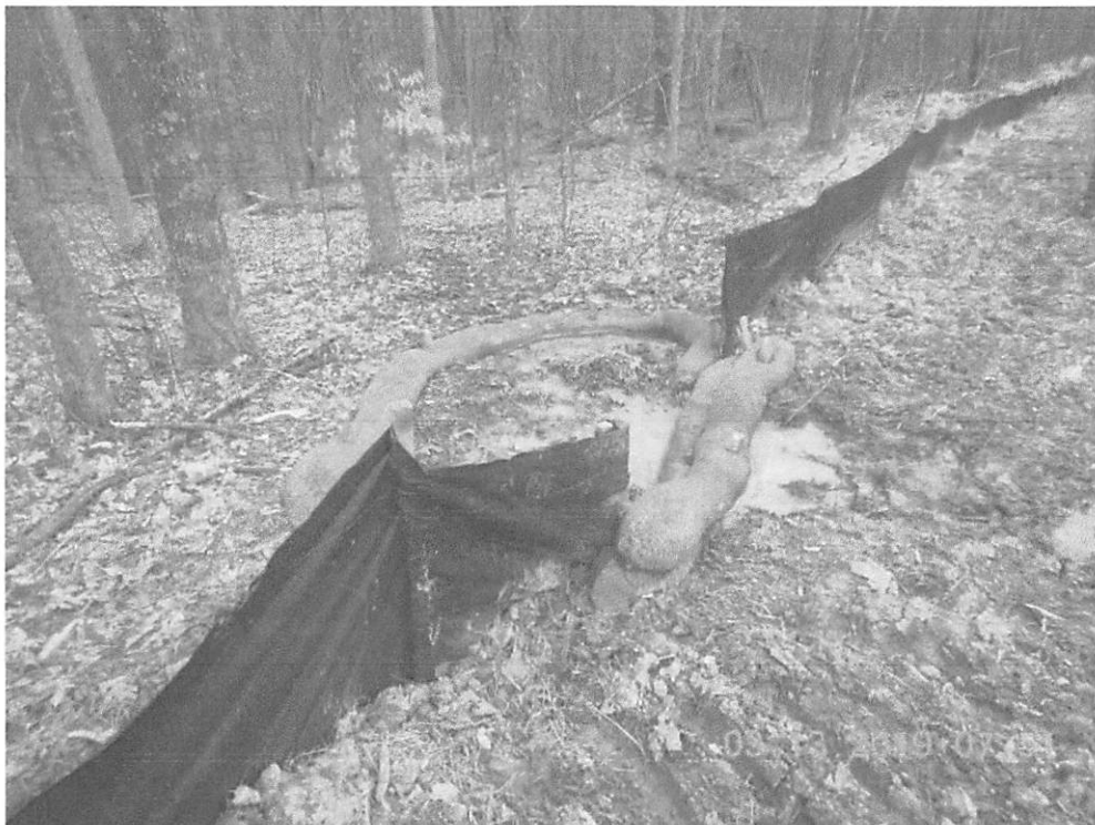
Stat. 192+75, CFS was not conjoined with SF correctly, creating a bypass. CFS was not in contact with the ground, creating bypasses.
