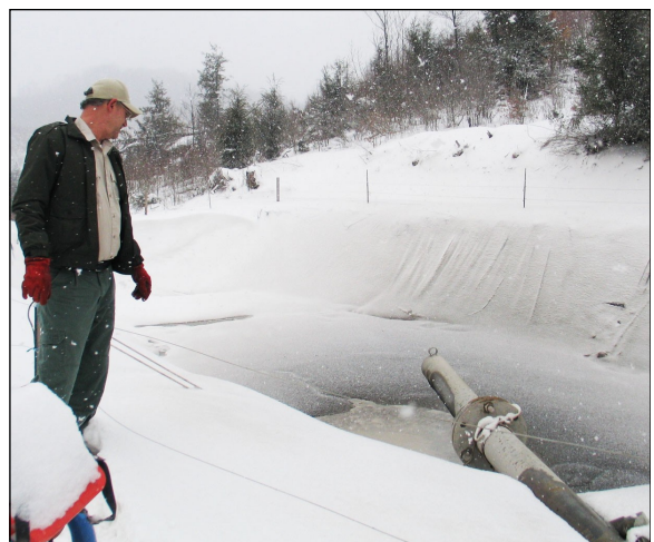
Gilbert takes a look at a pit constructed to collect waste materials at a Nicholas County gas well drilling site.
