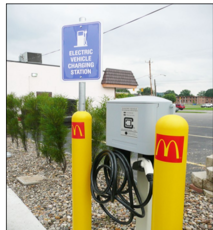
This charging station for electric cars at a McDonald’s restaurant in Huntington has two hook-ups and is wired for three, said store owner Tom Wolf.
