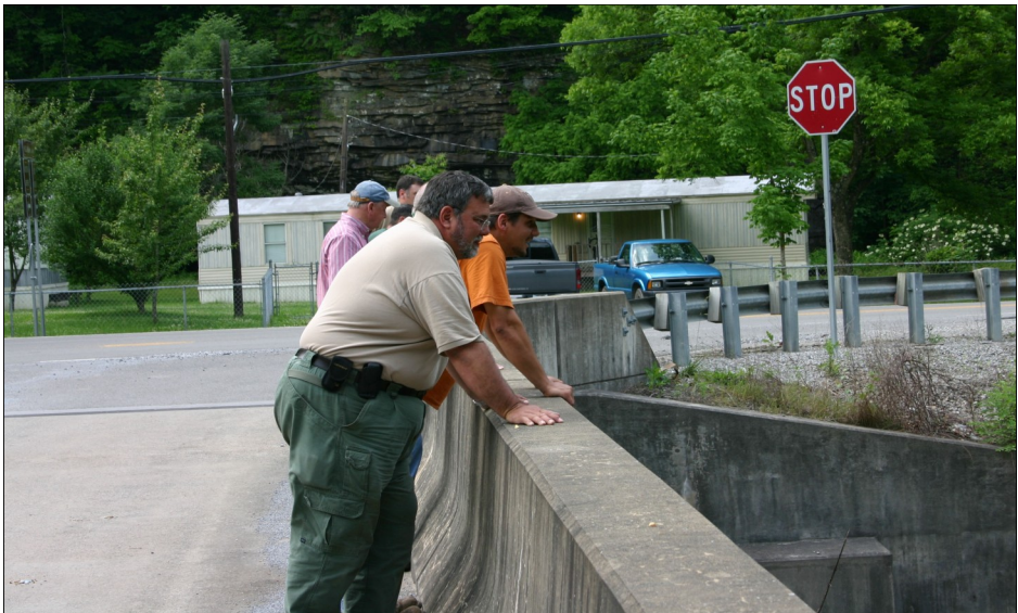
Greg Rote looks over debris-filled Little Huff Creek in Wyoming County during a recent stop in Southern West Virginia. Rote drives between 2,000-3,000 miles a month on the job.
