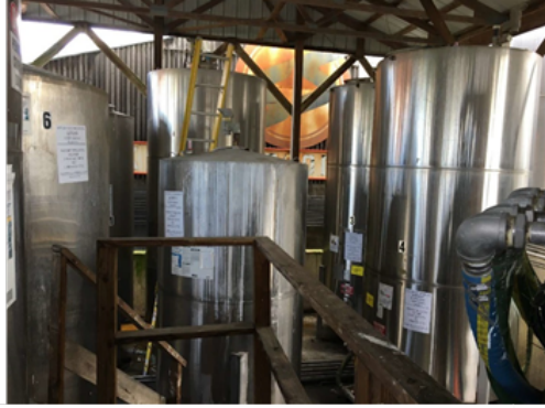
Secondary containment at a bulk facility.
