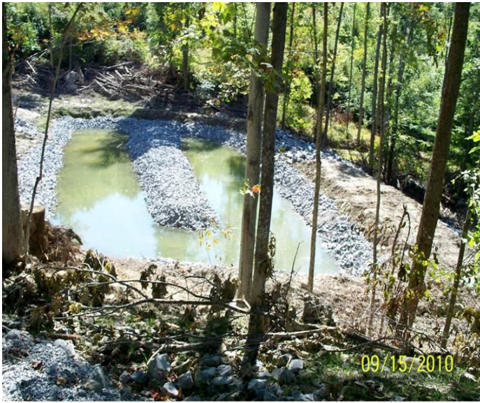
Polishing pond in the lower part of the drainage
