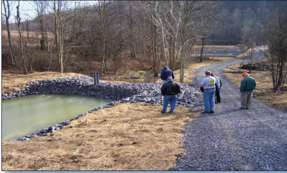
Figure 2. Water gains alkalinity as it flows through a leach bed at Site 3.
