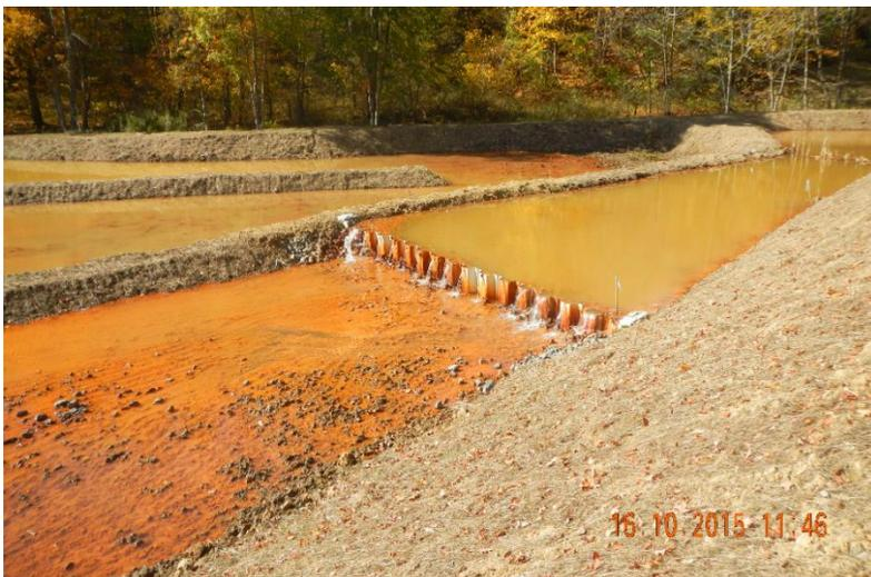
The project consisted of a combination of passive treatment technologies. The main treatment method for the passive treatment system at Site 7 is five aerobic wetland cells. Discharge from the impoundment makes its way over an in-channel aeration weir and is then culverted into wetland #1. Wetland #1 has three large aeration weirs to encourage oxidation of the metals. The water then makes its way through four more wetland cells with aeration drops at various locations. After the fifth and final
