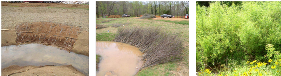
Figure 4: Brush mattress preparation, before tie-down, and after one-year growth
