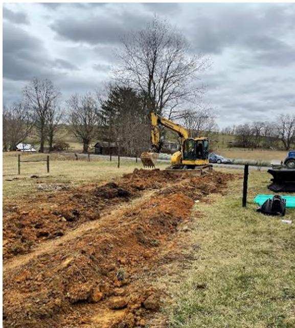
Figure 19. Digging out old drain lines.
