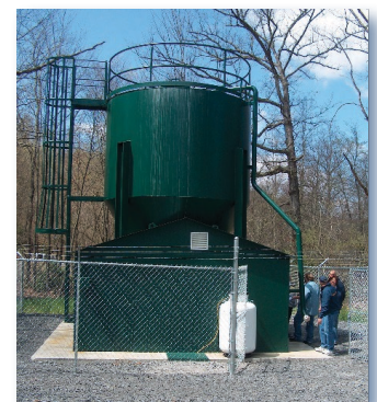
Figure 2. This lime doser was installed as part of the Three Fork Creek restoration.
