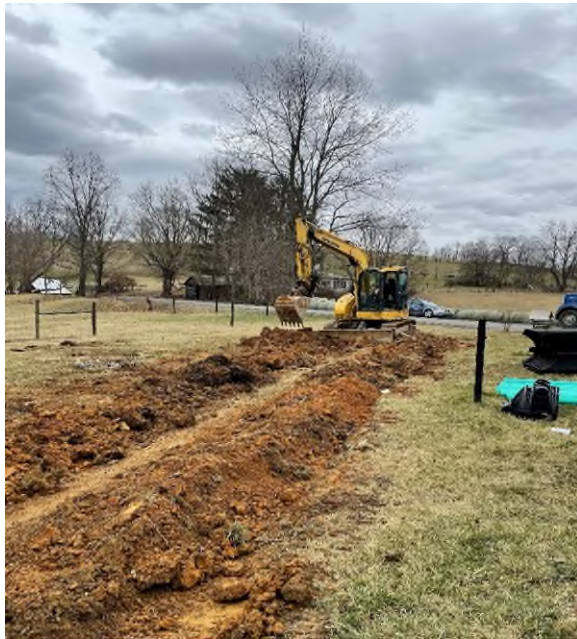
Figure 19. Digging out old drain lines.
