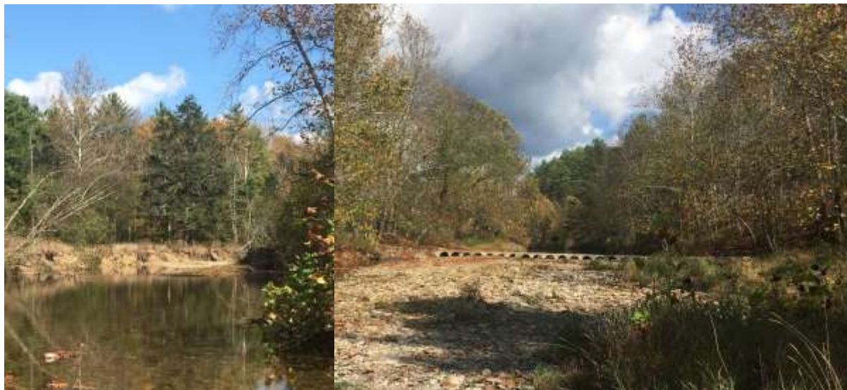
Figure 11. Left: Bank erosion causing excess sediment to build up and bars along the stream. Right: Low water Bridge preventing fish passage and causing excess sediment to build up.
