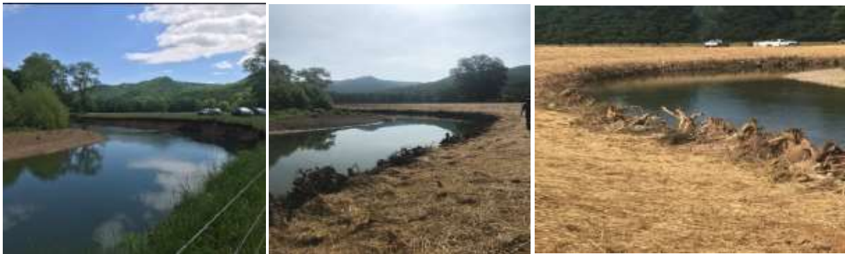
Figure 16. Before and after example of using toe wood structures to address streambank erosion along agricultural land in the Anthony Creek Watershed.
