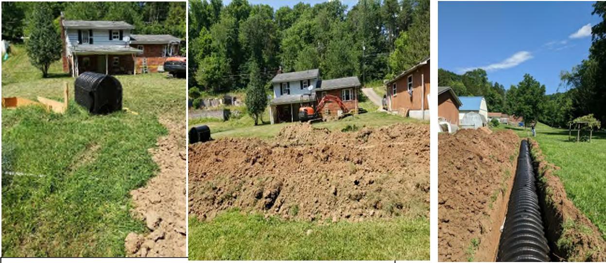
Figure 1, Images of completed septic replacement projects.
