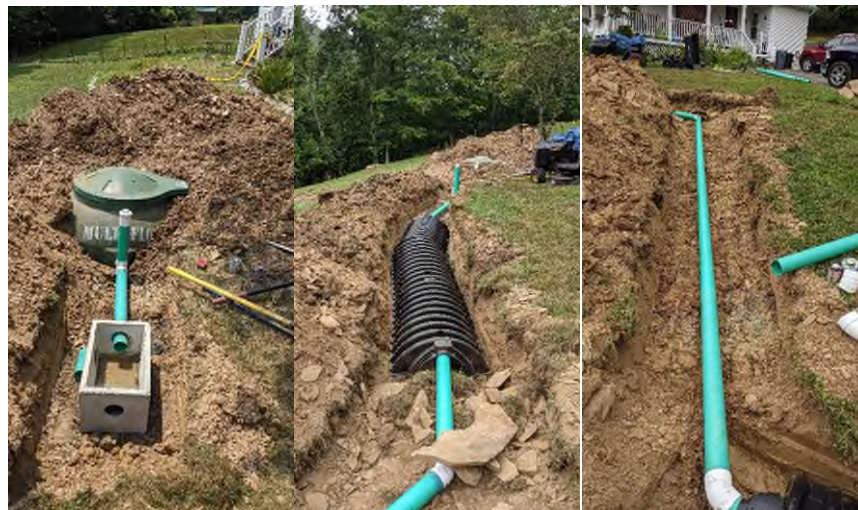
Fig. 1: Images of complete Septic Replacement
