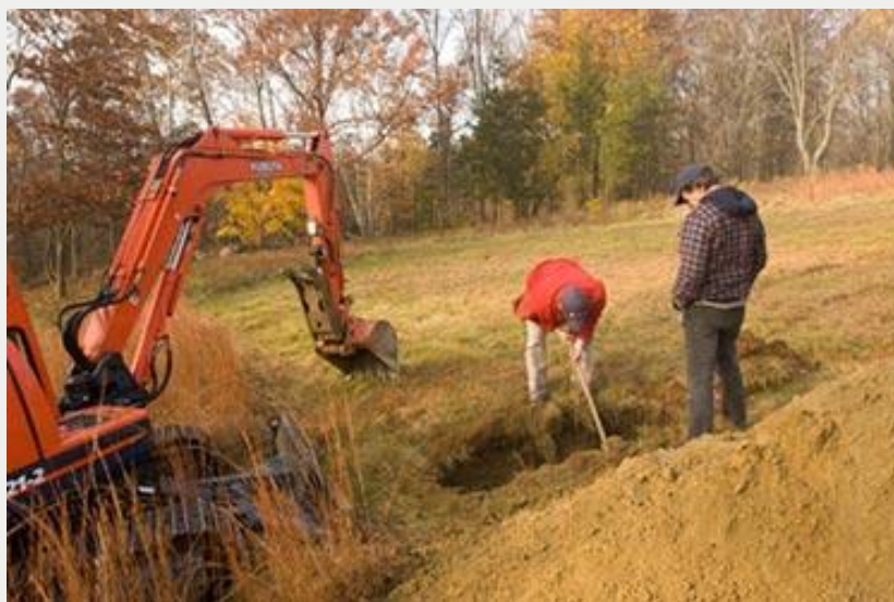
Figure B.1 Soil Profile Test Pit (photo source: Arthur J. Howland & Assoc., P.C.)
