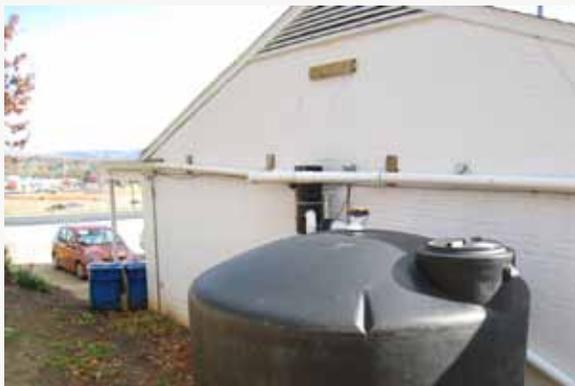
Rainwater Harvesting systems provide for the capture, storage, and release of rainwater for future beneficial use, either inside or outside the building. Systems usually capture rooftop runoff. Storage tanks can be a variety of materials and either above ground or underground.
