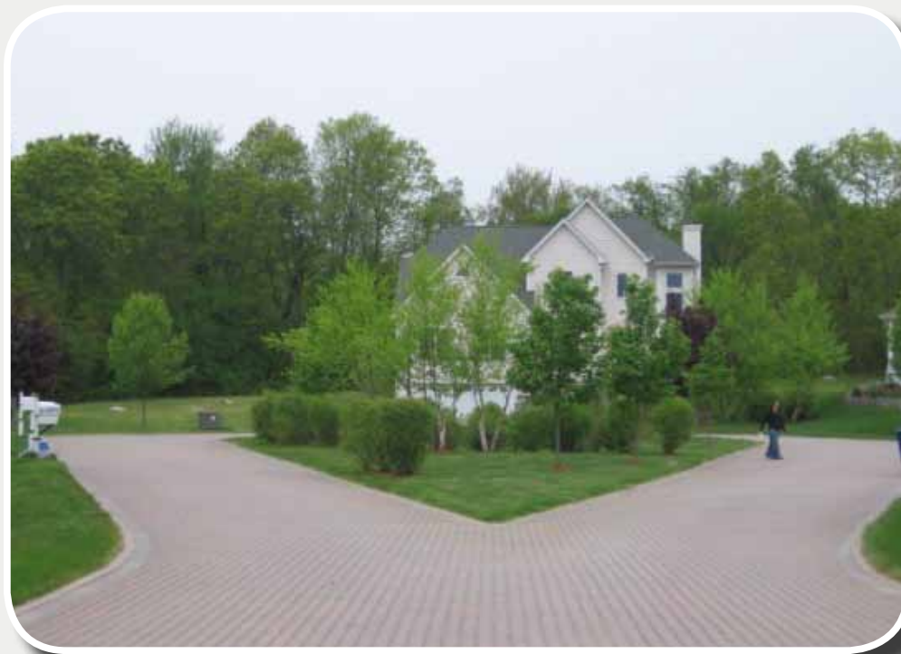
Figure BSD-4. Cul-de-sac with bioretention island
