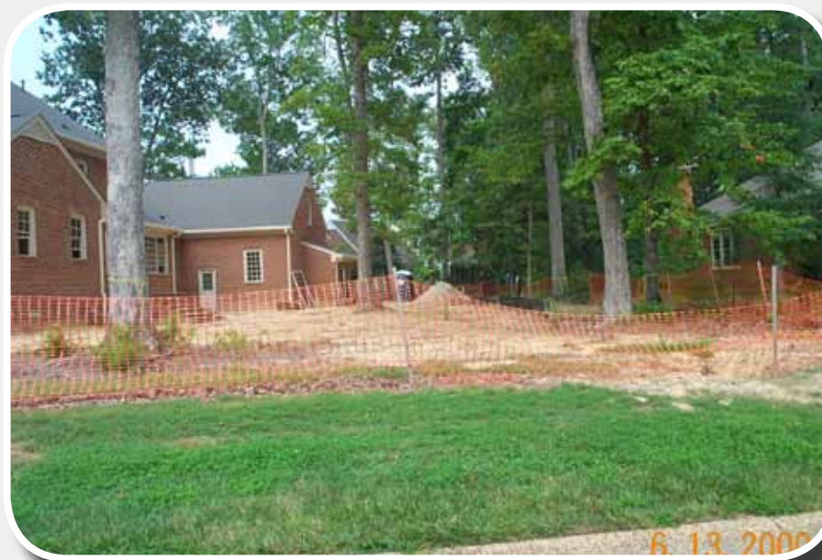
Figure BSD-1. Fencing to delineate limits of clearing and protect trees
