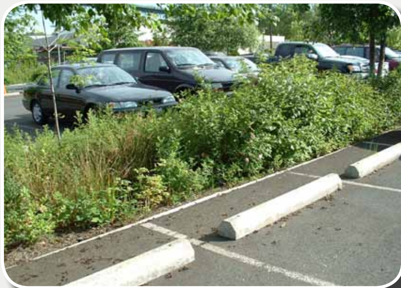
Figure BSD-5. Parking lot landscaping area that provides stormwater management
