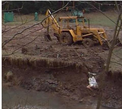
Appropriate best management practices can be used during construction to minimize the impacts on water quality. These practices can include silt fence, straw bales, revegetating and mulching, sediment ponds, and various other measures to either keep the soil in place on the land, or at least prevent the soil that moves from entering the stream.
