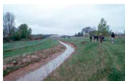
A headwater stream channel near Toledo, OH relocated to accommodate development. Photo courtesy of Marshal A. Moser
