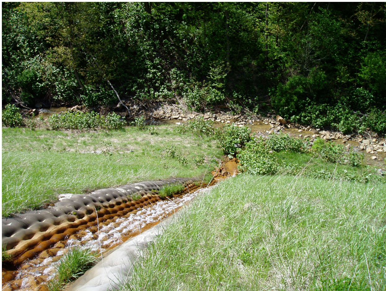
Figure A-5-4. Channelized drainage ditch with iron staining entering Piney Swamp Run.
