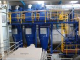
Figure 8. Photo of a typical dryer in operation from first floor level.
