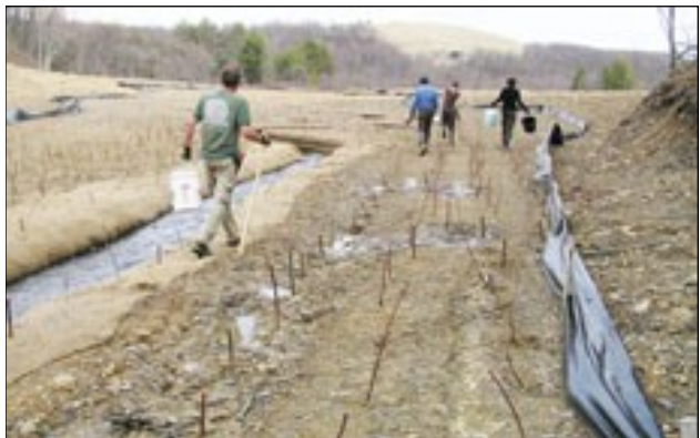
Live branch cuttings planted in stream channel riparian zones.
