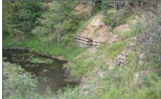
Highwall and dangerous impoundment.
