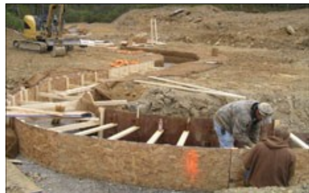
Constructing flexible forms.
