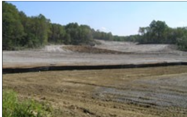
Regrading and liming complete.
