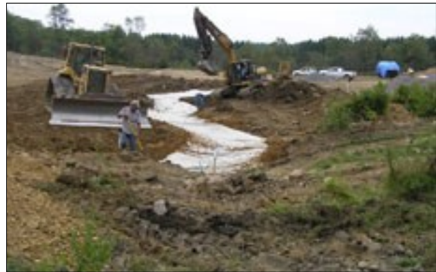
Backfilling anchor trenches for liner.
