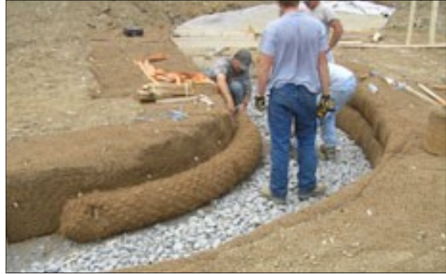
Installing coir logs for point bars on inside bends.
