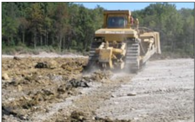
Dozer dragging ripper tooth to loosen soil.
