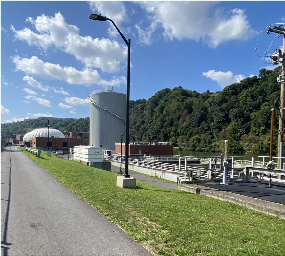
Completed SRF Project for Morgantown Utility Board (Star City WWTP)
