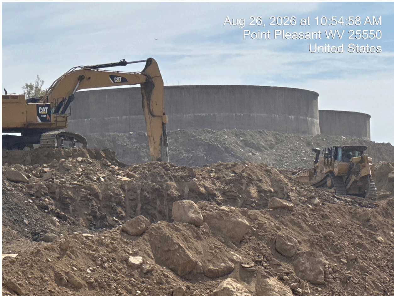
Figure 2: Photograph of the Two Existing Firewater Tanks
