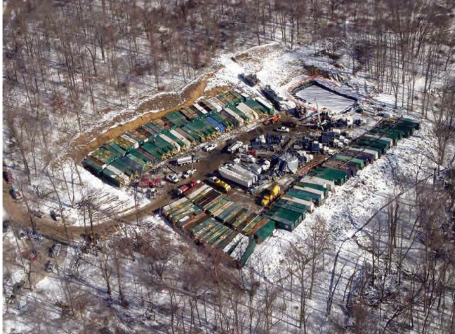
Marcellus well location, with large number of frack tanks and other equipment hauled to the site.
