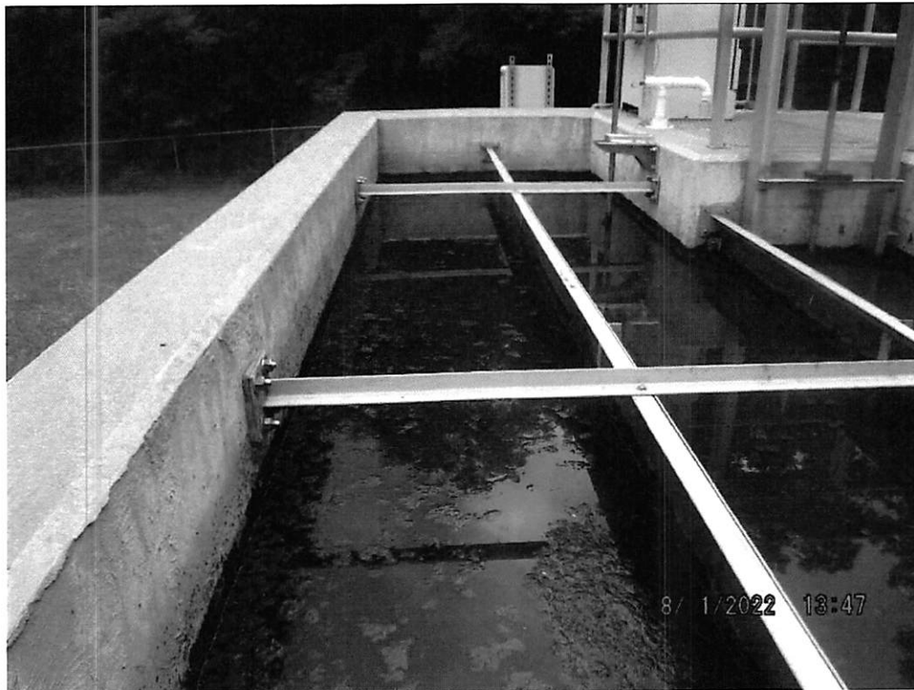
DSCF9231: Sludge was in the contact chamber. Wastewater was turbid and brown.
