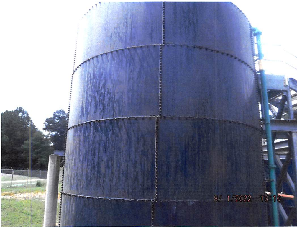
DSCF9174: Dried sludge was on the sides of the sludge digester.
