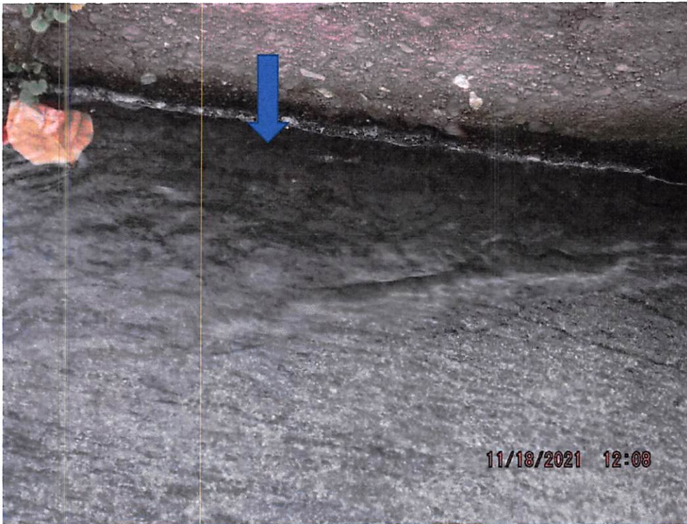
DSCF6069: Sludge was observed on the post aeration steps (blue arrow).
