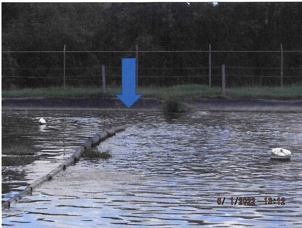
DSCF9176: A portion of the baffle (blue arrow) was down.
