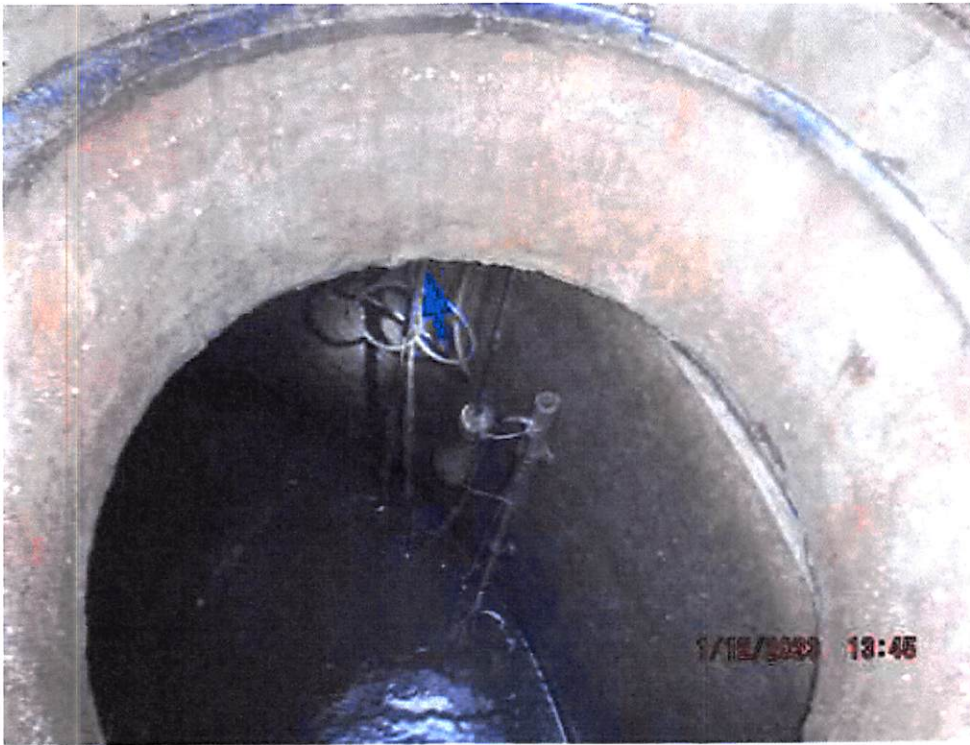
Blue arrow indicates the conduit that leads to the basement.
