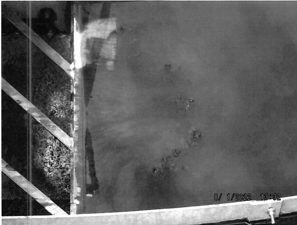
DSCF9217: Sludge was floating in the river clarifier. Wastewater was turbid and brown.
