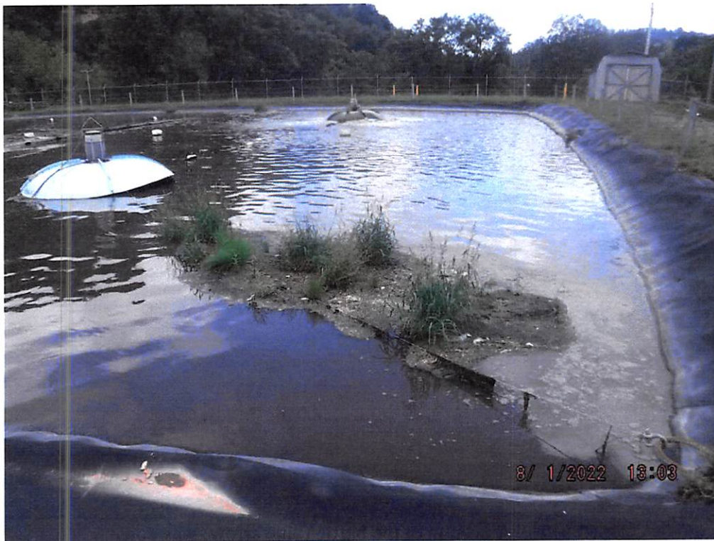
DSCF9168: On August 1, 2022, floating sludge and vegetation was observed in the aerated lagoon.
