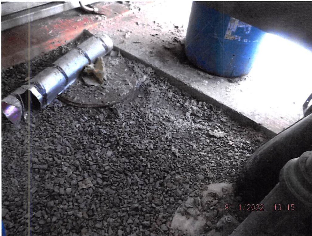
DSCF9180: Solids were present on the ground beneath the mechanical bar screen.
