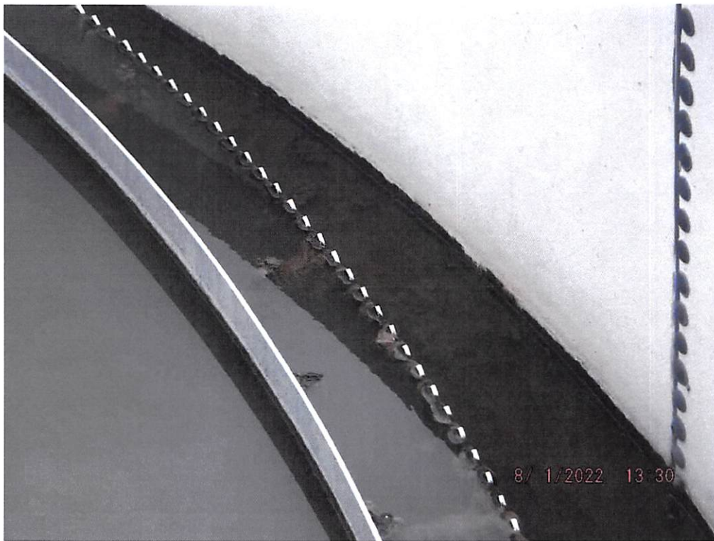
DSCF9210: Sludge was in the weir of the river clarifier.
