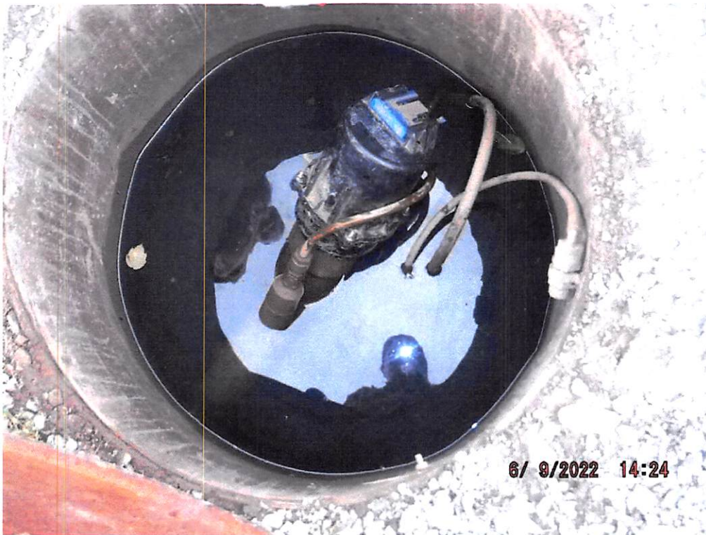
DSCF8744: Vacuum pit near 264 Main St., Worthington was not operating properly on June 9, 2022.
