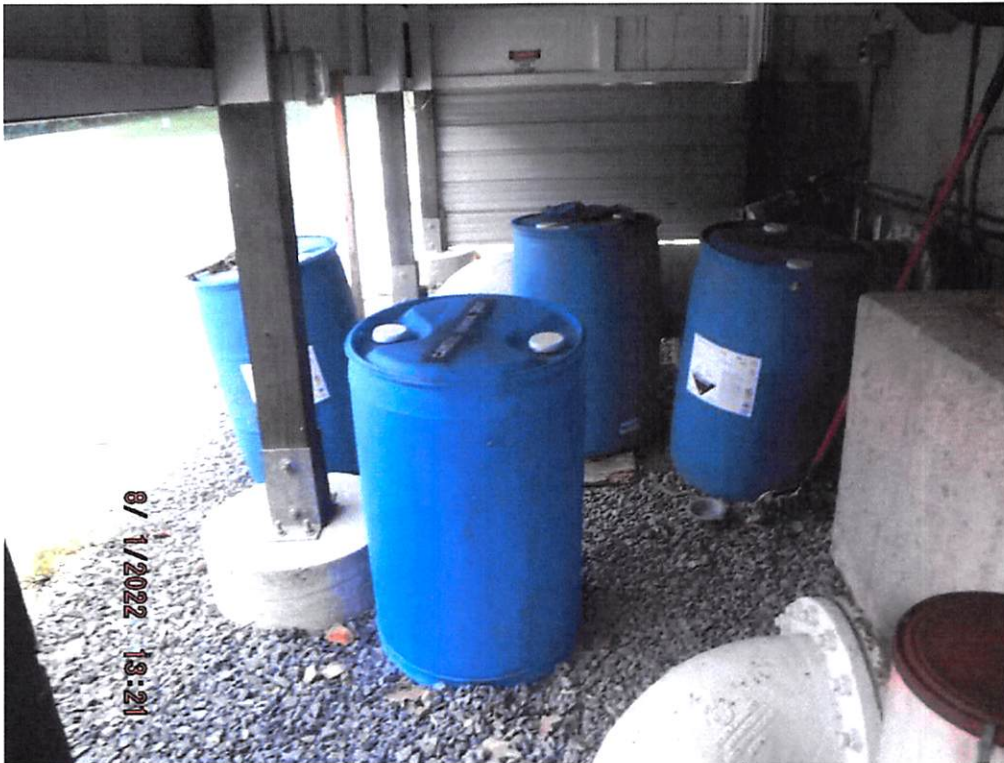
DSCF9185: Fifty-five-gallon drums filled with caustic soda were stored on the ground.
