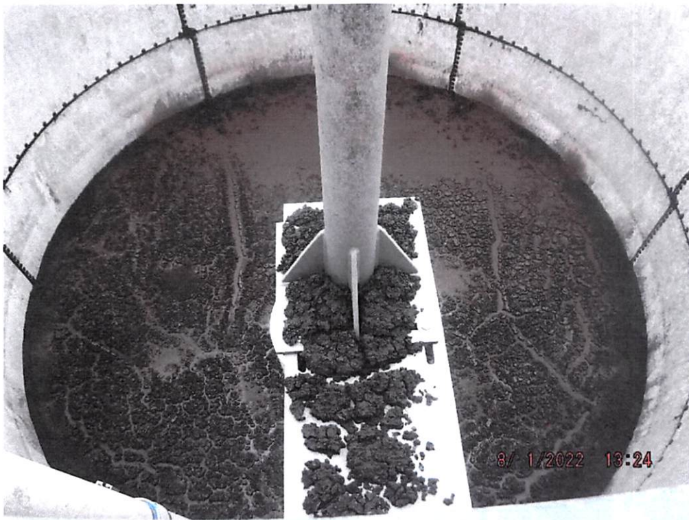
DSCF9190: Dried sludge was on a ledge near the top of the sludge digester.
