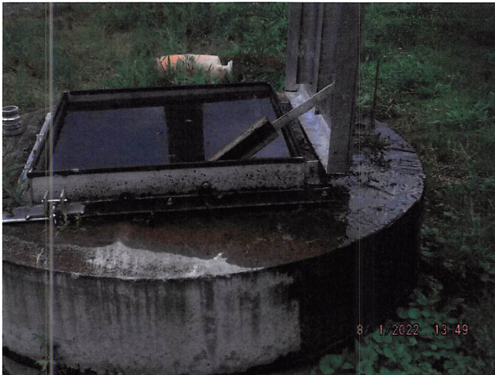
DSCF9240: The wet well for the surge pond was overflowing during the inspection.
