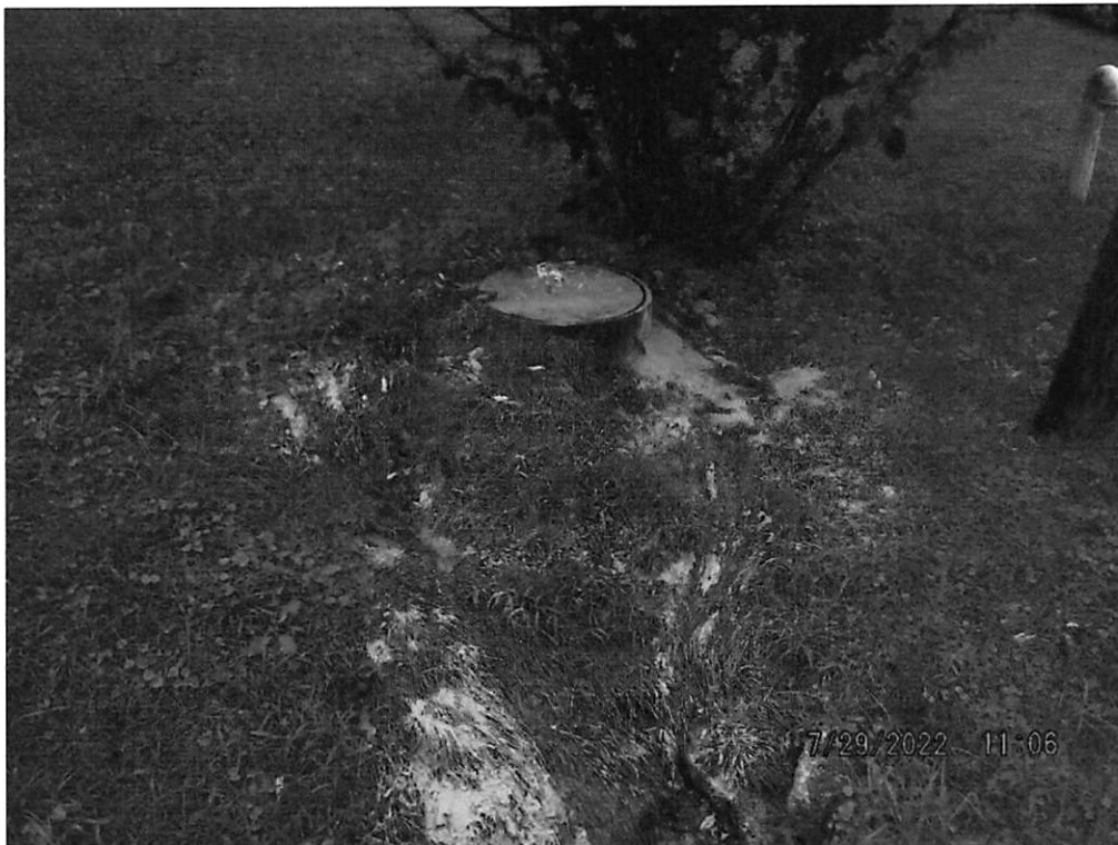
DSCF9158: The vacuum pit located at Woodlands Assisted Living was overflowing on July 29, 2022. The area had been limed.
