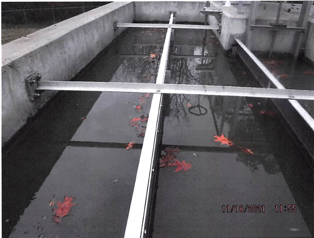
DSCF6050: The contact chamber was turbid.
