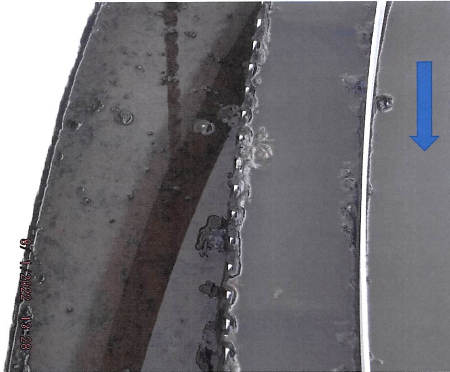
DSCF9198: Sludge was in the weir of the trail clarifier. Partially treated wastewater was turbid and brown in the center of the clarifier (blue arrow).
