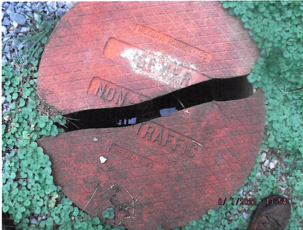
DSCF9246: The vacuum pit located at the WWTP had a broken lid.
