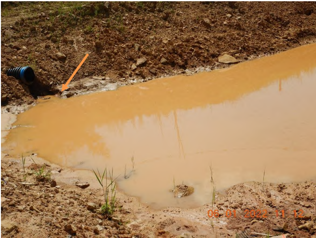
An unstable inlet for Sediment Trap 2.
