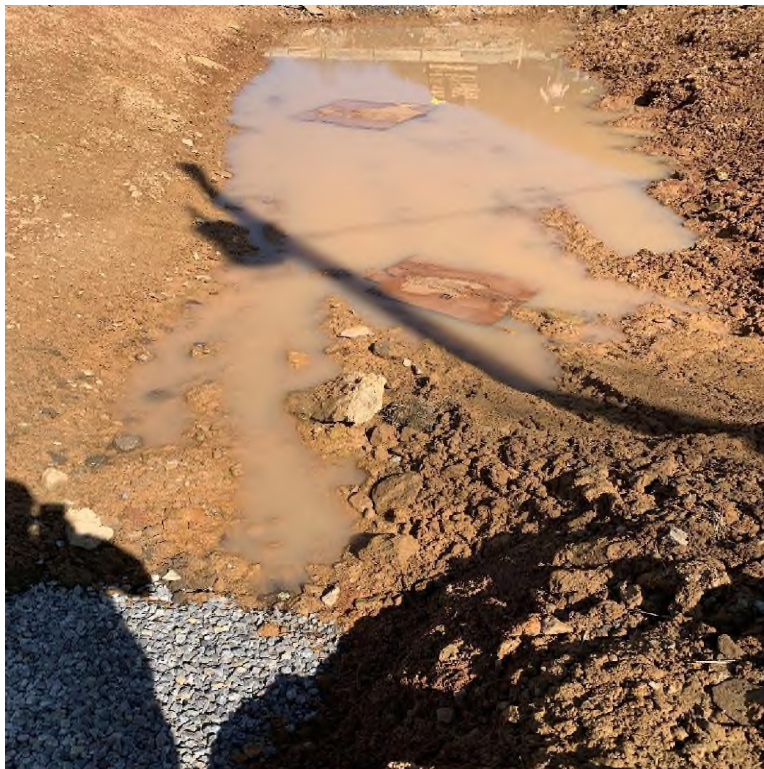
Area where Sediment Trap 2 should have been installed.
