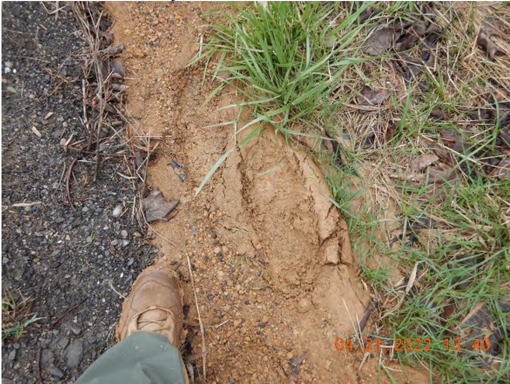
Fresh sediment deposits in the adjacent ditch.
