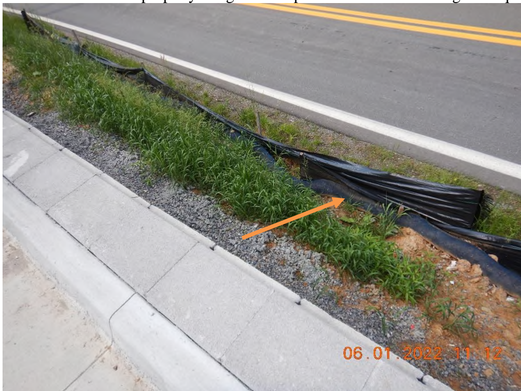
Compost filter sock that is missing the required staking.
