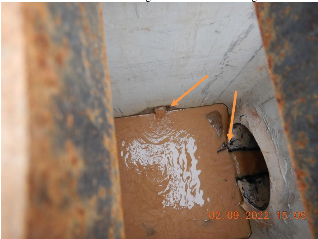
Sediment laden water discharging through the underdrain and leaving the site via culvert. There is no protection for the existing drop inlet.
