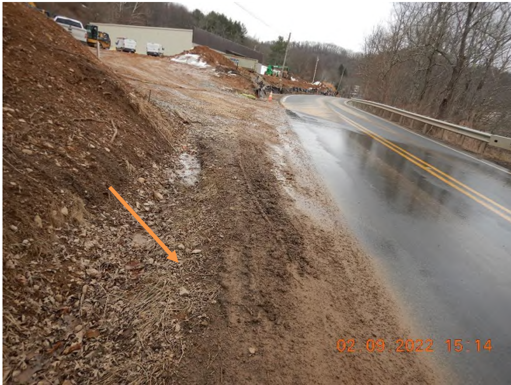
Sediment deposits in the adjacent ditch line.
