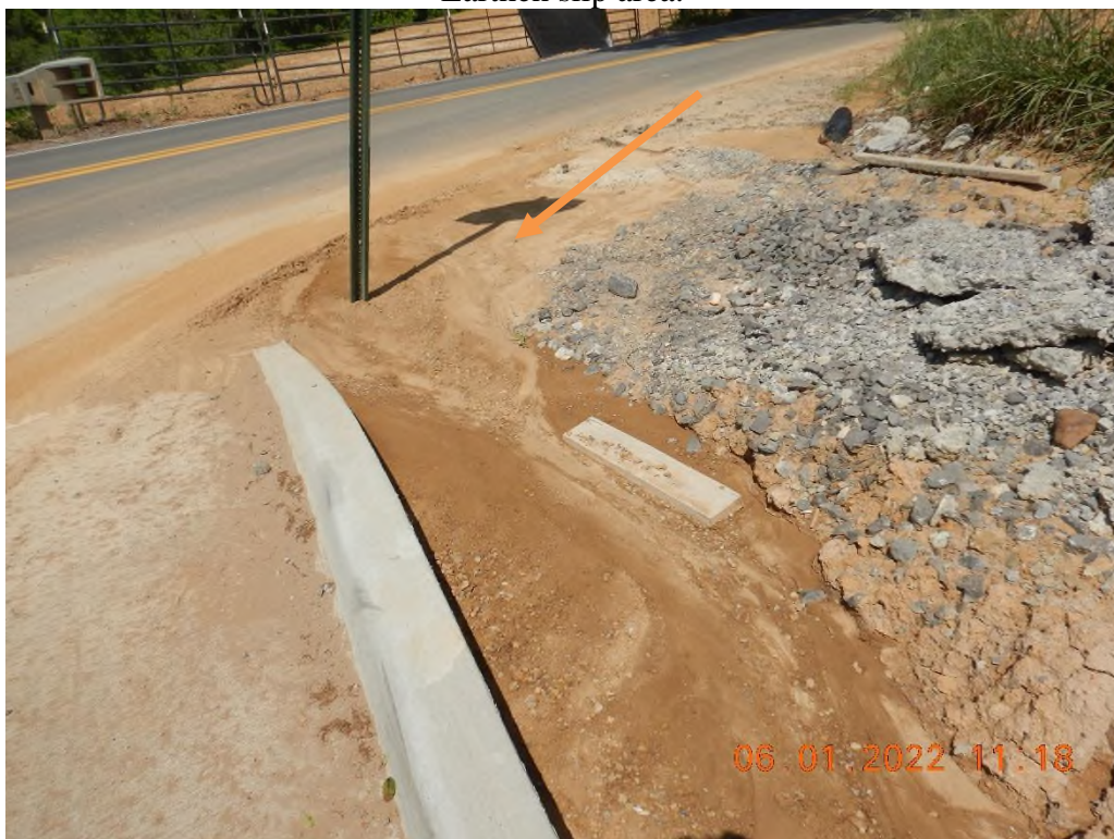
Sediment discharging off the LOD.
