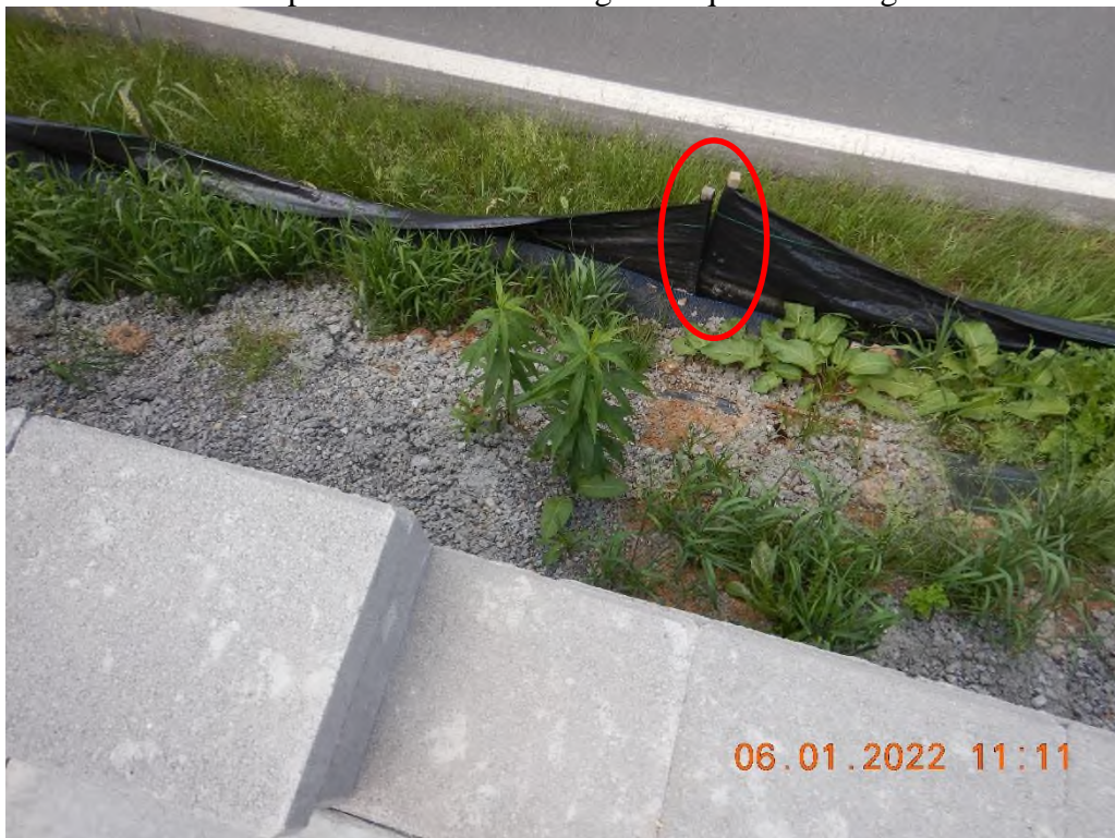
Perimeter controls not properly merged.
