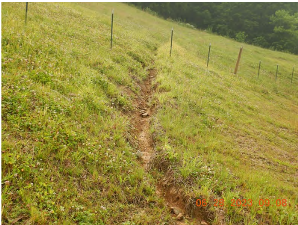
Another erosion gully noted near the earthen slip portion of the site. This is due to a concentrated flow going across a non-stabilized surface.
