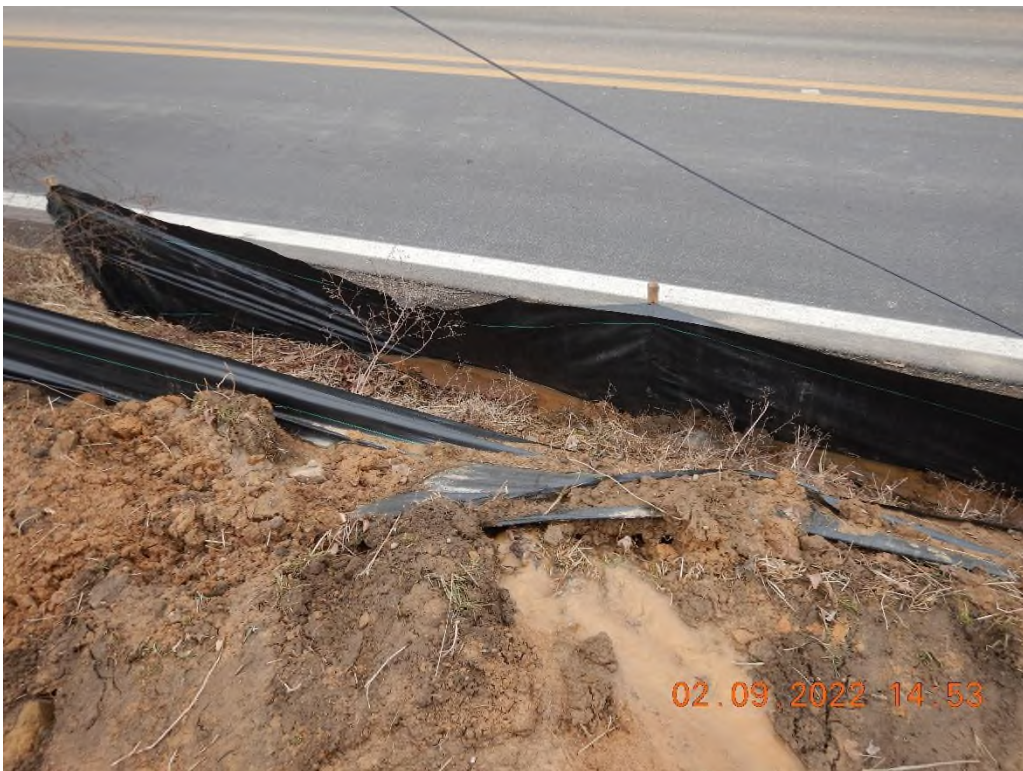
Silt fence needing maintenance.
