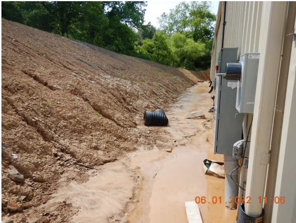
The eastern portion of the site, with fill slope erosion and no stabilization.
