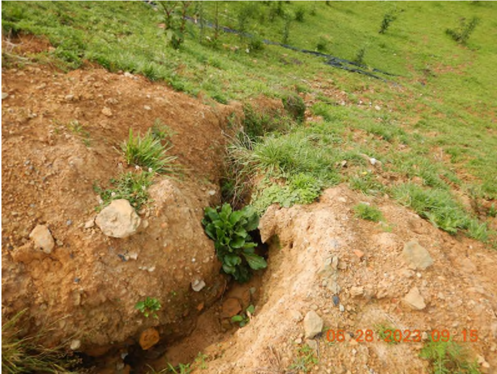
An erosion gully noted in the waste area. This is due to a concentrated flow going across a non-stabilized surface.
