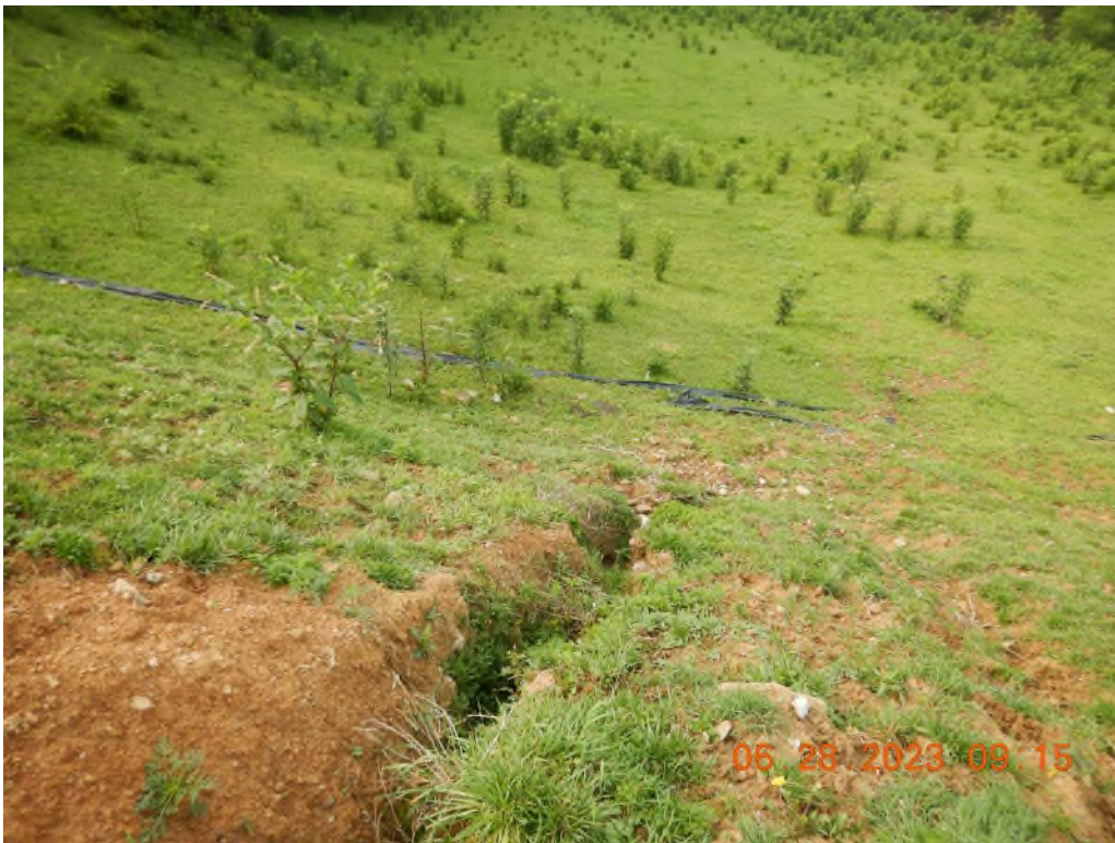
Silt fence showing the need for maintenance in the waste area.
