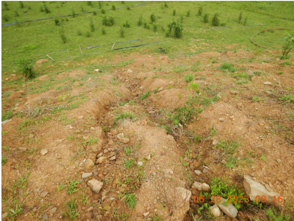
Silt fence showing the need for maintenance. As a result, sediment deposits were noted beyond the installed controls. Also shown are more erosion gullies. This is due to a concentrated flow going across a non-stabilized surface.
