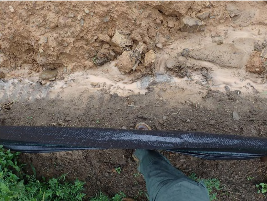
Photo 8: Silt fence not properly implemented around the waste site.
