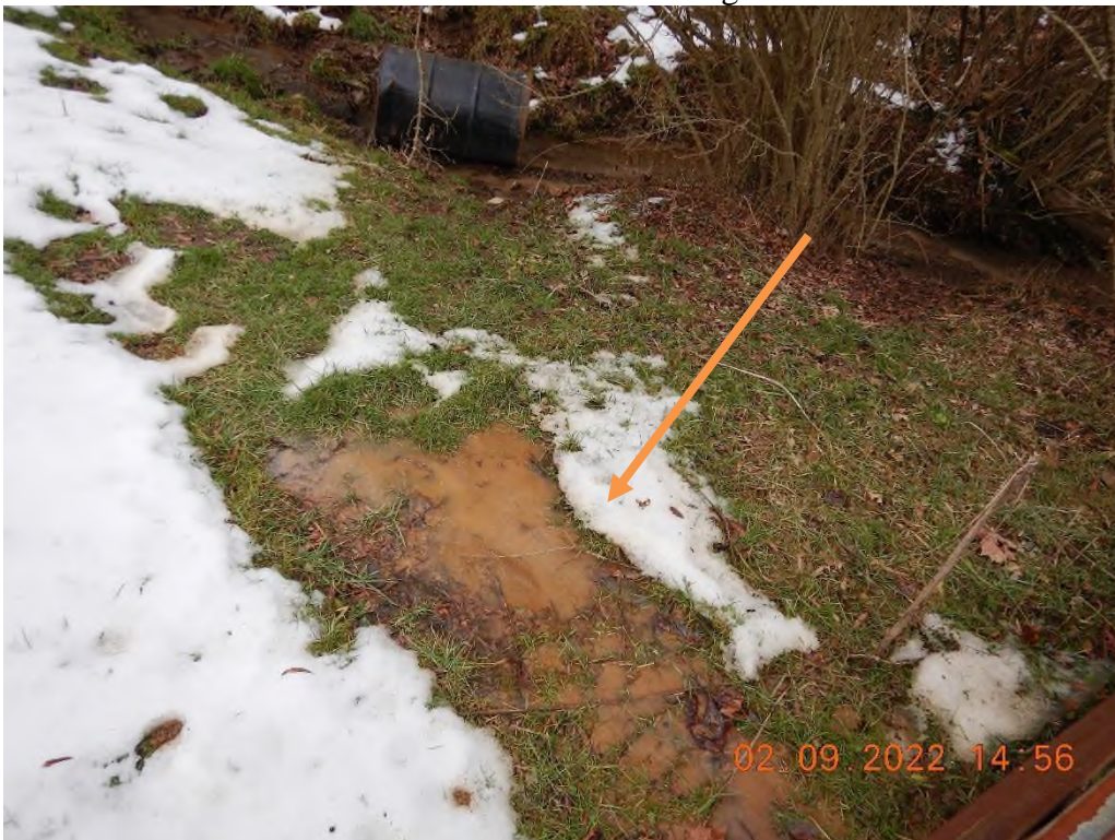
Sediment laden water that has left the site.
