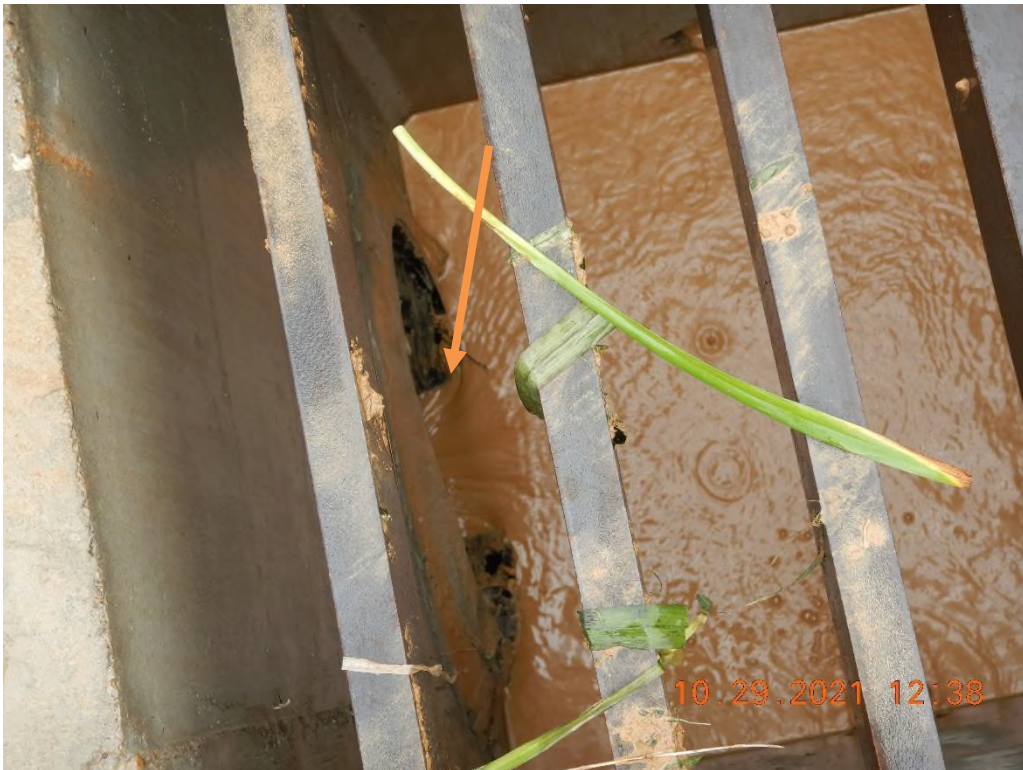
Sediment laden water entering the culvert and discharging toward Little Tenmile.
