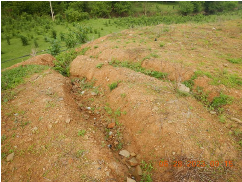
More erosion gullies noted in the waste area. This is due to a concentrated flow going across a non-stabilized surface.
