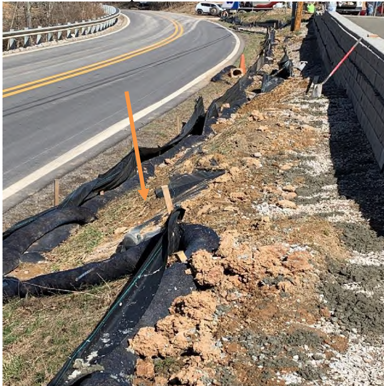
Silt fence that is in need of maintenance.
