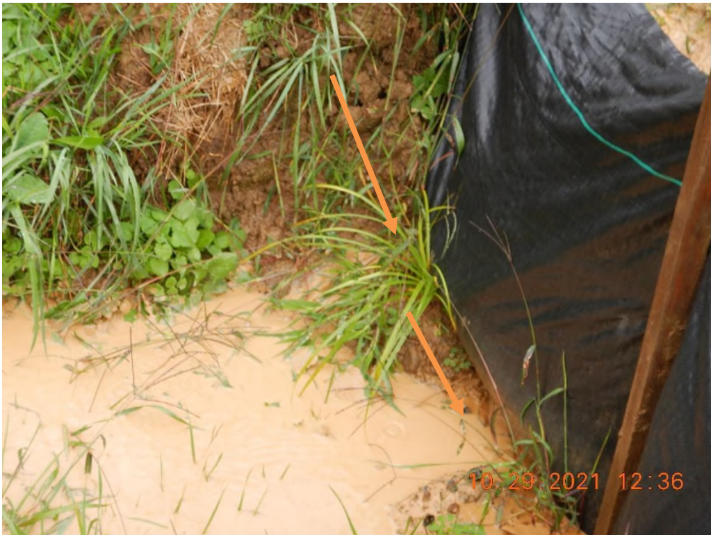
Sediment laden water is bypassing treatment due to a lack of maintenance to the installed silt fence.
