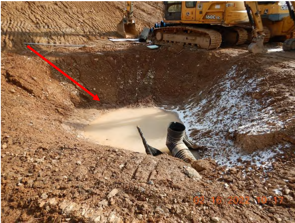
Sediment Trap 1 not installed, as stated in the SWPPP.
