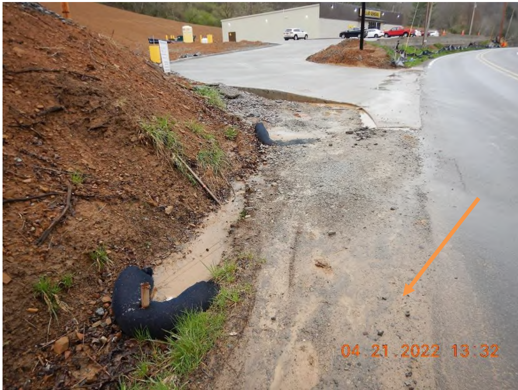
Evidence of sediment laden water leaving the site.
