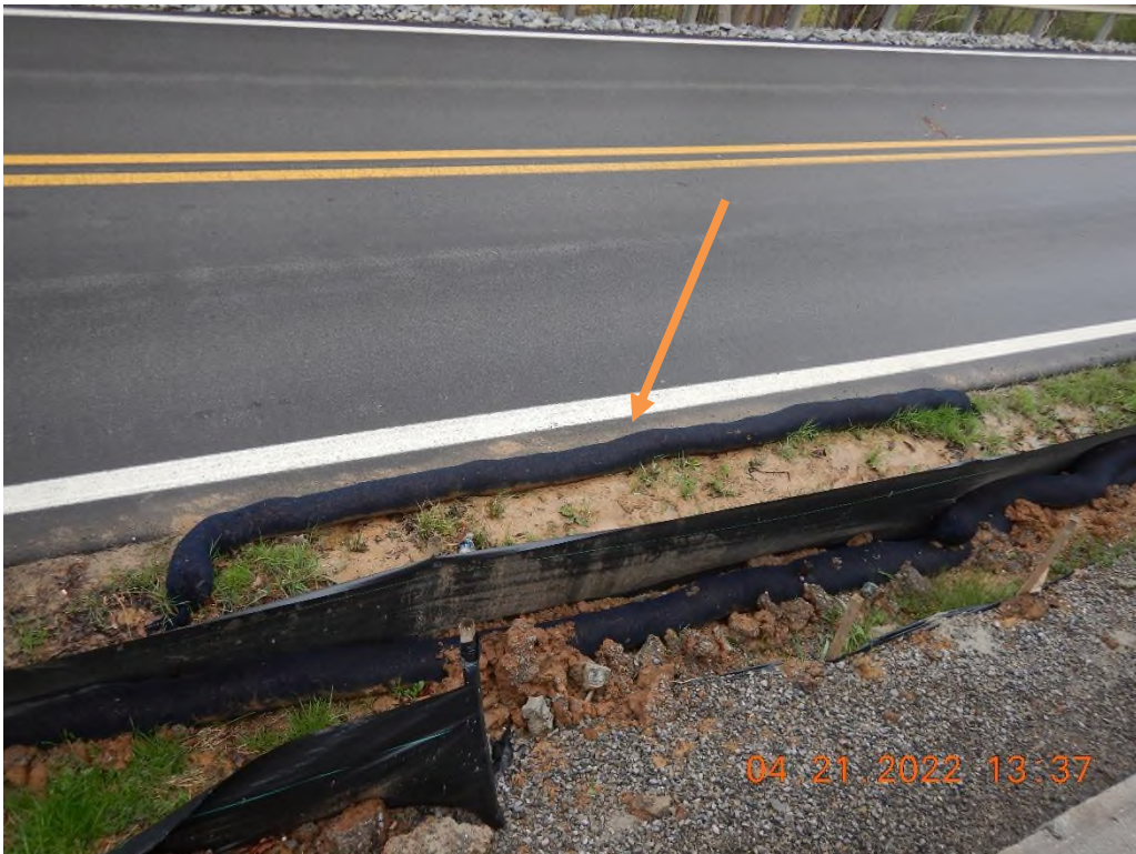
Compost filter sock lacking the required staking.
