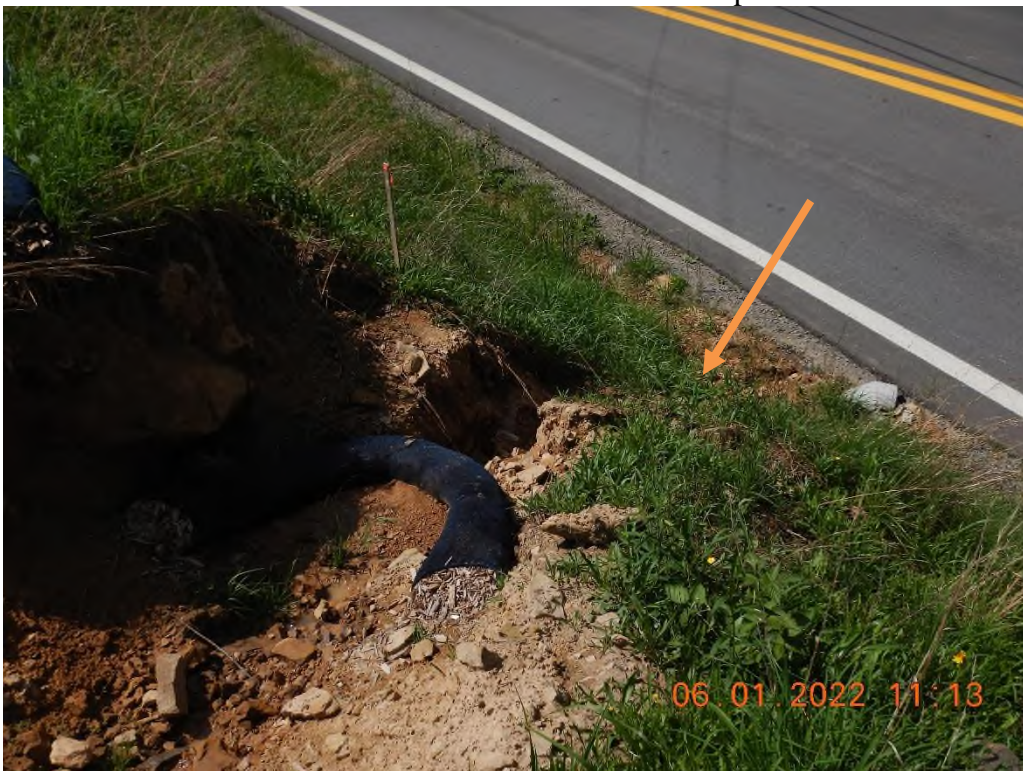
Sediment deposits discharging off the LOD.
