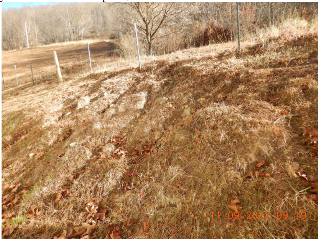
A portion of the hill behind the building, with erosion gullies due to concentrated flow across a non-stabilized area.
