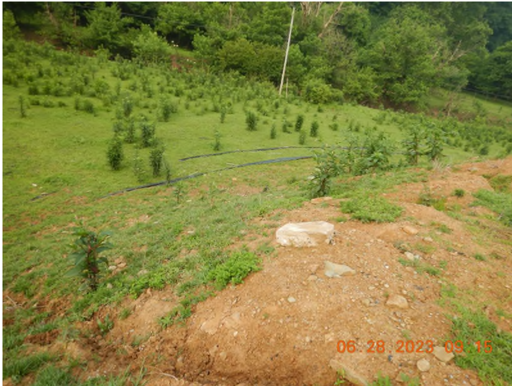
More silt fence showing the need for maintenance.
