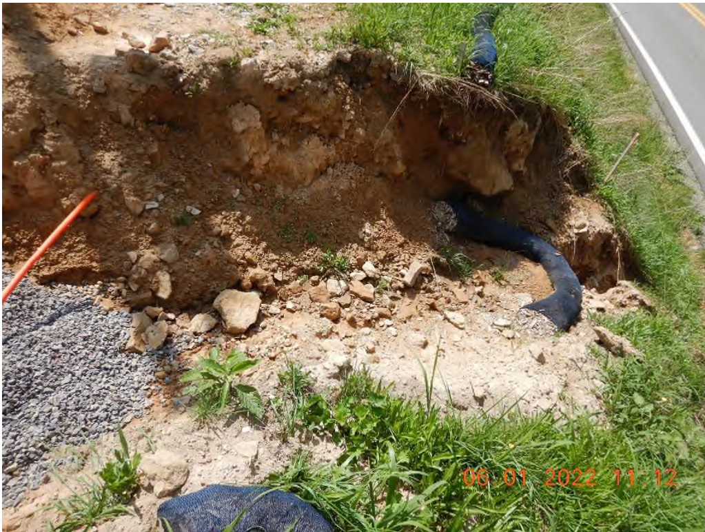
An unstable outlet from Sediment Trap 2.
