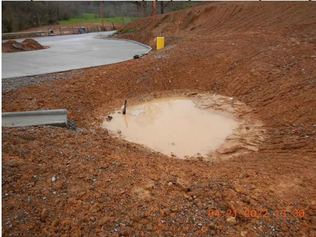
The area where Proposed Sediment Trap 1 should have been installed.
