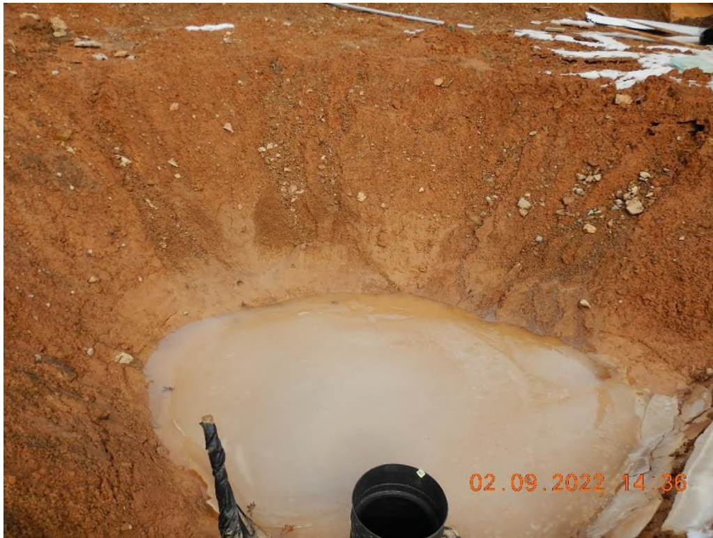
Proposed Sediment Trap 1 not installed, as stated in the SWPPP.
