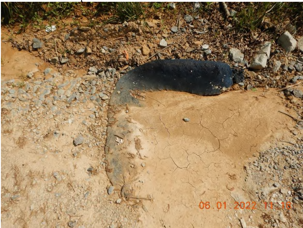
Compost filter sock is missing the required staking.
