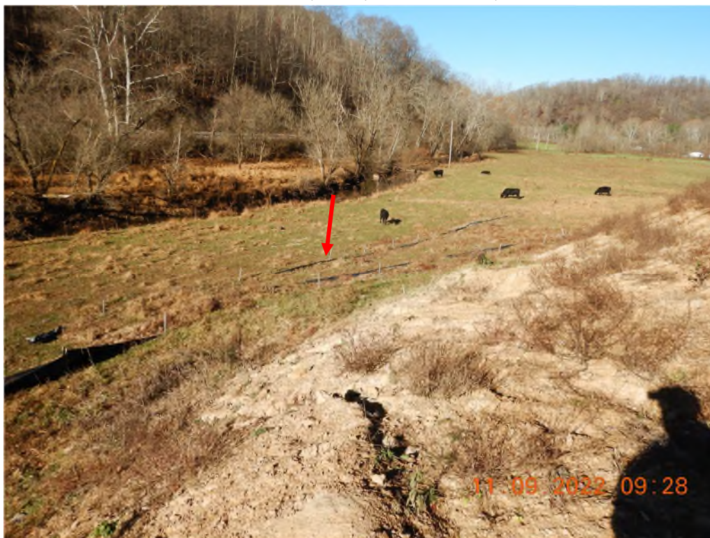
Silt fence needed maintenance at the waste area, allowing sediment laden water to leave the site untreated.
