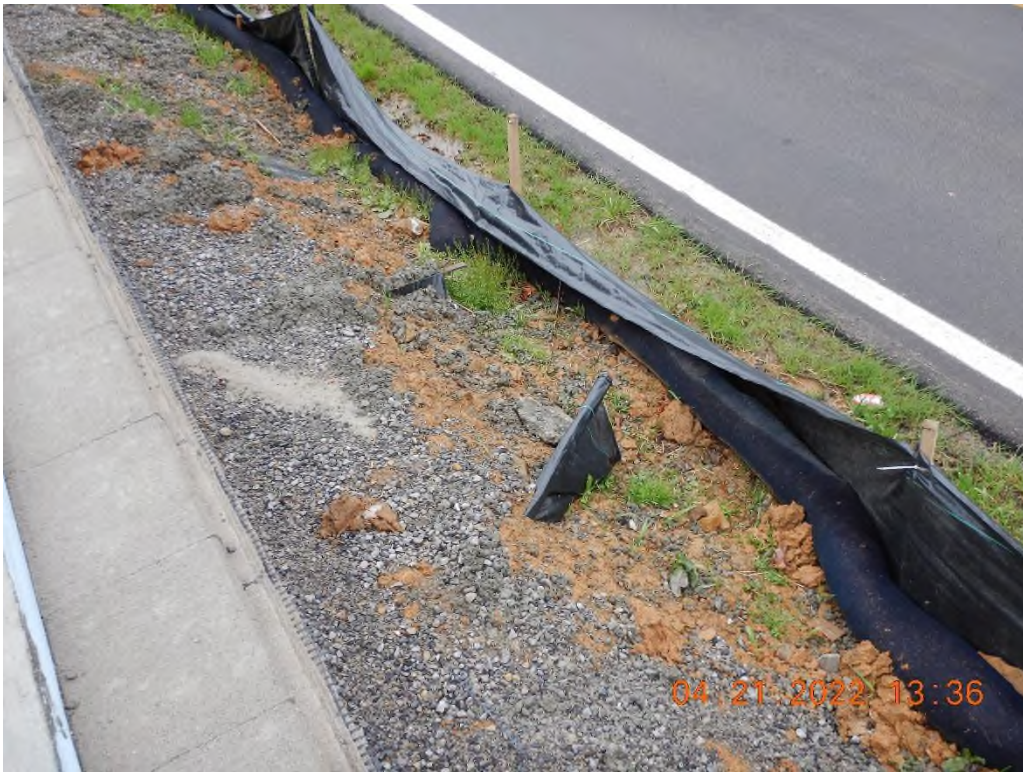
Silt fence needed maintenance.
