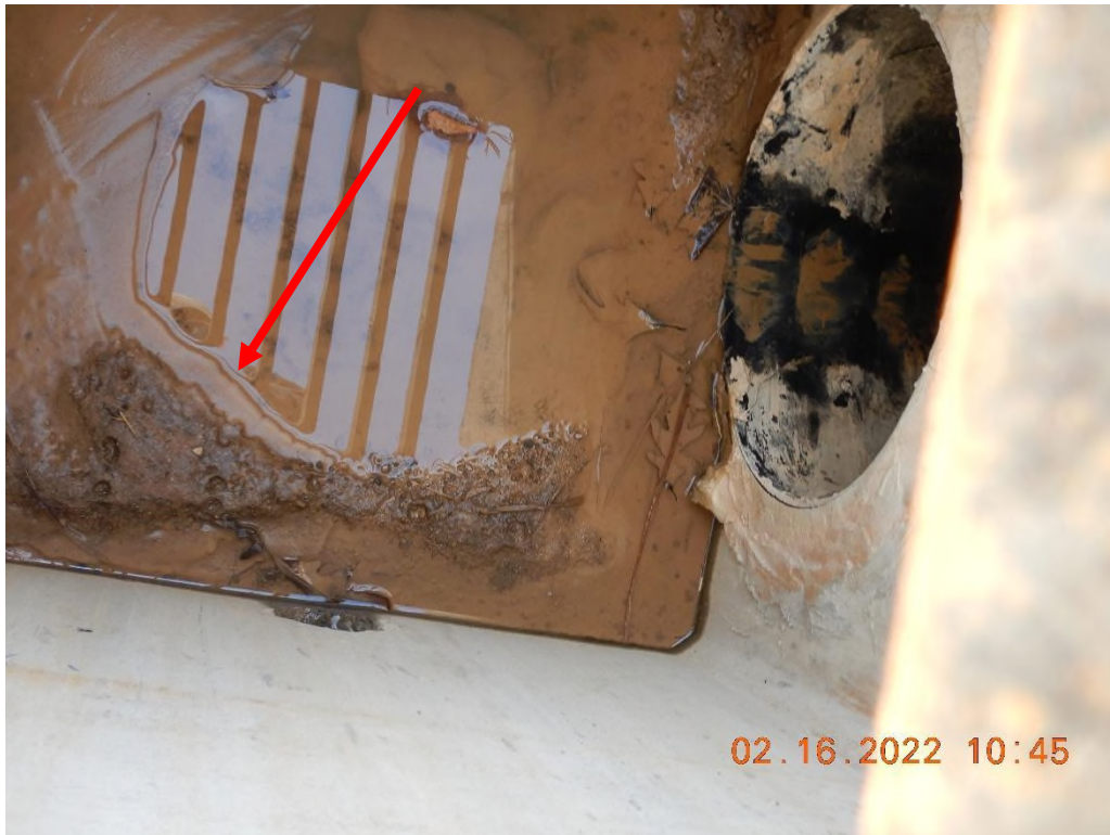
Sediment deposits in the bottom of the drop inlet. There is no drop inlet protection in place.
