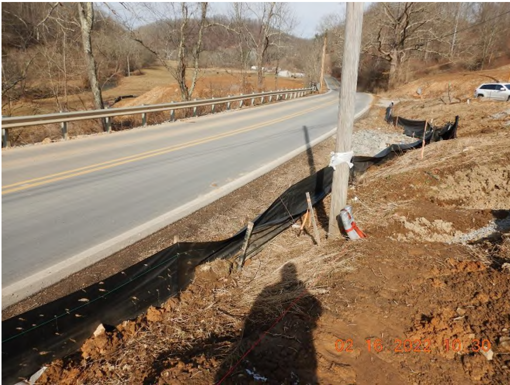
Controls were not toed into the ground.
