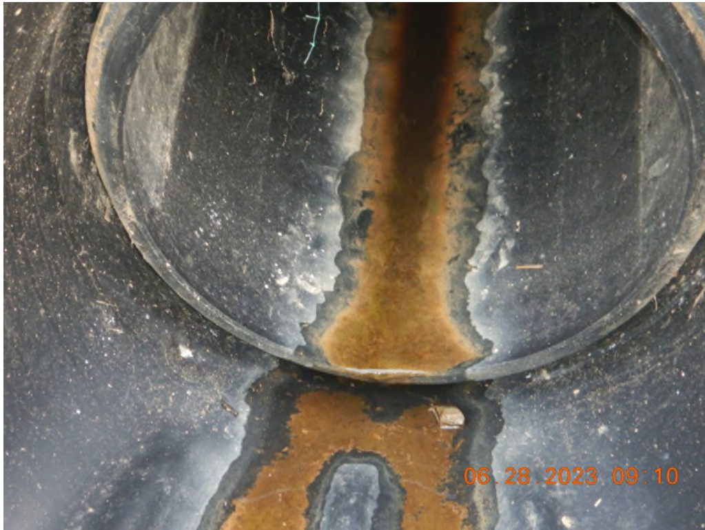
This is the outlet of Sediment Trap 1 showing evidence of a leak within the structure as water is discharging through the outlet despite not being at a 50% wet storage.
