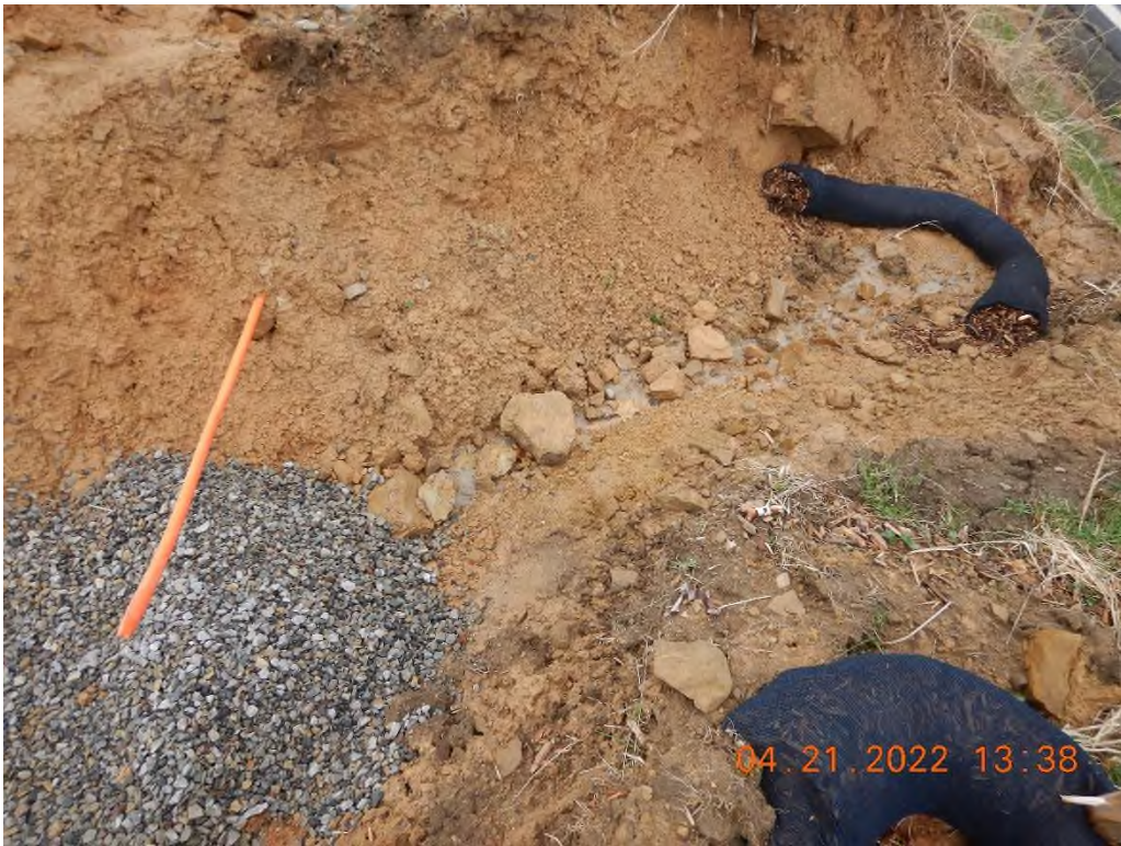
Unstable outlet of Sediment Trap 2.
