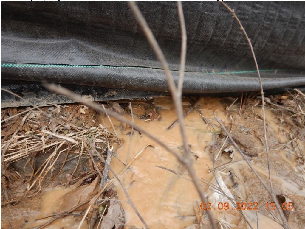
Sediment laden water bypassing improperly installed silt fence and leaving the site.
