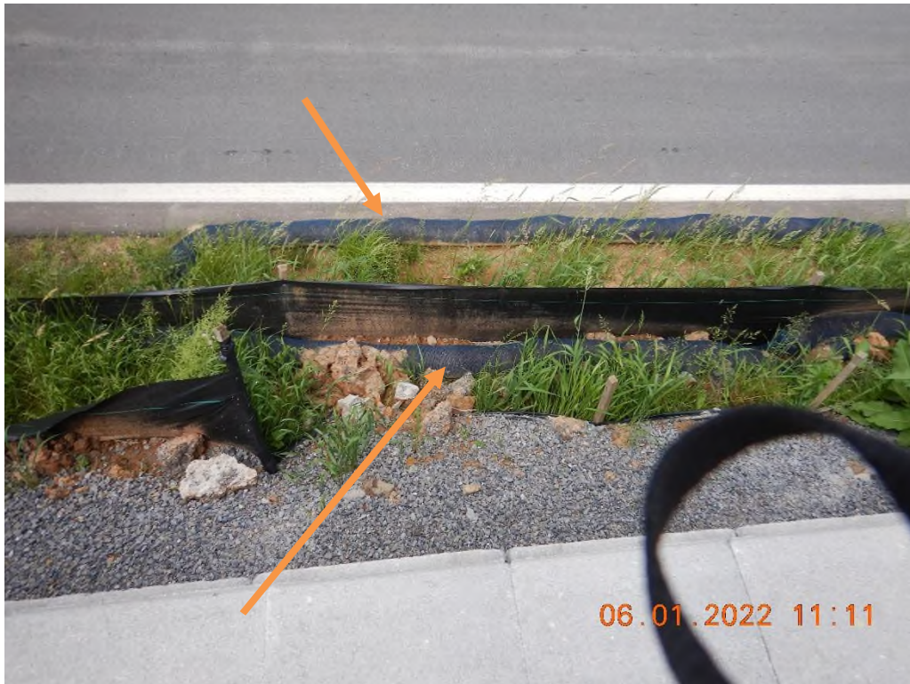
Compost filter sock missing the required staking.
