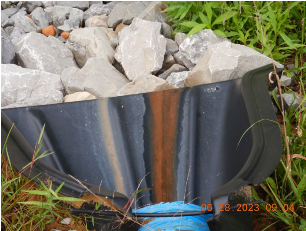
A photo taken at the outlet of the Sediment Trap 2. As shown, there is evidence of water discharging through the outlet meaning there is a leak within the structure of the trap.
