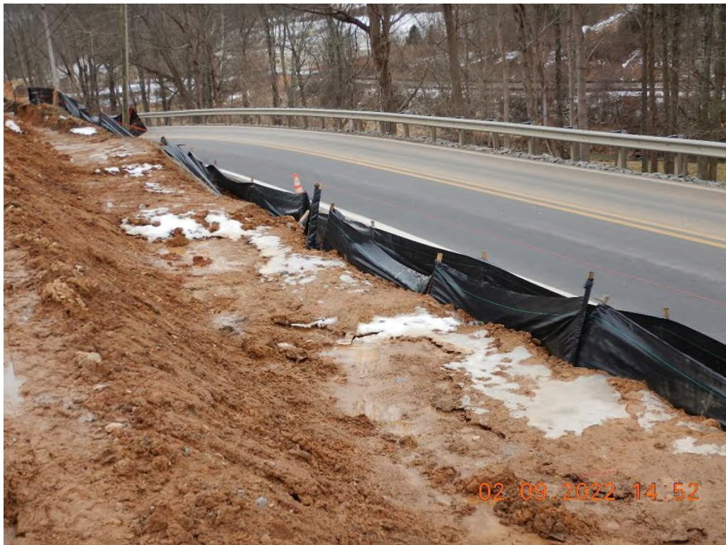
Silt fence in need of maintenance.
