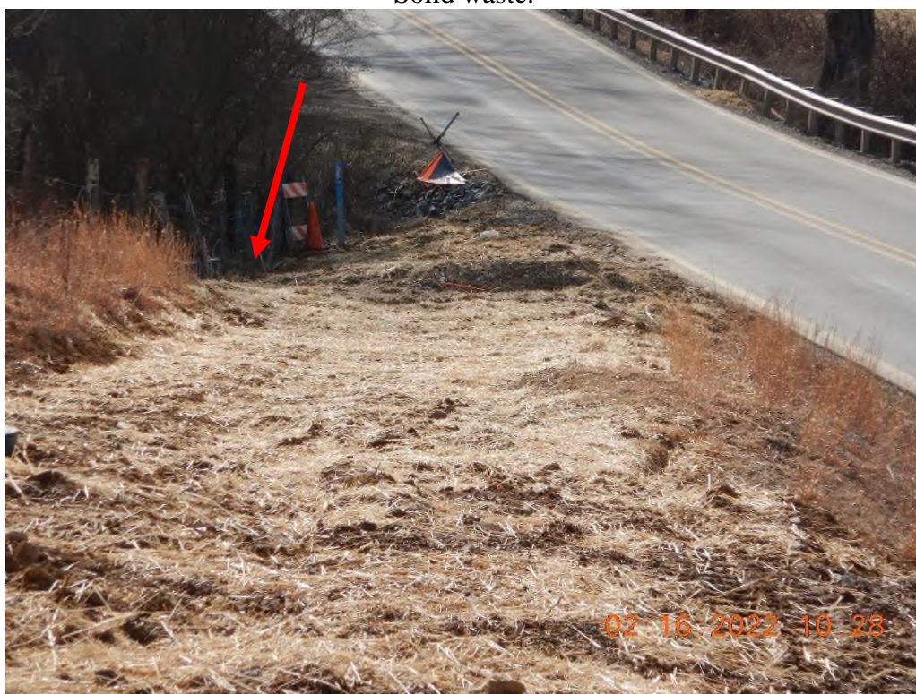
Area where the SWPPP was not modified to add perimeter controls.
