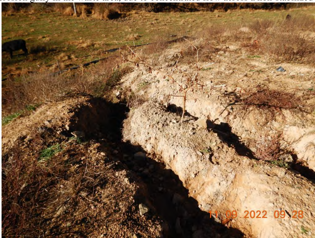
Erosion gullies in the waste area.
