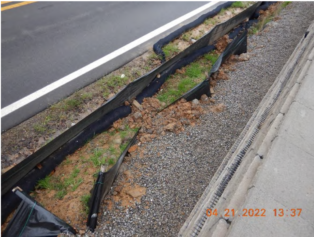
Silt fence needed maintenance.
