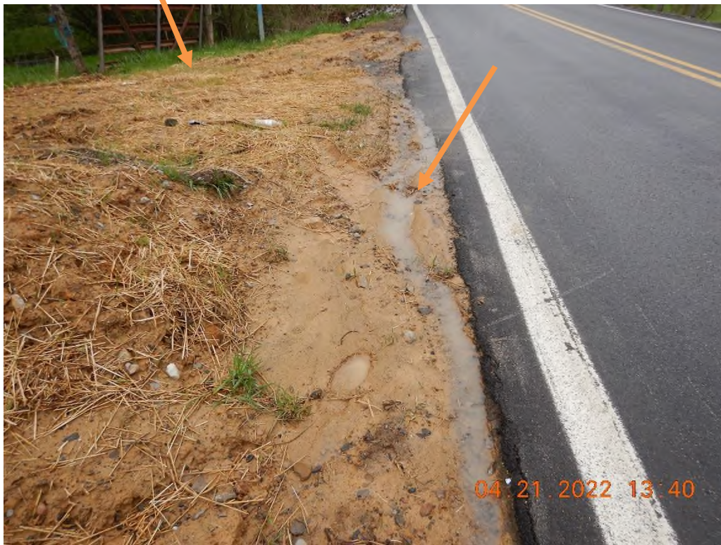
Sediment and sediment laden water leaving the site. The southern portion of the site was not within the permitted LOD, and the SWPPP has not been modified to add perimeter controls.
