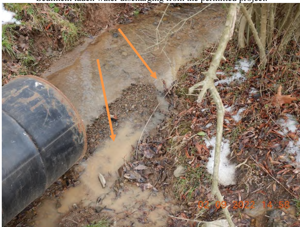
The sediment laden water that left the site discharged into an ephemeral stream (UNT of Little Tenmile Creek) causing Conditions Not Allowable in waters of the state (39° 23'27.70" N, -80° 27'41.69" W).
