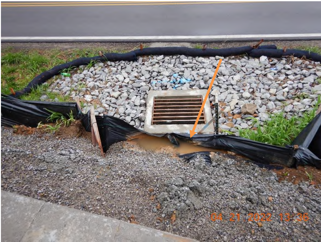
Silt fence in a concentrated flow area.
