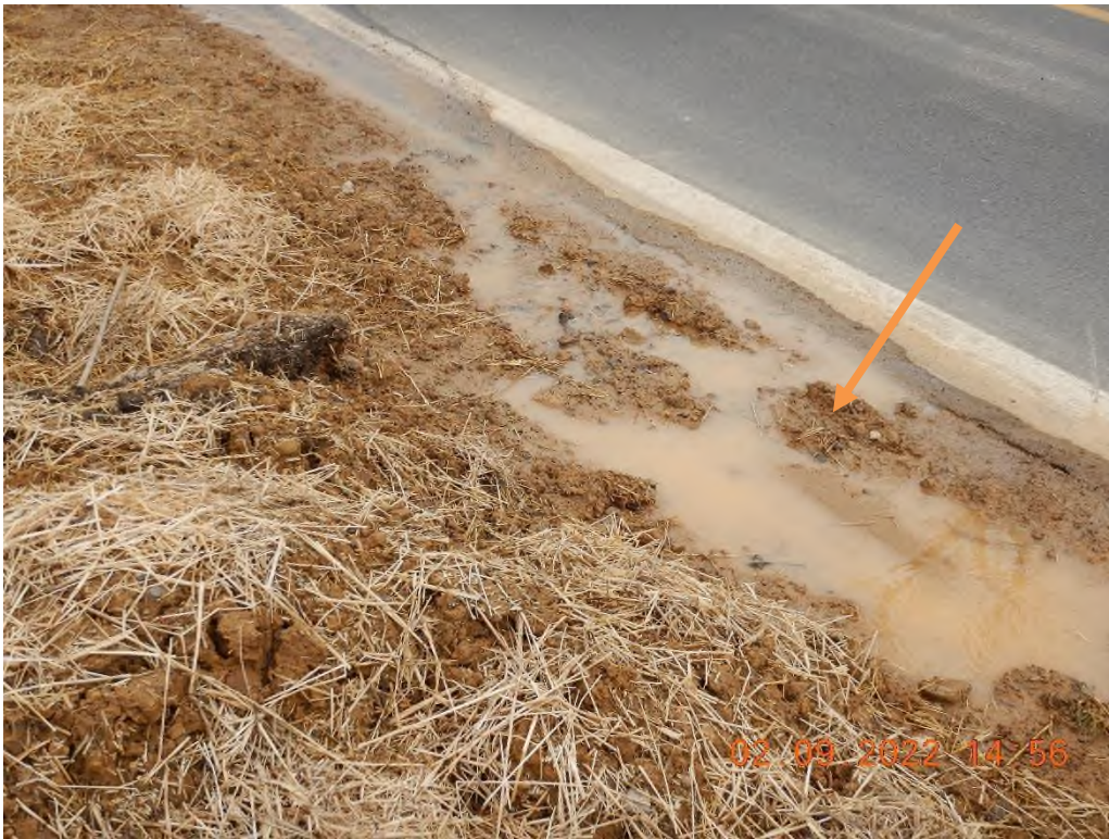
The area on the southern portion where perimeter controls are not required by the SWPPP; however, sediment laden water was leaving the site.
