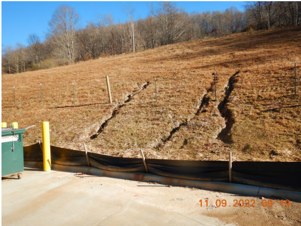
Erosion gullies near the earthen slip area, due to concentrated flow across a non-stabilized surface.
