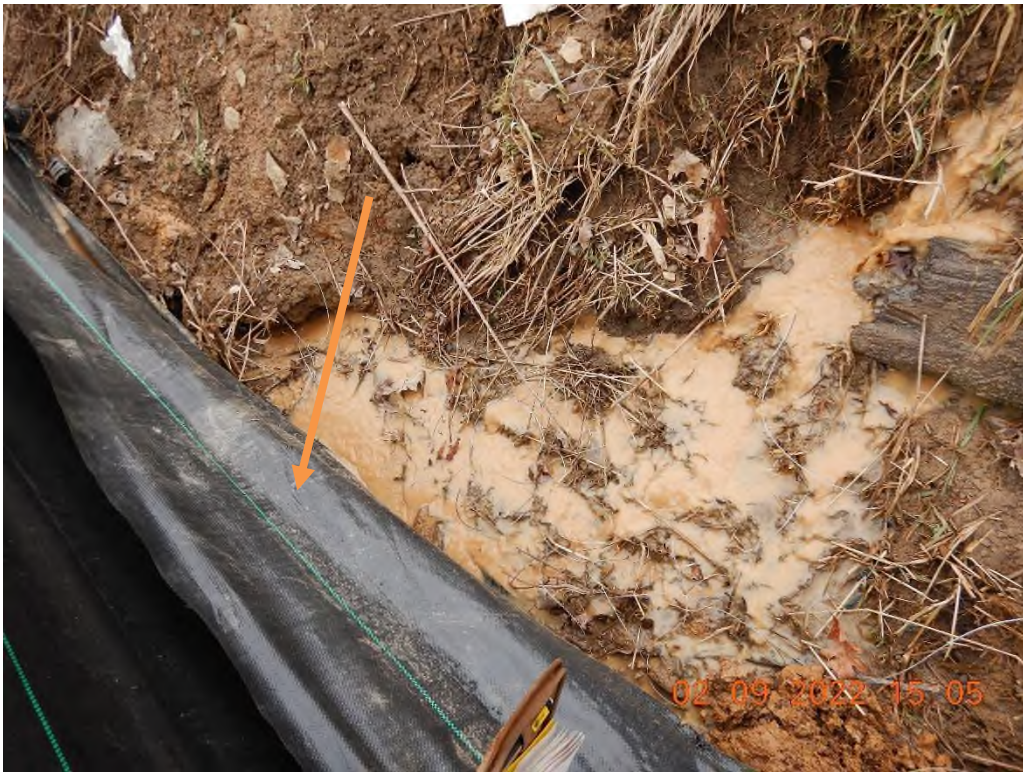
Silt fence was not properly toed-in, and sediment laden water can bypass treatment and leave the site.
