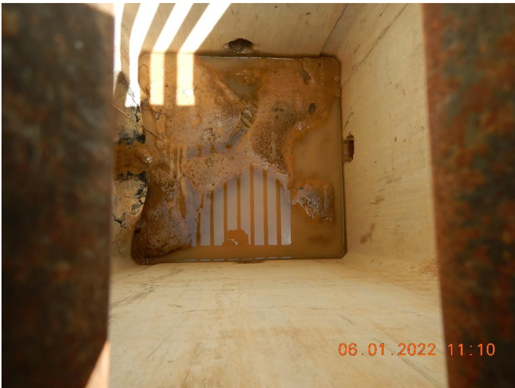
Sediment laden water and sediment deposits in the bottom of the drop inlet, as a result of improper implementation of silt fence.
