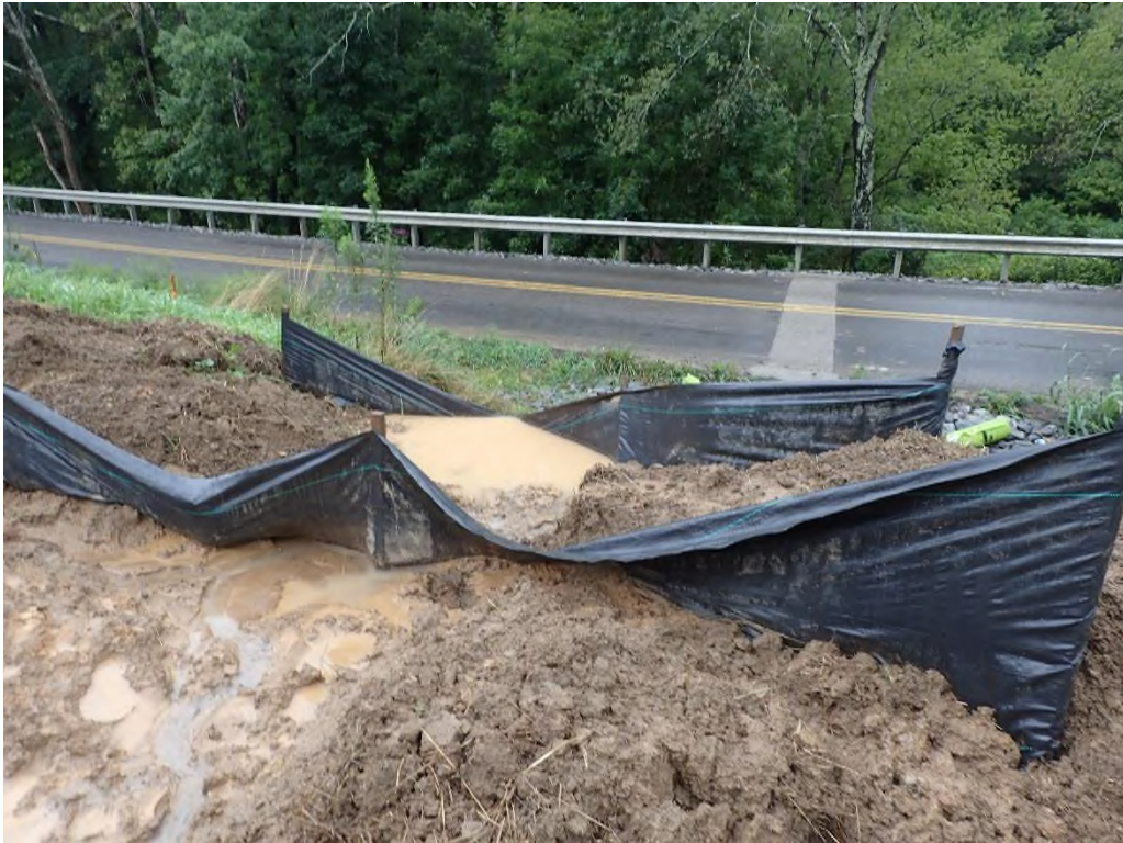
Photo 4: Silt fence overwhelmed with turbid water.
