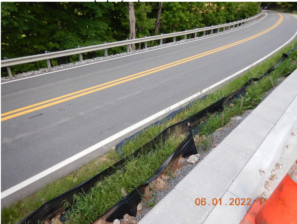
Perimeter controls needed maintenance.
