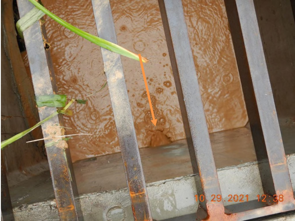
Sediment laden water entering the adjacent drop inlet
