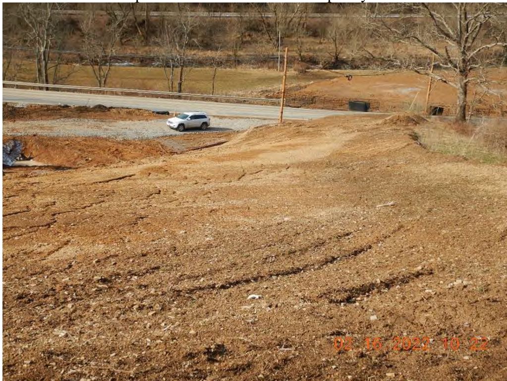
The slip area, showing the lack of temporary stabilization.
