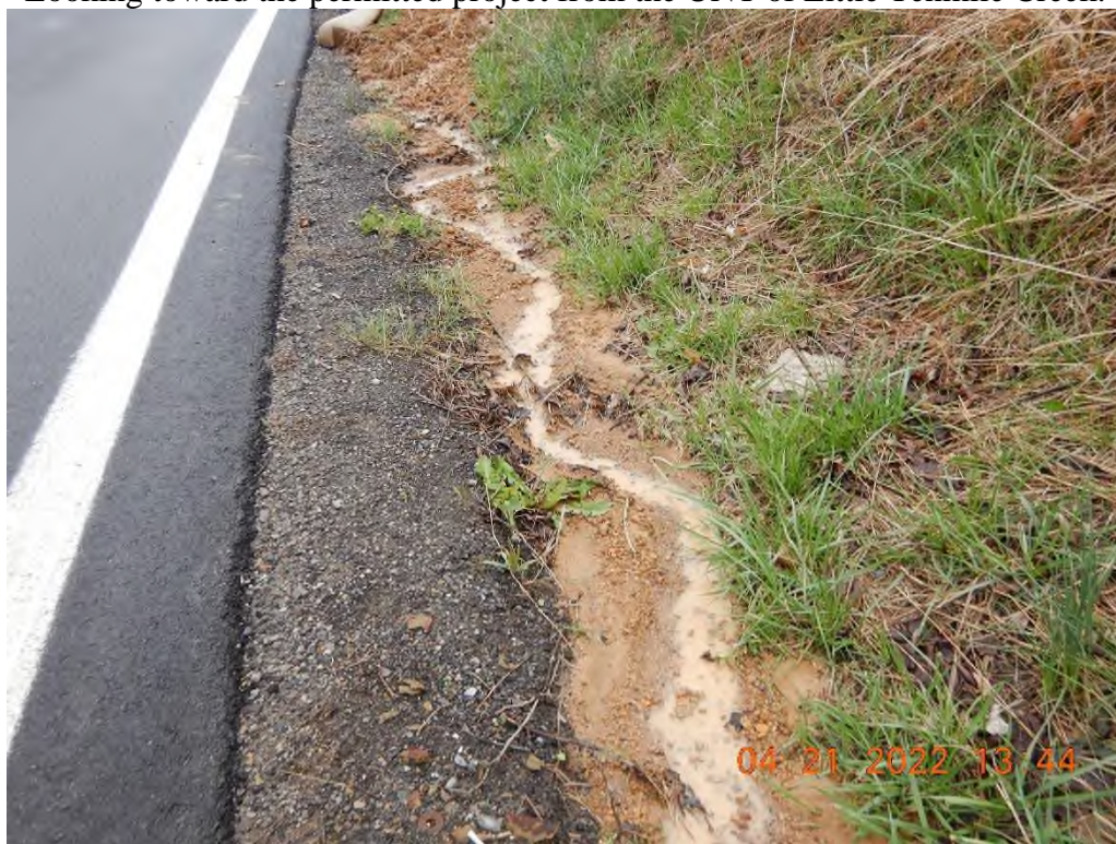
The ditch and the sediment and sediment laden water that has discharged into it.
