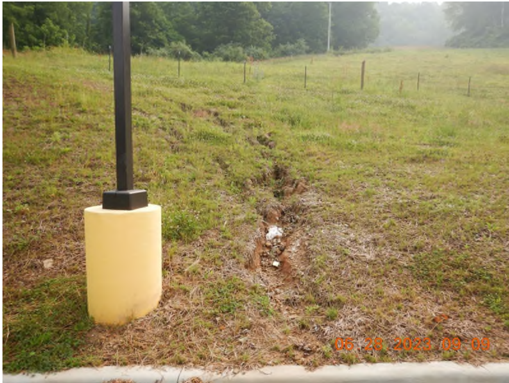
An erosion gully noted near the earthen slip portion of the site. This is due to a concentrated flow going across a non-stabilized surface.
