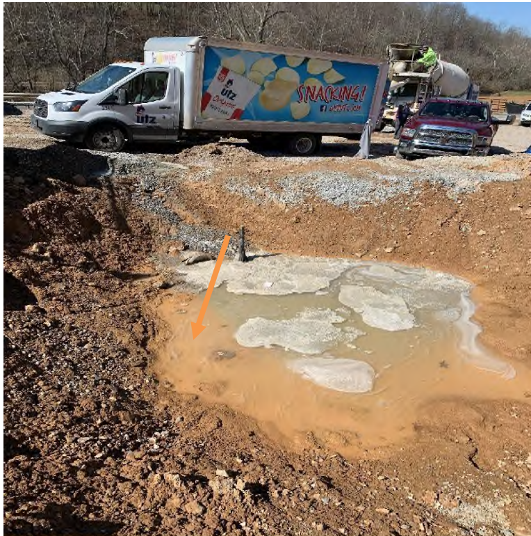
The area where Sediment Trap 1 should have been installed. Concrete is being washed into the proposed Sediment Trap 1 area. The orange arrow indicates the culvert inlet that discharges toward a drop inlet adjacent to the project.
