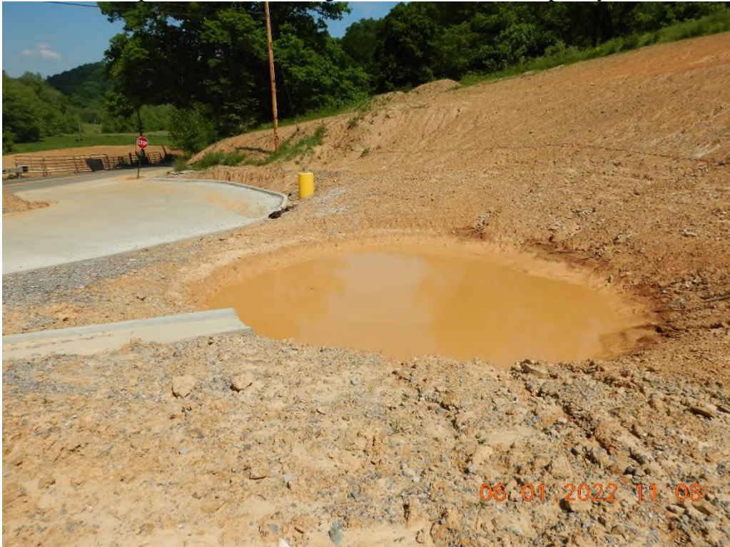
Sediment Trap 1 is not functional or fully installed.
