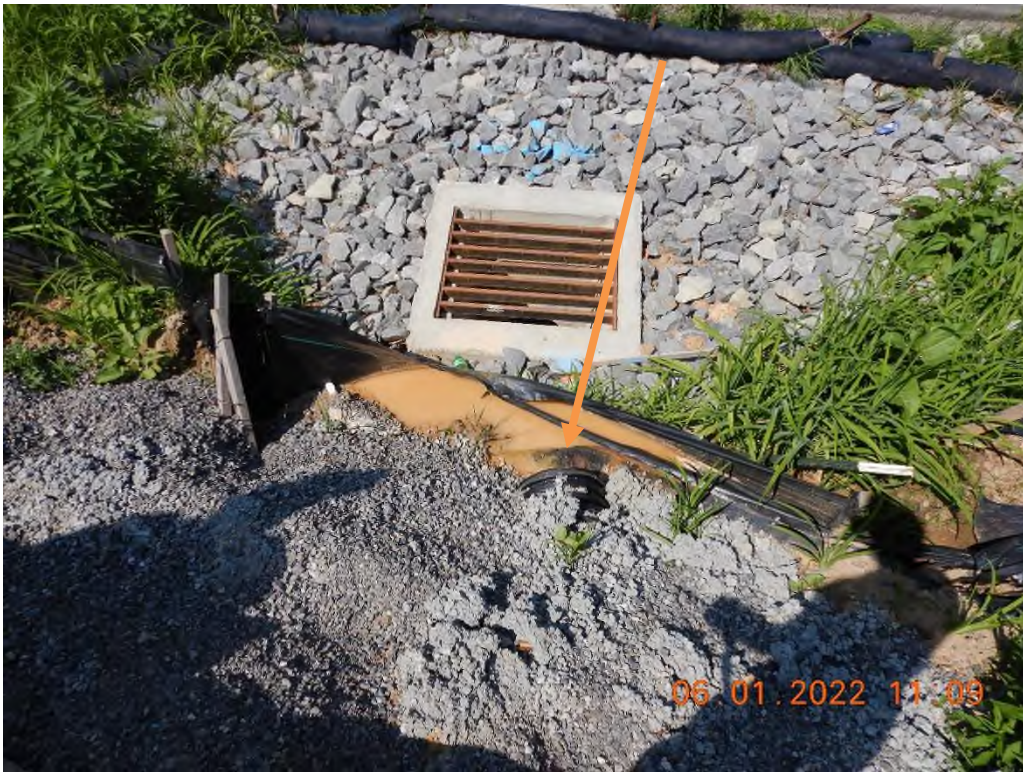
Silt fence installed in a concentrated flow area at the outlet of non-functional Sediment Trap 1.
