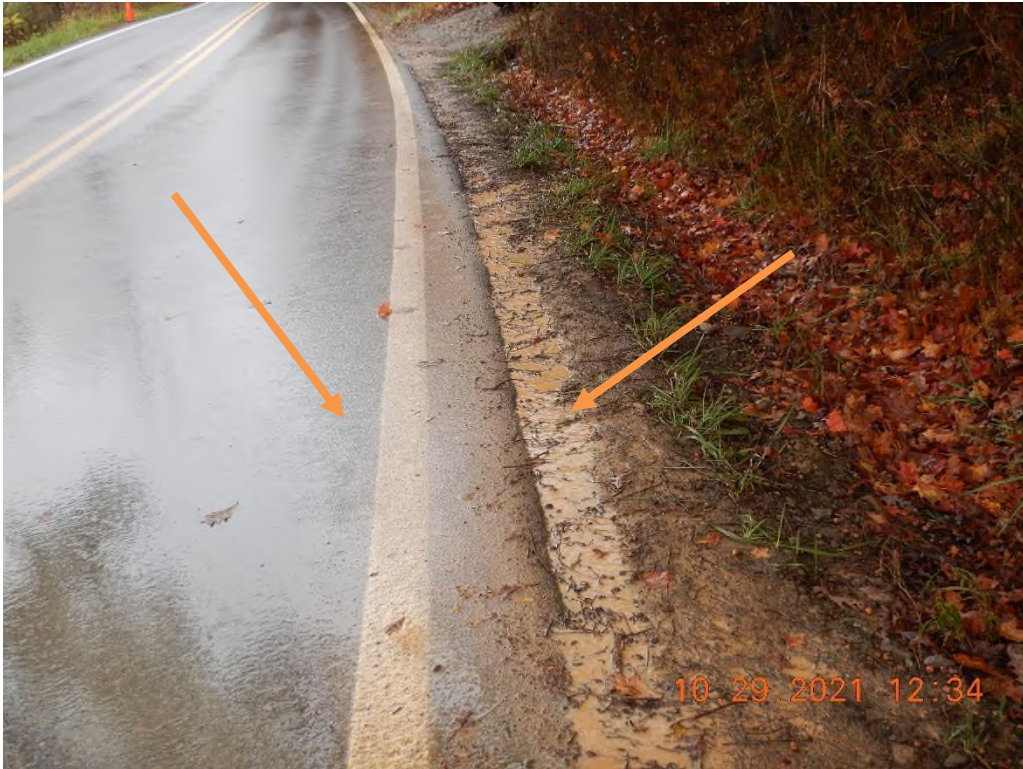
Sediment laden water leaving the project and traveling down the ditch line and across Rt. 20.
