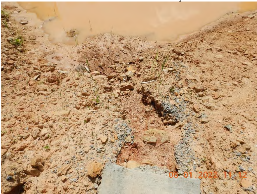
An unstable inlet for Sediment Trap 2.
