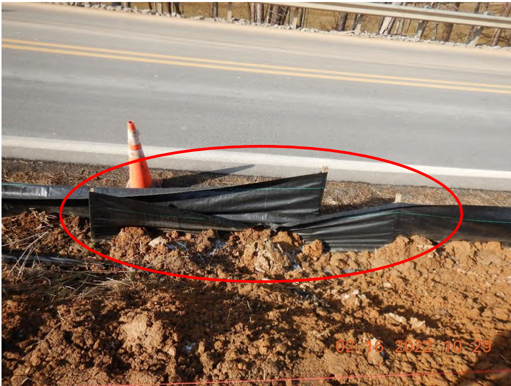
Perimeter controls not properly implemented.
