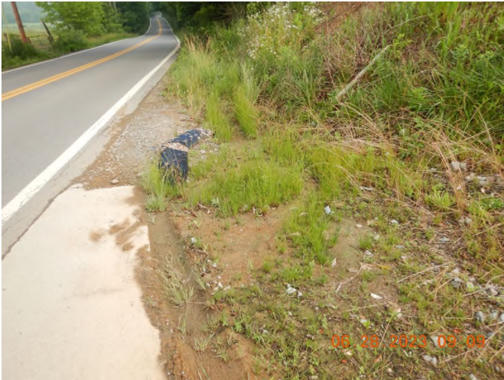
Compost filter sock showing the need for maintenance. As shown, sediment and sediment laden water from the project have bypassed treatment and left the site.
