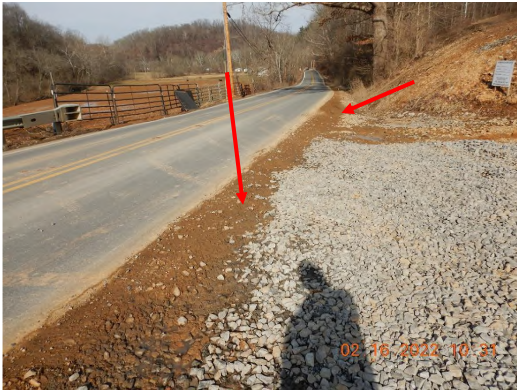
Sediment laden water leaving the site at the unstabilized construction entrance.
