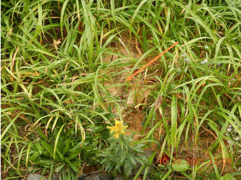
The path of sediment laden water leaving the site.
