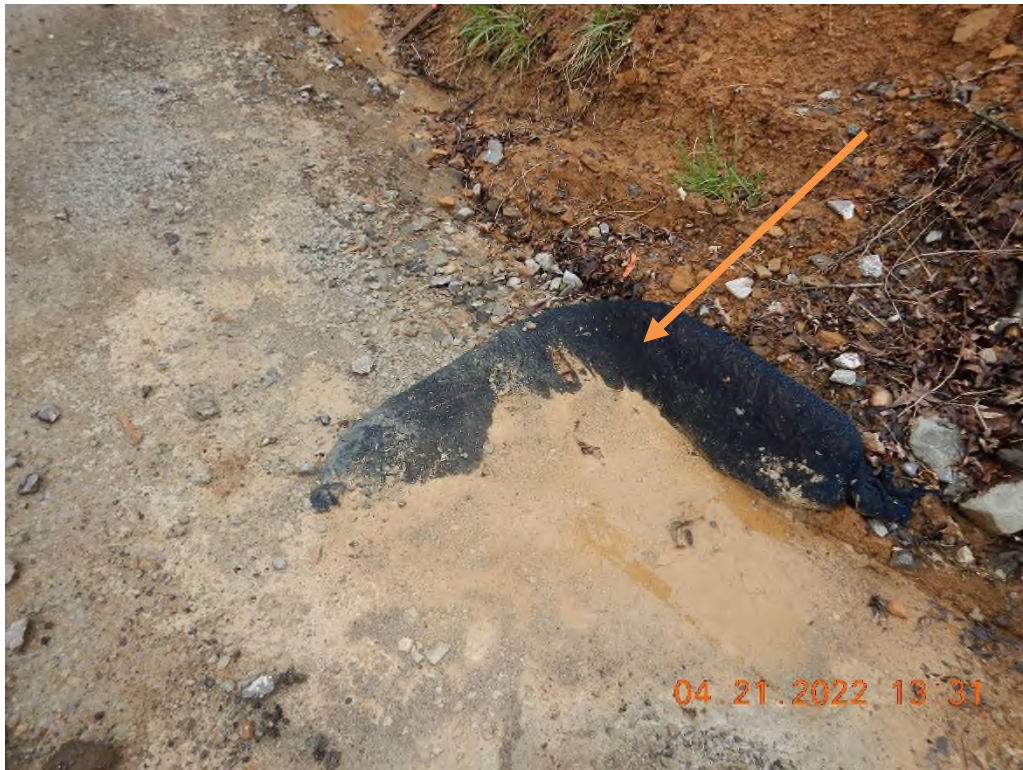
A compost filter sock that was not properly implemented and required staking.
