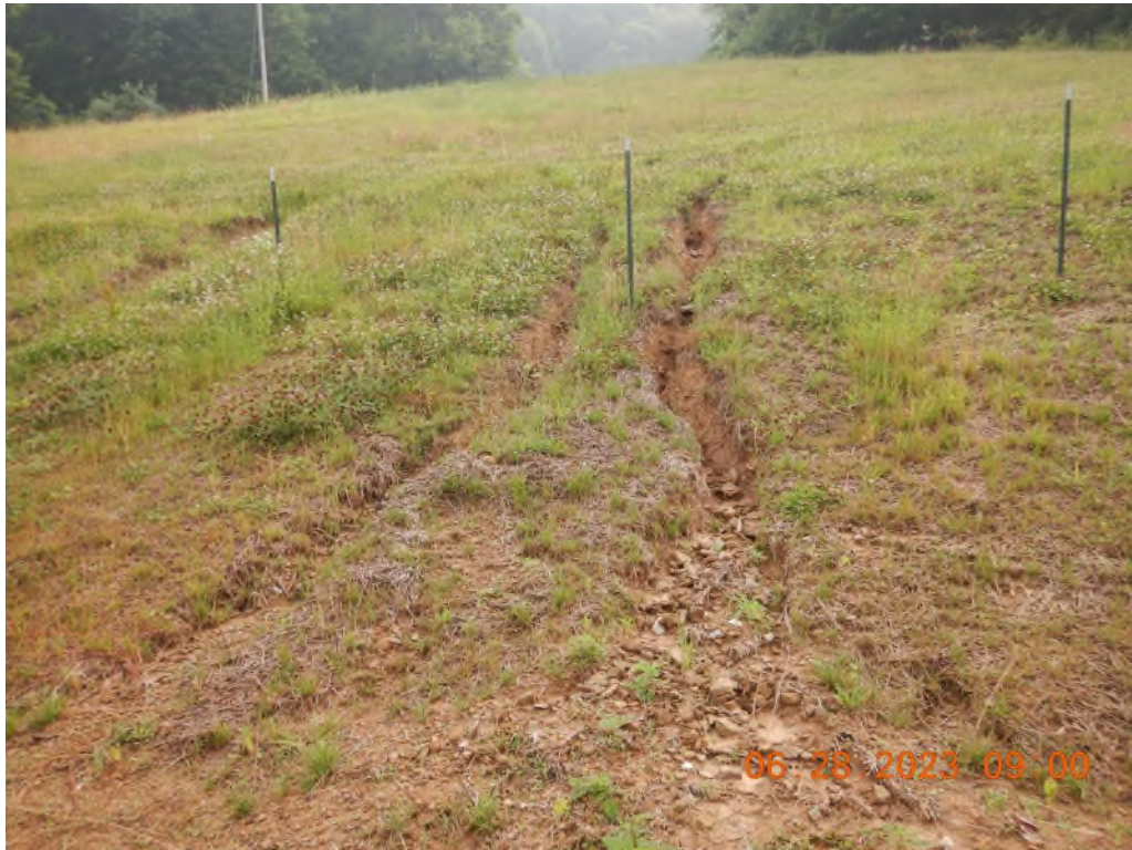
More erosion gullies noted near the earthen slip portion of the site. This is due to a concentrated flow going across a non-stabilized surface.
