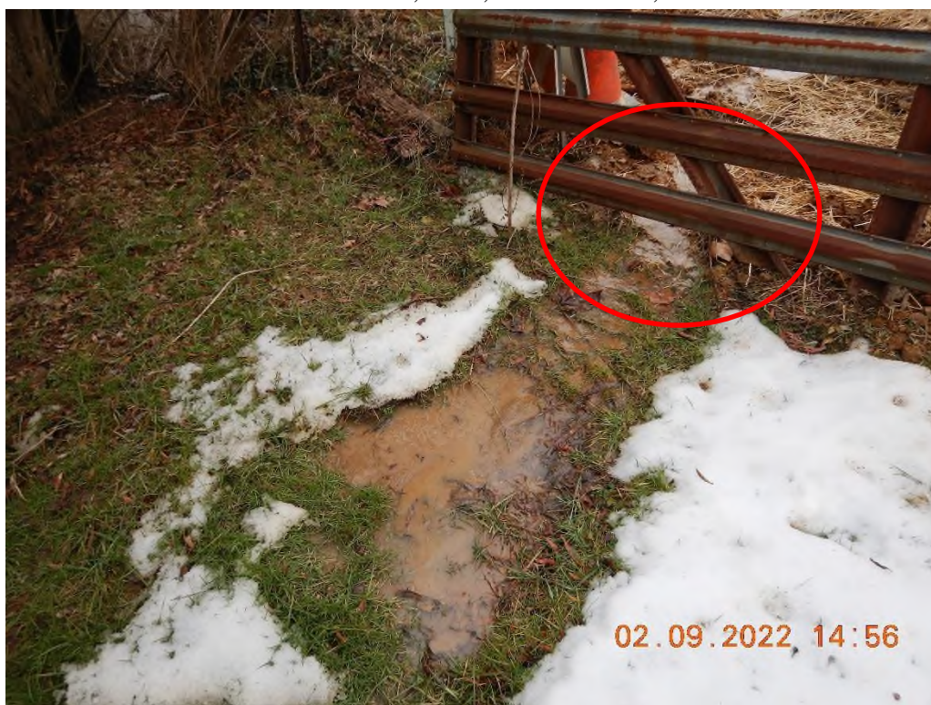
Sediment laden water discharging from the permitted project.
