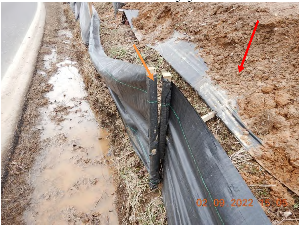
Silt fence was not properly merged (orange arrow) and needed maintenance (red arrow).
