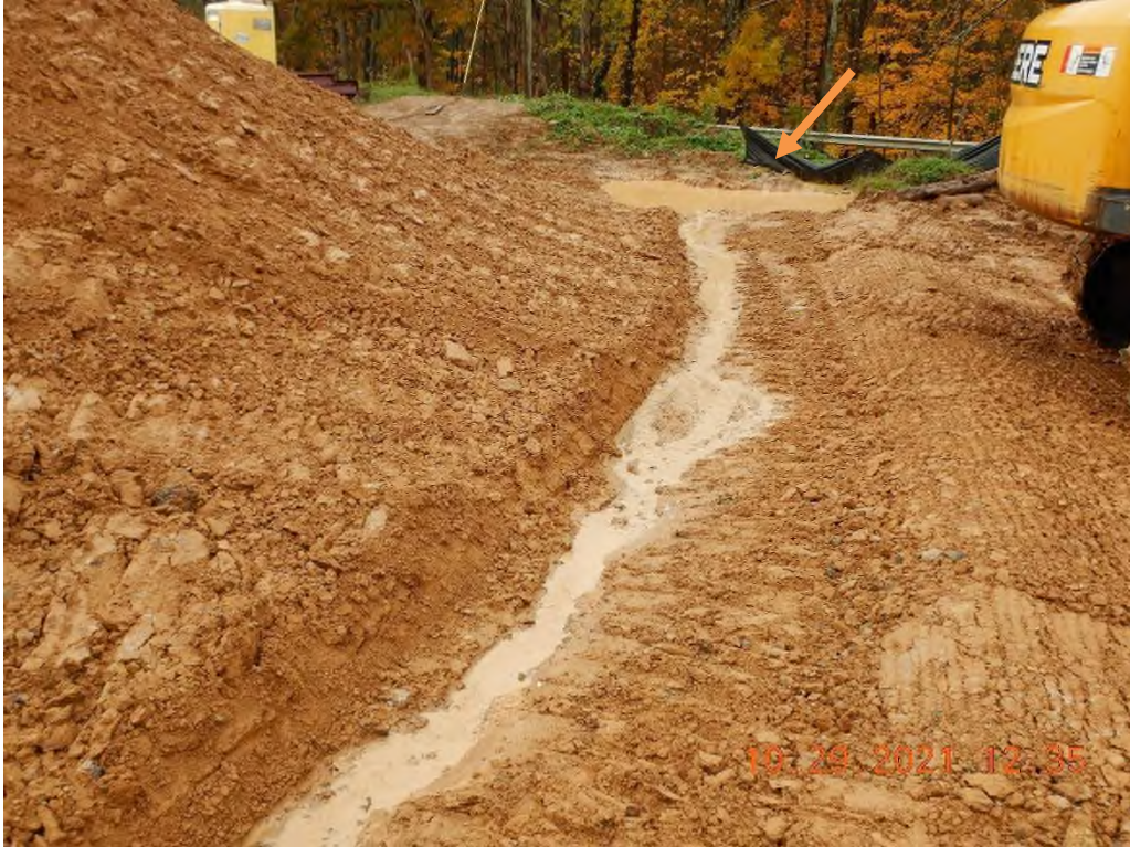
The orange arrow indicates silt fence that is in need of maintenance.
