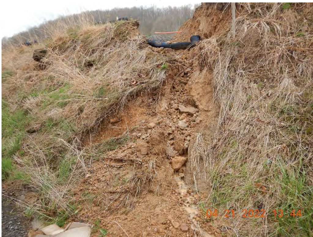
The unstable outlet of Sediment Trap 2.
