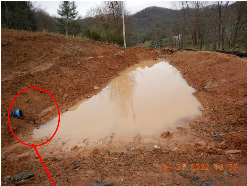
Proposed Sediment Trap 2 with an unstable inlet/outlet.
