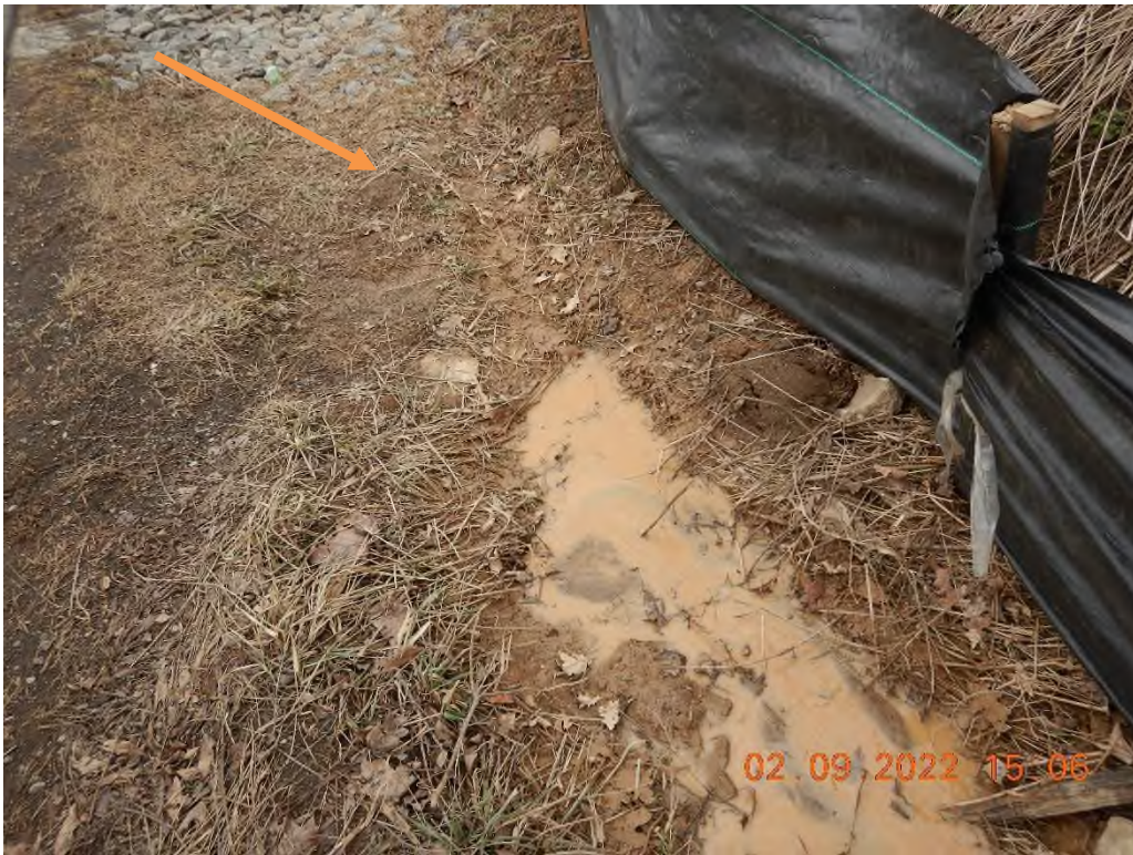
Sediment laden water entering an underdrain and leaving the site.
