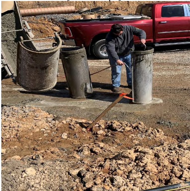
Washing concrete onto the ground, allowing it to integrate with storm water.
