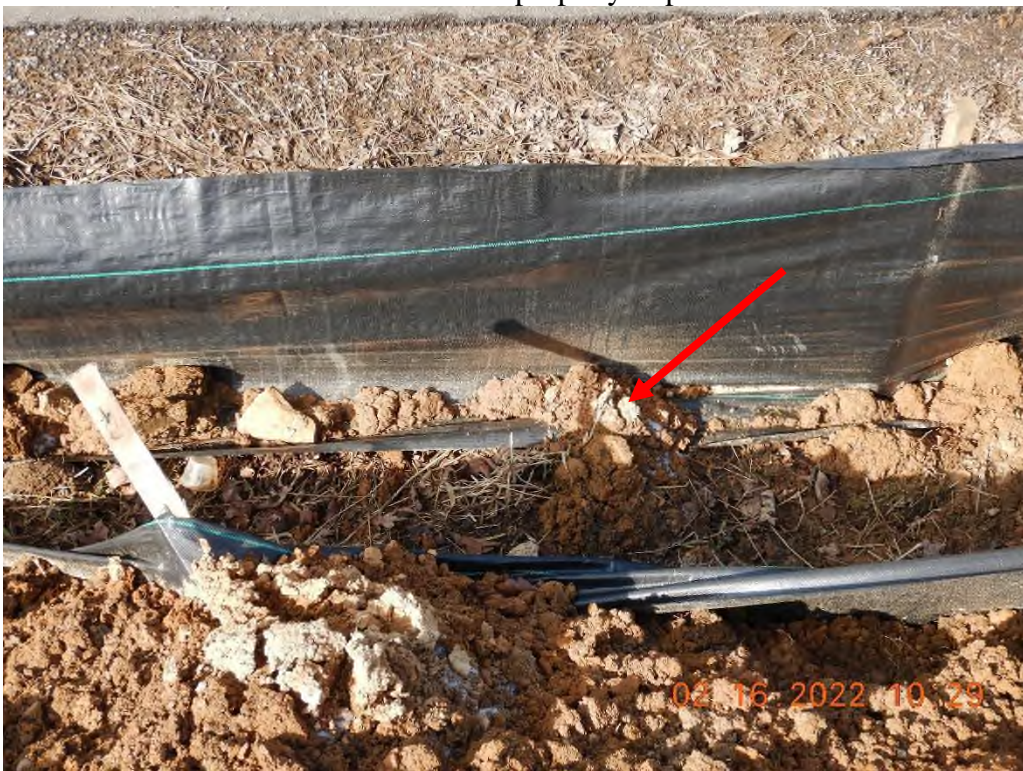
Silt fence not properly toed into the ground.
