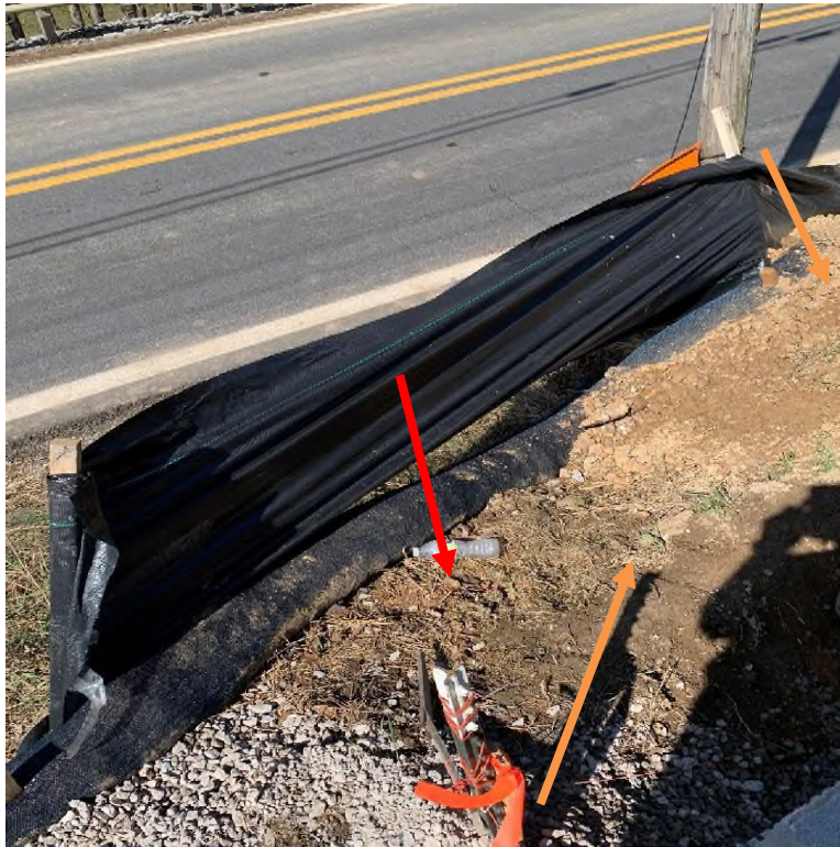
Compost filter sock that is in need of maintenance (orange arrow) and silt fence that was not properly implemented (red arrow).
