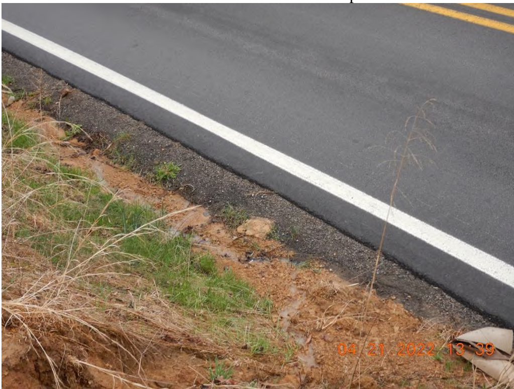
Sediment and sediment laden water in the adjacent ditch.
