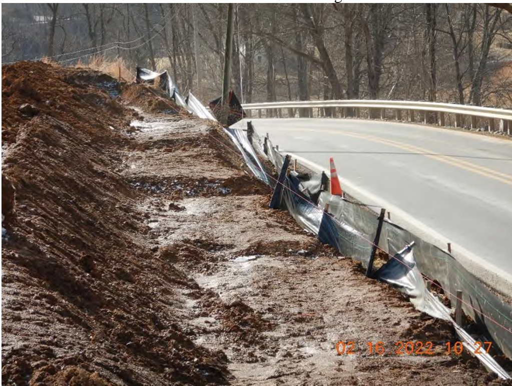
Multiple pieces of silt fence needed maintenance.
