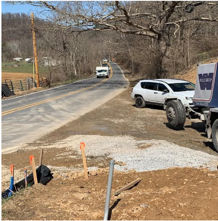
The non-stabilized construction entrance, with track-out onto a public roadway (WV-20).
