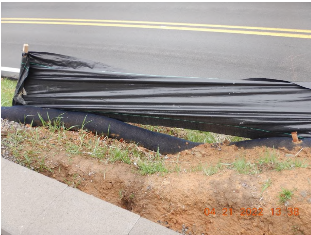
Silt fence was not properly toed into the ground.
