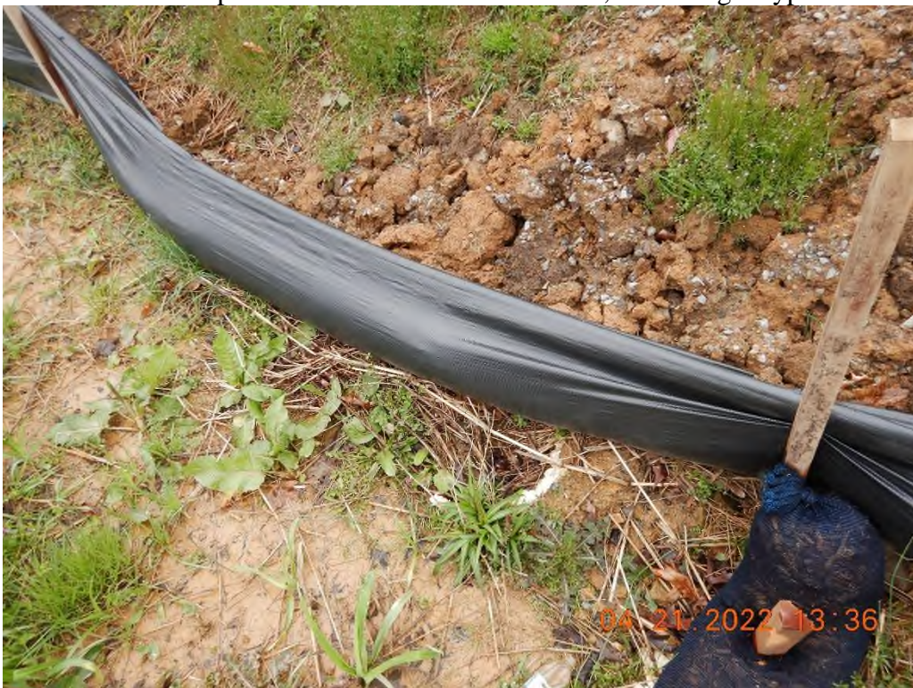
Silt fence needed maintenance.
