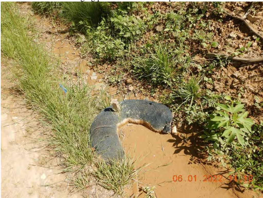
Sediment bypassing the compost filter sock, which needed maintenance.
