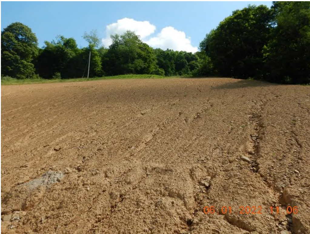
The earthen slip area, with erosion gullies and a lack of temporary stabilization.
