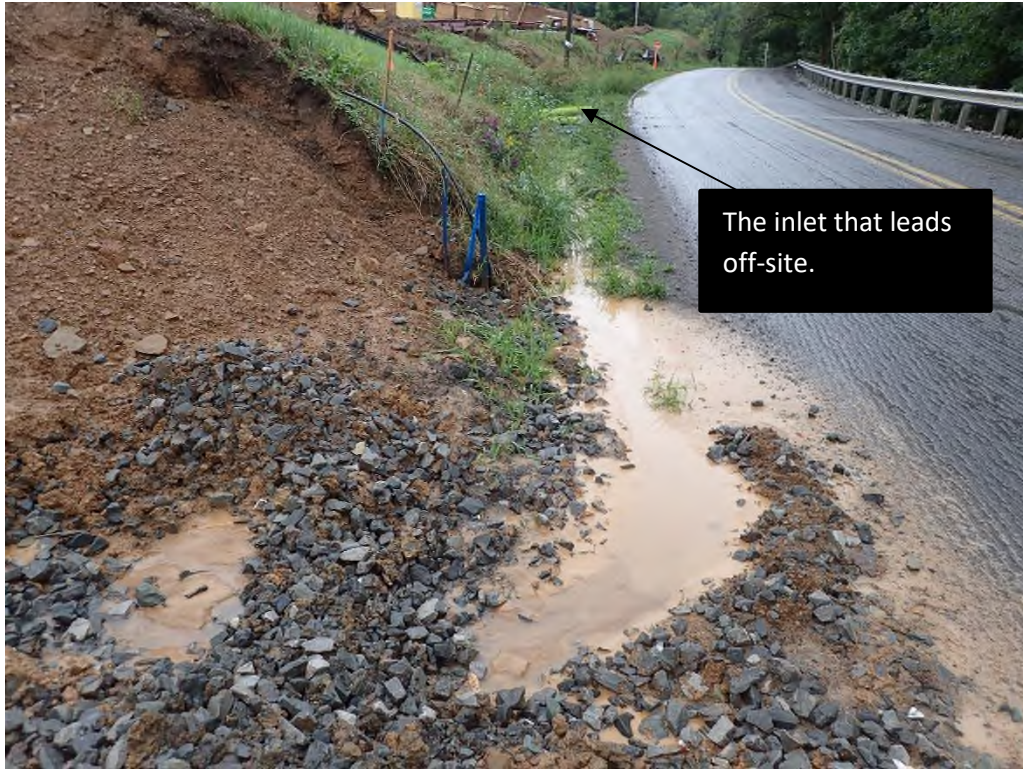
Photo 1: The ditch conveying turbid water toward the inlet.
