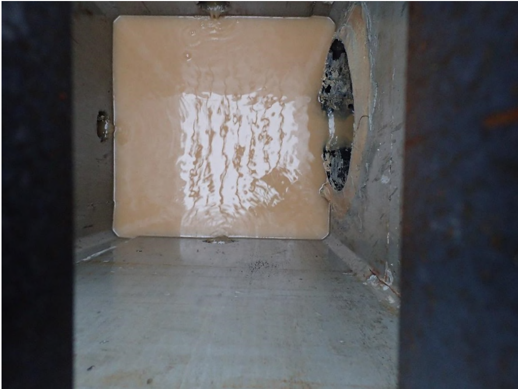
Photo 2: Turbid water inside the inlet that leads underneath Rt. 20 and discharges off-site.
