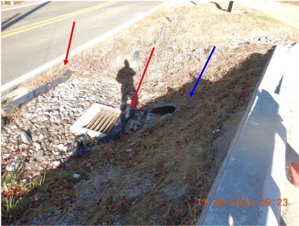
The red arrows show compost filter socks lacking the required staking, and the blue arrow shows the outlet of Sediment Trap 1 with no marker.
