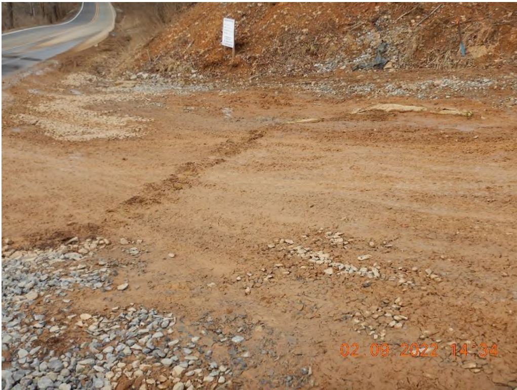
A non-stabilized construction entrance.
