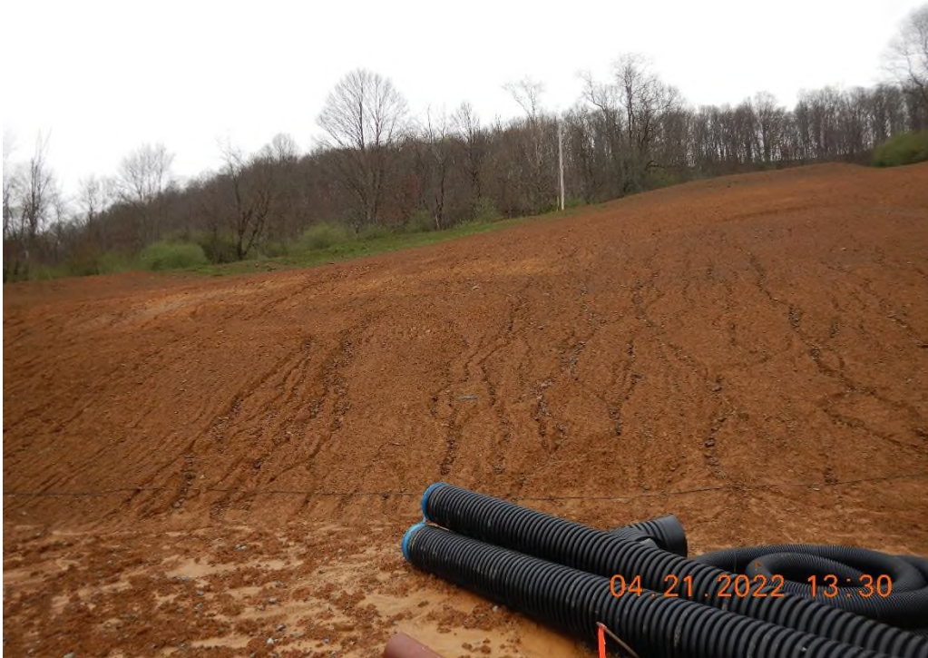
The earthen slip area on the eastern portion of the site, with no temporary stabilization.
