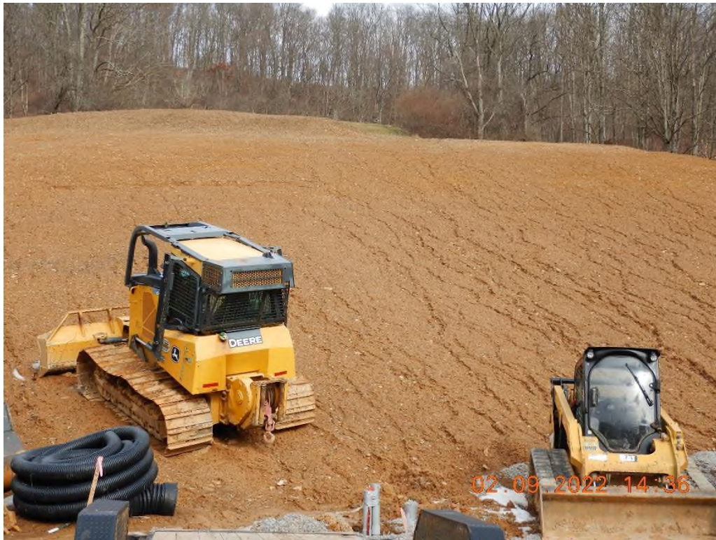
The eastern portion of the site, where there is no temporary stabilization.
