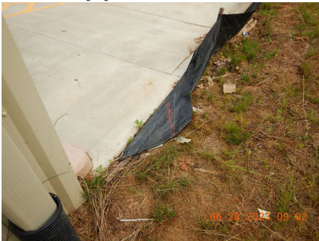
Silt fence installed near the building and parking area is in need of maintenance.
