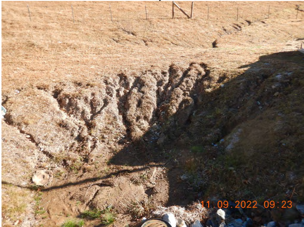
Unstable inlets to Sediment Trap 1.
