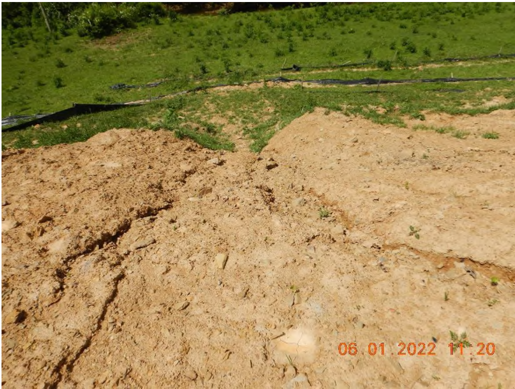
The waste area with a lack of temporary stabilization and erosion gullies. Silt fence needed maintenance.
