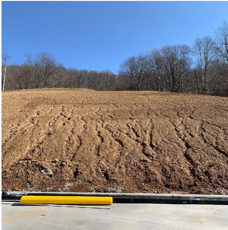
Earthen slip area on the eastern portion of the site, without temporary stabilization.
