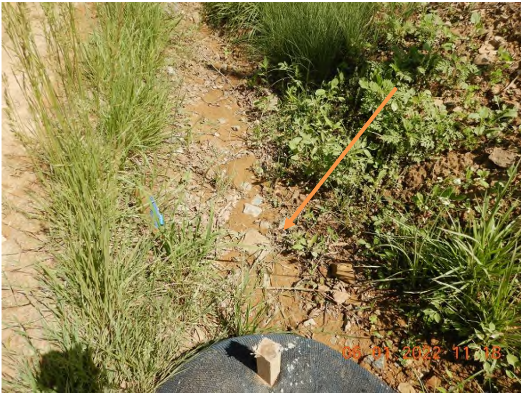
Sediment discharging past the installed compost filter sock check.
