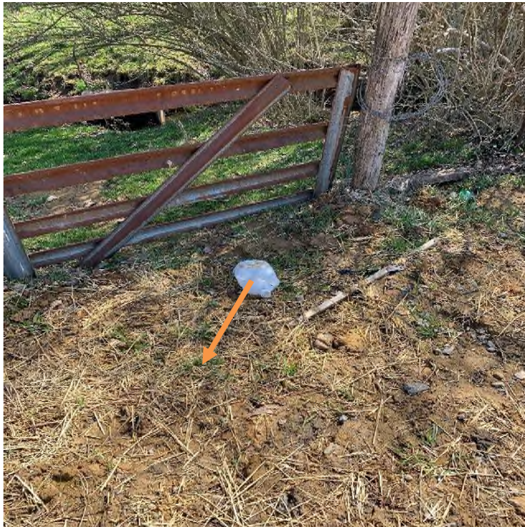
Perimeter controls are not in place, and sediment deposits were present beyond the permitted LOD; however, the SWPPP had not been modified.
