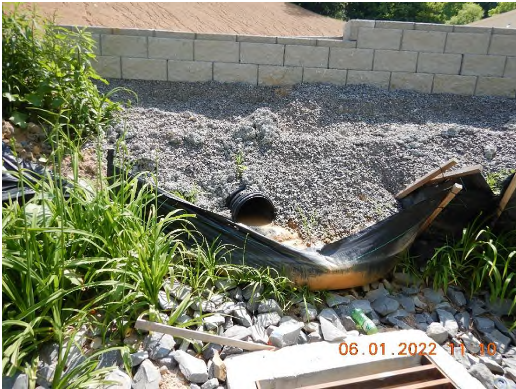
Improperly implemented silt fence.
