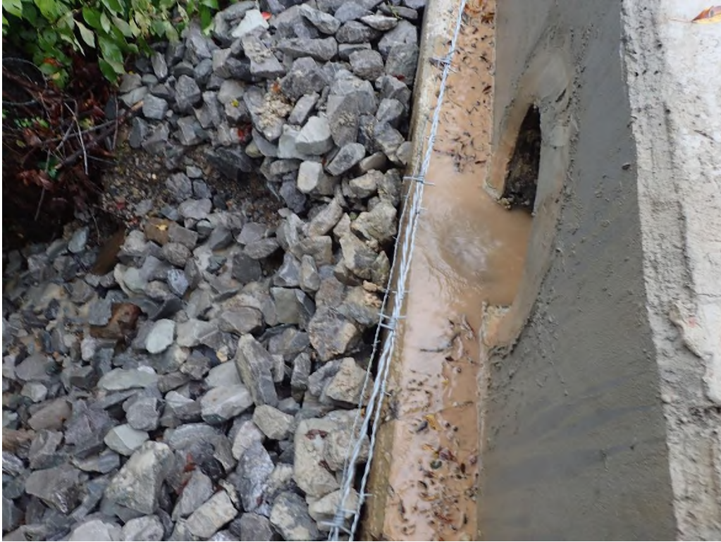
Photo 3: The outlet that discharges to Little Tenmile Creek. Turbid water was being discharged.
