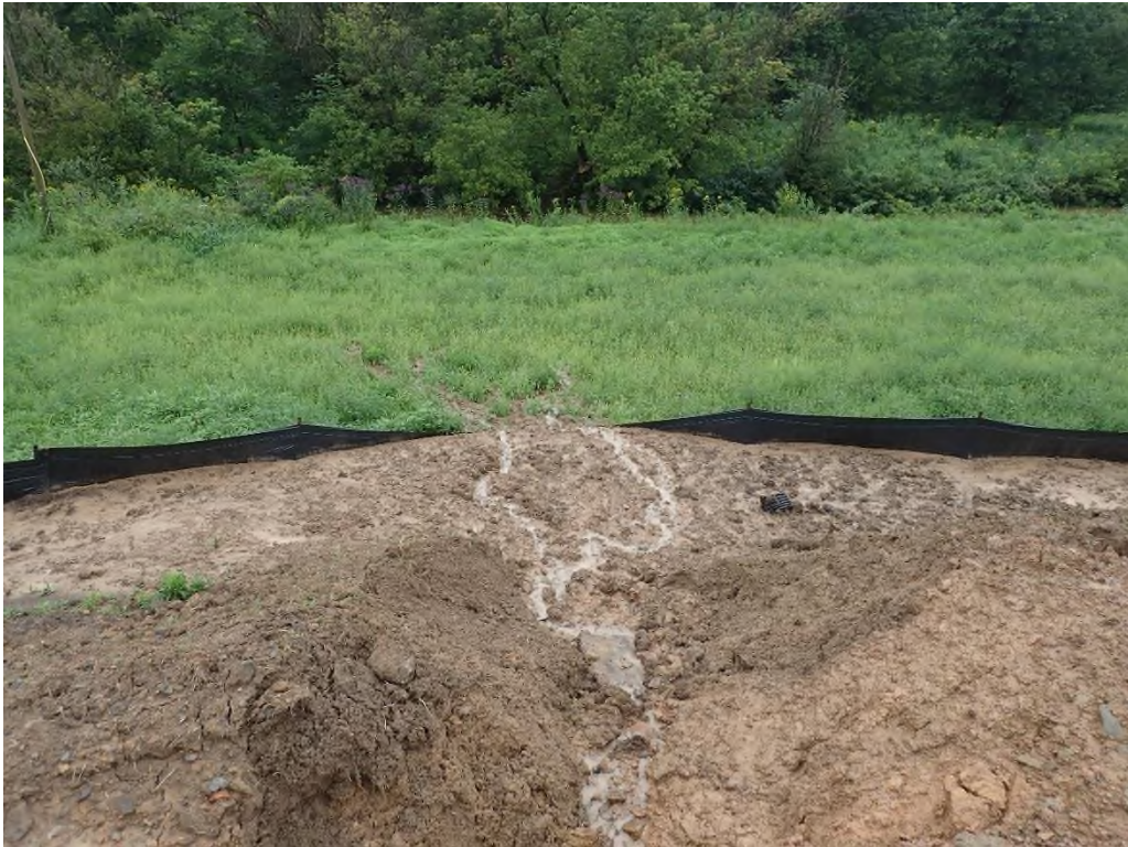
Photo 6: Silt fence overwhelmed at the waste area across the road from the site.
