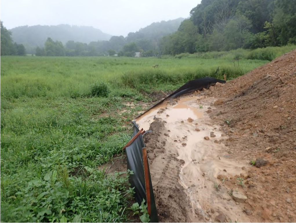
Photo 7: Silt fence is being overwhelmed, and sediment is being discharged into the adjacent field.
