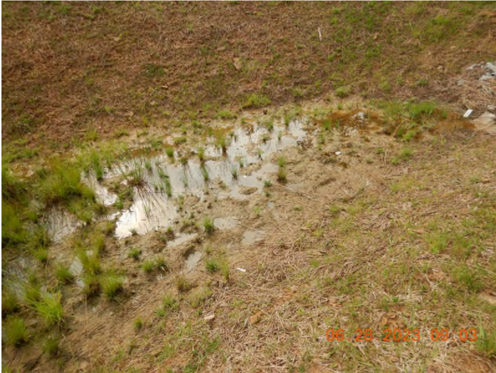
Sediment Trap 2 not holding the required 50% wet storage as required.
