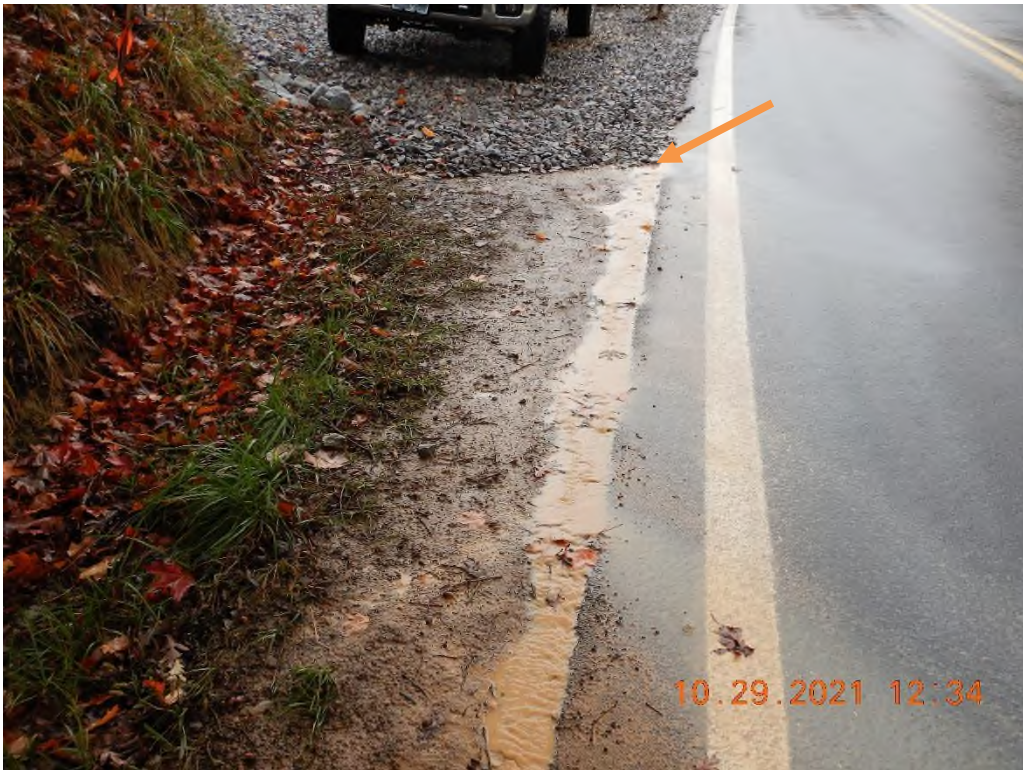
Sediment laden water leaving the site.
