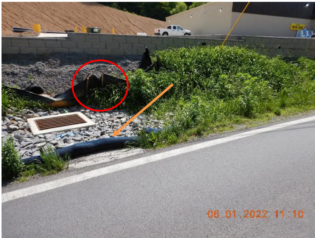
Perimeter controls that were not properly merged. Compost filter sock is missing the required staking.
