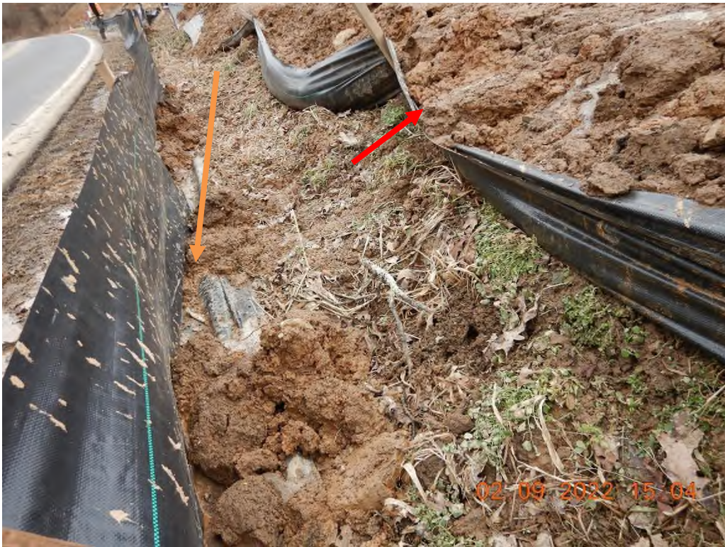
Silt fence that was not properly toed-in (orange arrow) and is in need of maintenance (red arrow).
