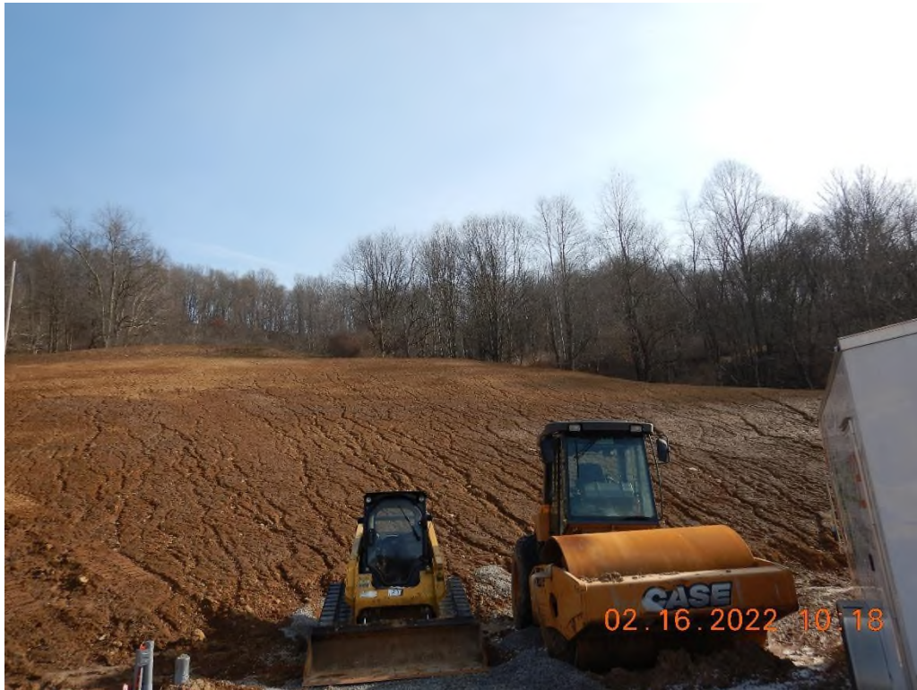
The eastern portion of the site with no temporary stabilization.
