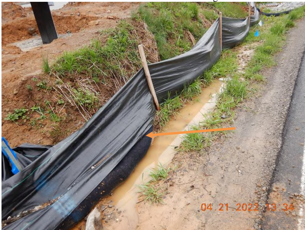
Silt fence was not toed into the ground.
