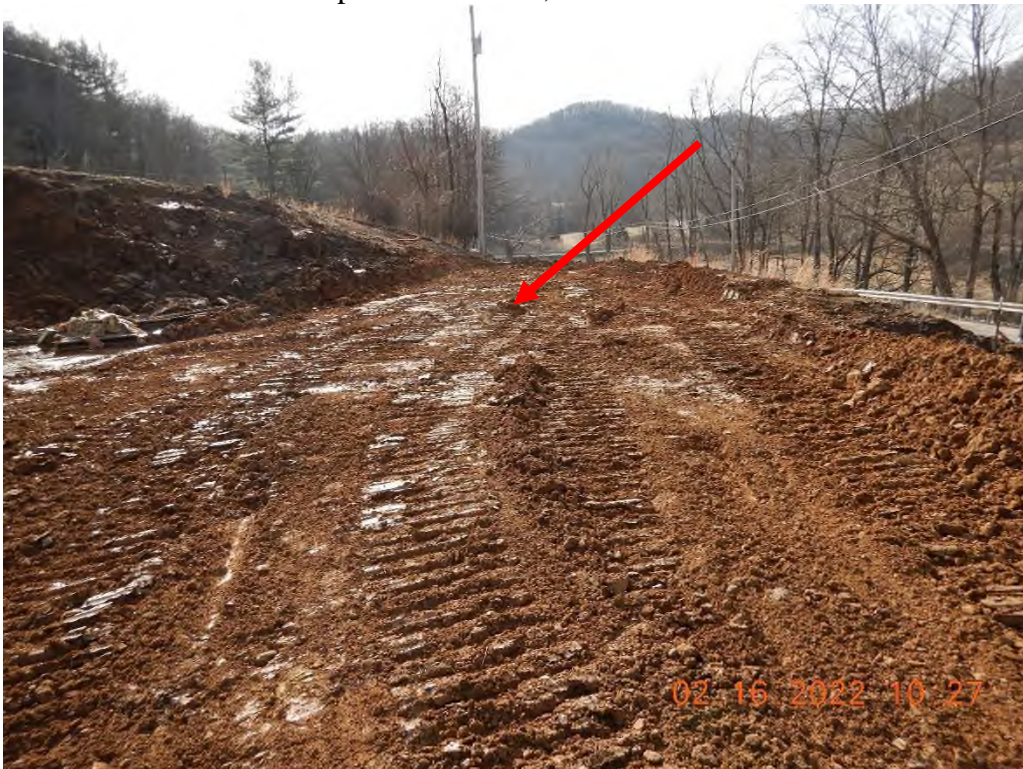
Sediment Trap 2 not installed, as stated in the SWPPP.
