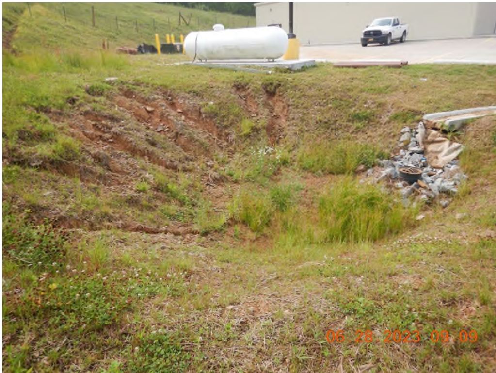
Unstable inlets traversing into Sediment Trap 1. Also shown is a lack of a 50% wet storage as required in the SWPPP.
