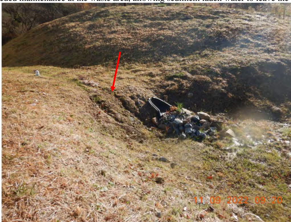
An unstable inlet to Sediment Trap 2.
