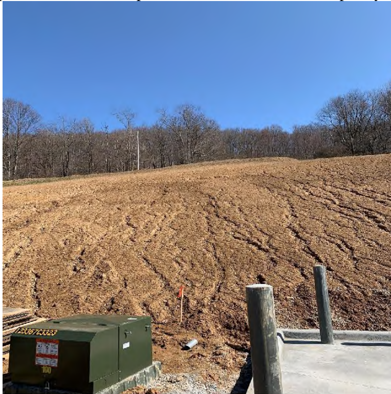
A continuation of the earthen slip area that has not been temporarily stabilized.
