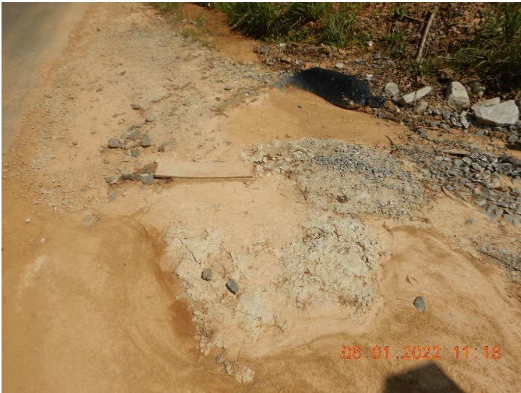
Compost filter sock check needed maintenance.
