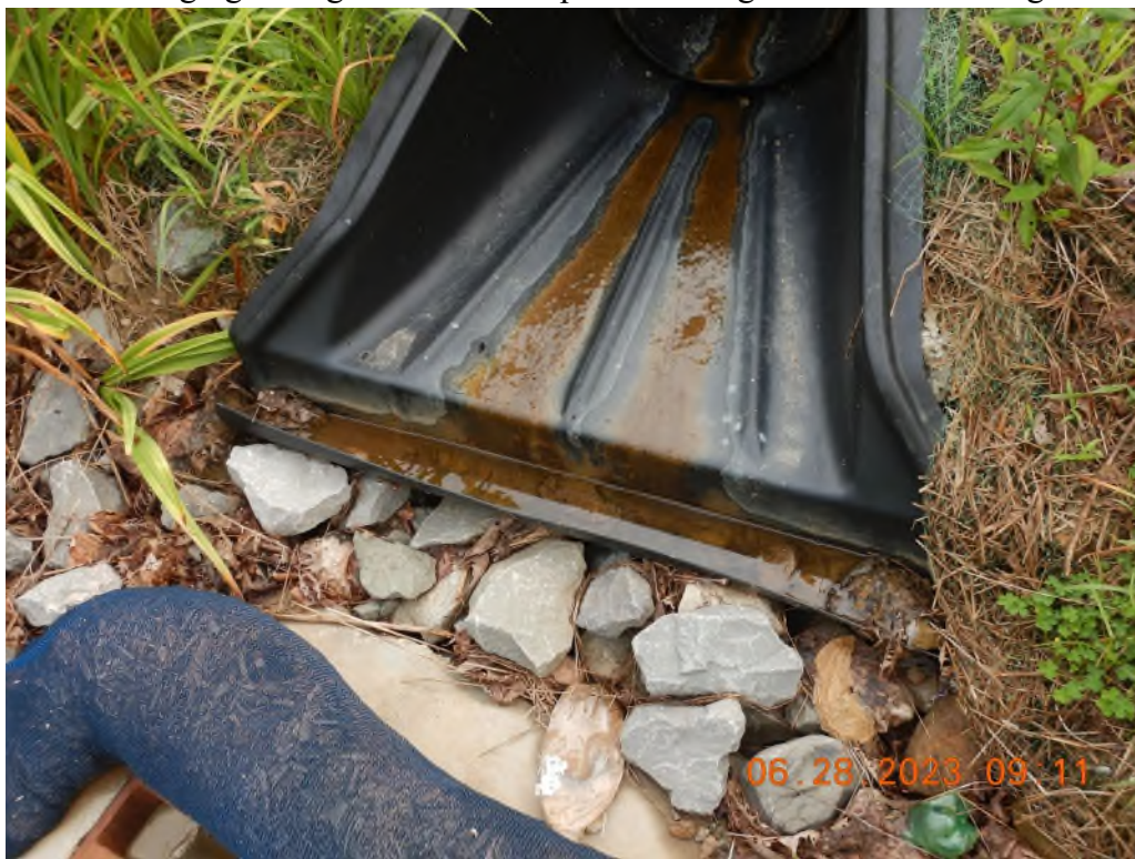
No outlet marker in place at the outlet of Sediment Trap 1.
