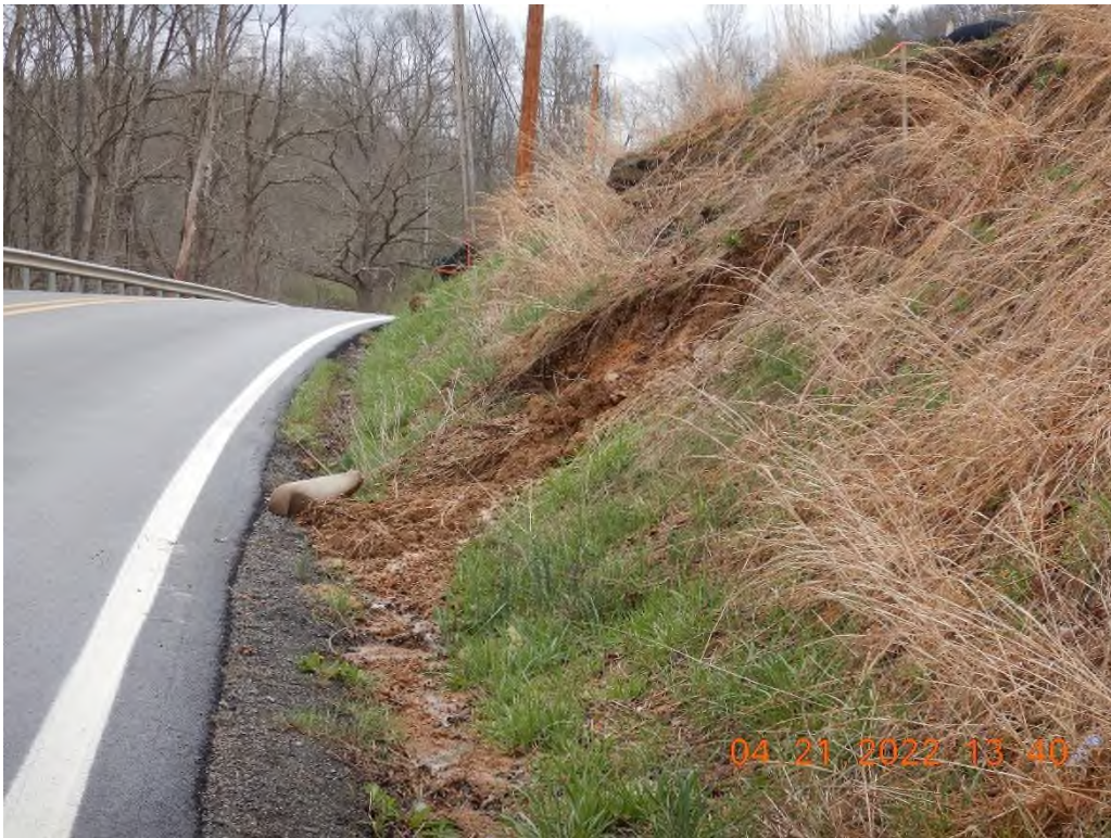
Unstable outlet from the adjacent ditch, with sediment and sediment laden water.
