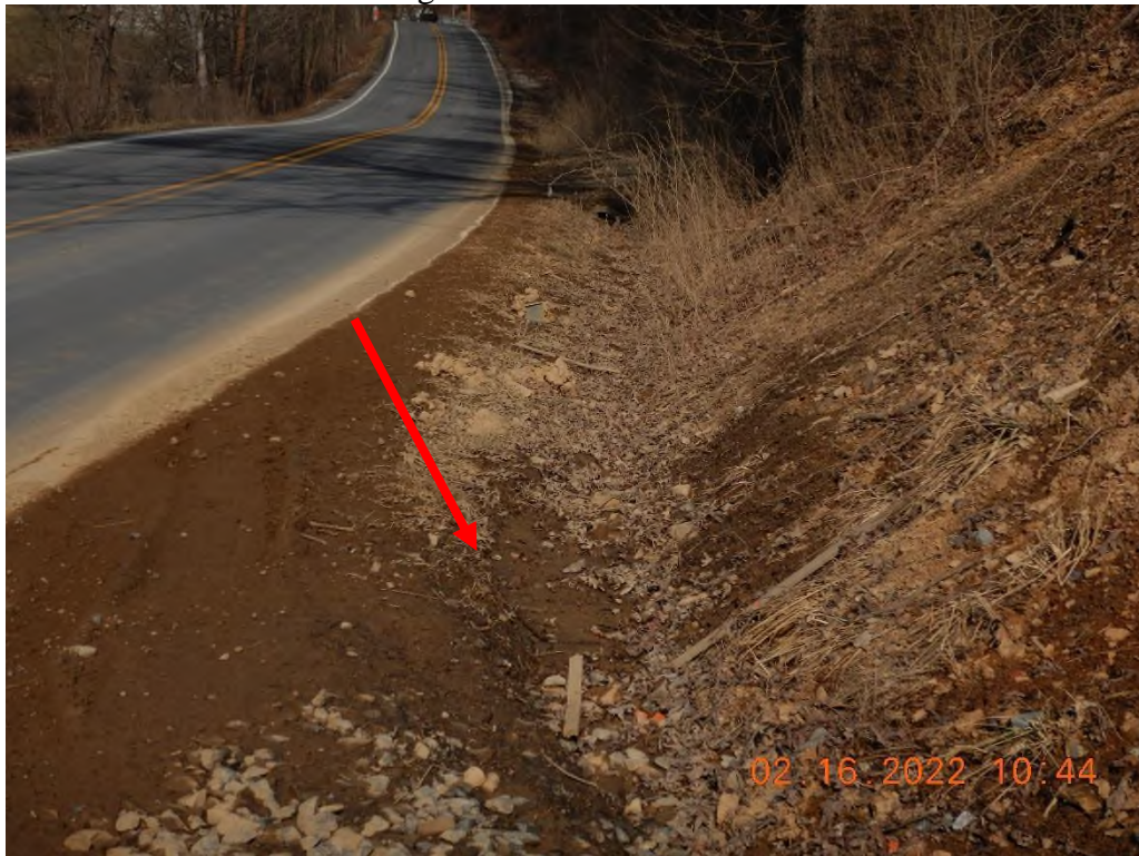
Sediment deposits in the adjacent ditch line.
