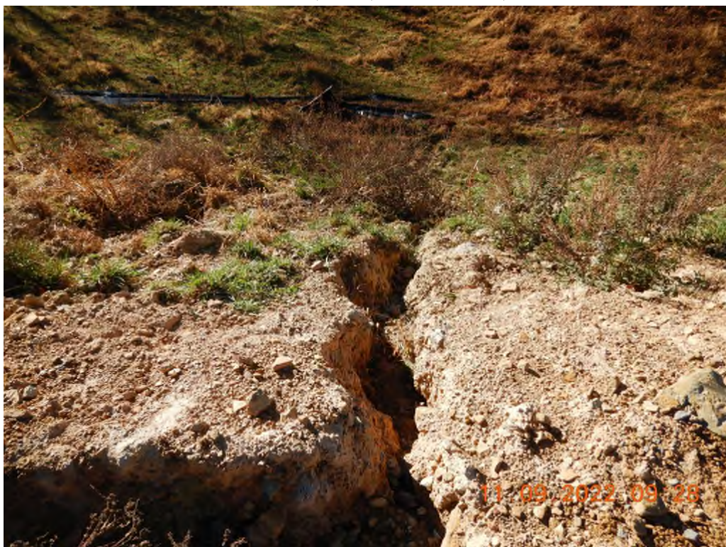
An erosion gully in the waste area, due to concentrated flow across a non-stabilized area.
