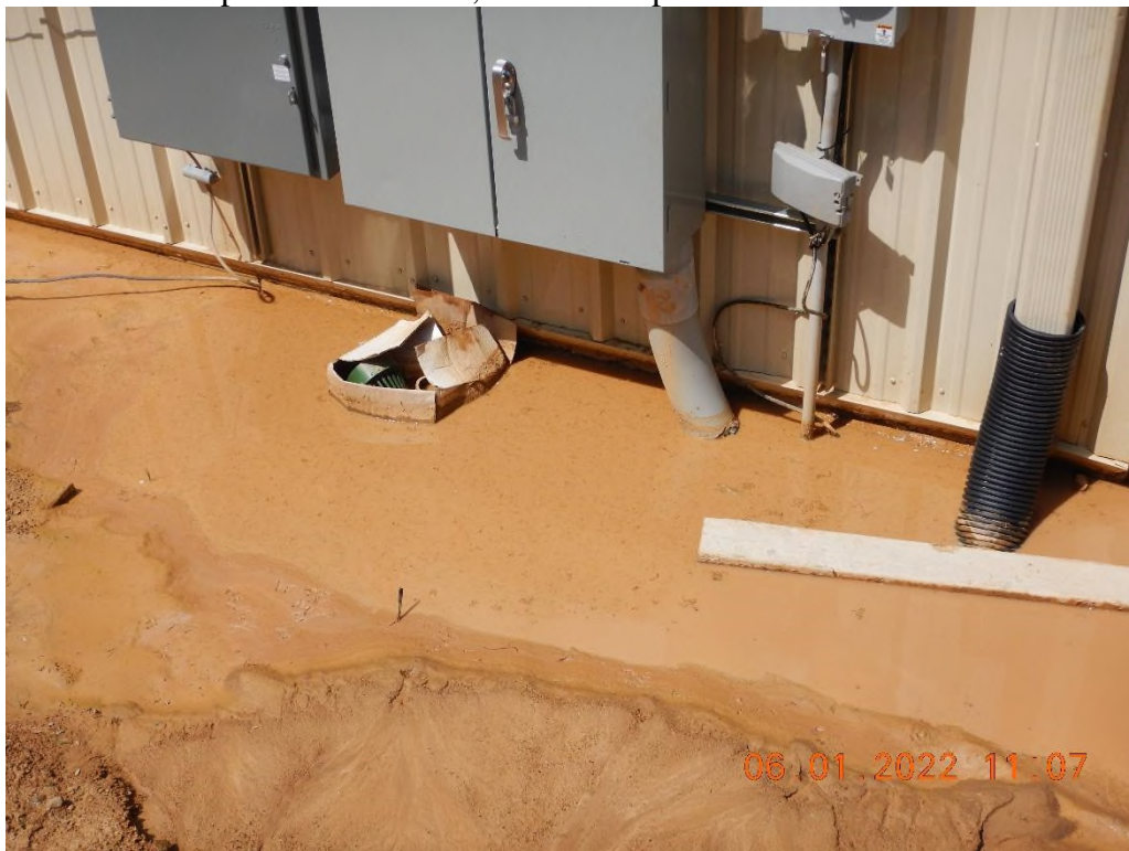
Sediment laden water that has started to pool against the building.
