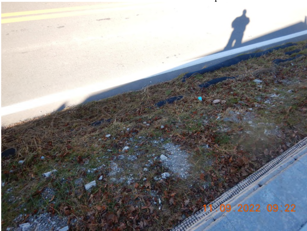
Compost filter sock lacking the required staking.
