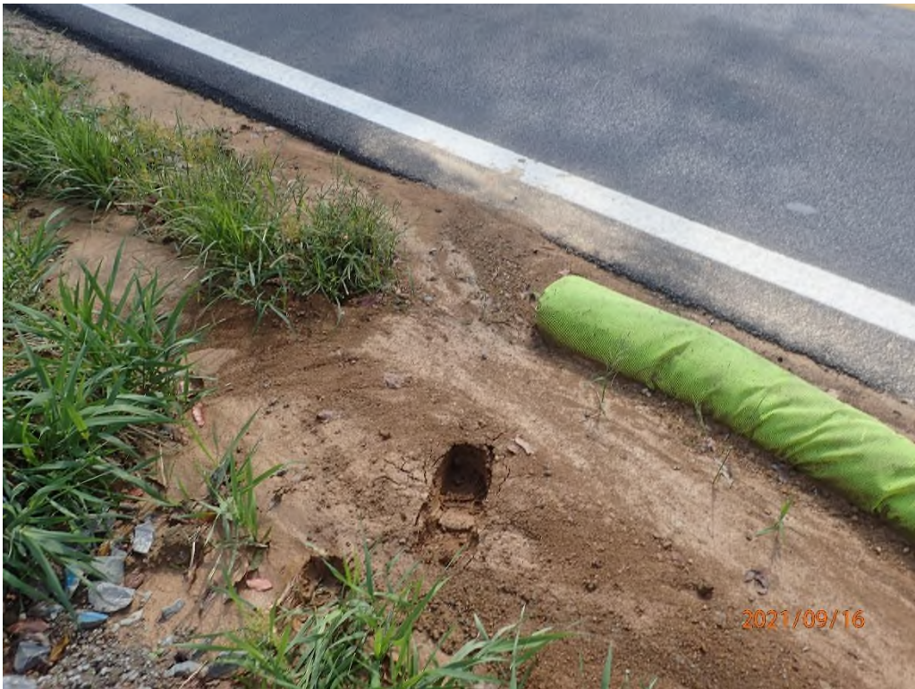
Photo 2: Sediment traveling along the road, toward an inlet that discharges into Little Tenmile Creek.
