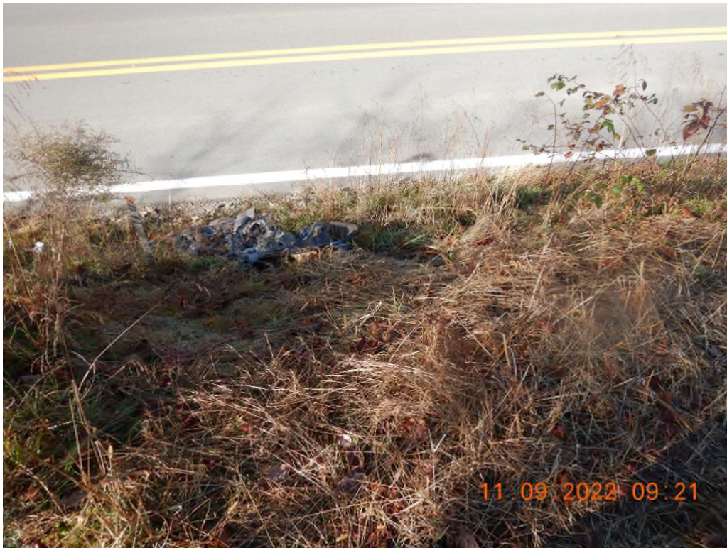
No outlet marker for Sediment Trap 2.
