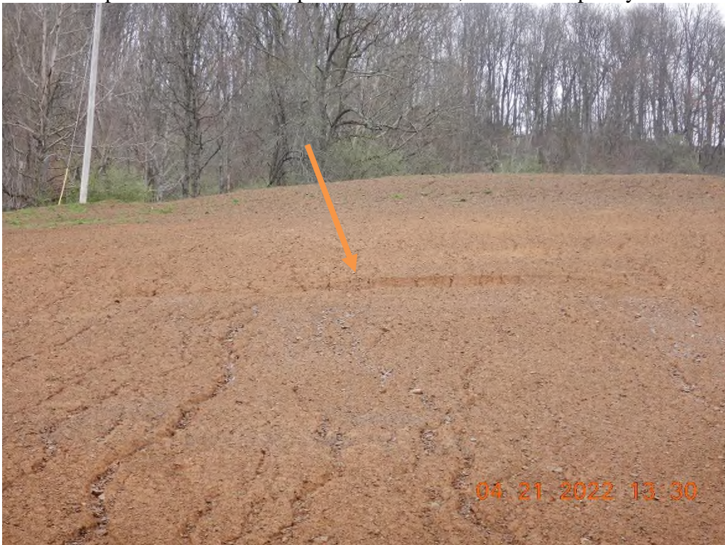
Sloughing on the earthen slip area on the eastern portion of the site.
