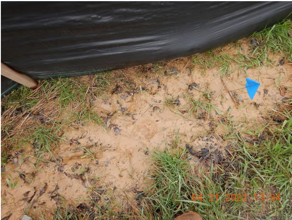
Sediment deposits behind the installed control, indicating a bypass.
