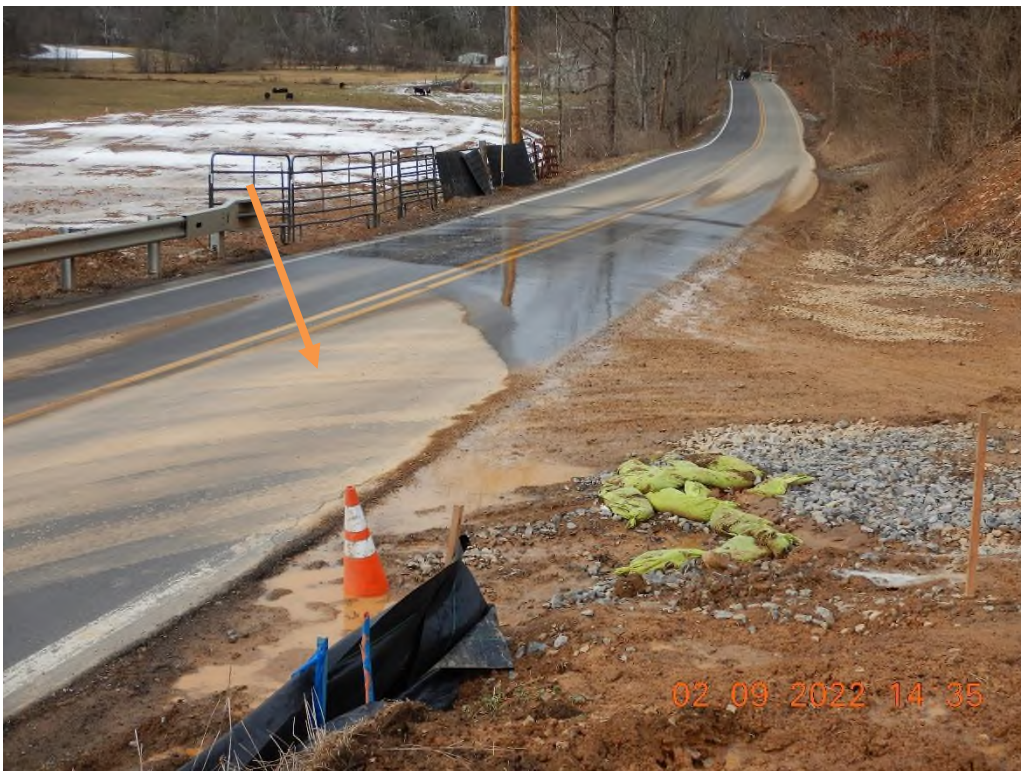
Track-out on WV-20, as a result of a non-stabilized construction entrance.
