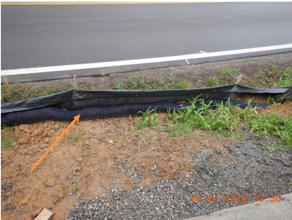
Compost filter sock that lacks the required staking.
